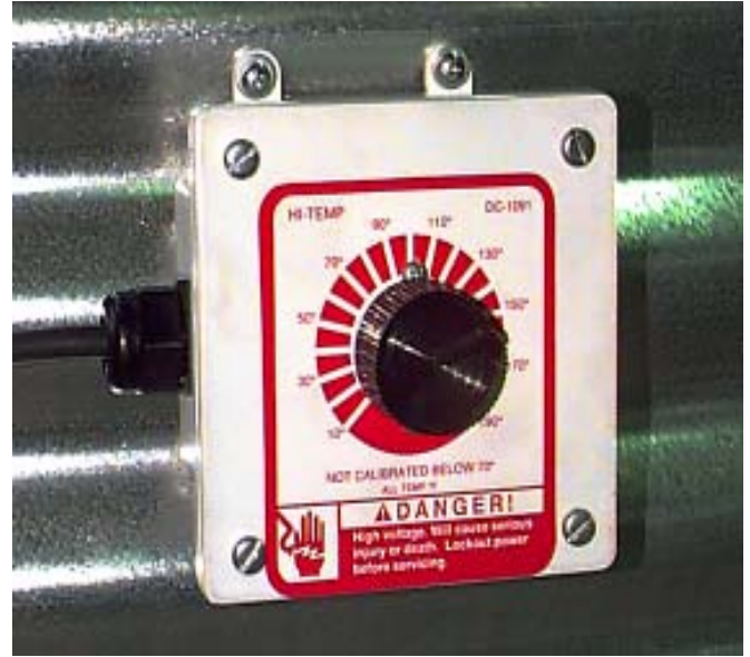
Plenum thermostat mounting on bin wall.
