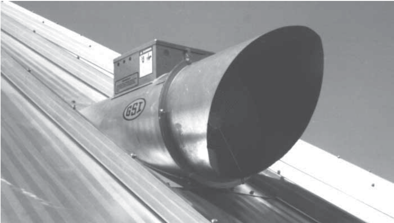
An 18" roof exhaust fan.
