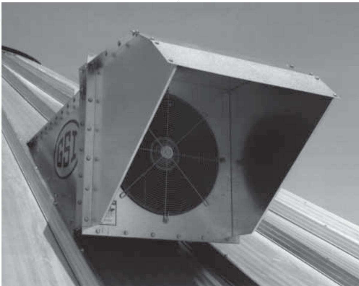
24" roof fan exhauster with the rainhood in place.
