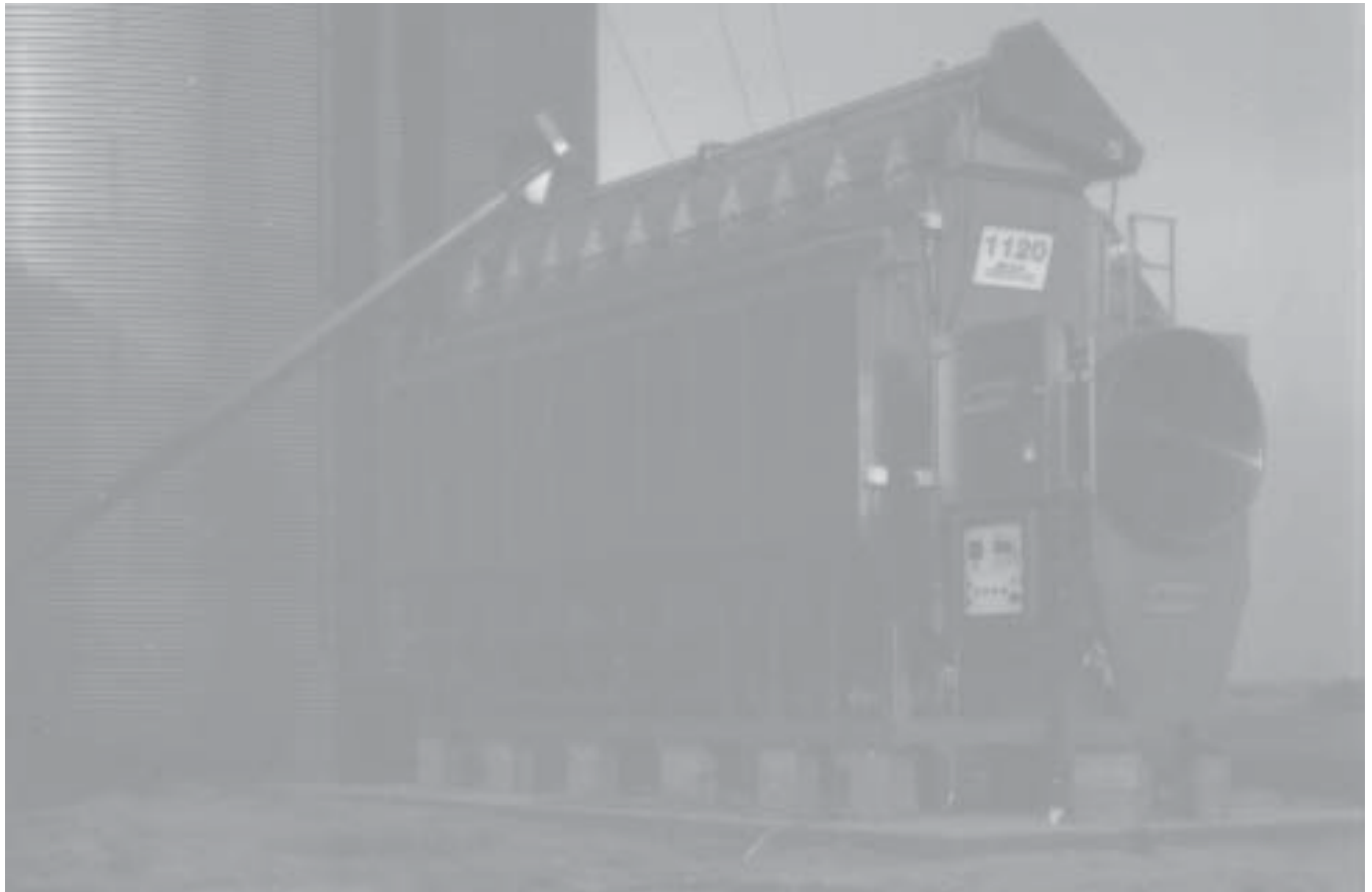
An installation using block support and cable tie-downs on a concrete slab foundation.
