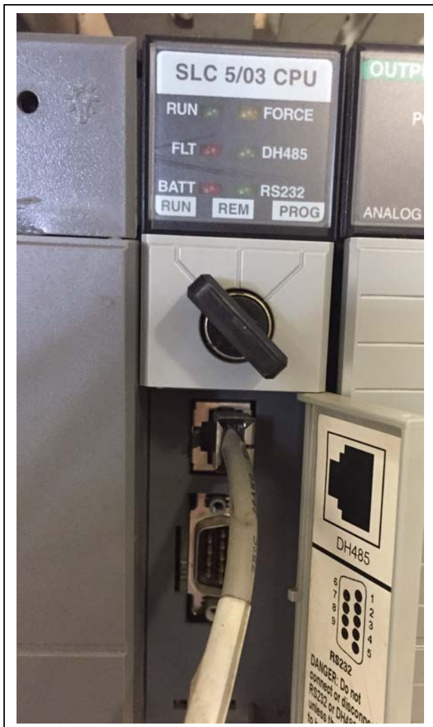
Figure 3 SLC 5/03 RJ45 Connection
