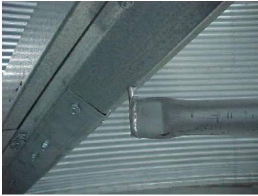
FIGURE 20. BRACE ROD PIN ASSEMBLED INTO BACK BRACE
