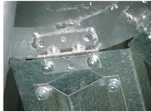
FIGURE 18. HINGE AND FLANGE NUTS
