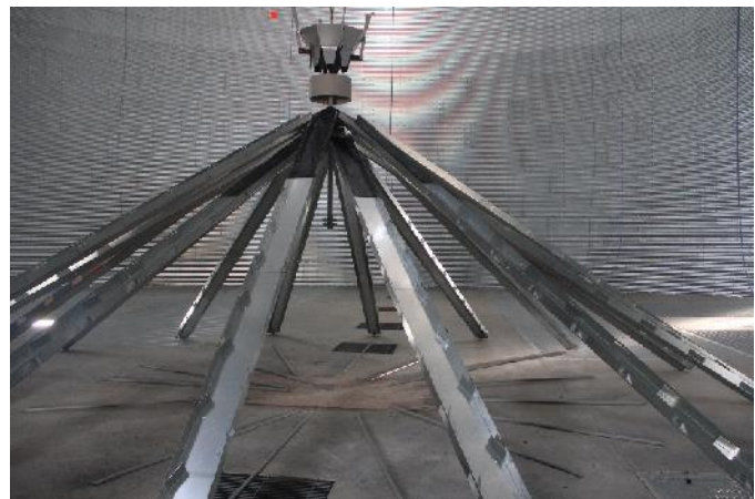
FIGURE 31. BOTTOM CHUTES ASSEMBLED BETWEEN TOP CHUTES
