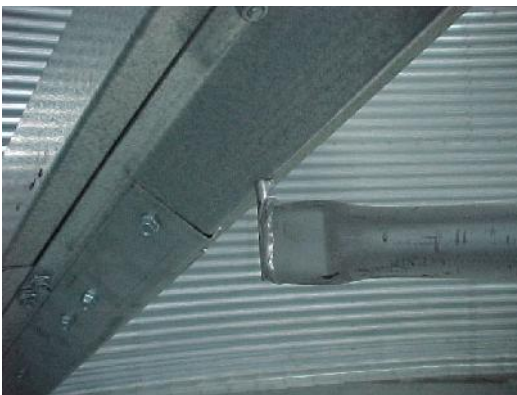
FIGURE 33. BRACE ROD PIN ASSEMBLED INTO BACK BRACE
