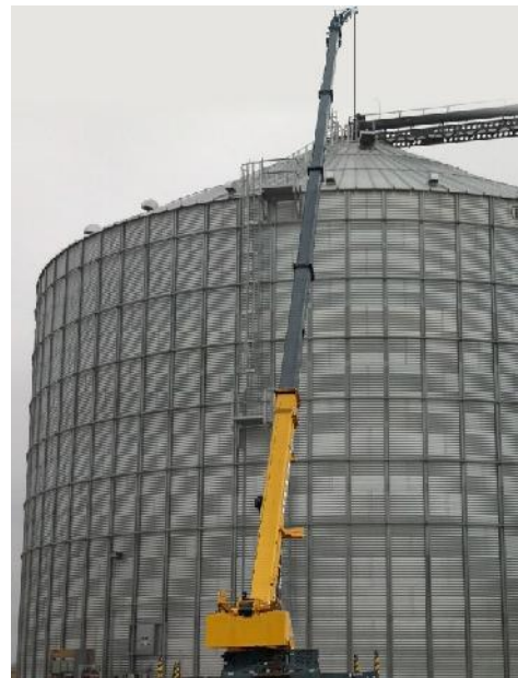
FIGURE 3. CRANE LIFT FOR COMMERCIAL SPREADER
