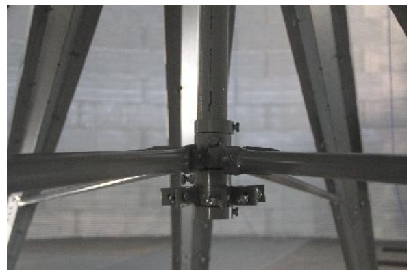
FIGURE 34. TOP BRACE RODS ASSEMBLED ON TOP SPIDER
