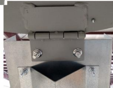
FIGURE 30. HINGE AND FLANGE NUTS
