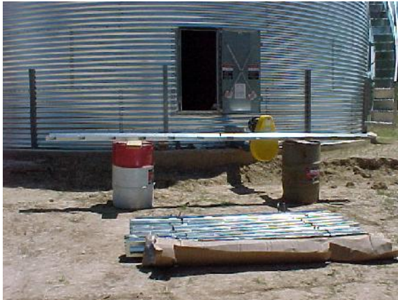
FIGURE 10. TOP AND BOTTOM CHUTE SUPPORTED OFF THE GROUND
