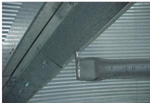
FIGURE 25. BRACE ROD PIN ASSEMBLED INTO BACK BRACE
