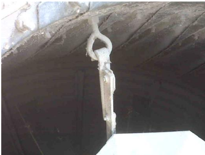
FIGURE 45. SPREADER HANGING FROM EYEBOLTS
