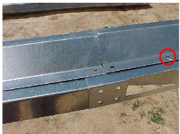
FIGURE 13. PRE-PUNCHED HOLES FULLY ALIGNED
