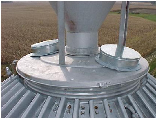
FIGURE 47. INSPECTION HOLES ON FARM BIN 180° FROM EACH OTHER
