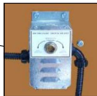
**IMPORTANT:** To adjust the air switch the grain columns need to be full of grain so that the plenum can build up air pressure and close the air switch.
