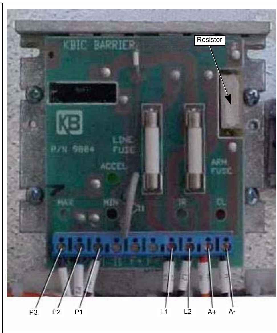
Figure 1C SCR Board Terminals
