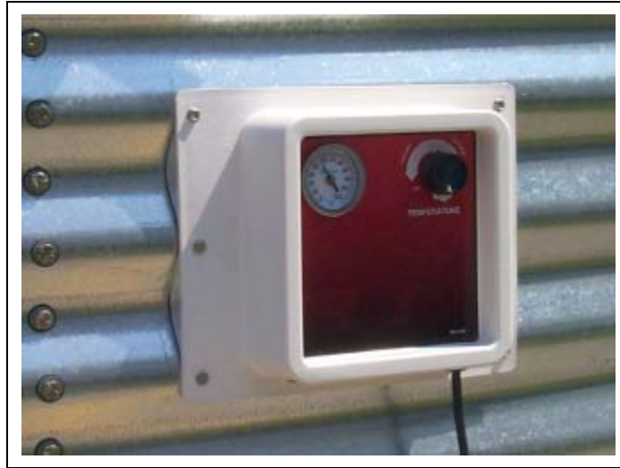
Figure 4G Plenum thermostat mounted on bin wall.
