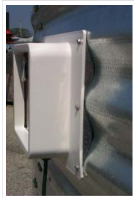
Figure 4H Side view of thermostat showing corrugation seal.
