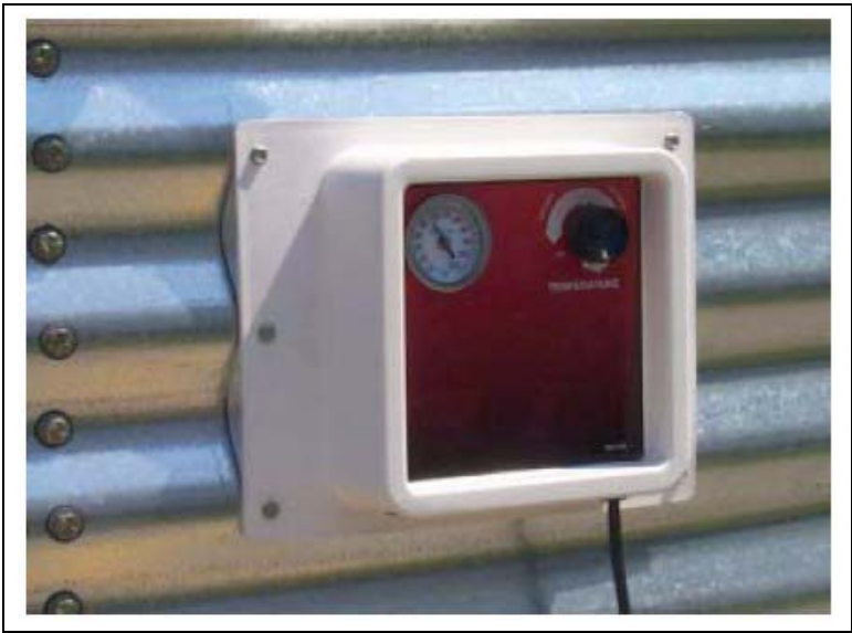
Figure 4R Fit Plenum Thermostat/High-Limit
