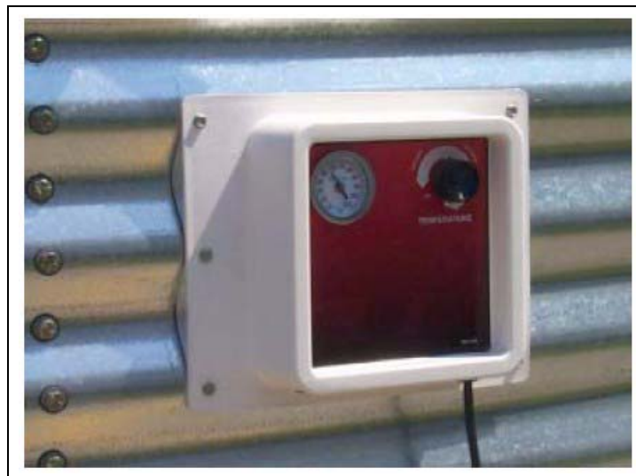
Figure 4I Fit Plenum Thermostat/High-Limit
