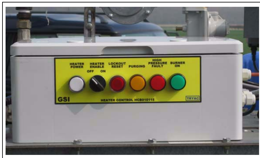
Figure 4K Heater Control Front
