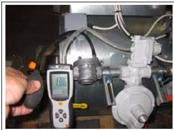
Figure 5C Pressure Test Equipment
