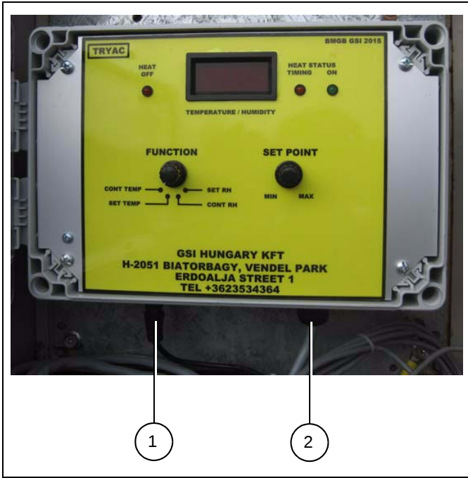
Figure 4M Modulating Control (HF-8444)
