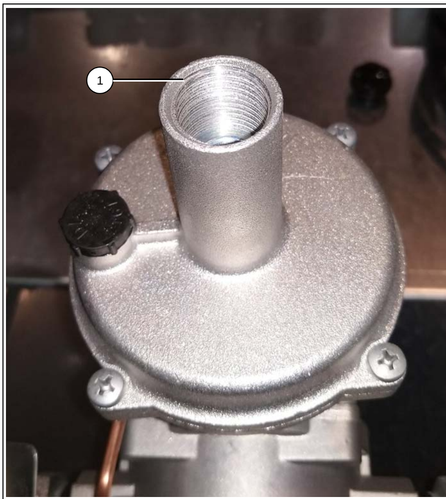
Figure 5B Over Pressure Safety Valve
