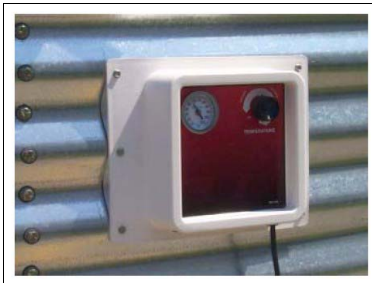
Figure 4Q Fit Plenum Thermostat/High-Limit
