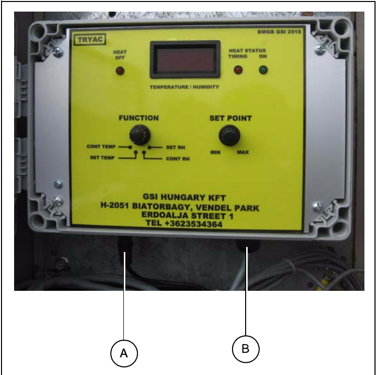
Figure 4L Modulating Control (HF-8444)
