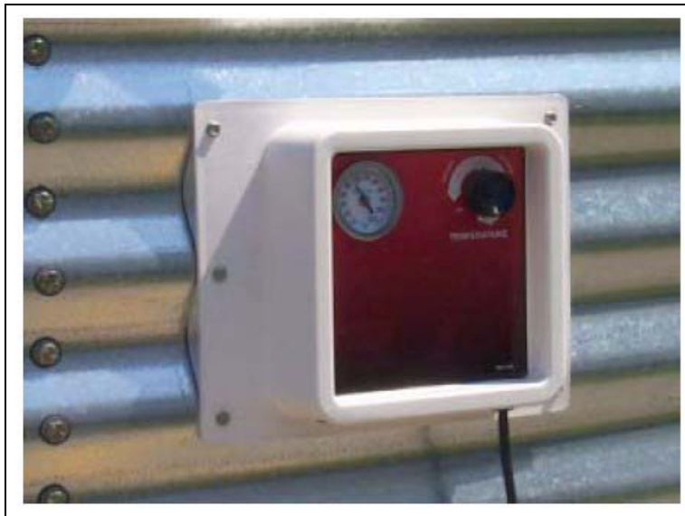
Figure 4H Fit Plenum Thermostat/High-Limit
