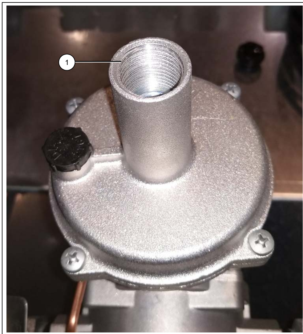
Figure 5B Over Pressure Safety Valve
