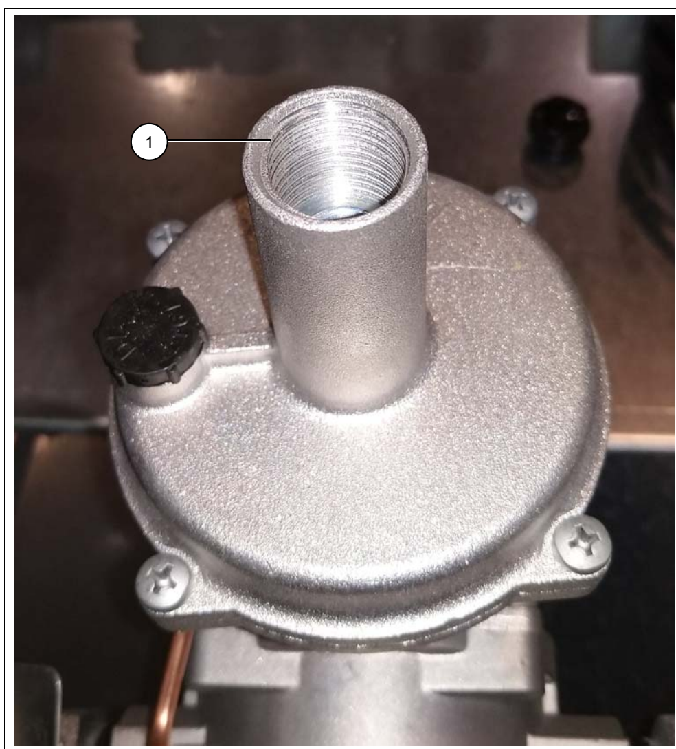
Figure 5B Over Pressure Safety Valve
