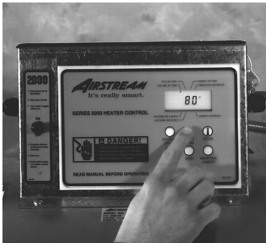
Programming the high-limit set point.
