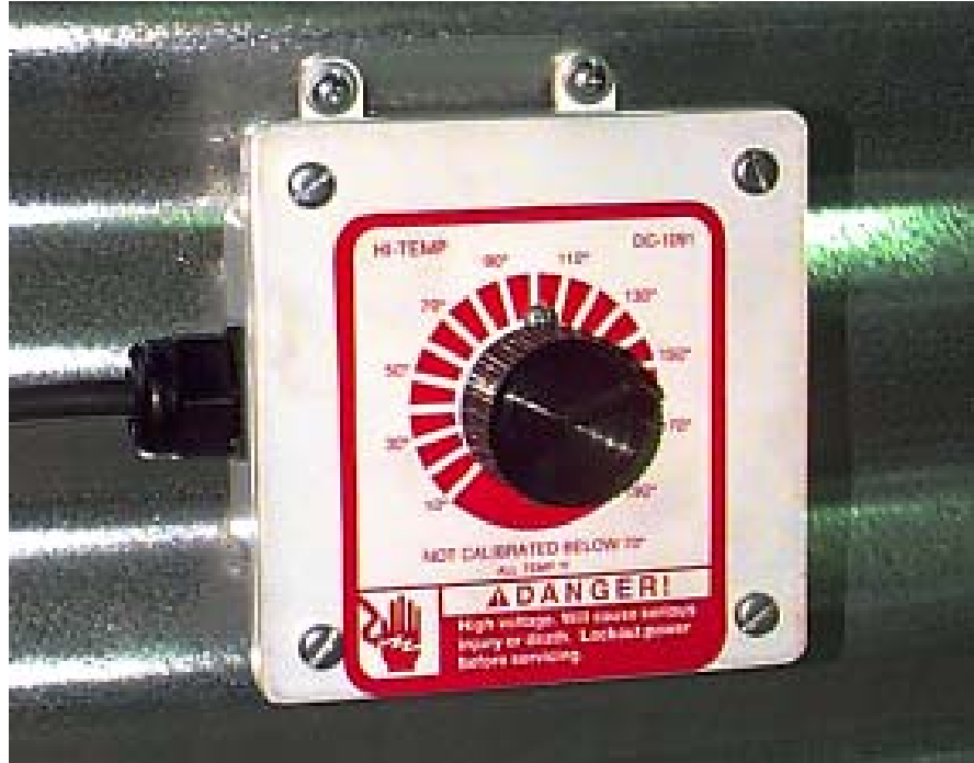
Plenum thermostat mounting on bin wall.
