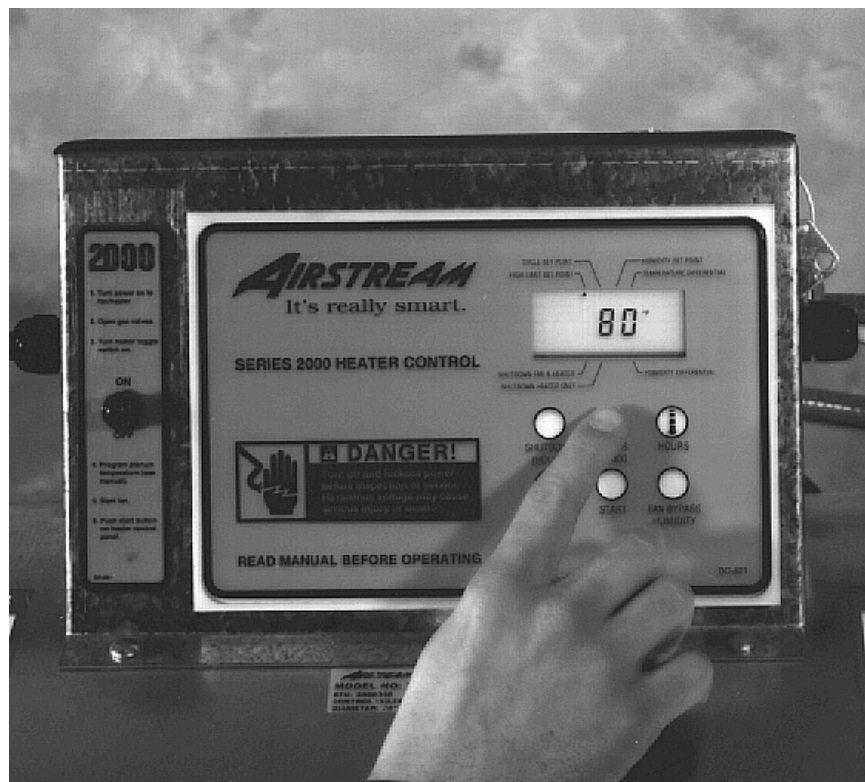
Programming the high-limit set point.
