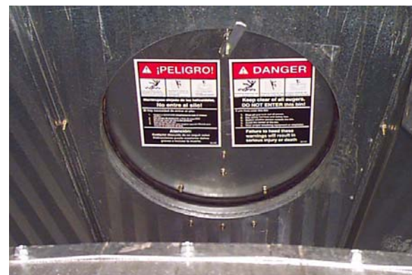
Inside view - Access port installed with decals in place.
