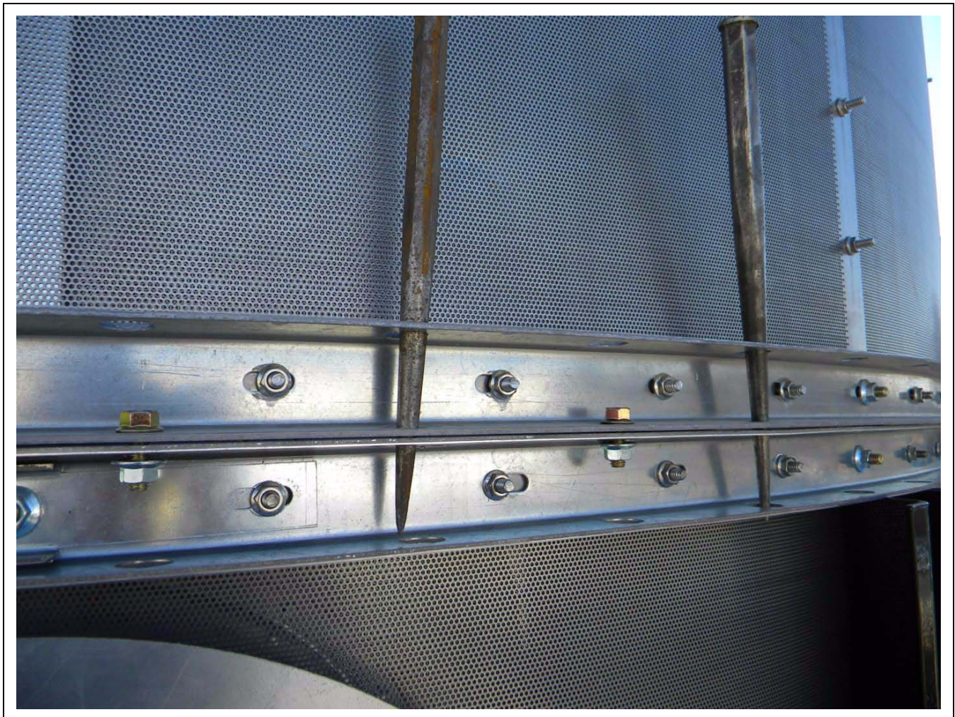
Figure 5C Line Up Punch Inserted Through Connecting Channels of Dryer
