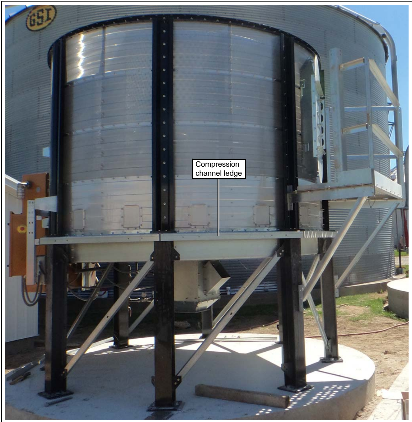
Figure 5G Unload Module with Compression Channel Marked
