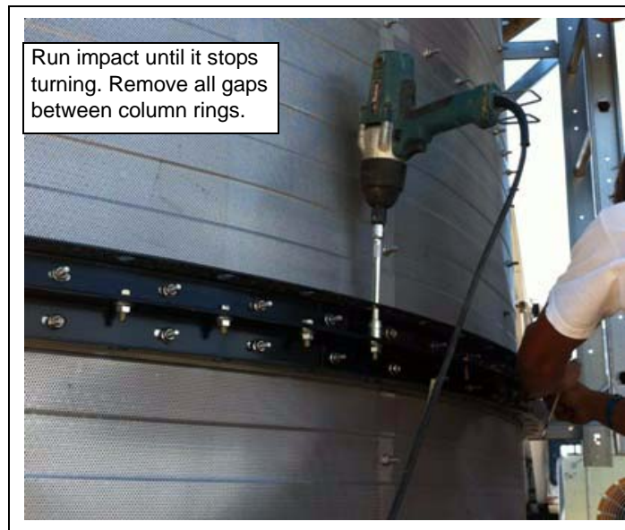
Figure 9N Connecting Dryer Sections on Outside
