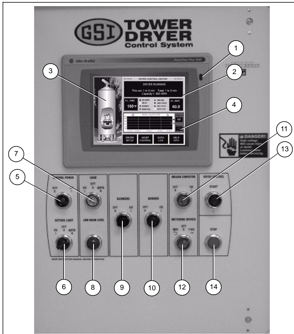
Figure 3H PLC Control Screen
