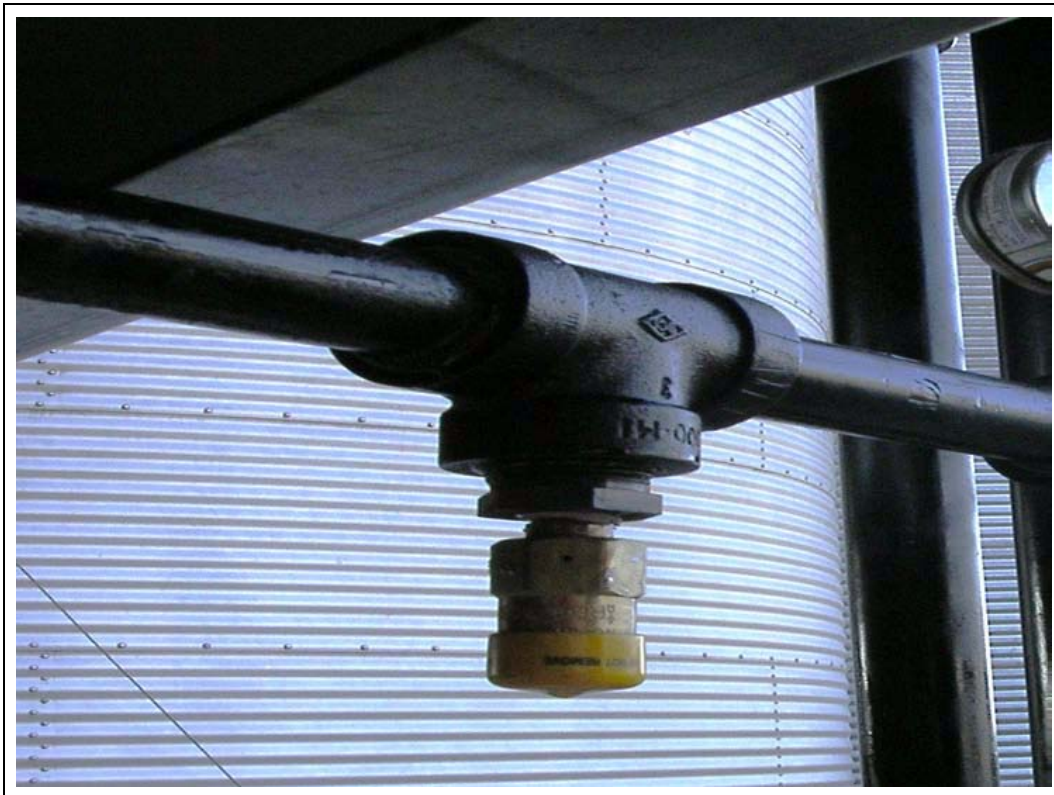
Figure 7E 3/4" Brass Pressure Relief Valve Assembly
