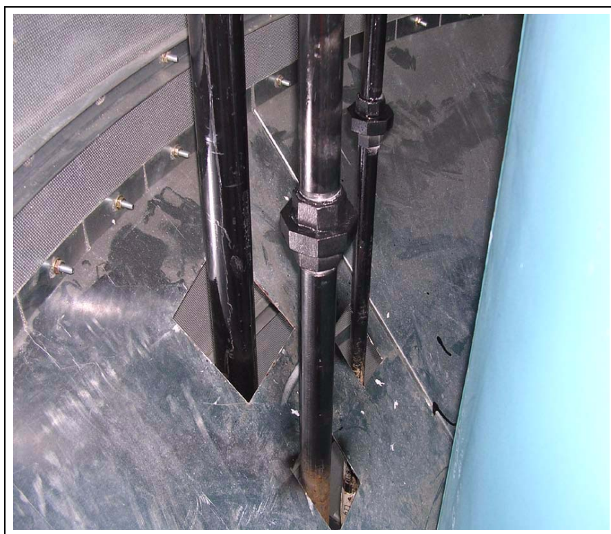
Figure 7N Piping 3/4", 1-1/4" and 2", going through the steel divider plate. Notice the use of unions for piping connections.
