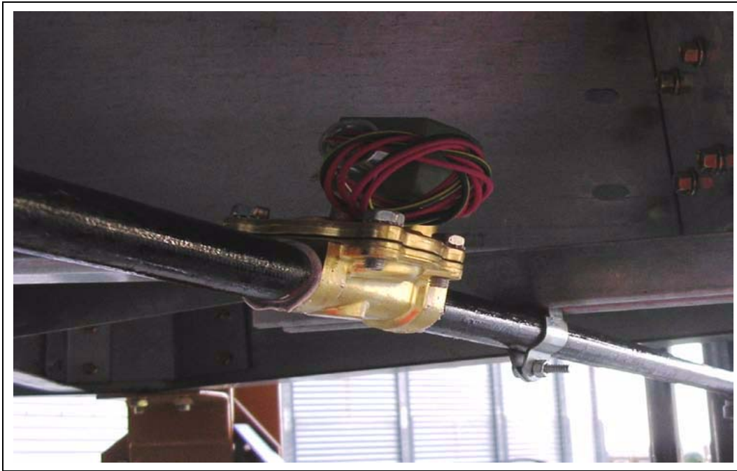
Figure 7D 3/4" ASCO Liquid Line Solenoid Valve (Normally Closed)
