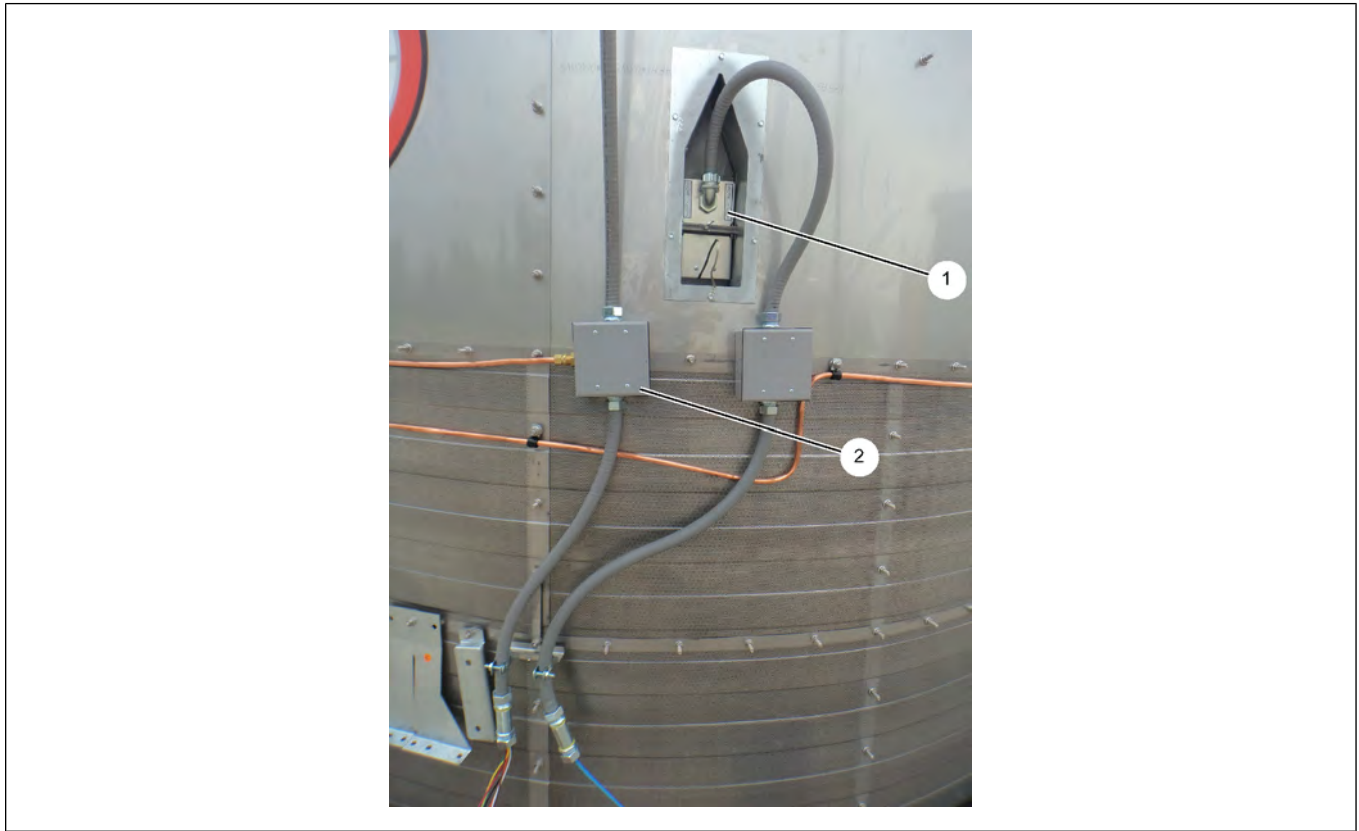
Figure 10-5 Outside Overheat Sensor (GT4-0148) and Wet Moisture Sensor (GT4-7187-2)
