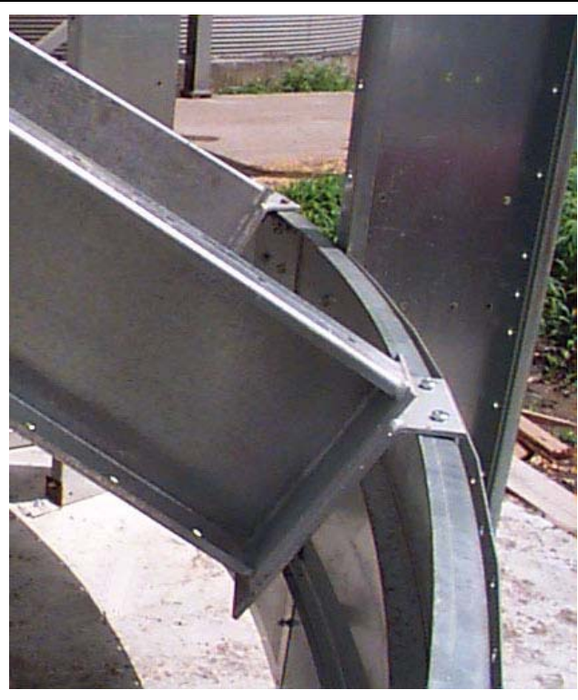
Figure 5AJ Close Up - Bolt bottom of plenum roof rafters to top of plenum roof eave channel (in pairs of bolt holes).
