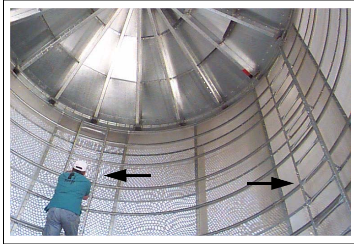
Figure 11H Auxiliary ladders installed. (2 of 4 shown.)
