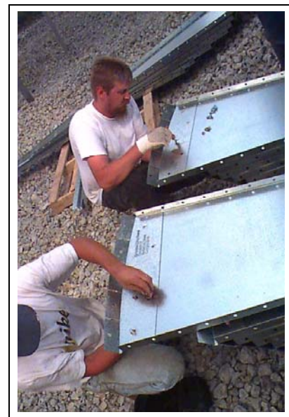
Figure 21AH Pre-assembling one (1) inside hopper flange to each inside hopper panel.
