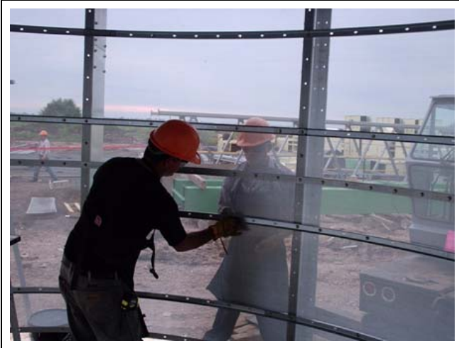
Figure 5AW Tightening inside top wall sheets. (Inspect all when completed. Access is restricted after this point.)
