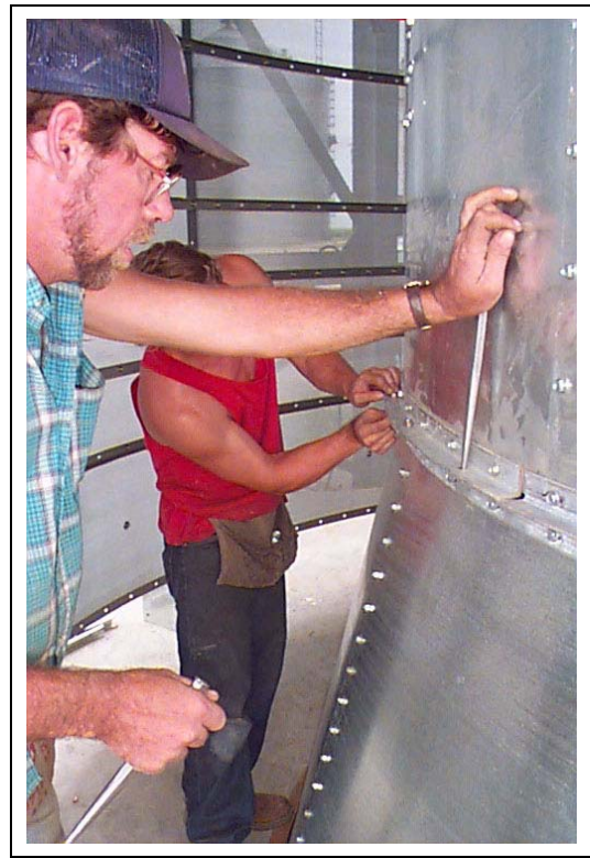
Figure 14AB Aligning and bolting reducer to burner housing.
