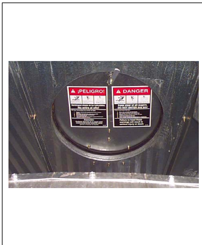
Figure 6AL Inside View - Access Port Cover Installed
