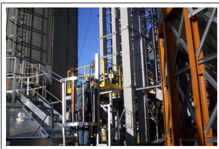
Figure 7T Trim and bolt safety hoops to platform vertical support as necessary.
