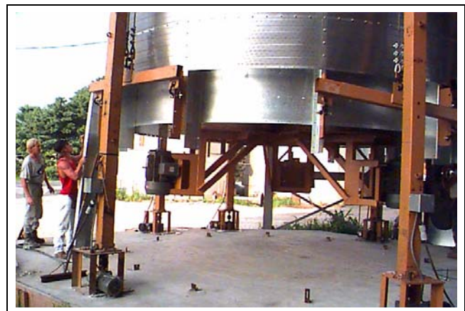
Figure 16K Fan motors installed to fan motor mounts.
