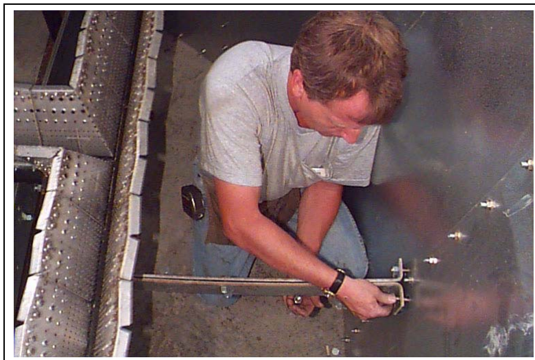
Figure 14S Installing a pair of burner support tees (back to back) to burner housing.
