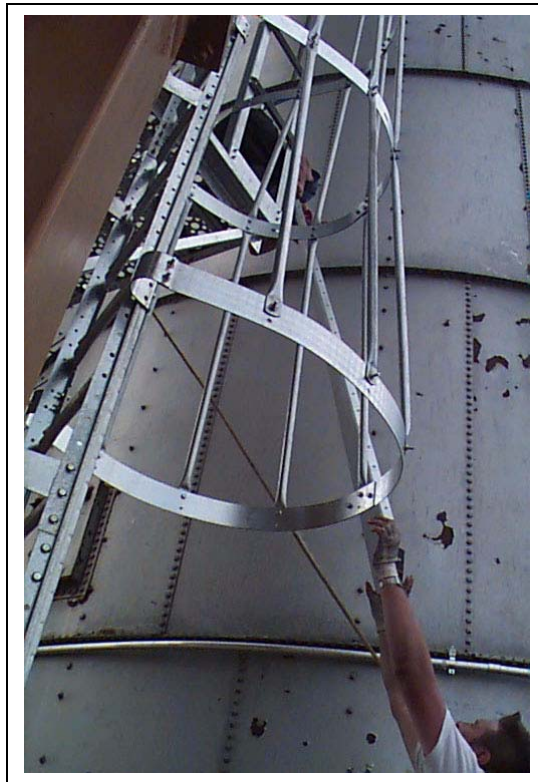
Figure 7V Bell safety cage installed.
