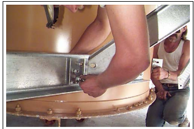
Figure 15AO Bottom of fan - Installing fan crossbeam to fan crossbeam clip.
