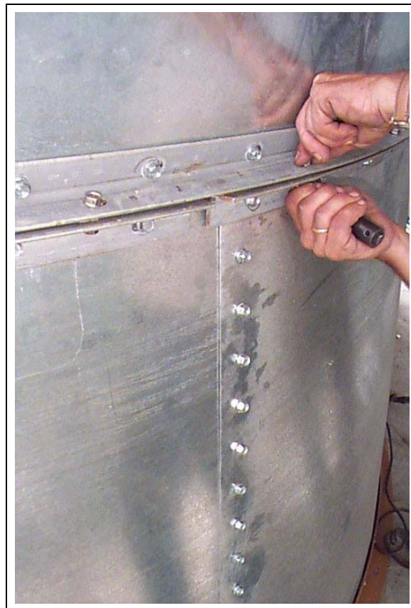
Figure 14AC Close Up - Bolting reducer to burner housing.
