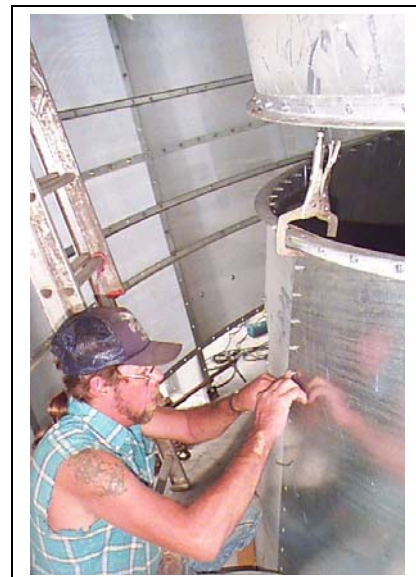
Figure 14Z Bolting halves of reducer together.
