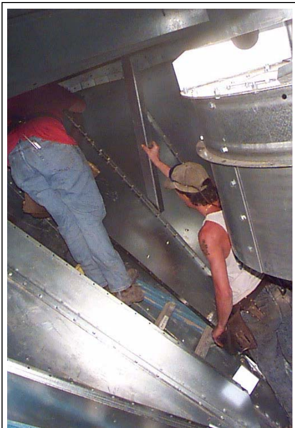
Figure 21AK Bolting cool section floor support to cool section floor beam.
