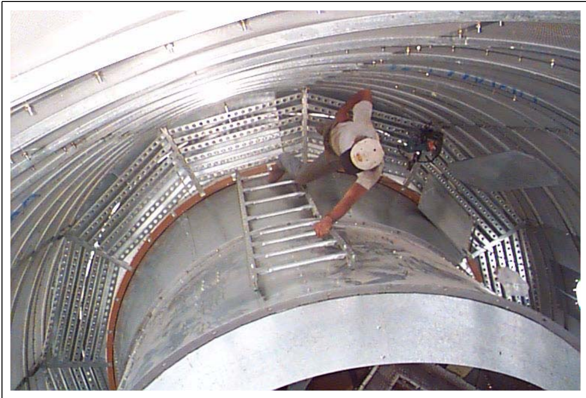
Figure 11N Installed burner housing ladder.
