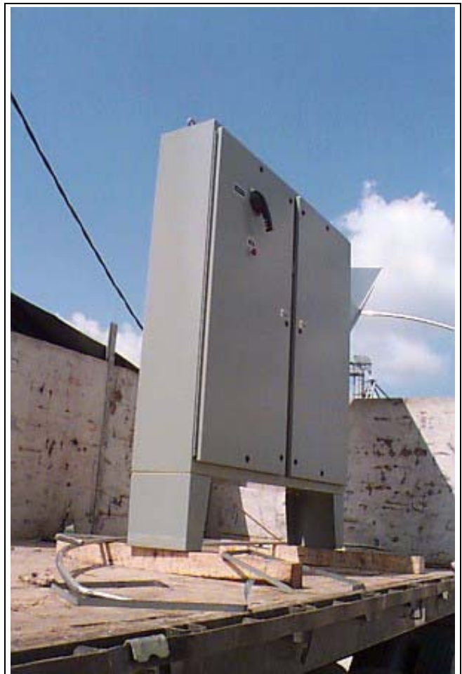
Figure 25B Electrical Control System
