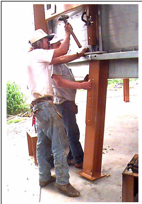
Figure 19Q Aligning upper leg to base stiffener weldment.
