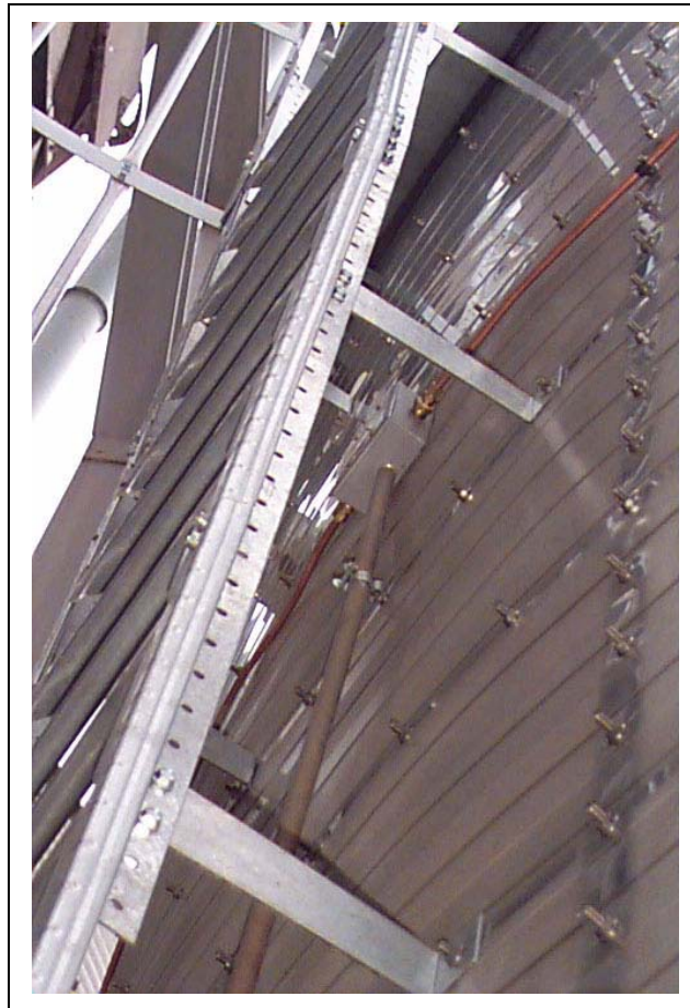
Figure 8P Close Up - Upper High-Limit installed with junction box positioned under outside ladder.
