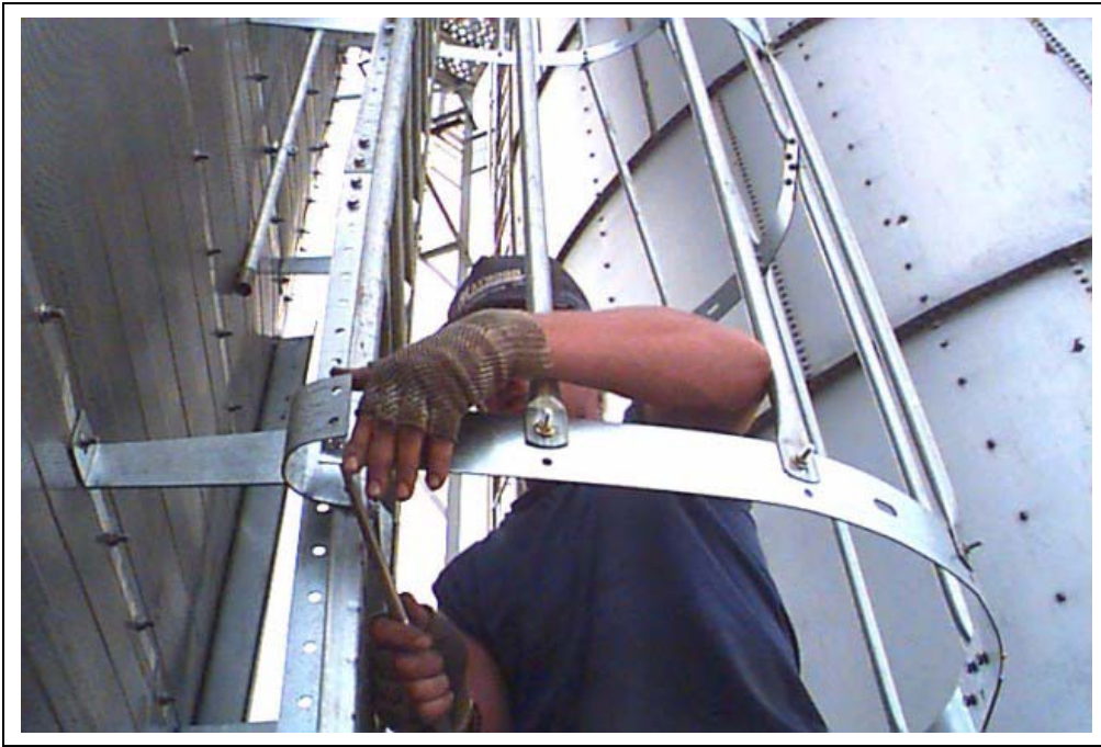
Figure 7U Close Up - Installing bell safety cage.
