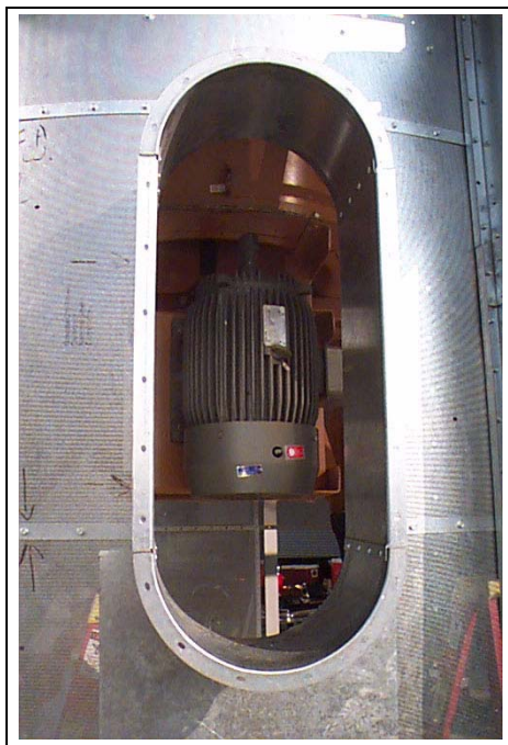
Figure 18AB Window is centered on fan motor.
