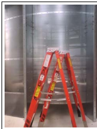
Figure 4Z Installing lift brackets to outside wall sheets of tower roof. (With 3/8" x 1" galvanized bolts and nuts.)
