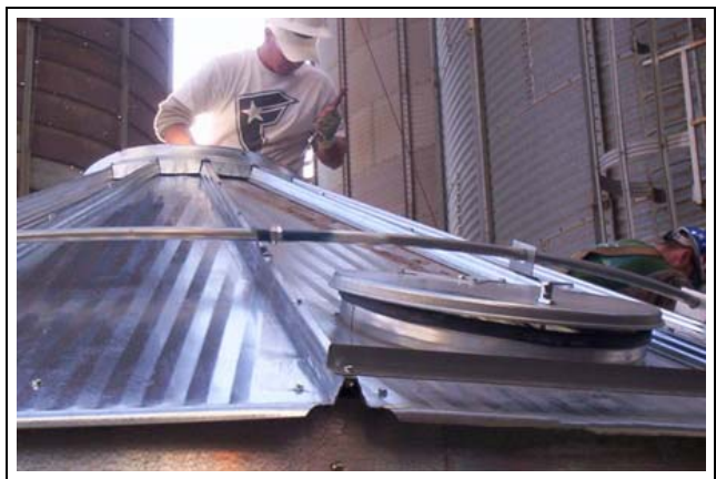
Figure 6AF Tightening center collar flashing bolts.
