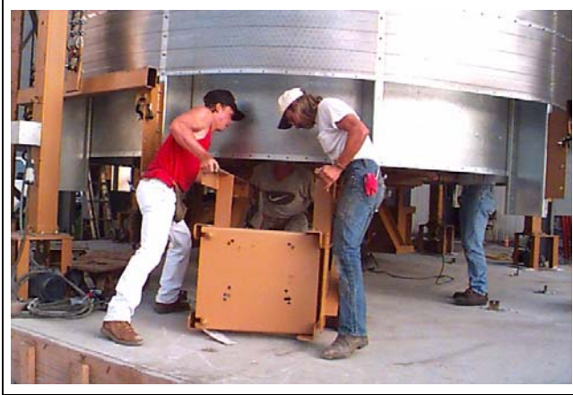
Figure 16C Moving fan motor mount under fan.
