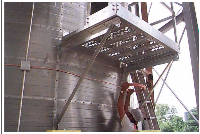
Figure 8S Installing lower High-Limit.
