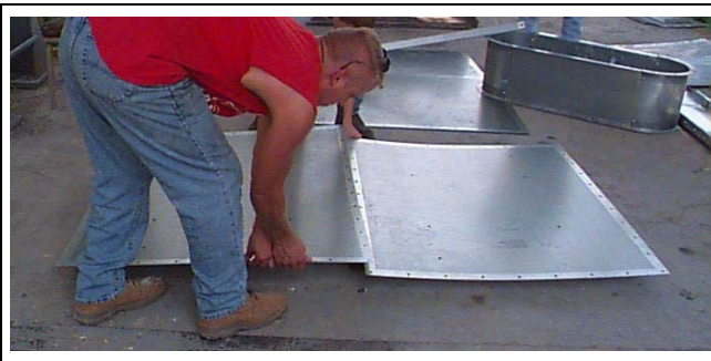
Figure 18H Align bolt holes in the two (2) wall sheets.
