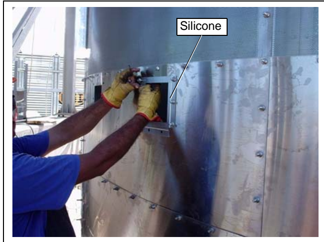
Figure 12B Installing slide gate plate to frame on outside bottom wall sheet and mid way sheet. (For emergency discharge and cleaning.)
