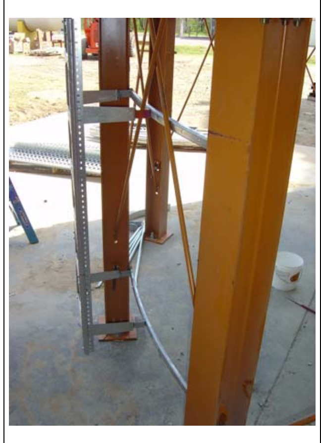
Figure 19AM X-Bracing rods installed.
