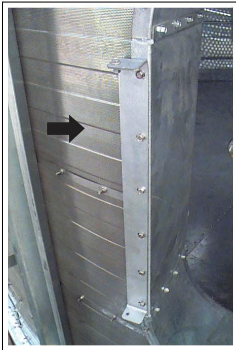
Figure 18AG Use common bolts on latch/hinge bracket, window frame, and outside wall sheets (arrow). Insert bolts toward inside of dryer.
