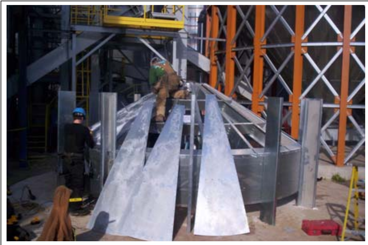
Figure 5AR Aligning Plenum Roof Sheets
