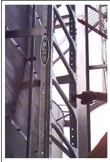
Figure 7L Close Up - Pointing to ladder stiffener splice. Install ladder stiffener splice with 4 bolts (circle).
