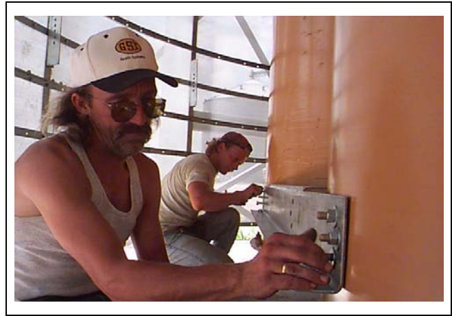
Figure 15AI Installing bottom intermediate fan support beam across two (2) fans.
