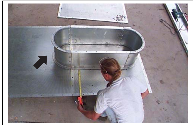
Figure 18K See Orientation Section on Page 19 for assembly layout for placement of window frame on wall sheets. Leave room below window frame (arrow) for air deflector.
