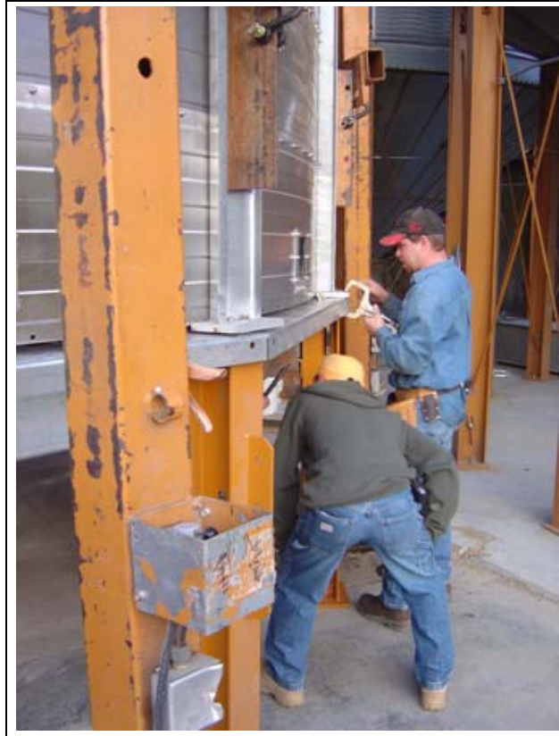
Figure 19N Compression angle weldments encircle base of dryer.
