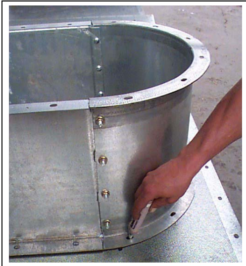
Figure 18M Close Up - Mark window frame bolt holes.
