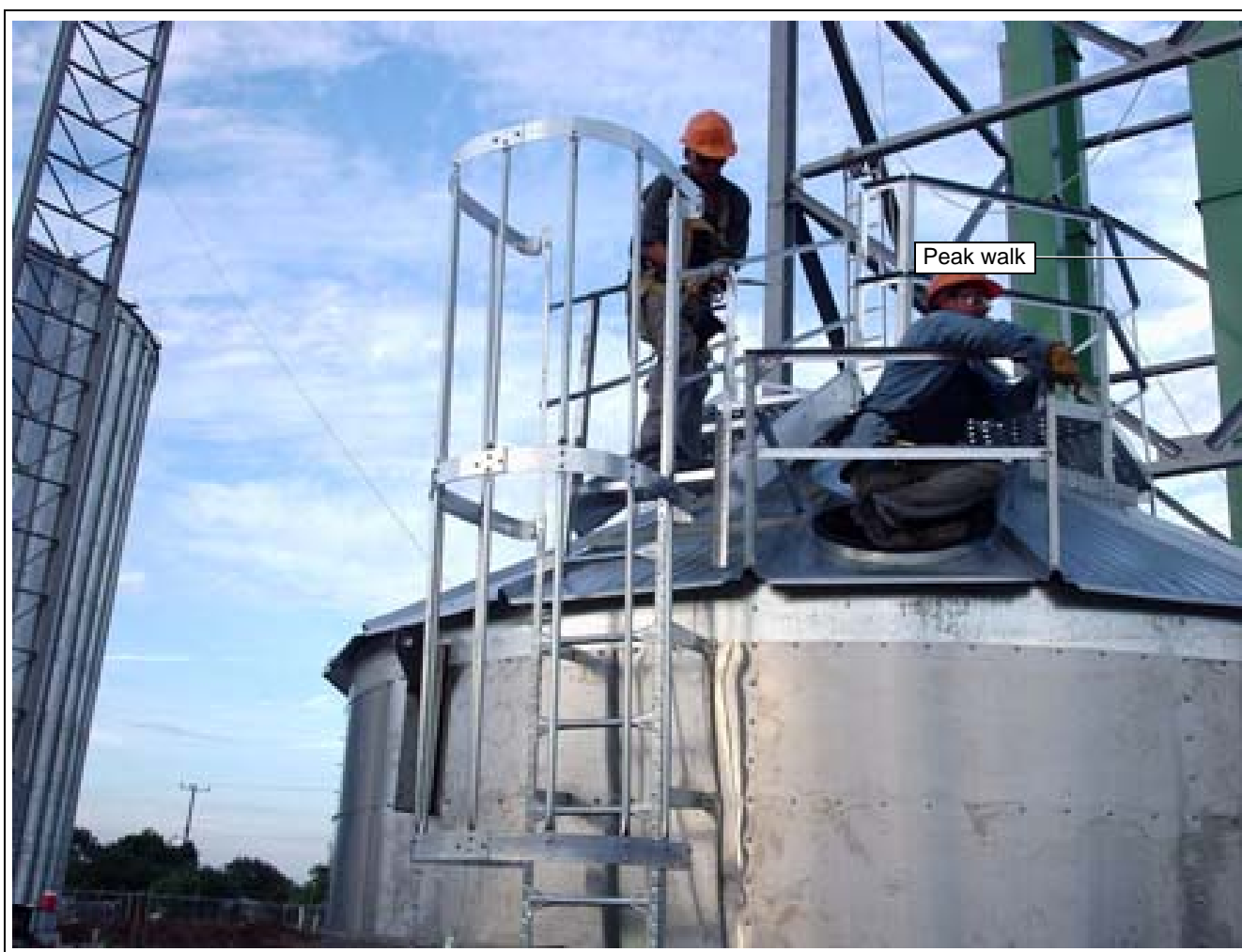
Figure 7K Installing top safety railing and peak walk to tower roof.
