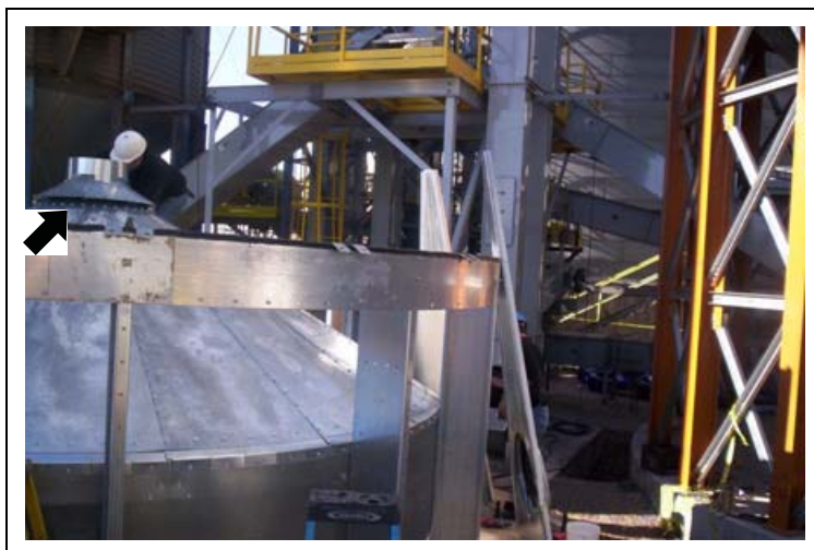
Figure 6G Pressing bulb seal over top of roof band.
