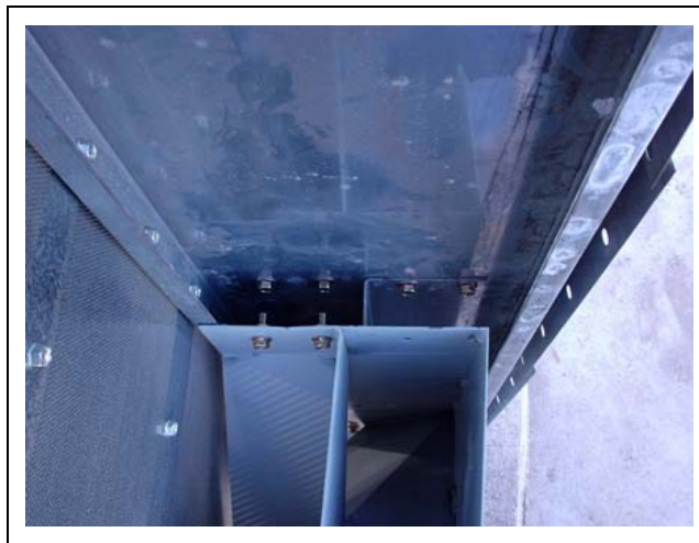
Figure 13C Installing outside grain turner sections.
