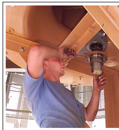
Figure 16T Tightening set screw on fan hub.
