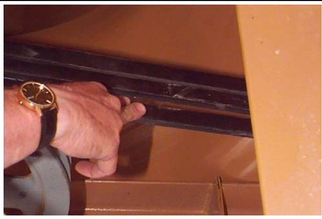
Figure 16AB Checking fan belt tension. Can press down about one fan belt width.
