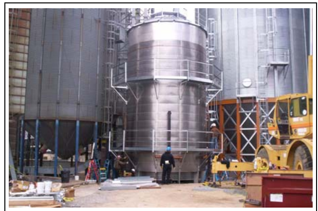
Figure 10Z Completed Outside Catwalks
