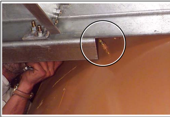
Figure 17F Grease zerk on fan (circled).
