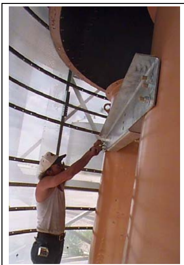
Figure 15AH Installing top intermediate fan support beam across two (2) fans.
