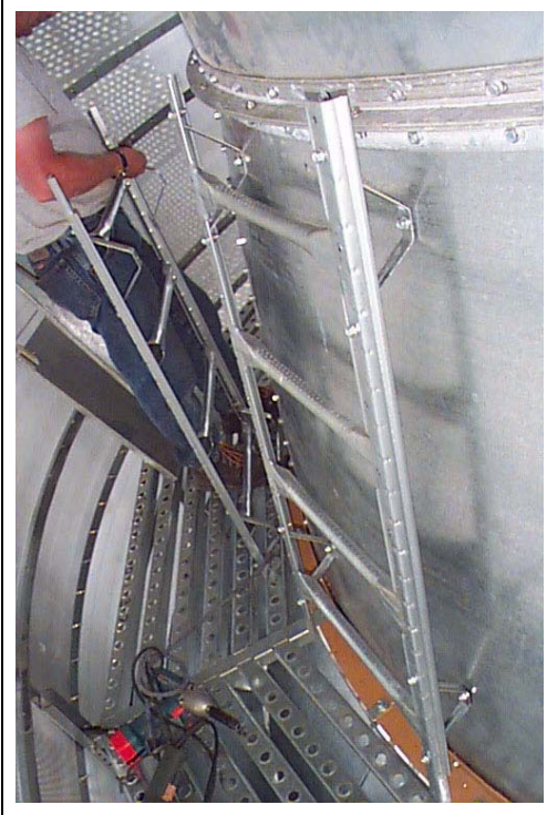
Figure 11L First 44" formed ladder section installed to reducer housing.
