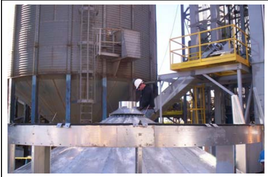
Figure 6I Installing bulb seal, eave clips, and intermediate eave clips to roof band.
