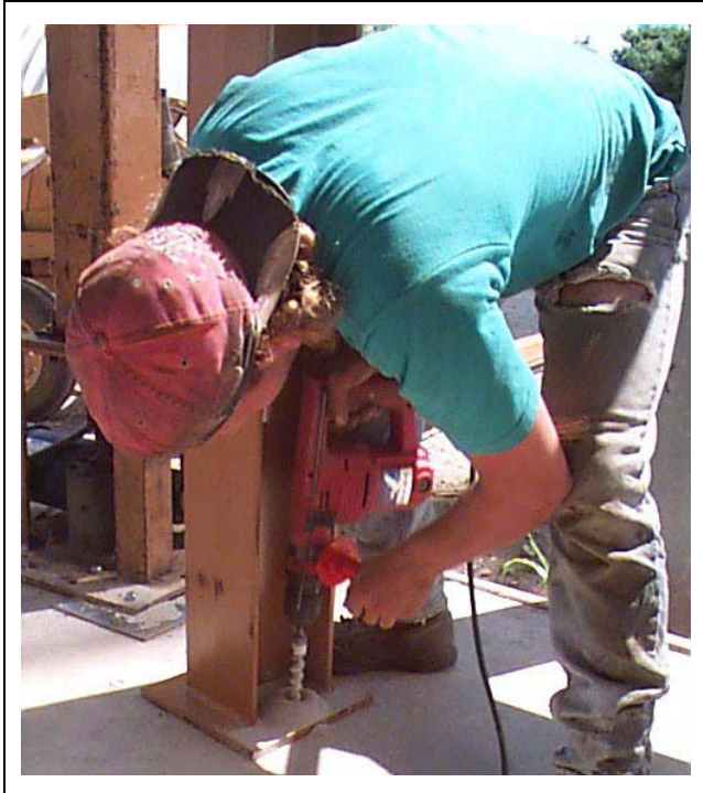
Figure 19AE Drill proper size hole.
