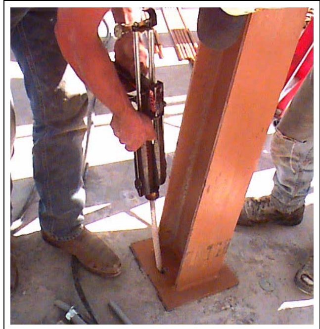
Figure 19AG Fill hole with ceramic epoxy.
