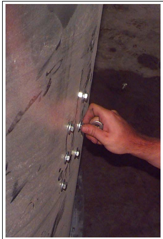
Figure 14O View outside burner housing - Installing burner mounting bracket with washers.
