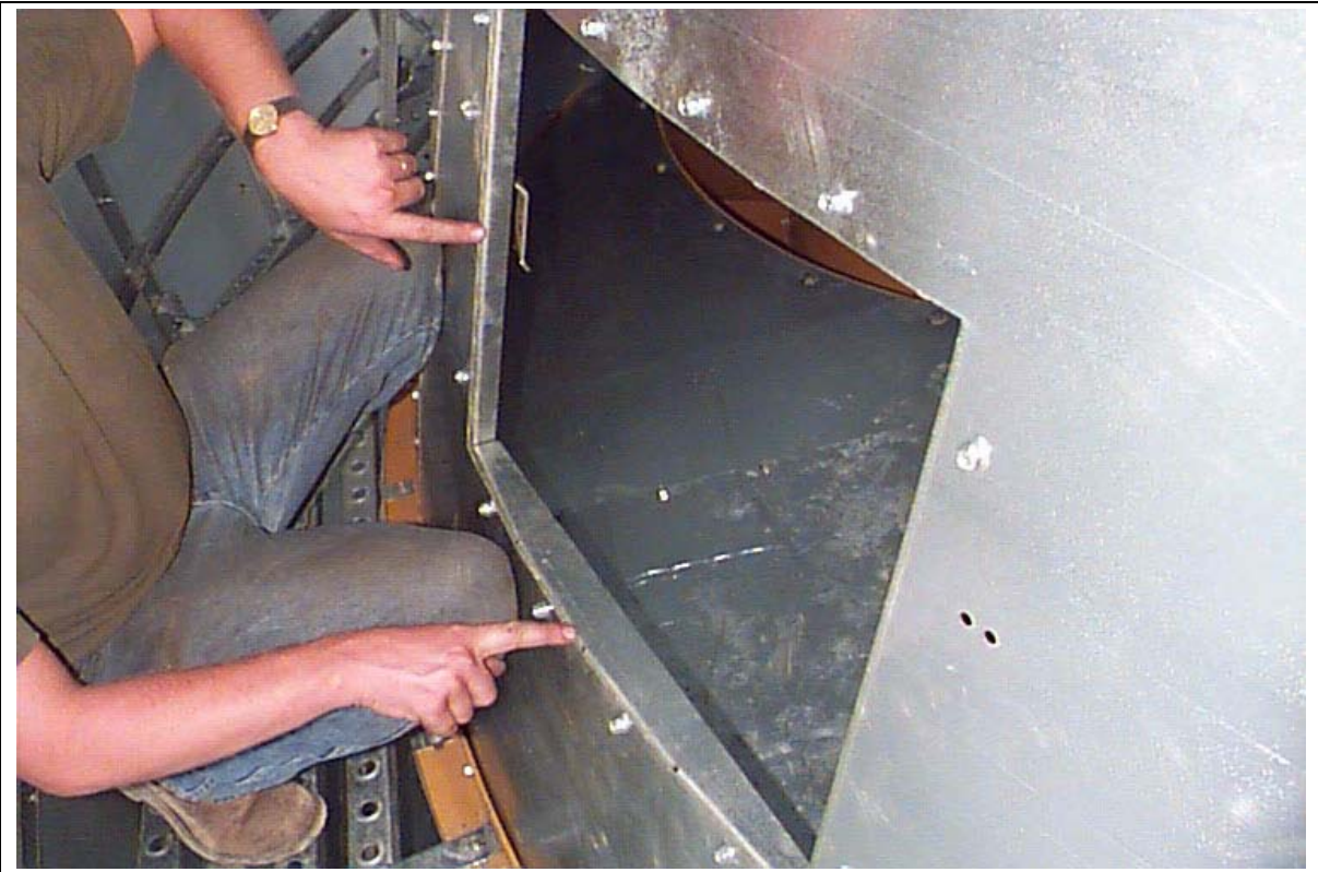
Figure 18BB Front of installed reducer door.
