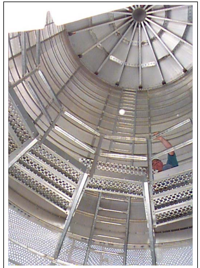
Figure 10AK View from below - Inside Catwalk installed. (Inside catwalk door is open.)
