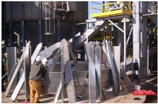
Figure 5AG Bring first pair of plenum roof rafters together to plenum roof center collar in center of dryer
