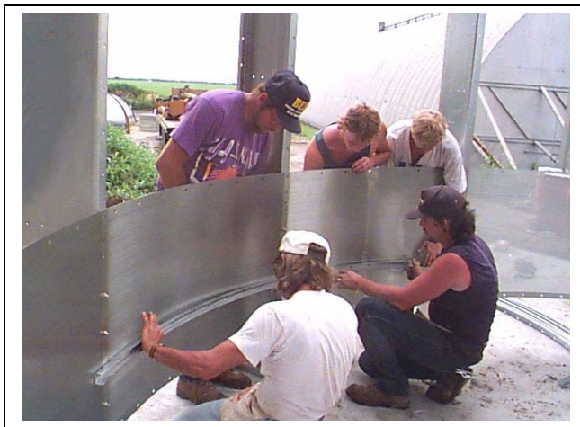
Figure 5S Installing rolled plenum channel to inside top wall sheets.
