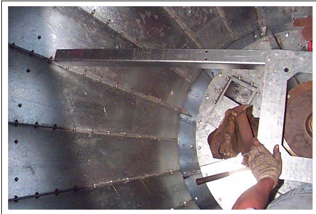
Figure 22Q Gearbox torque arm assembly installed to inside hopper wall.
