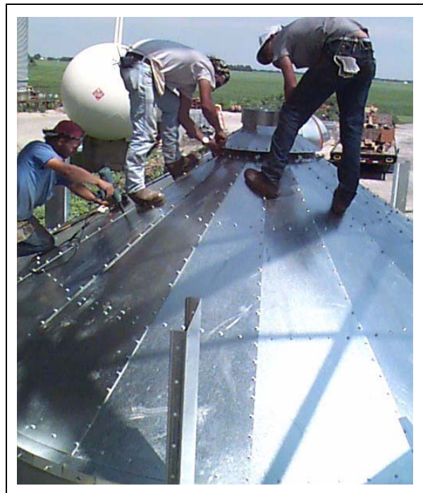
Figure 5AU Installing peak cap to plenum roof sheets.
