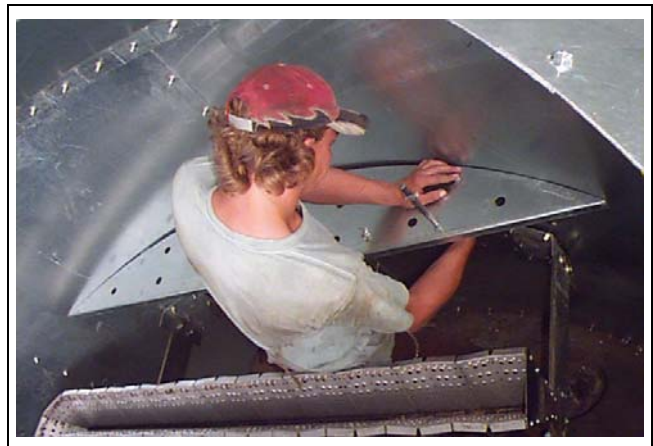
Figure 14V Installing burner baffles.
