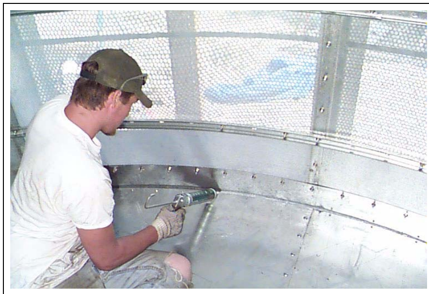
Figure 20C Caulking outside edge of hopper.
