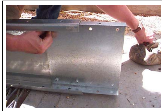
Figure 9C Splicing vertical channels.
