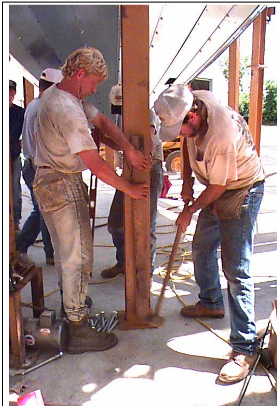
Figure 19X Tapping dryer legs into position.
