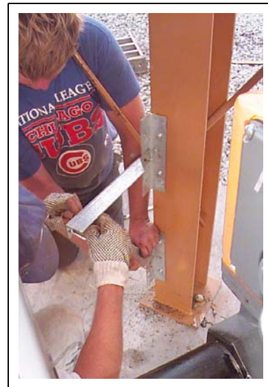
Figure 24Y Close Up - Bolting fuel train stand.
