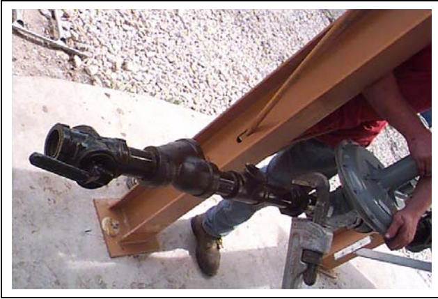
Figure 24AA Installing shut off section.
