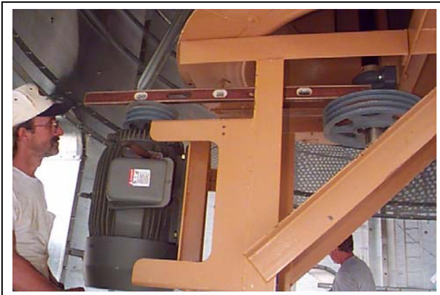
Figure 16V Checking top of motor sheave is level with top of fan sheave.
