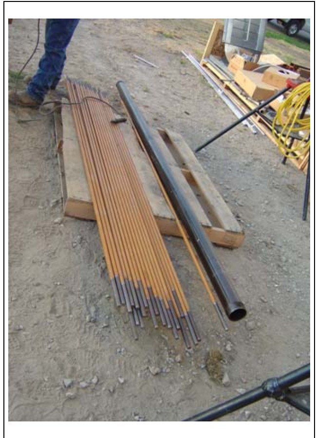
Figure 19AJ X-Bracing Rods
