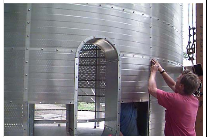
Figure 18Z Bolt outside wall sheets inside window frame.
