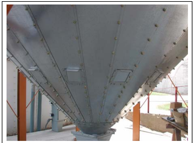
Figure 21AL Hopper installed with emergency discharge slide gates. (See Slide Gates on Page 140.)
