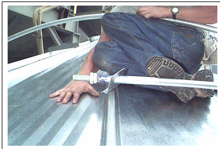
Figure 6AB Close Up - Installing expansion ring and clips.
