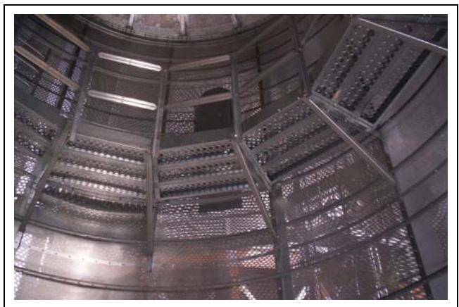
Figure 10AG View from below - Completed inside catwalk.
