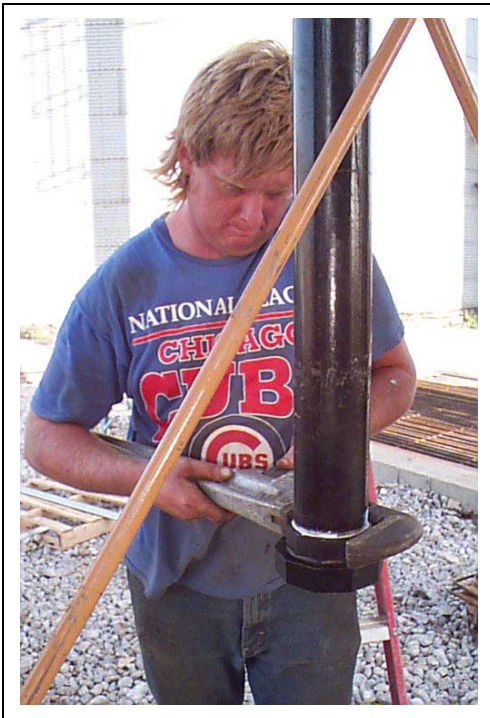
Figure 24P Tightening union to fuel pipe.
