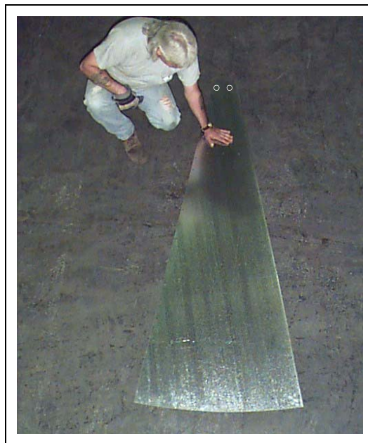
Figure 5AQ Plenum roof sheet. Do not fill top two (2) outside bolt holes on plenum roof sheets (circled) until peak cap installation.
