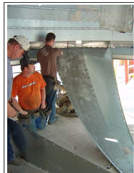
Figure 21P Aligning Outside Hopper Panels
