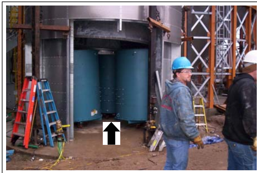
Figure 15W Three (3) fans form a cluster inside dryer.
