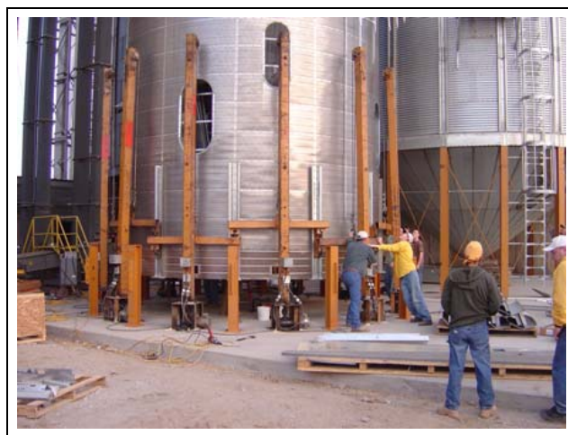
Figure 9I Jacks in place around dryer.
