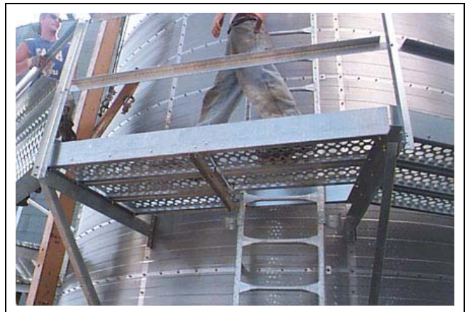
Figure 10Y Outside Catwalk Door - Closed
