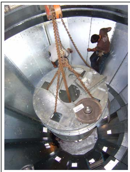
Figure 21AE View from above - Installing R.H. and L.H. hopper channels to bracket each other.
