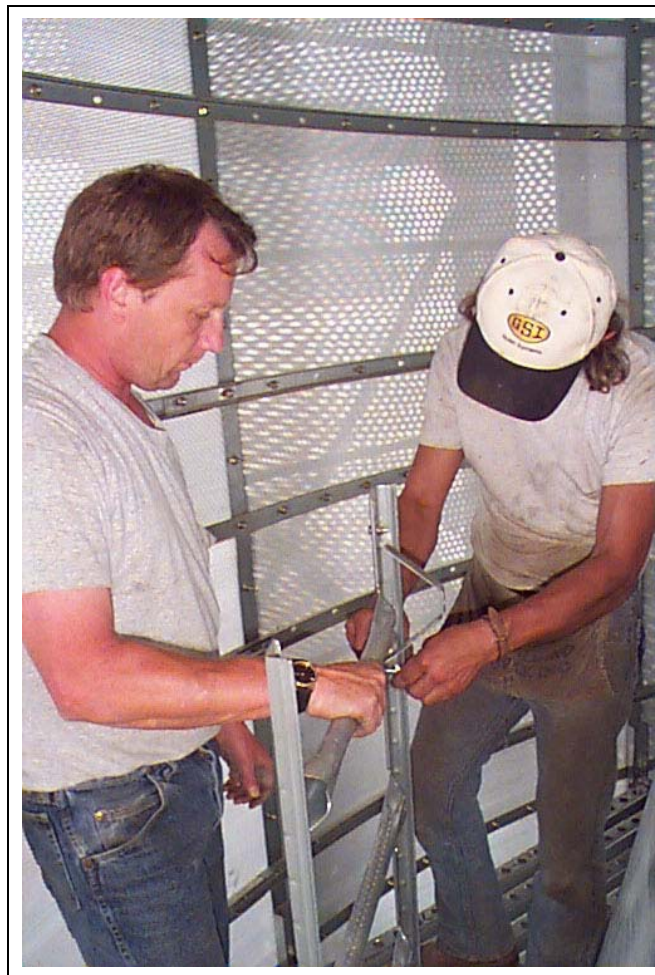
Figure 11K Bolting inside ladder standoff to 44" formed ladder section.
