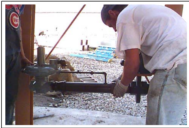
Figure 24V Installing regulator section.
