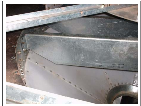
Figure 21AG Snug bolt all R.H./L.H. hopper channels in place, then tighten.
