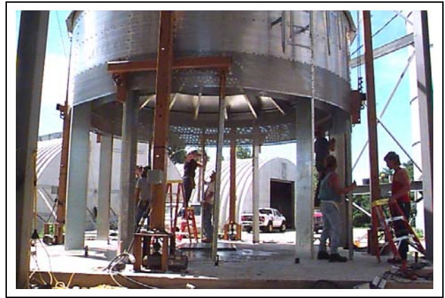
Figure 9M Bolting vertical channels.
