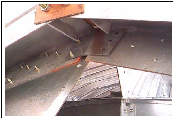
Figure 21L In photo, to demonstrate orientation, compression angle splice (arrow) is temporary bolted to compression angles. In actual installation, use common bolt to install outside hopper panels (over compression angle splice) to compression angles.
