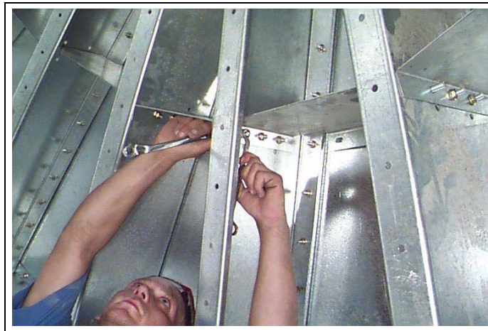
Figure 5AY Hand tightening rafter crossmembers.
