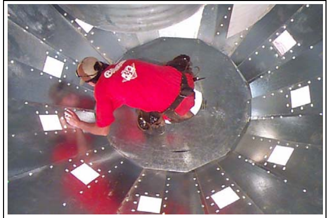
Figure 21Z Installing metering drum floor to underside of metering drum floor clips. Check for level.
