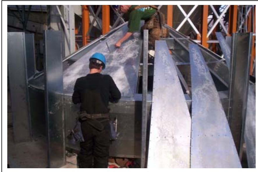
Figure 5AP Bolting Plenum Roof Sheets
