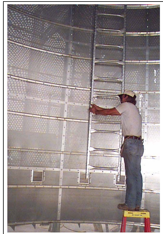
Figure 11G Installing first auxiliary ladder past slide gates - Clean out (grain turners).
