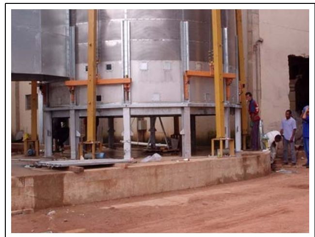
Figure 19U Upper legs are installed.
