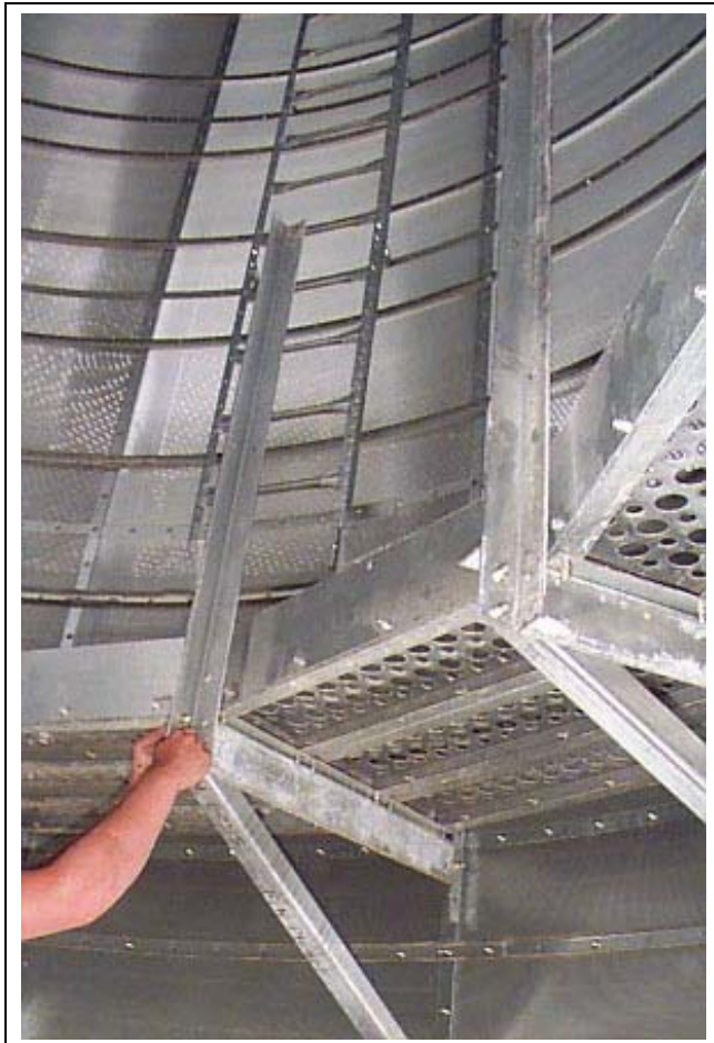
Figure 10AE Bolting inside catwalk vertical support to inside catwalk section.
