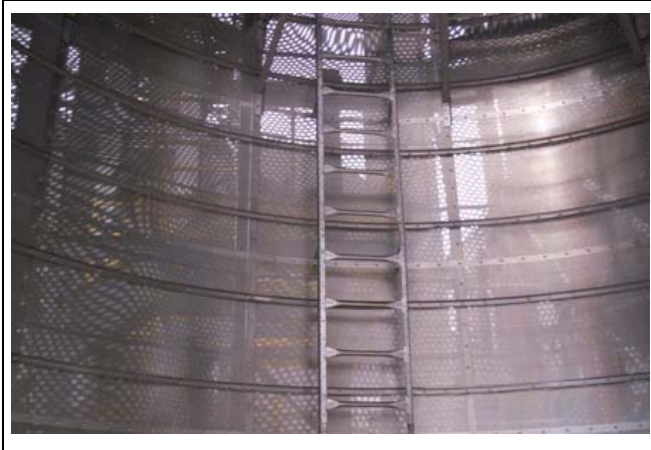
Figure 11D Installing auxiliary ladder from roof section down.
