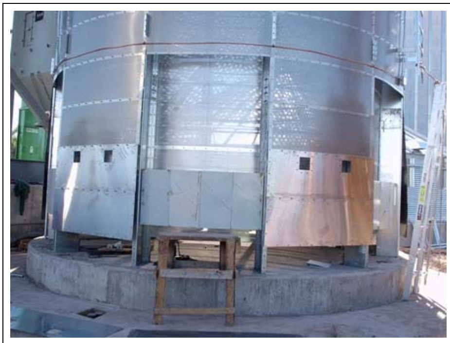
Figure 13F Installed grain turners.
