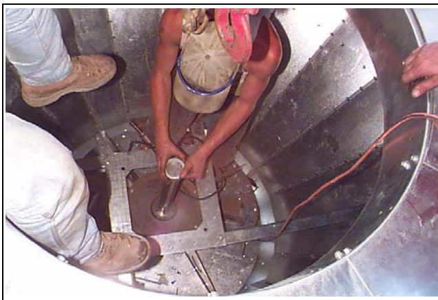
Figure 22R Sliding gearbox set collar (2-3/8") onto metering drum drive shaft.
