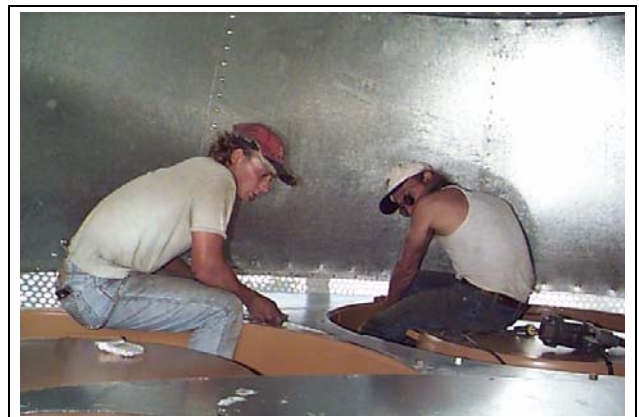
Figure 15AE Bolting fan reducer panel.
