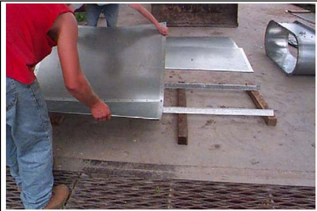
Figure 18G On a raised support, layout inside wall sheets that will support assembled window. Lap wall sheets as they should be lapped on dryer.
