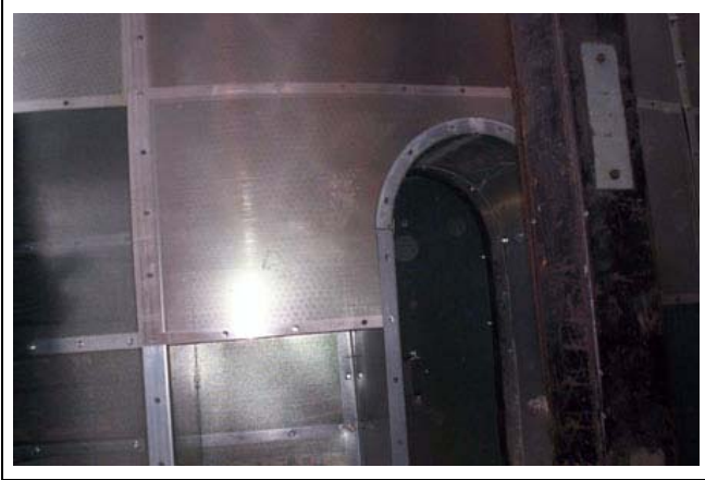
Figure 18AD 18" Window is installed. (Screening is not yet installed.)
