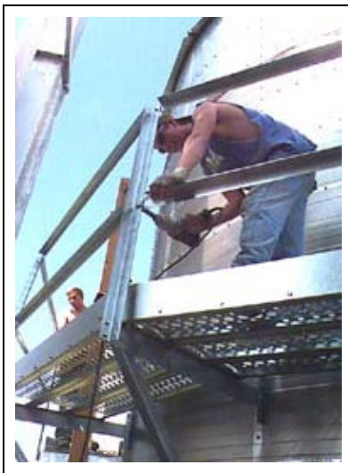
Figure 10V Tightening outside catwalk bottom handrail.
