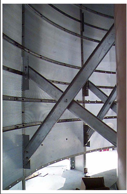
Figure 15AP X-Bracing installed.
