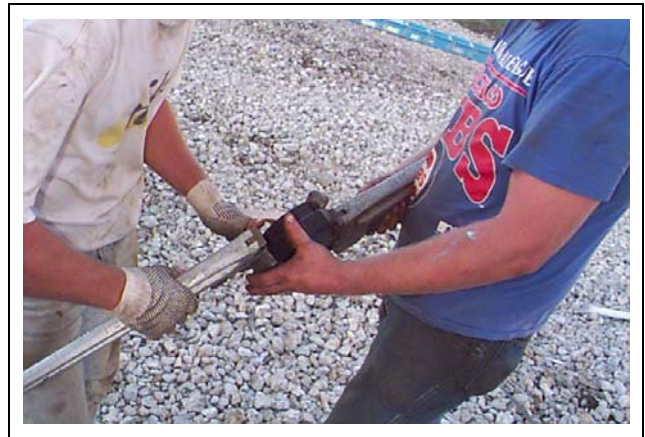
Figure 24N As required, break apart fuel train components, and install as shown in (see Figure 24A on Page 244 ), fuel train.
