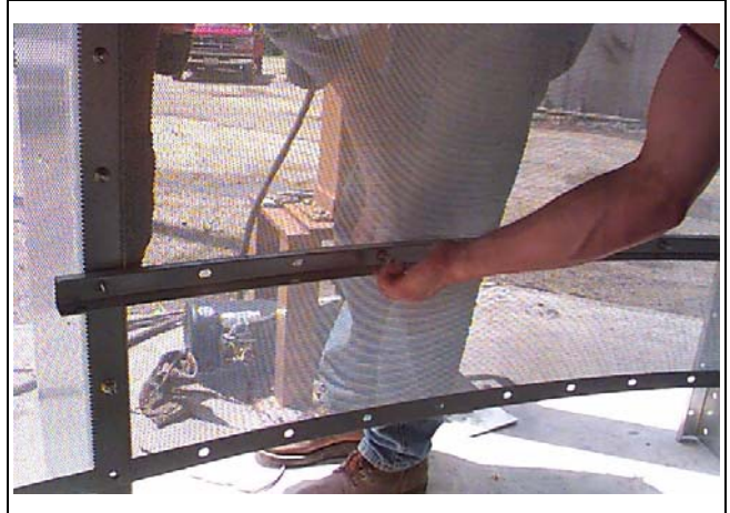
Figure 4X Close Up - Installing rolled plenum channels.
