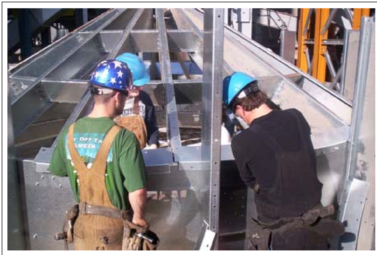
Figure 5AN Installing plenum roof flashing with tabs over inside top wall sheets.
