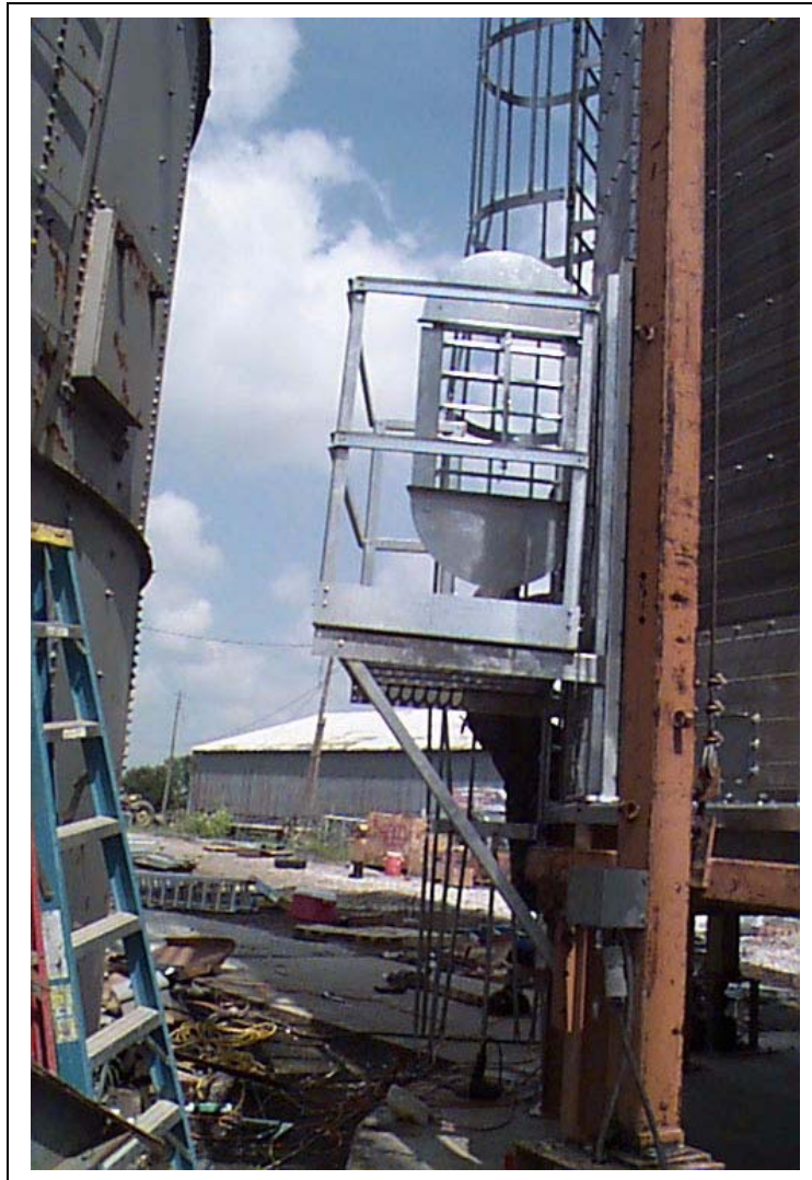
Figure 18AK Cool section door is installed.
