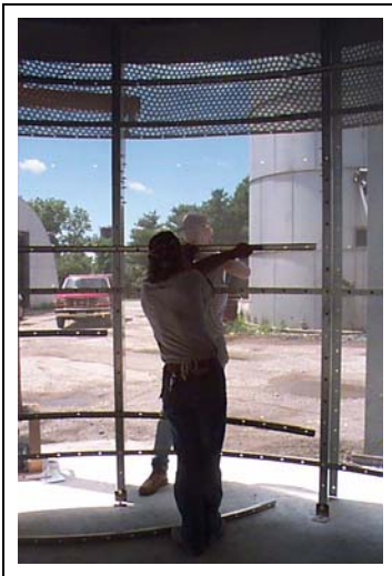
Figure 4W Installing rolled plenum channels.
