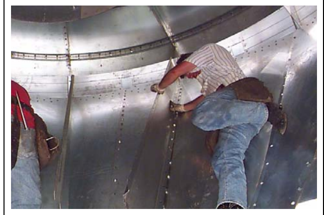
Figure 21AF View from below - Installing R.H. and L.H. hopper channels.
