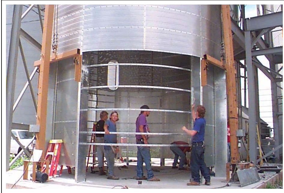
Figure 14G Install rolled plenum channels across gap to maintain shape and stability. Remove rolled plenum channels when ready to move burner into dryer.
