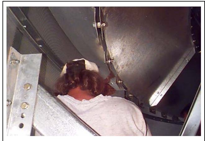
Figure 15BA Bolting outer divider hopper to inner divider hopper.
