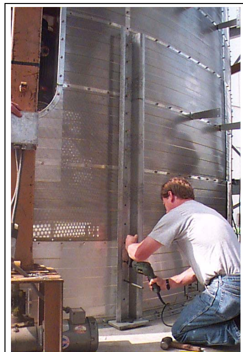
Figure 19J Tightening base stiffener weldment to vertical base channel.
