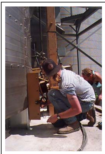
Figure 9D Installing lift brackets.
