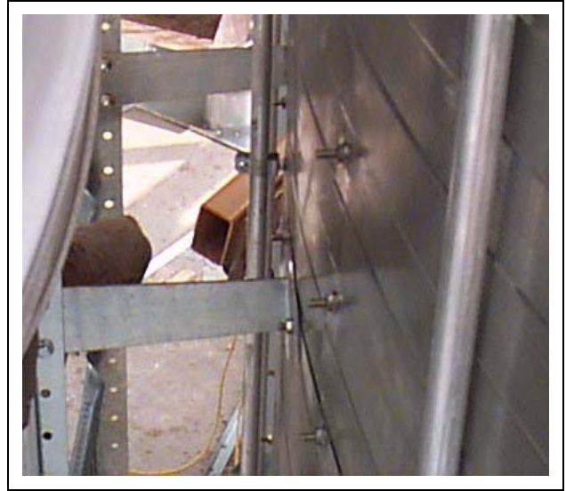
Figure 7N Close Up - Outside Ladder Brackets
