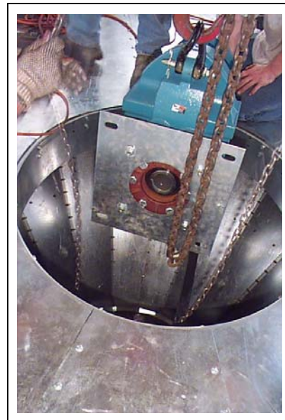
Figure 22V Lowering metering drum gearbox over metering drum.
