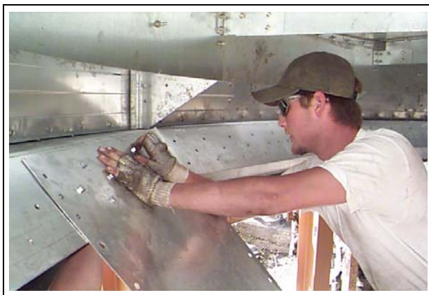
Figure 21M View from above - Bolting outside hopper panels over compression angles and compression angle splices.
