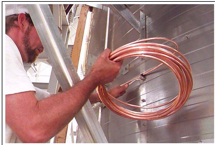
Figure 8U Close Up
