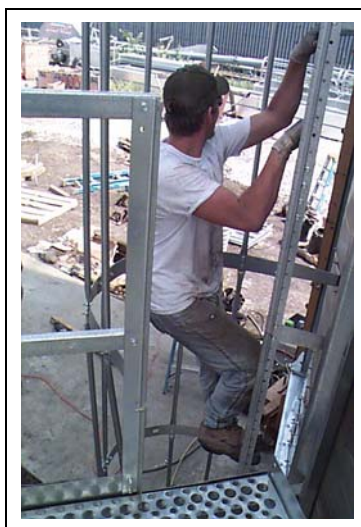
Figure 7S View from platform - Safety hoops installed to platform vertical supports.
