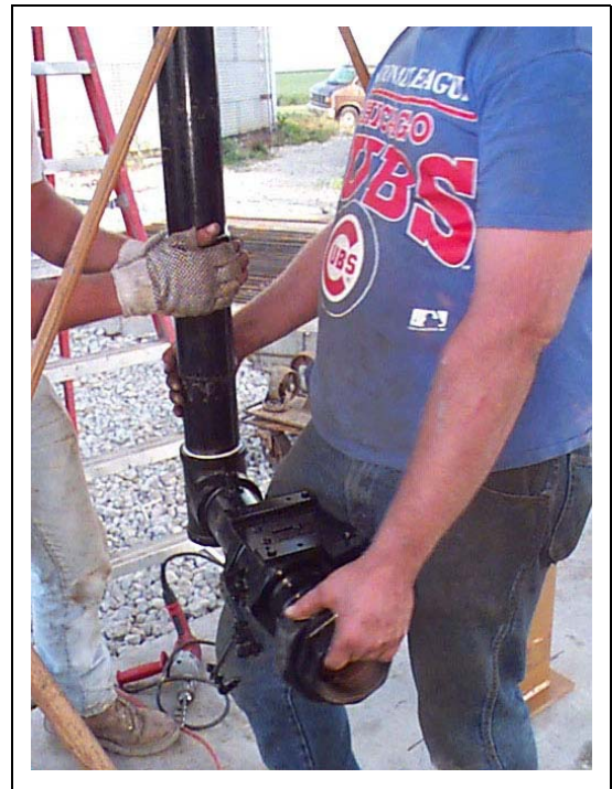
Figure 24R Connecting modutrol section to fuel pipe.
