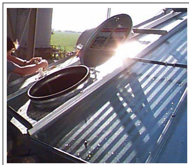
Figure 6AM Outside View - Access port cover installed.
