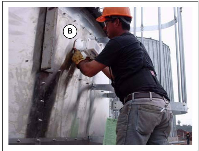
Figure 8L Upper bindicator (A) and lower bindicator (B) installed.
