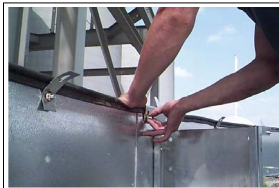
Figure 6K Installing eave clip and intermediate eave clips.
