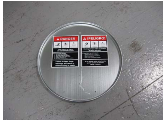
Tower roof access port with decals in place.
