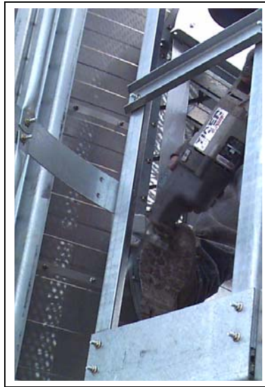
Figure 7P Close Up - Securing safety hoop to vertical support.
