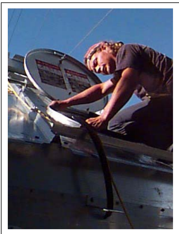
Figure 6AJ Pressing pre-cut bulb seal on rim of access port cut out on tower roof sheet.
