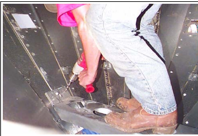
Figure 21X Drilling two (2) outside bolt holes at each end of metering drum bearing support. NOTE: Center bolt hole (arrow) is bolted with common bolt to a flat edged outside hopper panel seam. Check for level.
