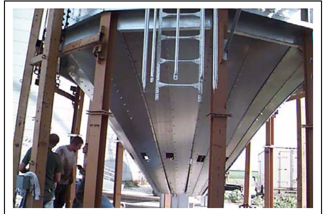
Figure 7O As dryer is constructed, continue installing outside ladder with safety cage.
