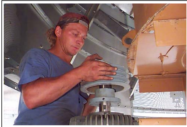
Figure 16P Sliding motor sheave on motor drive shaft.
