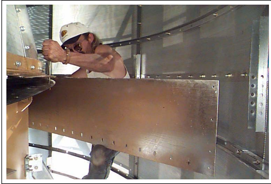
Figure 15AT Aligning fan skirting section to bottom ring of reducer.
