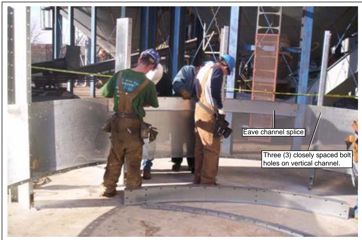
Figure 5X Installing eave channels to vertical channels.
