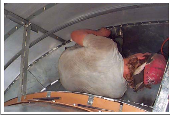
Figure 15BC Drilling bolt holes in inside wall sheets to bolt to outer divider hopper.
