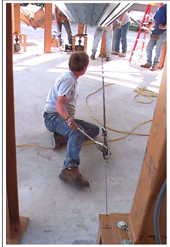
Figure 19Y Winching dryer legs into position.
