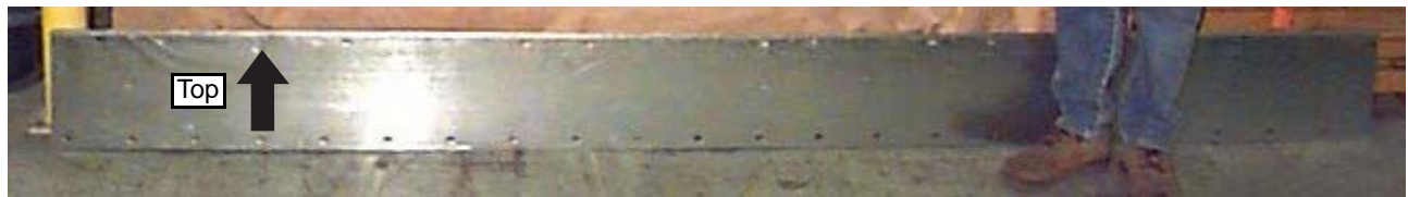
Figure 6D Roof band section. Top of roof band has pairs of bolt holes alternating with single bolt holes. Bottom of roof band has evenly spaced bolt holes.
