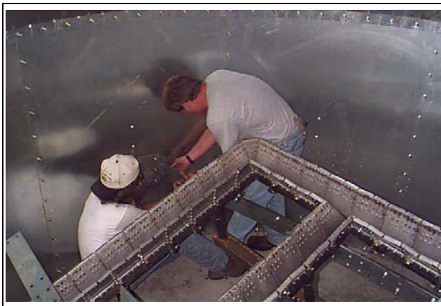
Figure 14Q Installing second burner support bracket to burner mounting brackets.
