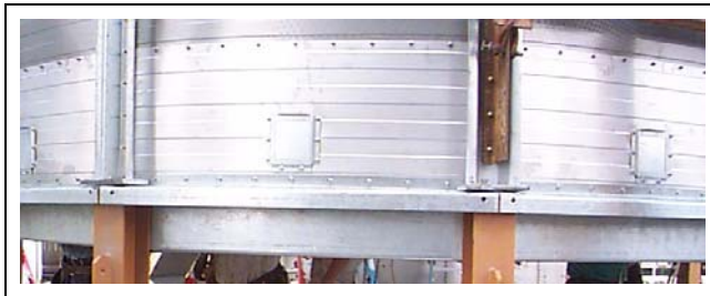
Figure 12C Slide gate installed to outside bottom wall sheet. (For emergency discharge.)
