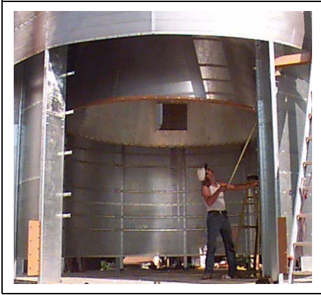
Figure 15Q Checking clearance for fan under reducer/burner.
