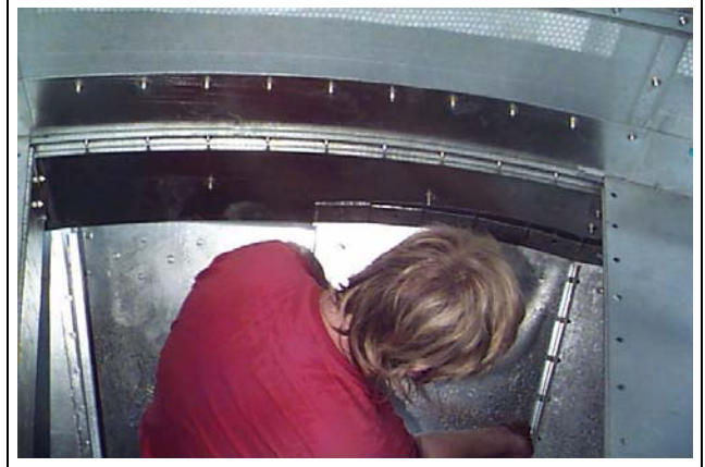
Figure 21AJ Self - Tapper inside hopper flange to inside solid wall sheet.
