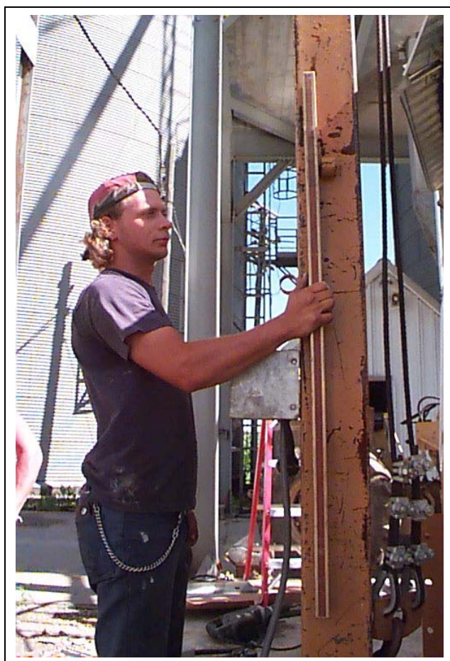
Figure 9H Checking jack is plumb and level.
