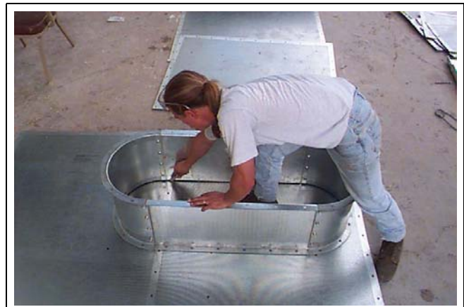
Figure 18L Mark around inside perimeter of window frame.
