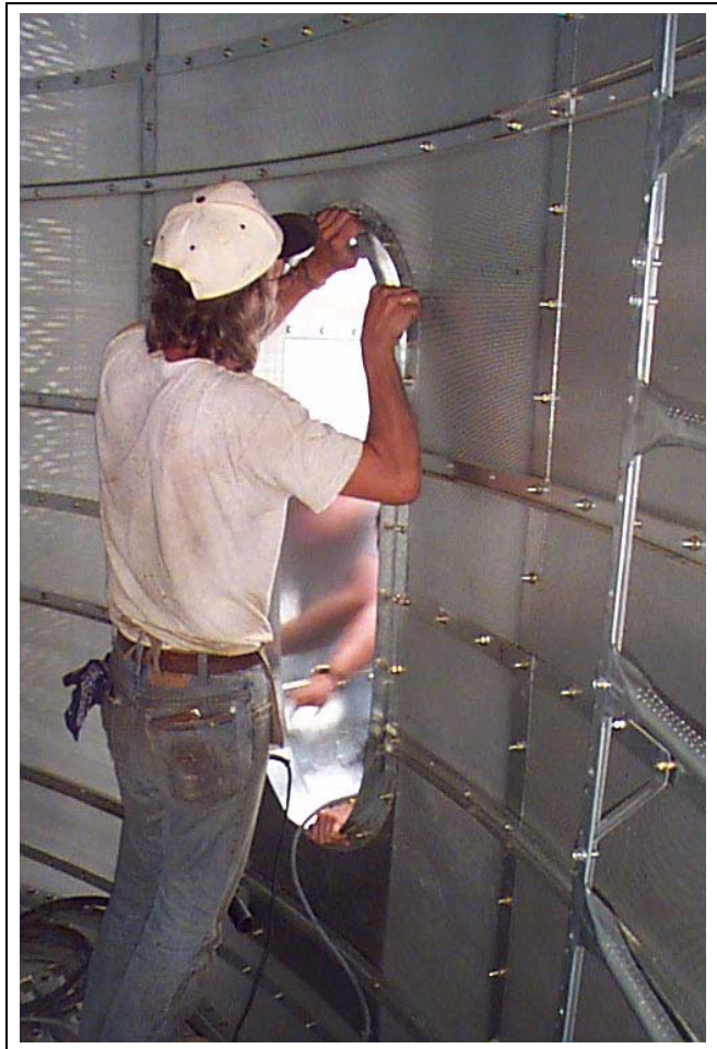
Figure 18AP Wrapping heat section door sleeve around inside of door frame.
