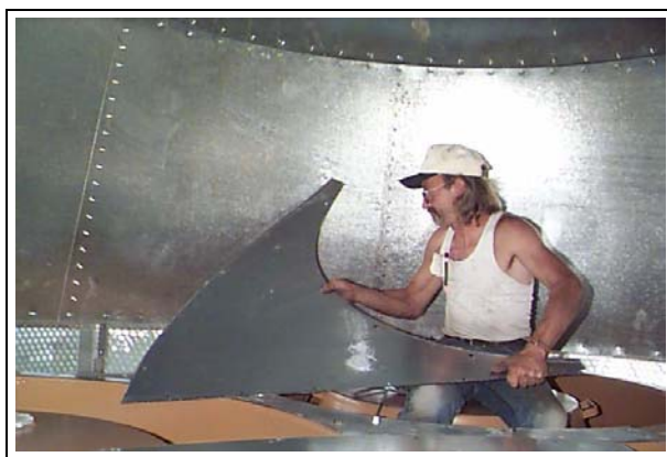
Figure 15AD Positioning fan reducer panel.
