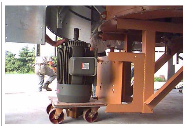
Figure 16I Moving fan motor to fan motor mount.
