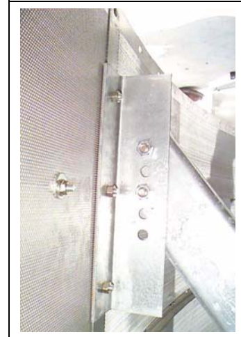
Figure 15AM L.H. View of bracing installed to fan support clip.
