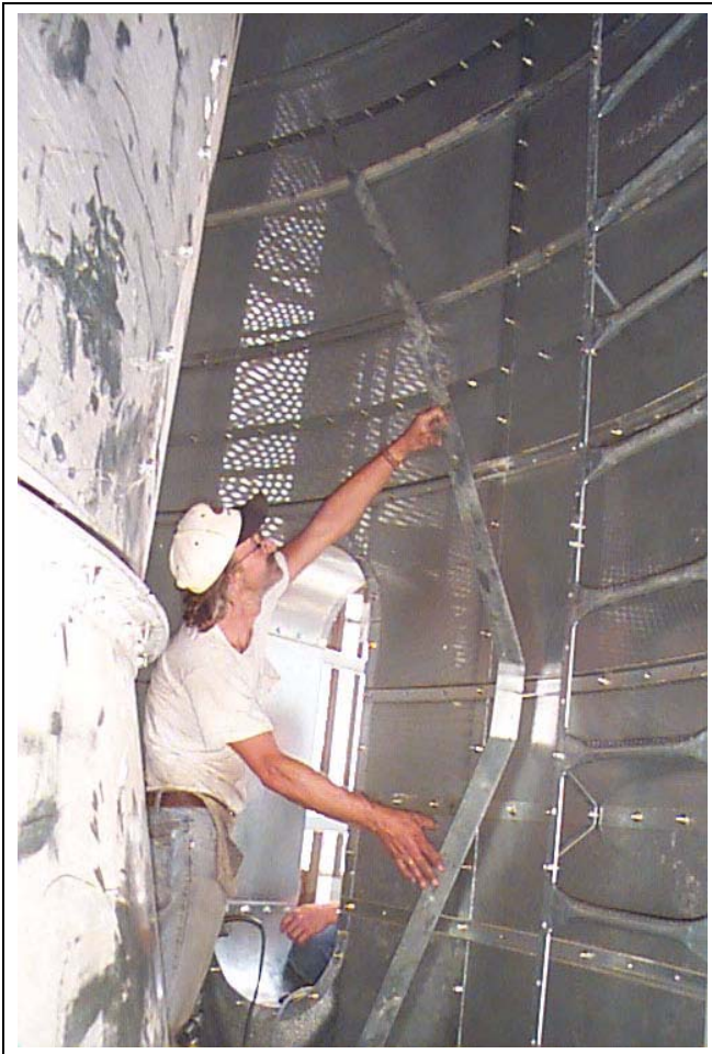
Figure 18AO Installing 3" wide heat section door sleeve.
