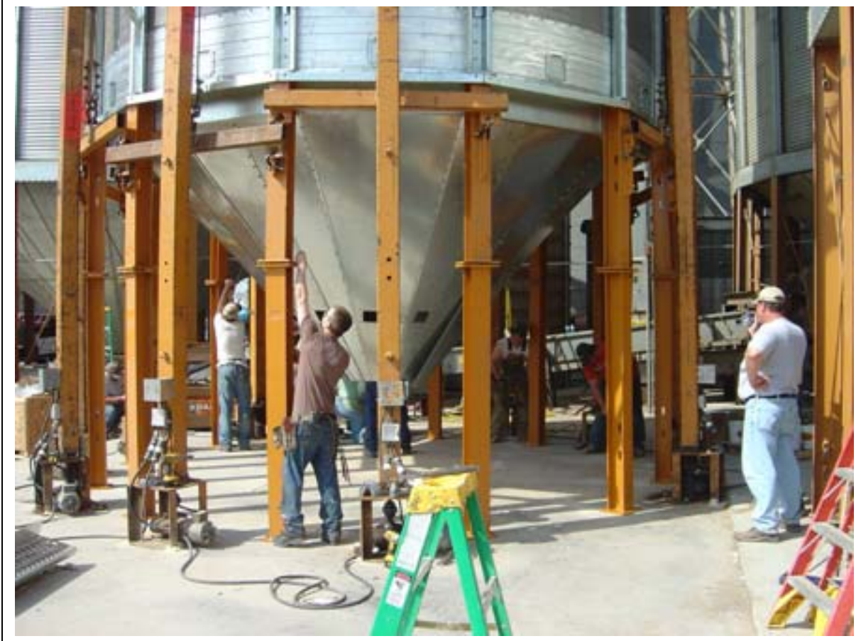
Figure 19V Bolting lower leg to upper leg.
