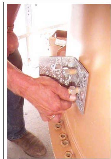
Figure 15AJ Installing fan cross beam clip to fan.
