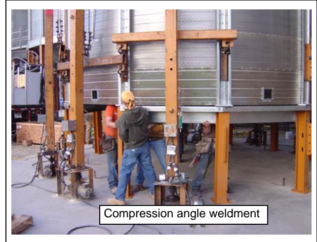
Figure 19L Bolting compression angle weldments to bottom of sealing strip.
