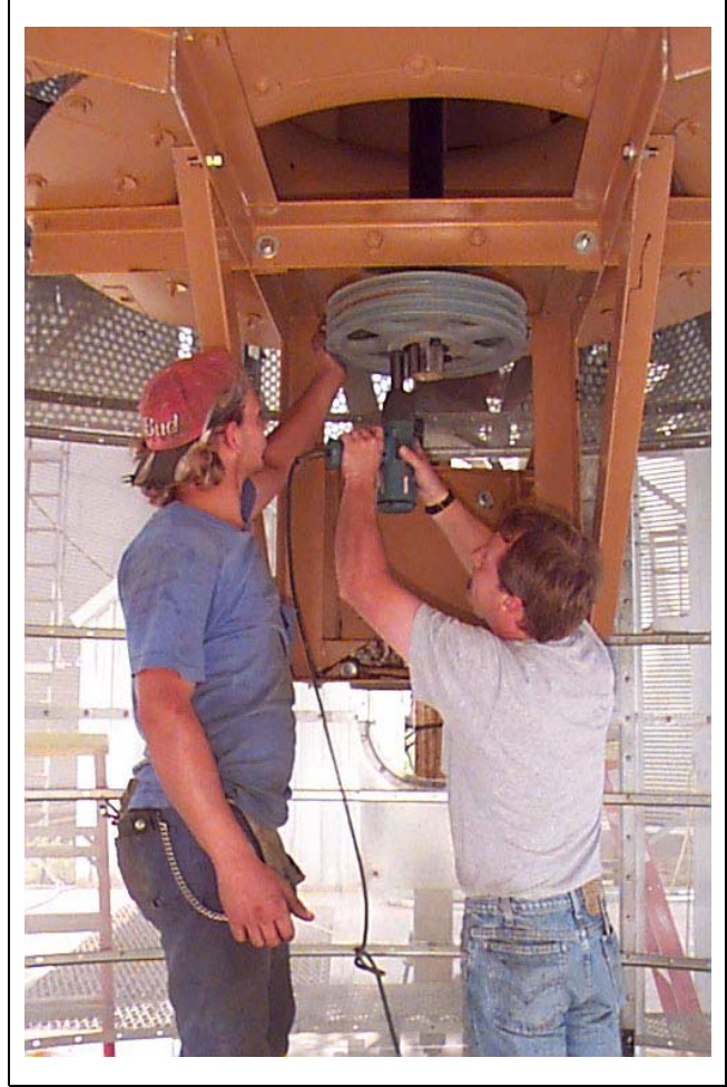
Figure 16W Tightening fan sheave bolts.
