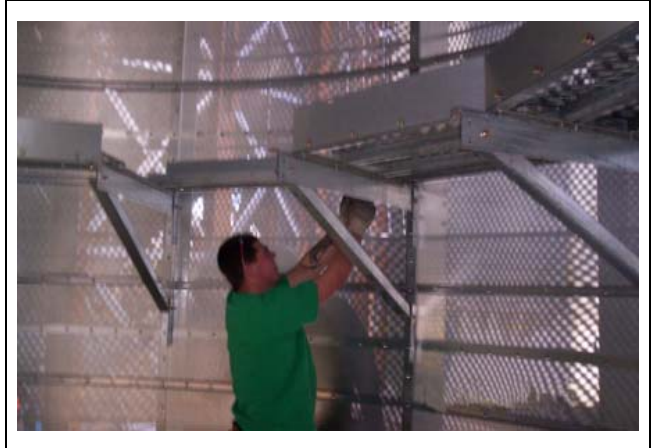
Figure 10AF Bolting inside catwalk splice plate to inside catwalk section.
