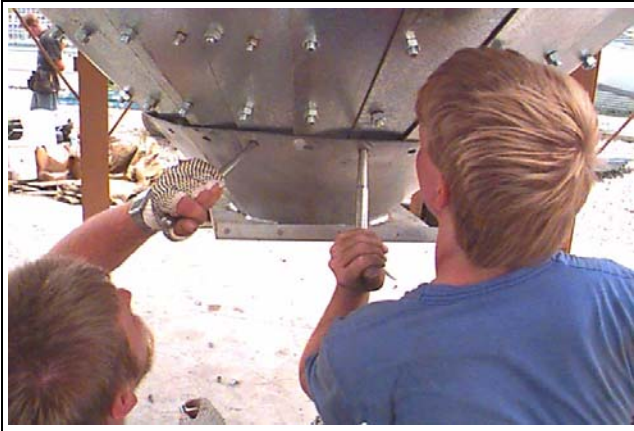
Figure 21W Aligning hopper discharge weldment to outside hopper panels.
