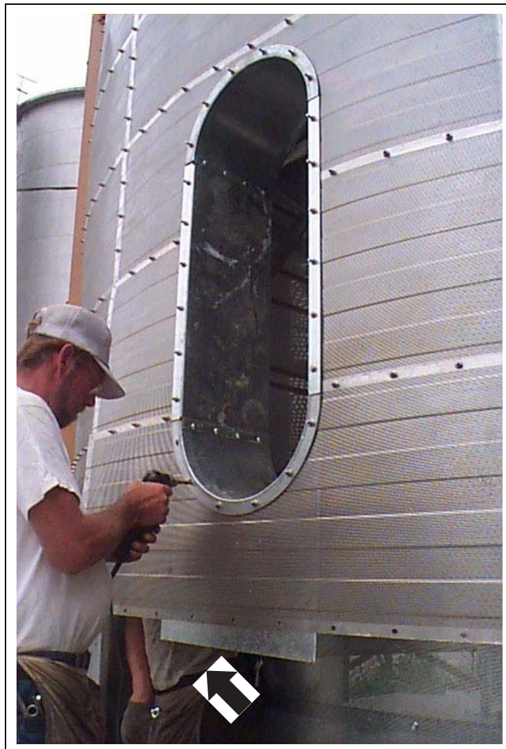
Figure 18AA Bolt window frame to outside walls.
