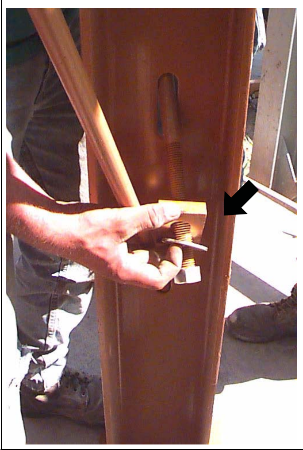
Figure 19AL Secure X-bracing rods with 3/4" nut, 3/4" washer, and cast washer (arrow).
