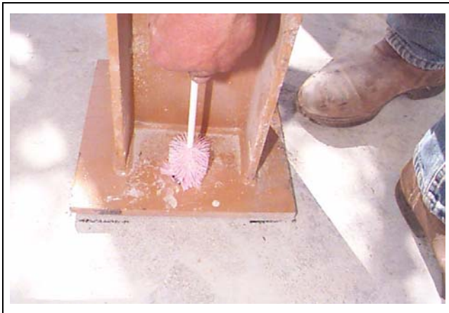
Figure 19AF Clean Out Hole
