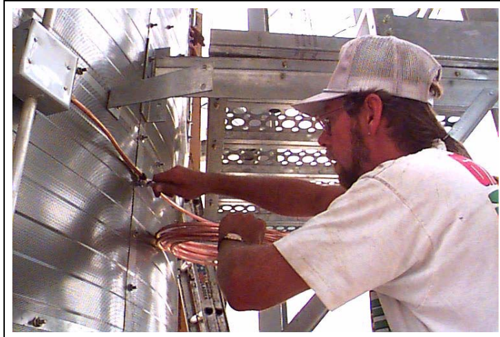
Figure 8T Installing copper capillary tubing with insulated clips.
