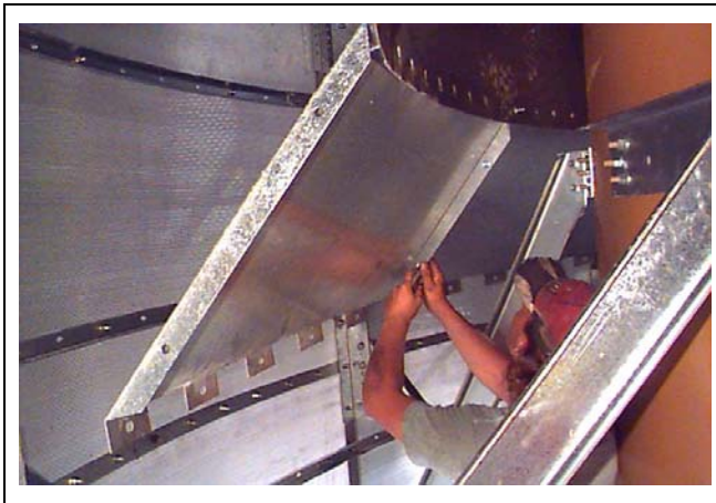
Figure 15AZ Bolting inner divider hopper sections together.
