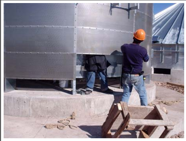
Figure 4V Hanging inside wall sheets.
