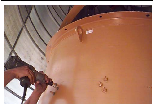
Figure 15AG Use existing bolts on fans to install intermediate fan support beams and some fan cross beam clips.
