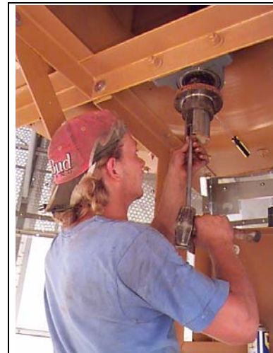
Figure 16S Placing fan hub key in fan hub.
