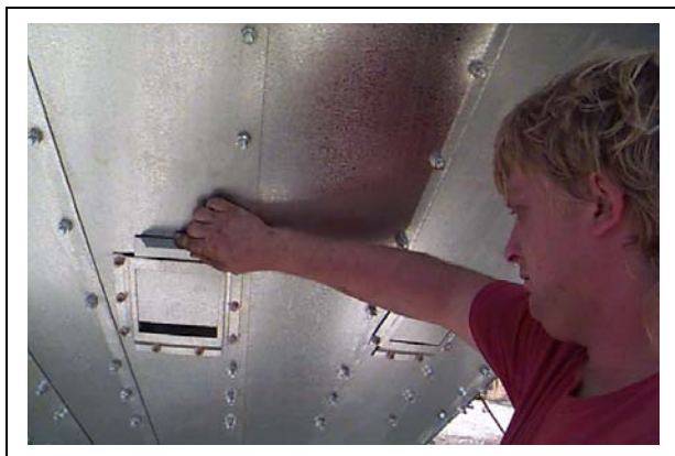
Figure 12D Installing slide gate plate to frame on outside hopper panels. (For emergency discharge.)
