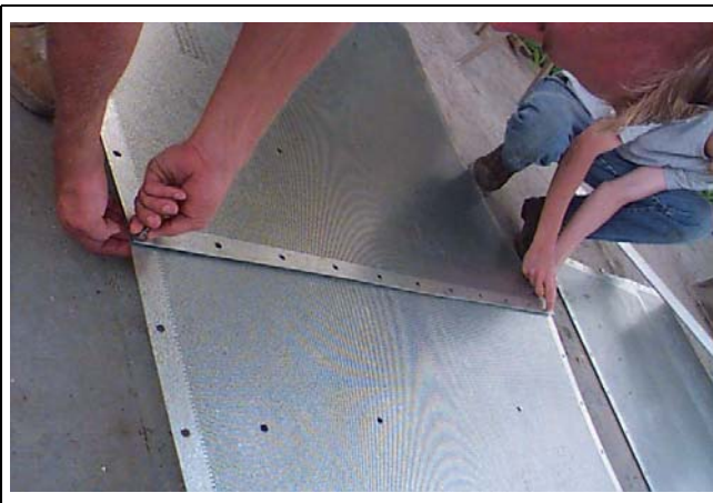
Figure 18I Temporarily snug bolt corners of two (2) wall sheets.
