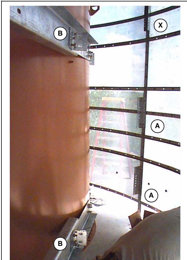
A. Fan support clips B. Fan crossbeam clips X. Reducer walkway support clips can be installed at this point. Reducer walkway is installed in later step.
