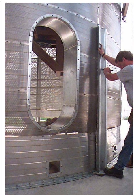
Figure 19I Positioning base stiffener weldment flush over vertical base channel (that is under outside solid wall sheets.)
