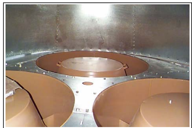
Figure 15AF Fan housing splice installed.
