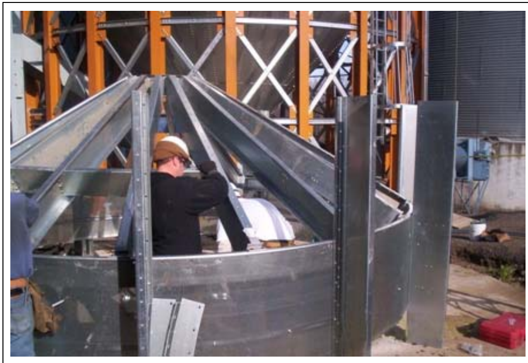
Figure 5AM Installing rafter crossmembers.
