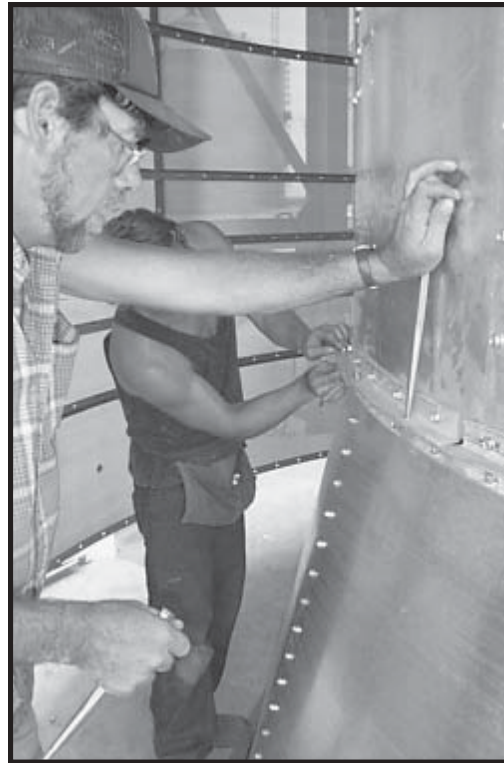
Photo 12-26 Aligning and bolting Reducer to Burner Housing.
