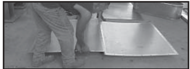
Photo 16-8 Align bolt holes in the two Wall Sheets.
