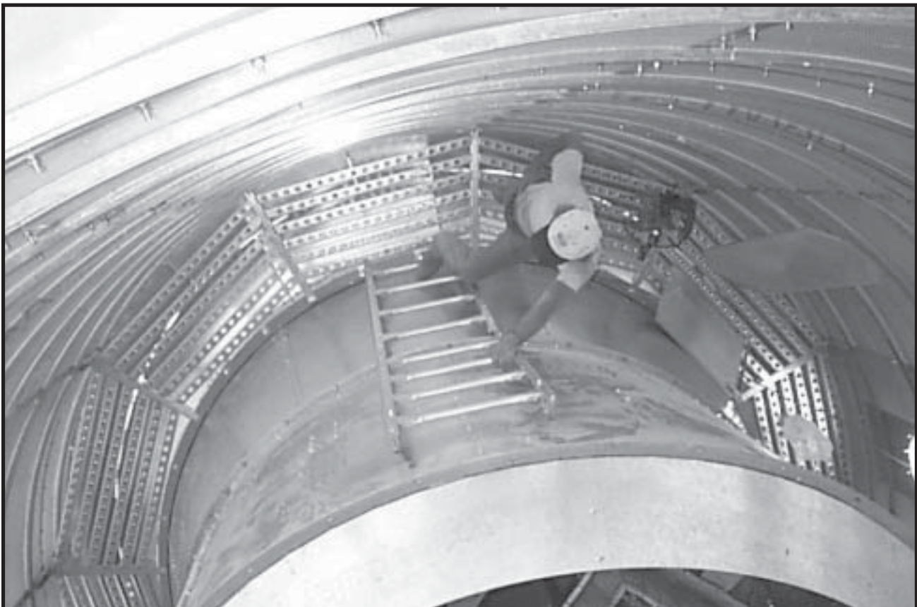
Photo 9-14 Installed Burner Housing Ladder.
