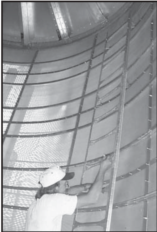
Photo 9-4 Installing Auxiliary Ladder from roof section down.
