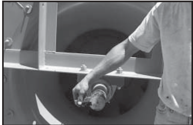
Photo 13-12 Remove Fan Drive Shaft Key and save it.
