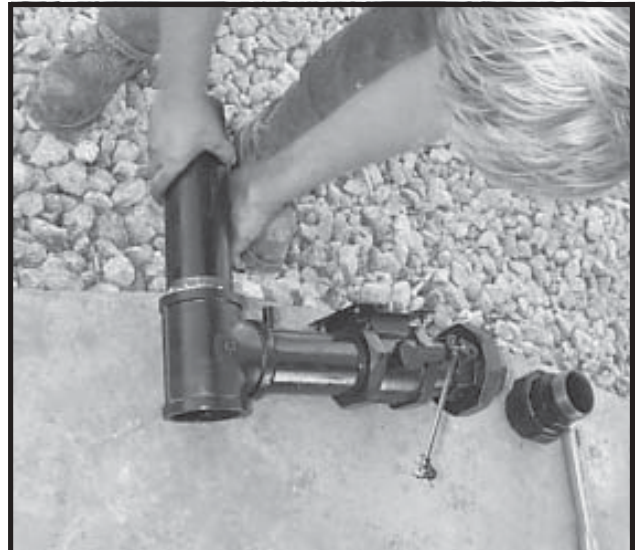
Photo 22-16 Attaching 12" Nipple to Modutrol Section.
