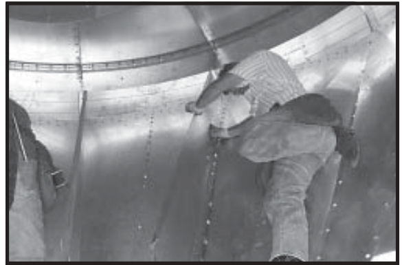
Photo 19-32 View from below - Installing RH and LH Hopper Channels.
