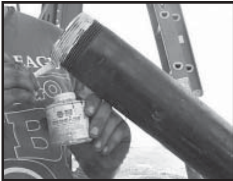
Photo 21-9 Seal all threaded pipe connections with Heavy Duty Pipe Sealing Compound.
