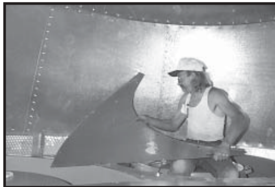
Photo 13-26 Positioning Fan Reducer Panel.
