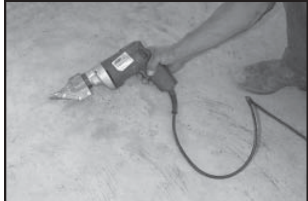
Photo A-2 Metal Shear to cut Wall Sheets and screen.
