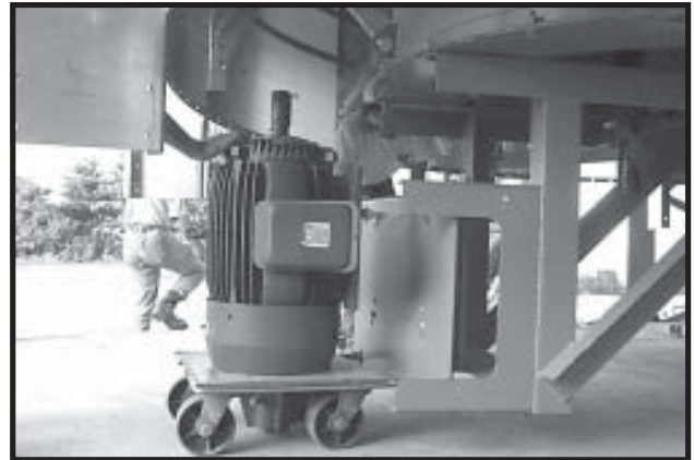
Photo 14-9 Moving Fan Motor to Fan Motor Mount.
