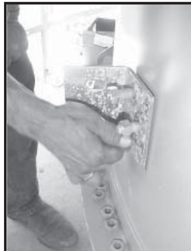
Photo 13-32 Installing Fan Cross Beam Clip to Fan.
