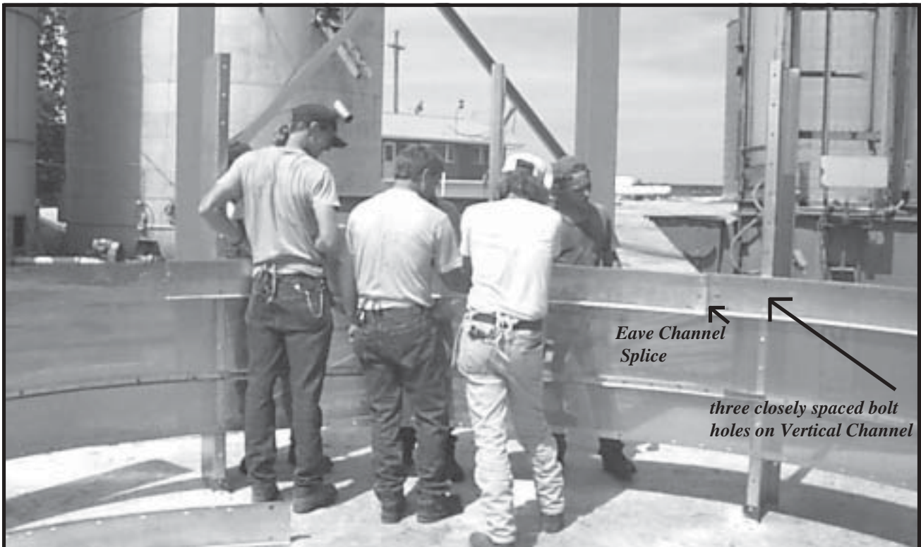
Photo 2-16 Installing Eave Channels to Vertical Channels.
