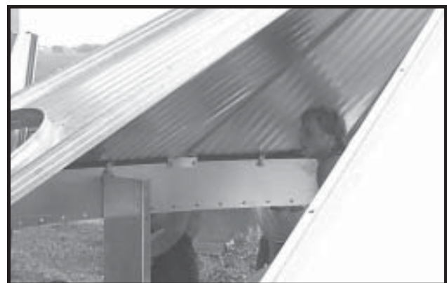
Photo 3-17 Inside view - Tower Roof Sheets bolt to Eave Clips, and Intermediate Eave Clips.
