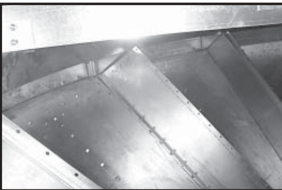
Photo 19-33 Snug bolt all RH/LH Hopper Channels in place, then tighten.
