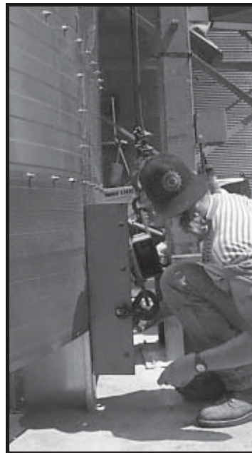
Photo 7-4 Installing Lift Brackets.
