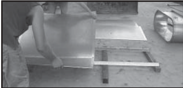
Photo 16-7 On a raised support, layout Inside Wall Sheets that will support assembled Window. Lap Wall Sheets as they should be lapped on dryer.
