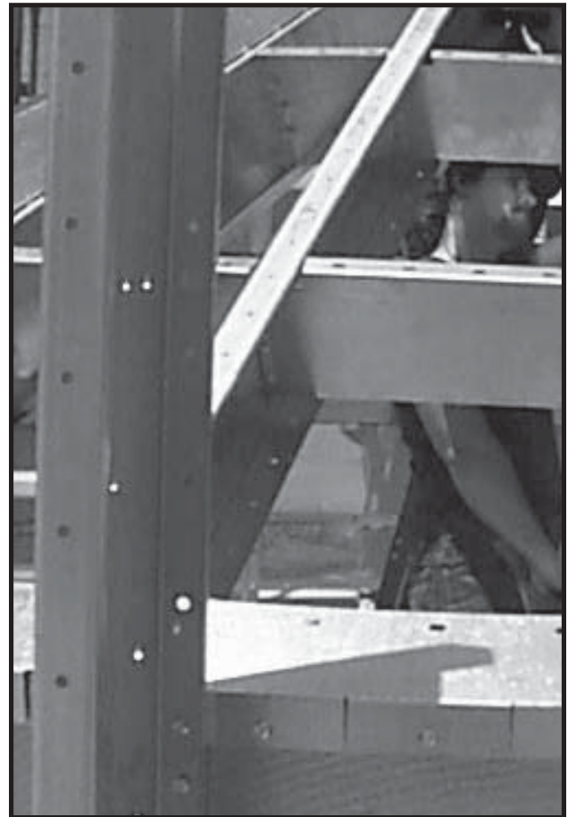
Photo 2-29 Installing Plenum Roof Flashing with tabs over Inside Top Wall Sheets.
