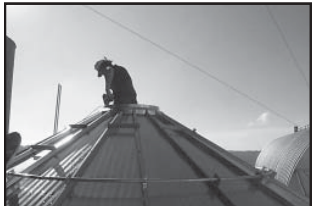
Photo 3-29 Tightening Center Collar Flashing bolts.
