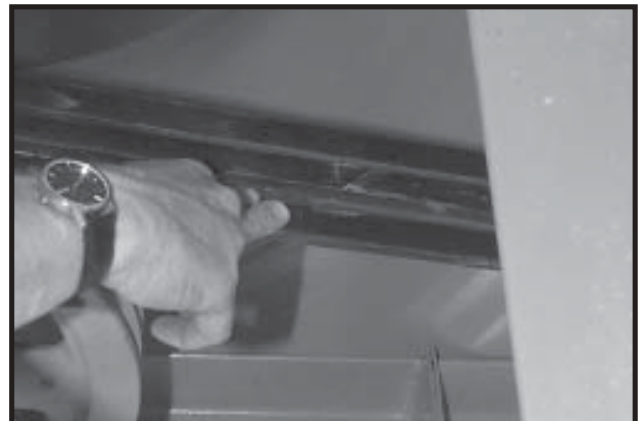
Photo 14-29 Checking Fan Belt tension. Can press down about one Fan Belt width.
