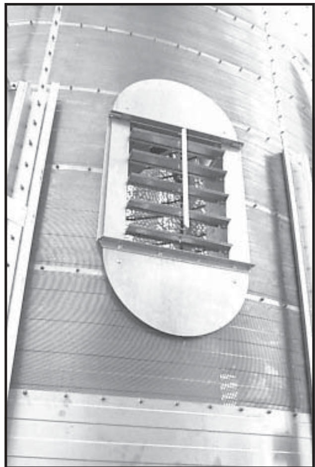
Photo 16-36 Outsided view - installed 24” Louvered Window, with louvers open.
