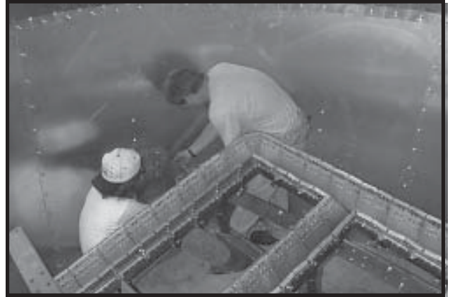
Photo 12-15 Installing second Burner Support Bracket to Burner Mounting Brackets.
