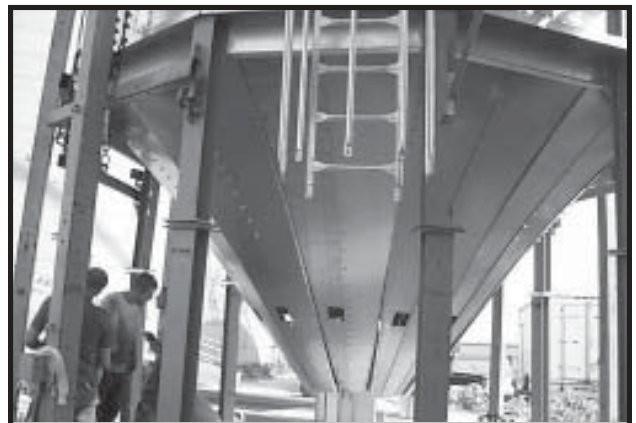
Photo 4-15 As dryer is constructed, continue installing Outside Ladder with Safety Cage.
