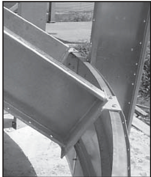
Photo 2-25 Close Up - Bolt bottom of Plenum Roof Rafters to top of Plenum Roof Eave Channel (in pairs of bolt holes).
