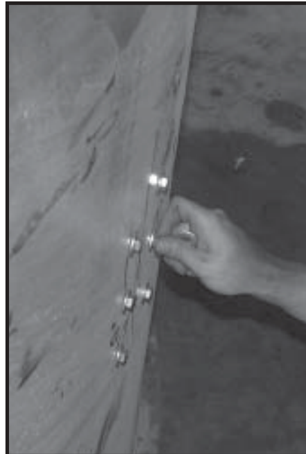
Photo 12-13 View outside Burner Housing - Installing Burner Mounting Bracket with washers.
