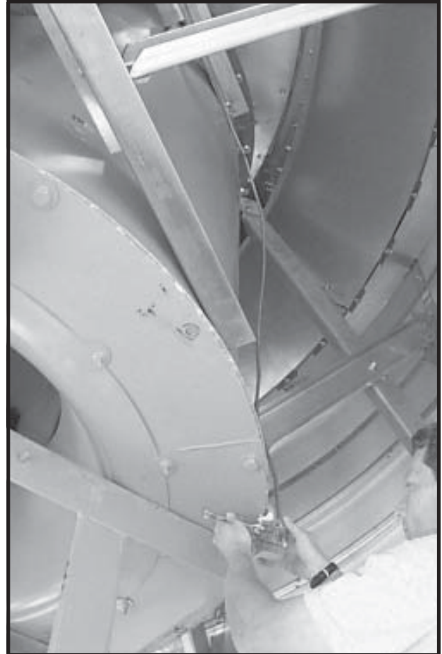
Photo 15-11 Attaching Beam Clamp to bottom edge of Fan.
