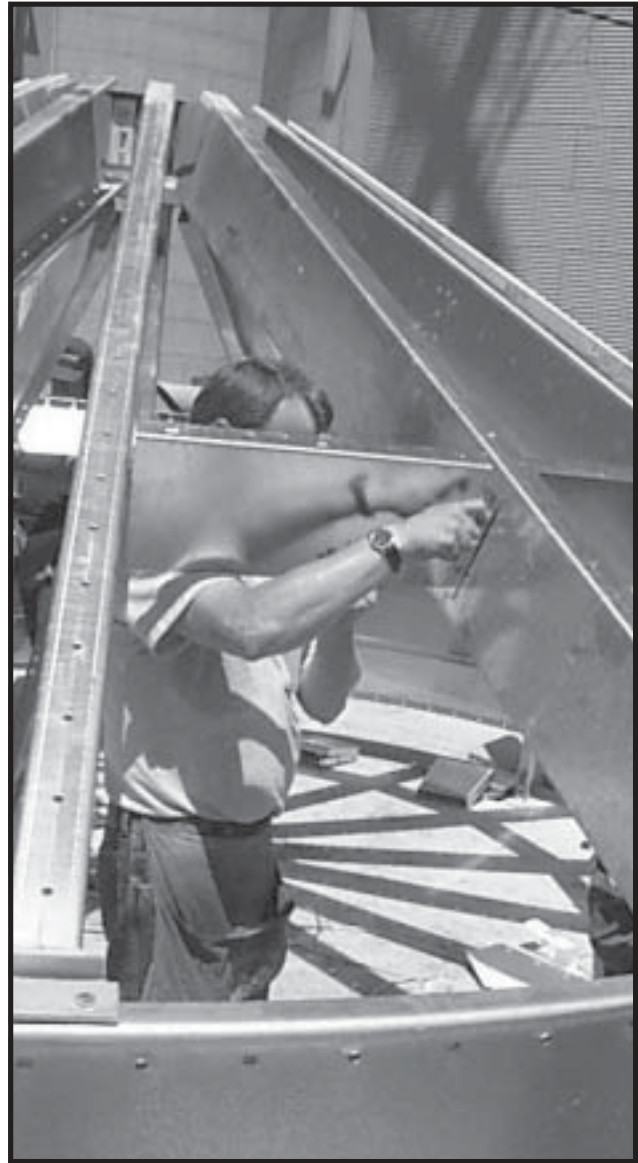
Photo 2-28 Installing Rafter CrossMembers.
