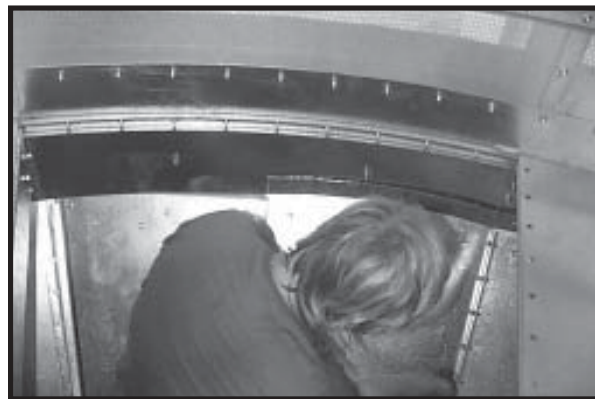
Photo 19-38 Bolting Inside Hopper Flange to Inside Solid Wall Sheet.
