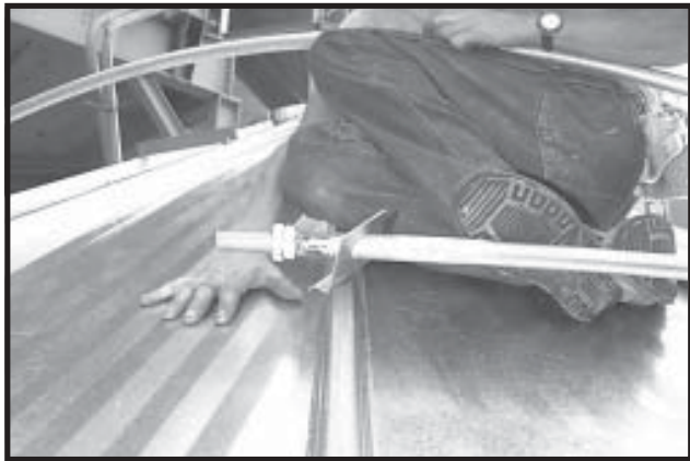
Photo 3-25 Close Up - Installing Expansion Ring & Clips.
