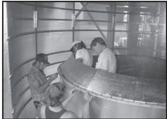
Photo 12-8 Installing Burner Housing Outlet Baffle to top rim of Burner Housing.
