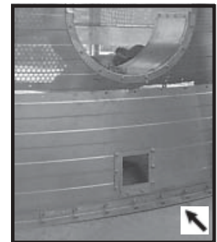
Photo 17-4 Sealing Strip (arrow) is installed to bottom of Outside Solid Wall Sheets.
