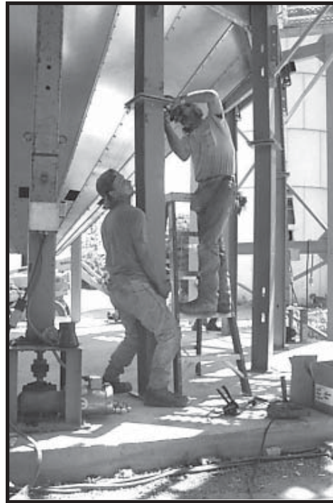
Photo 17-21 Bolting Lower Leg to Upper Leg.
