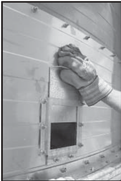
Photos 10-5 Installing Slide Gate Plate to frame on Outside Bottom Wall Sheet. (For emergency discharge.)
