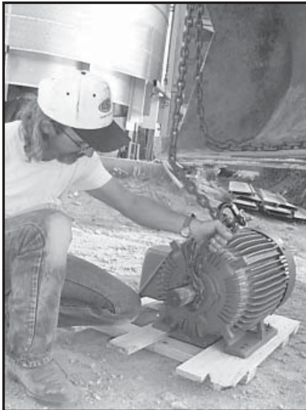
Photo 14-8 Attach lifting tackle to Fan Motor.
