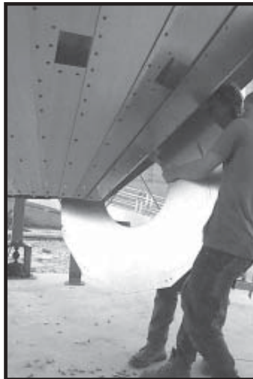
Photo 19-20 Bring Metering Drum Floor into Outside Hopper before closing in with last panel.
