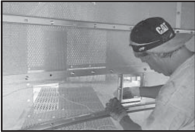
Photo 10-2 Installing Slide Gate Frame to Inside Clean Out Wall Sheet. (For Grain Turner clean out.)
