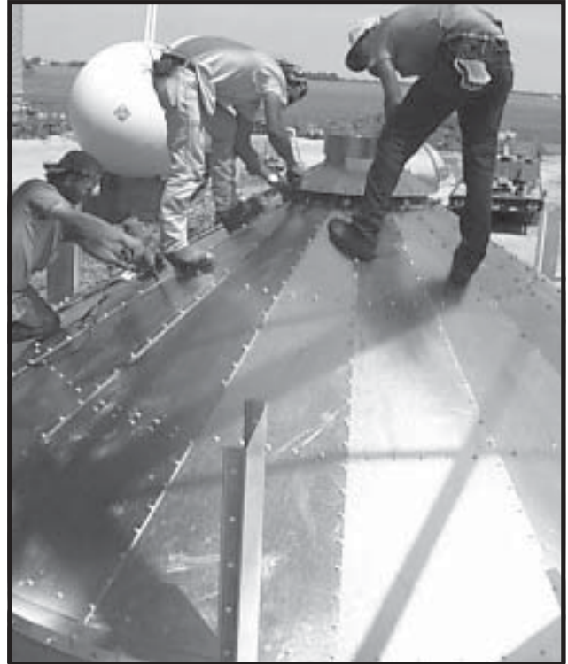
Photo 2-36 Installing Peak Cap to Plenum Roof Sheets.
