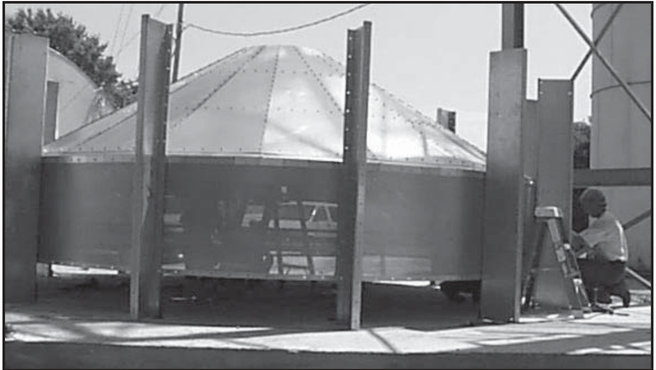
Photo 2-34 Plenum Roof is ready for Peak Cap Assembly installation.
