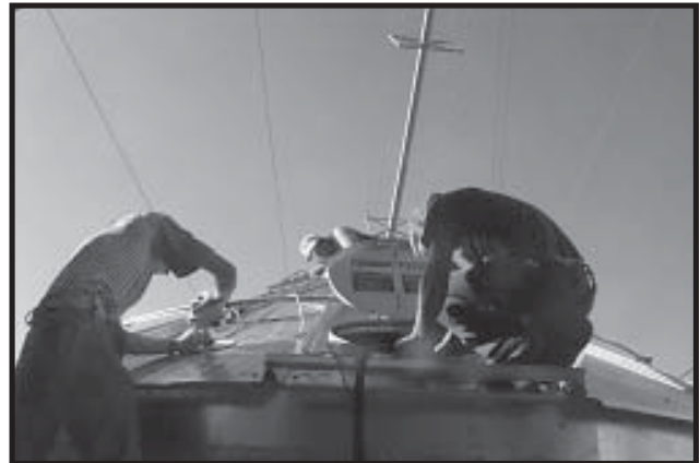
Photo 5-9 Installing Upper Bindicator.
