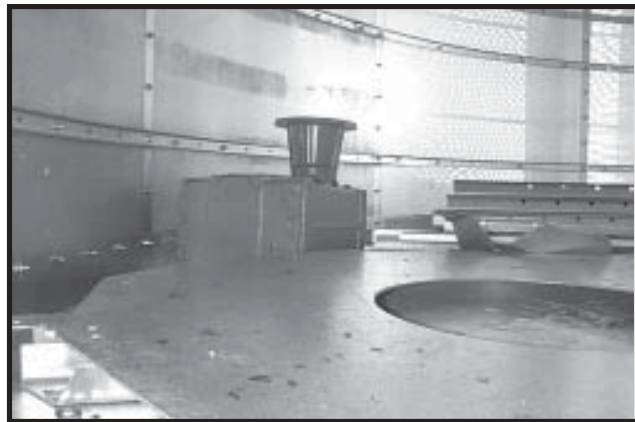
Photo 18-21 Temporarily store parts for Hopper and Metering Drum on Cool Section Floor.
