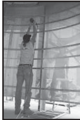
Photo 1-8 Tightening Inside Wall Sheets.
