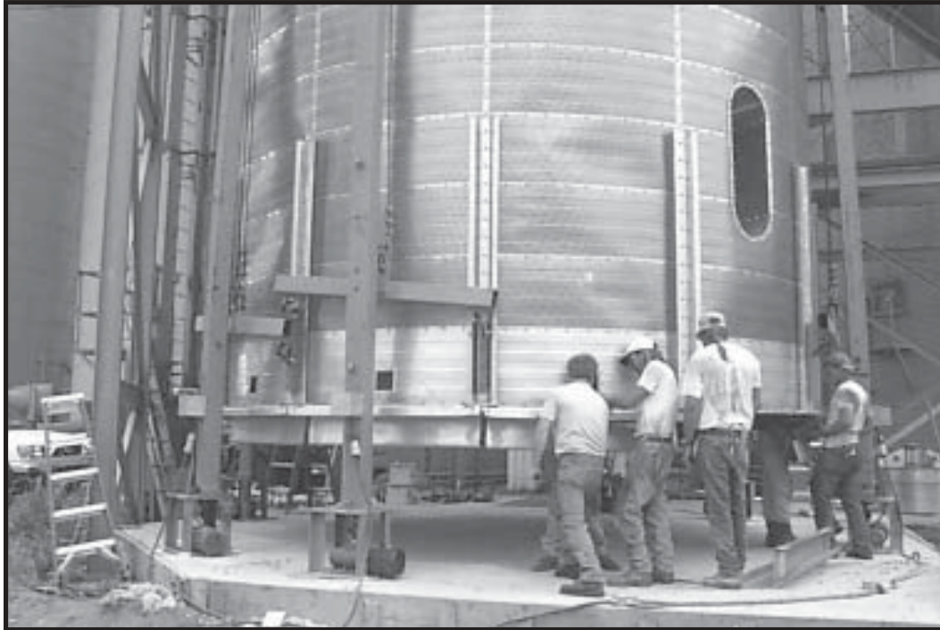
Photo 17-11 Compression Angle Weldments encircle base of dryer.
