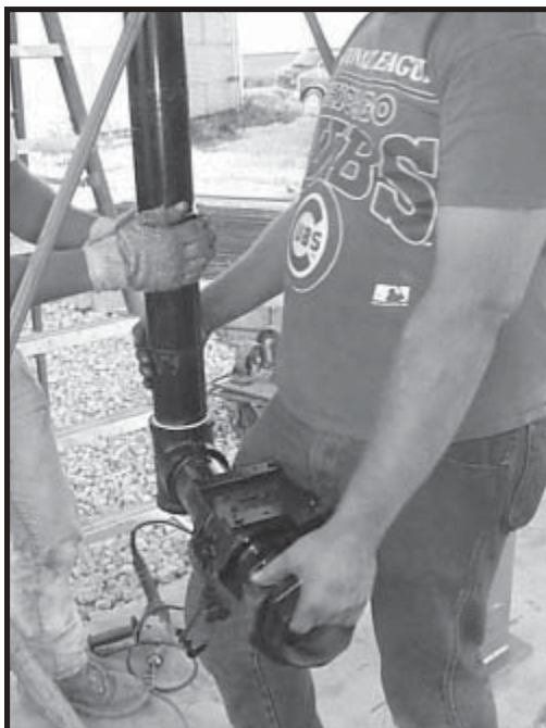
Photo 22-17 Connecting Modutrol Section to Fuel Pipe.
