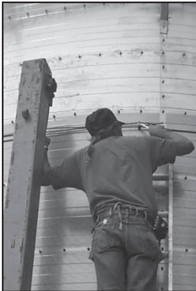
Photo 5-17 Caution - do not cut ends of Copper Capillary Tubing. Overlap them.
