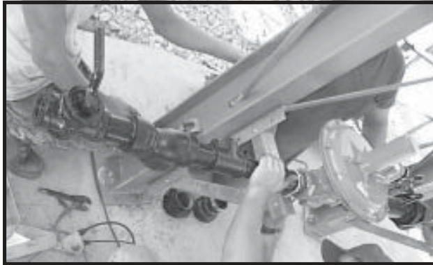
Photo 22-27 Second Fuel Train stand installed.
