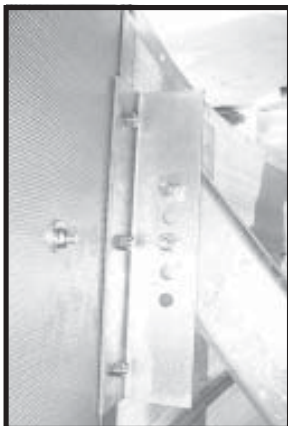
Photo 13-35 LH view of Bracing installed to Fan Support Clip.
