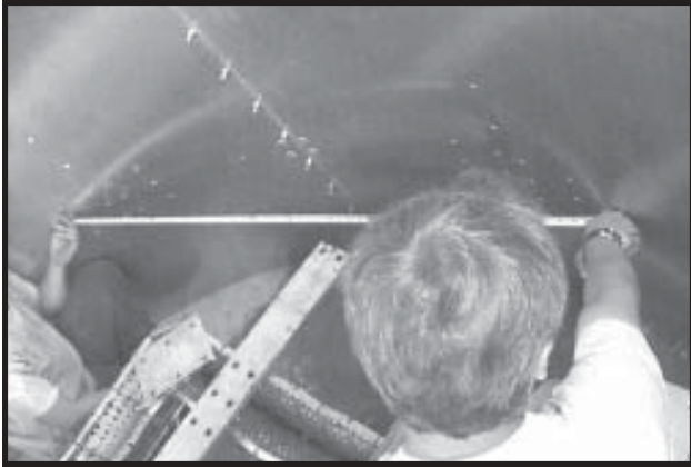
Photo 12-10 Measuring to determine correct knock-outs for bolt holes.
