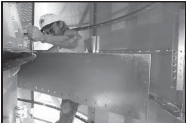
Photo 13-42 Aligning Fan Skirting section to bottom ring of Reducer.
