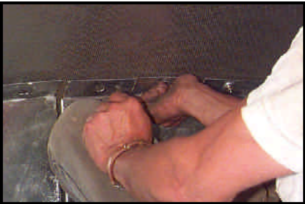
Photo 13-52 Close up - Bolting Outer Divider Hopper to Inside Wall Sheet.
