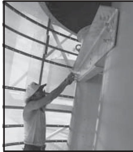
Photo 13-30 Installing top Intermediate Fan Support Beam across (2) Fans.
