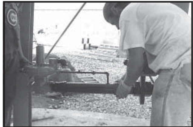
Photo 22-21 Installing Regulator Section.
