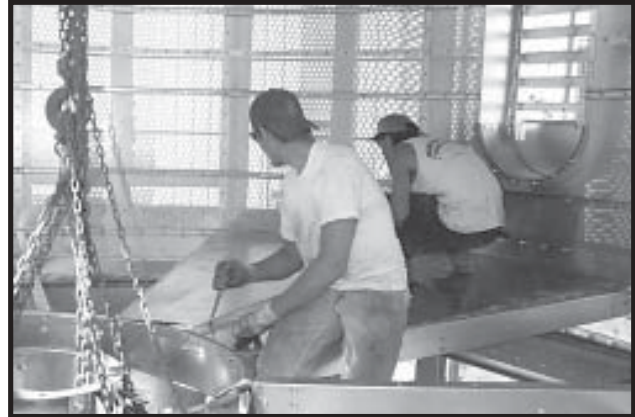
Photo 18-19 Aligning Cool Section Floor Sheets.
