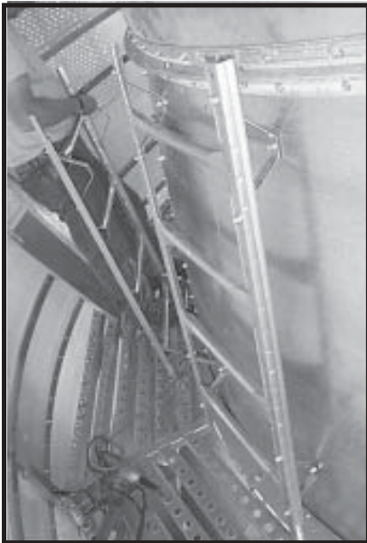
Photo 9-12 First 44" Formed Ladder Section installed to Reducer Housing.
