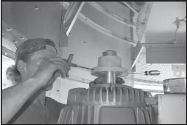
Photo 14-15 Tightening set screw on Motor Hub.
