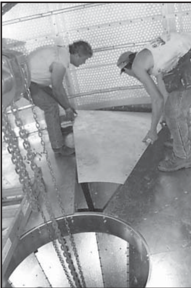
Photo 19-43 Closing Cool Section Floor.
