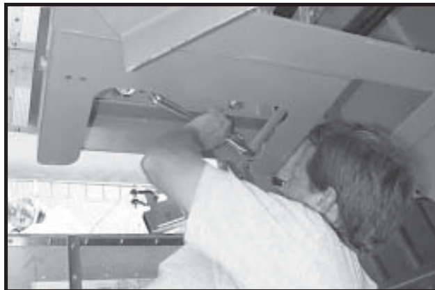
Photo 14-28 Tightening adjusting nuts on bottom rod of Motor Mount.
