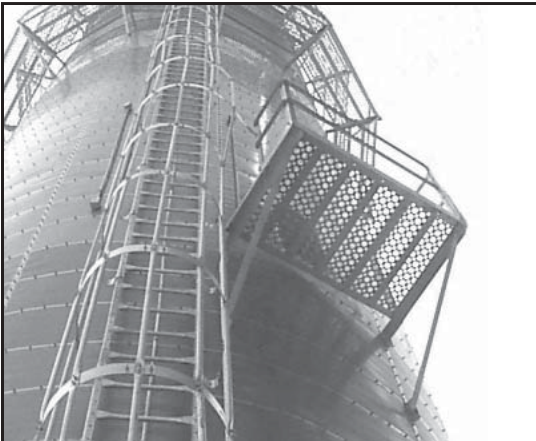
Photo 4-17 Ground View - Ladder with Safety Cage installed through Catwalks and to Platform.
