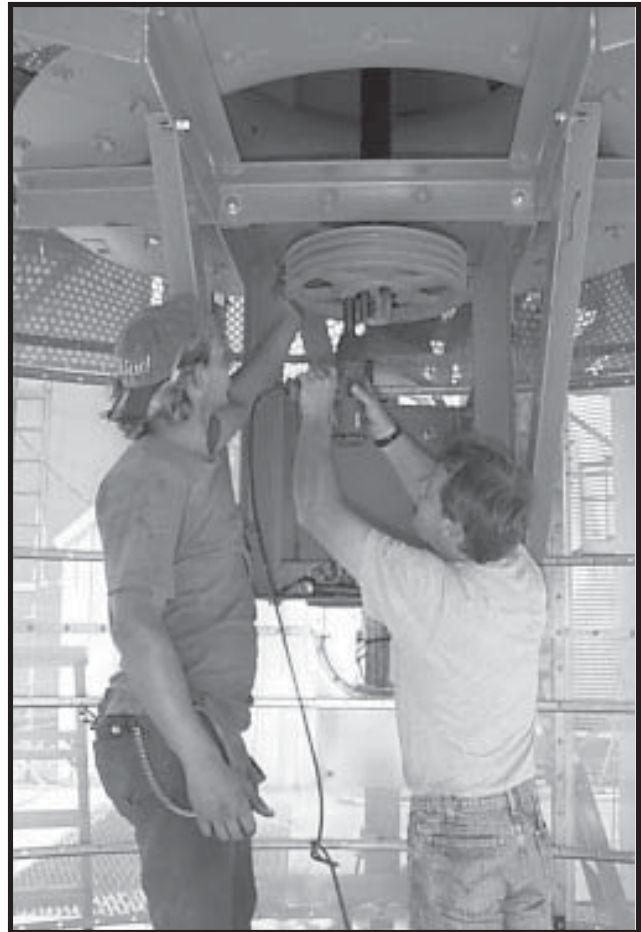
Photo 14-23 Tightening Fan Sheave bolts.
