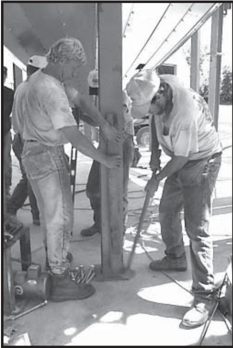
Photo 17-23 Tapping Dryer Legs into position.
