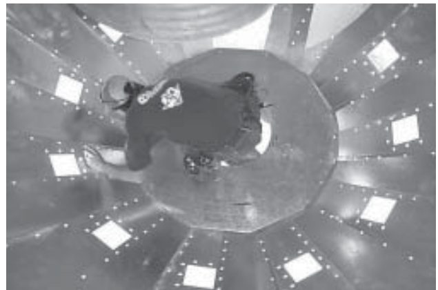
Photo 19-26 Installing Metering Drum Floor to underside of Metering Drum Floor Clips. Check for level.
