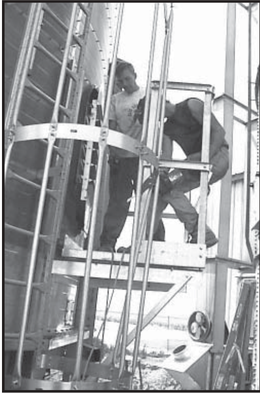
Photo 4-18 Close Up - Installing upper and lower Safety Hoops to Platform Vertical Supports.
