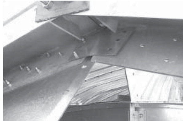
Photo 19-12 In Photo, to demonstrate orientation, Compression Angle Splice (arrow) is temporary bolted to Compression Angles. In actual installation, use common bolt to install Outside Hopper Panels (over Compression Angle Splice) to Compression Angles.
