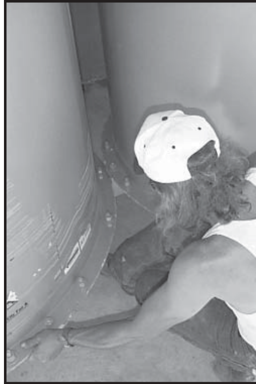
Photo 13-22 Positioning Fans in a cluster with Top and Bottom rings level and touching.
