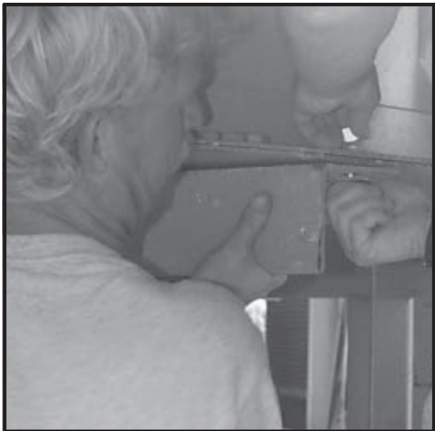
Photo 14-5 Bolting Motor Mount to bottom ring of Fan.
