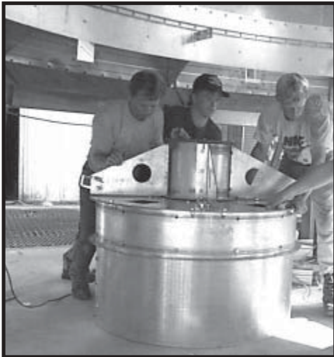
Photo 18-14 Moving Metering Drum into center of dryer (under Cool Section Floor Center Collar).
