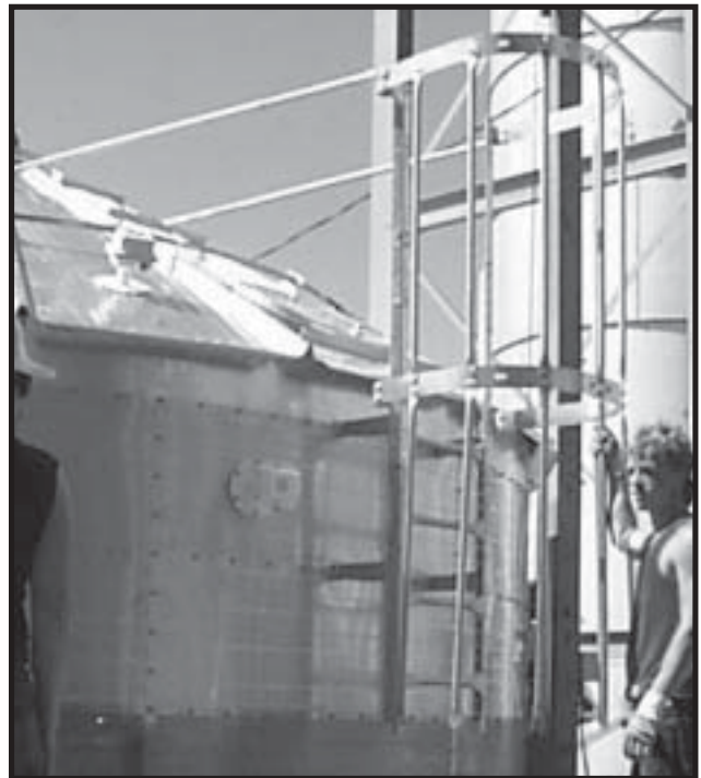
Photo 4-11 Installing Top Safety Cage to Tower Roof.
