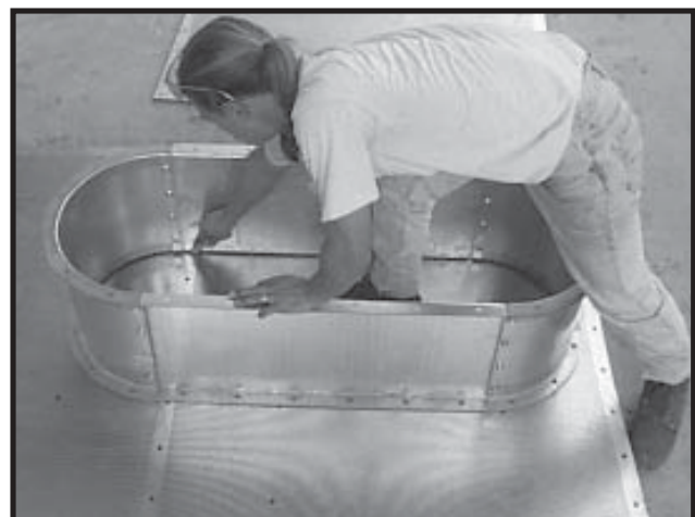
Photo 16-12 Mark around inside perimeter of Window Frame.
