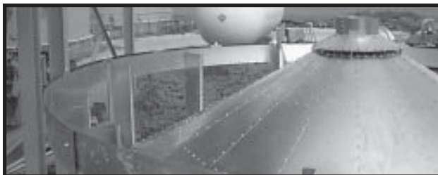
Photo 3-5 Installing Bulb Seal, Eave Clips, and Intermediate Eave Clips to Roof Band.
