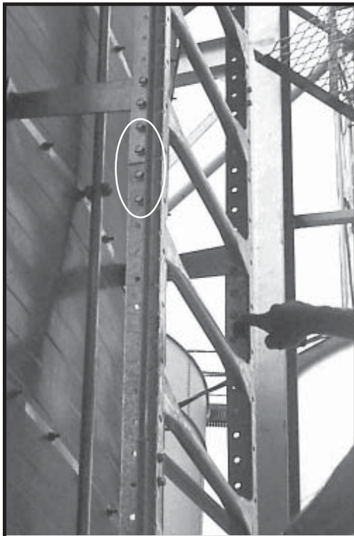
Photo 4-12 Close Up - pointing to Ladder Stiffener Slice. Install Ladder Stiffener Splice with 4 bolts (circle).
