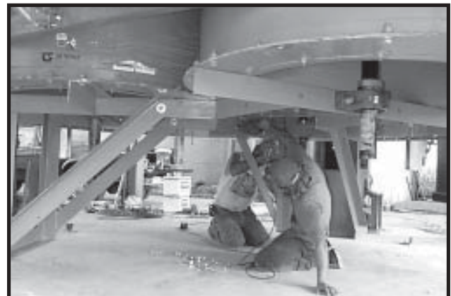
Photo 14-6 Tighting bolts on Fan Motor Mount.
