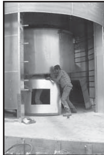
Photo 12-23 Orient Reducer Door Cutout so it faces same Vertical Channel as Heat Section Burner Door.
