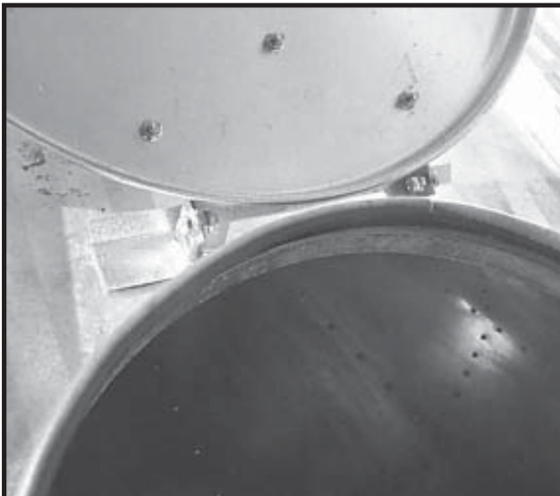
Photo 3-34 Close Up - Access Port Cover installed.
