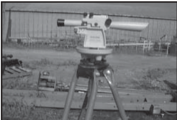
Photo A-5 Level-Transom.
