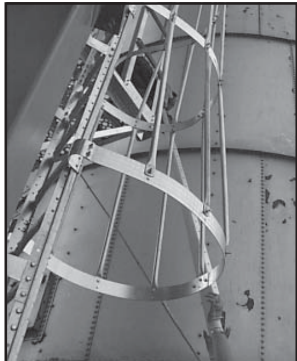
Photo 4-22 Bell Safety Cage installed.
