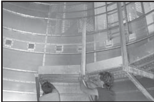
Photo 8-21 Installing Inside Catwalk.
