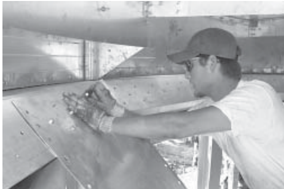
Photo 19-13 View from above - Bolting Outside Hopper Panels over Compression Angles and Compression Angle Splices.
