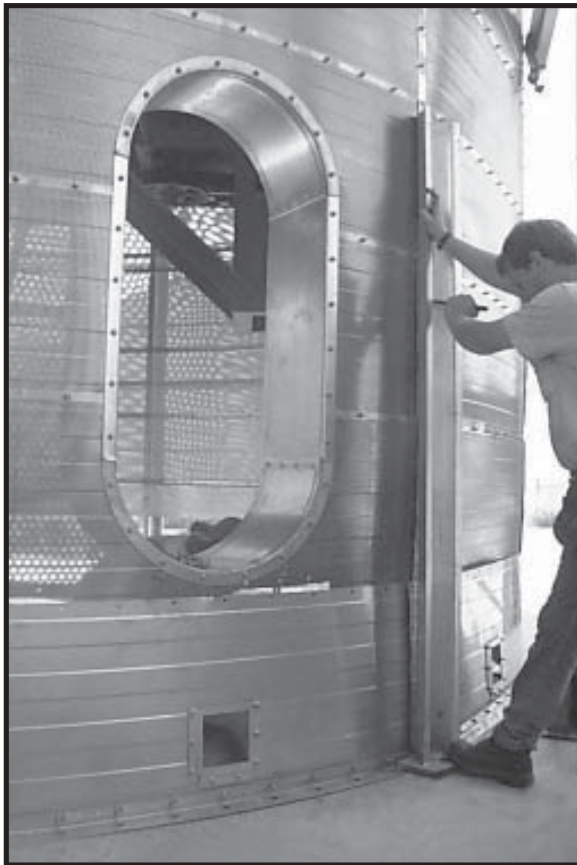
Photo 17-6 Positioning Base Stiffener Weldment flush over Vertical Base Channel (that is under Outside Solid Wall Sheets).
