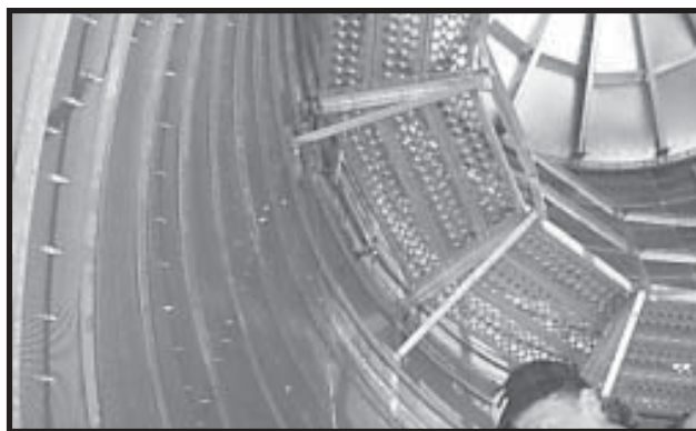
Photo 8-27 View from below - Inside Catwalk installed. (Inside Catwalk Door is closed.) (Ladder is not complete.)
