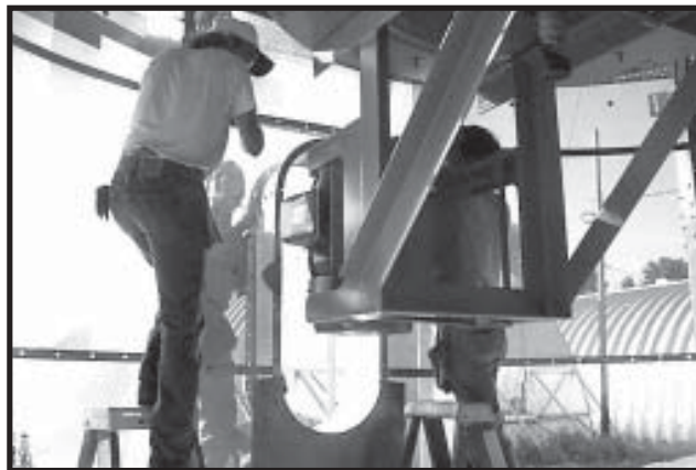
Photo 16-29 Inside View - Window is centered on Fan.
