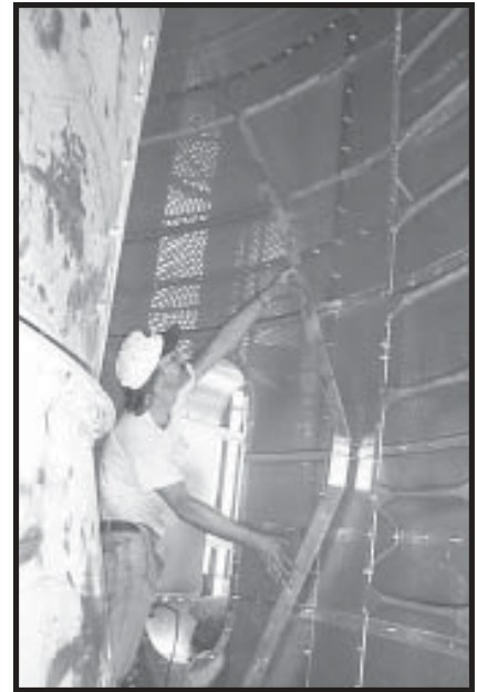
Photo 16-41 Installing 3" wide Heat Section Door Sleeve.
