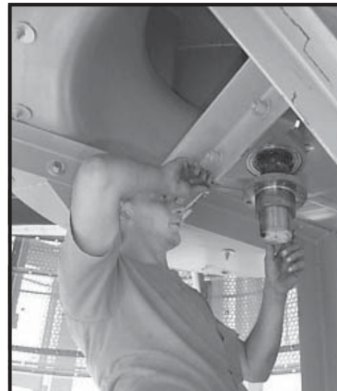
Photo 14-20 Tightening set screw on Fan Hub.
