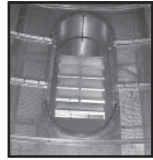
Photo 16-35 Installed 24” Louvered Window, with louvers open.
