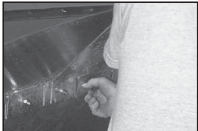
Photo 12-9 Close up inside Burner Housing - Installing Burner Housing Outlet Baffle to top rim of Burner Housing.
