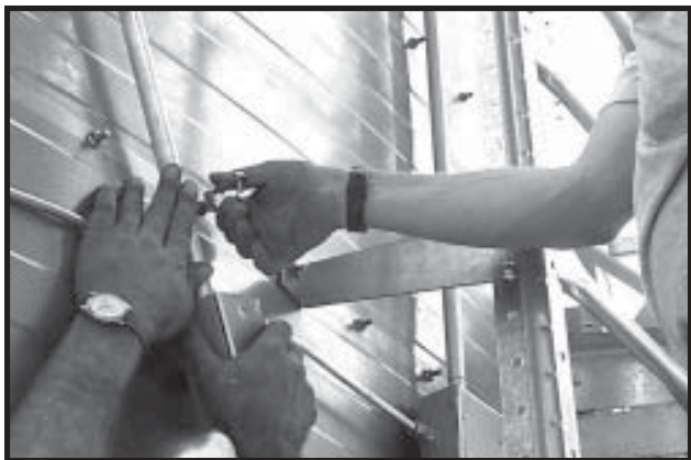
Photo 5-24 Close Up of LH-Bottom RTD - securing conduit near sensor with 1/2" conduit hanger on existing bolt on seam.
