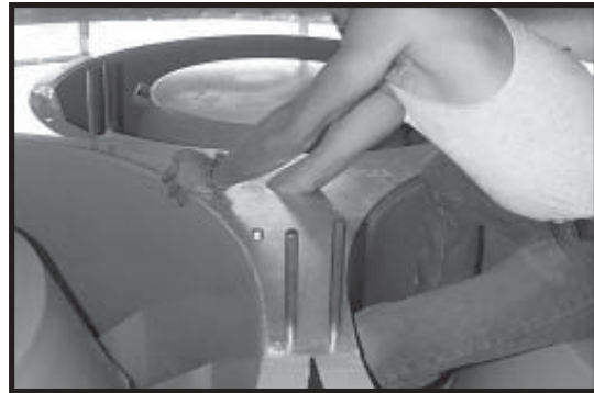
Photo 13-25 Bolting Fan Housing Splice, centered on top of Fan cluster.
