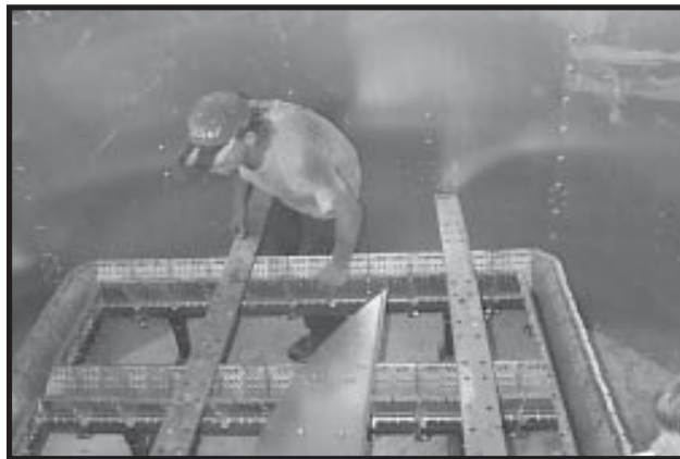
Photo 12-6 Moving Burner, Burner Baffles and other parts inside Burner Housing.
