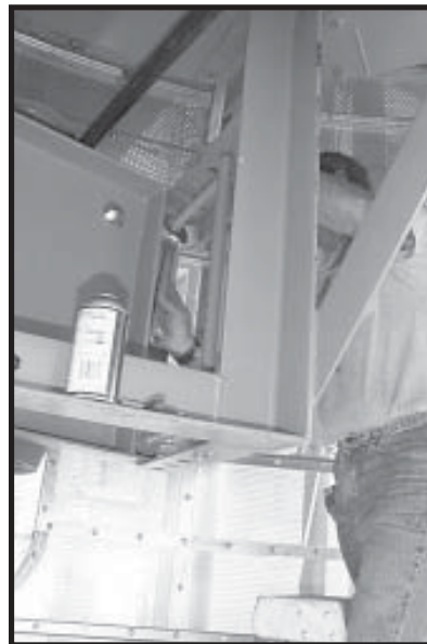
Photo 14-27 (To tighten Fan Belts) tightening adjusting nuts on top rod of Motor Mount.
