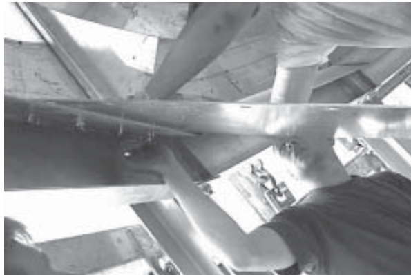
Photo 19-14 View from below - Bolting Outside Hopper Panels over Compression Angles and Compression Angle Splices.
