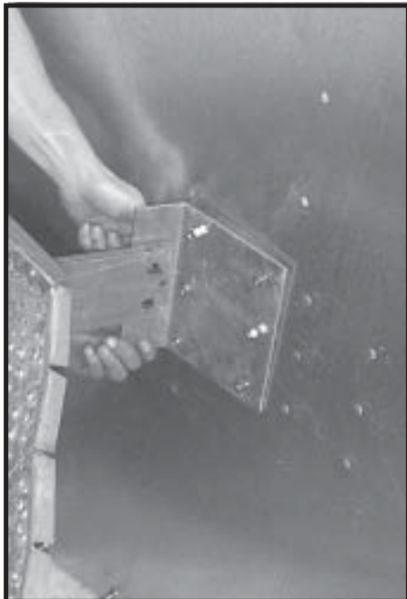
Photo 12-16 Close up - Installing Burner Support Bracket to Burner Mounting Bracket.
