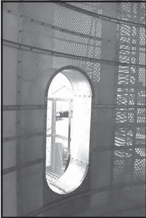
Photo 16-30 18" Window is installed. (Screening is not yet installed.)
