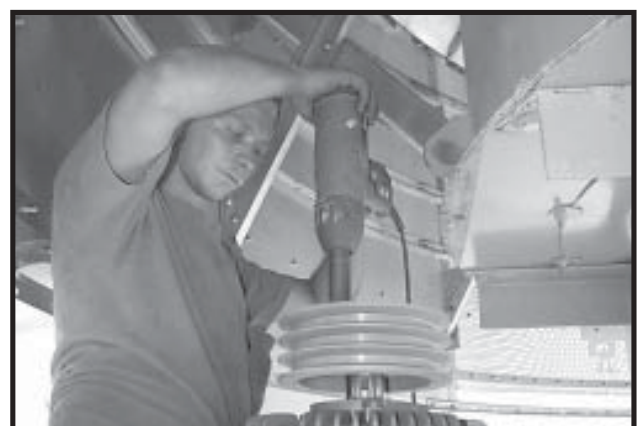
Photo 14-24 Tightening Motor Sheave bolts. Note final tightening of bolts should be with torque wrench.
