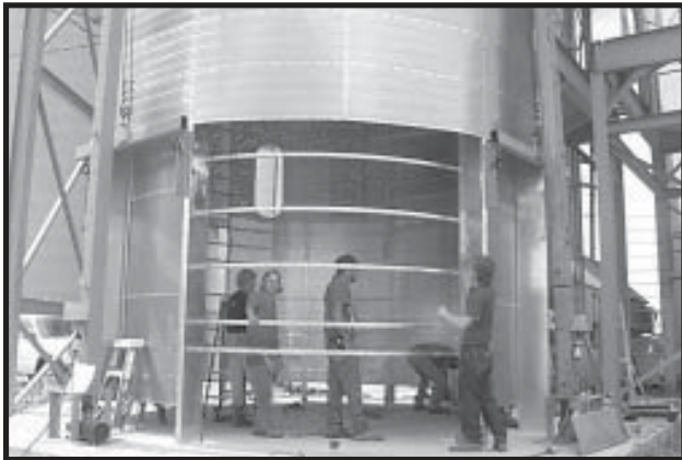
Photo 12-5 Install Rolled Plenum Channels across gap to maintain shape and stability. Remove Rolled Plenum Channels when ready to move burner into dryer.
