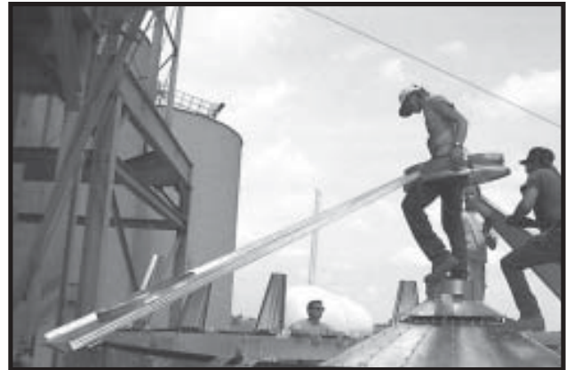
Photo 3-15 Bringing two opposing Tower Roof Sheets to Tower Roof Center Collar. Position Tower Roof Sheet with Access Port cutout directly above where outside ladder will be.
