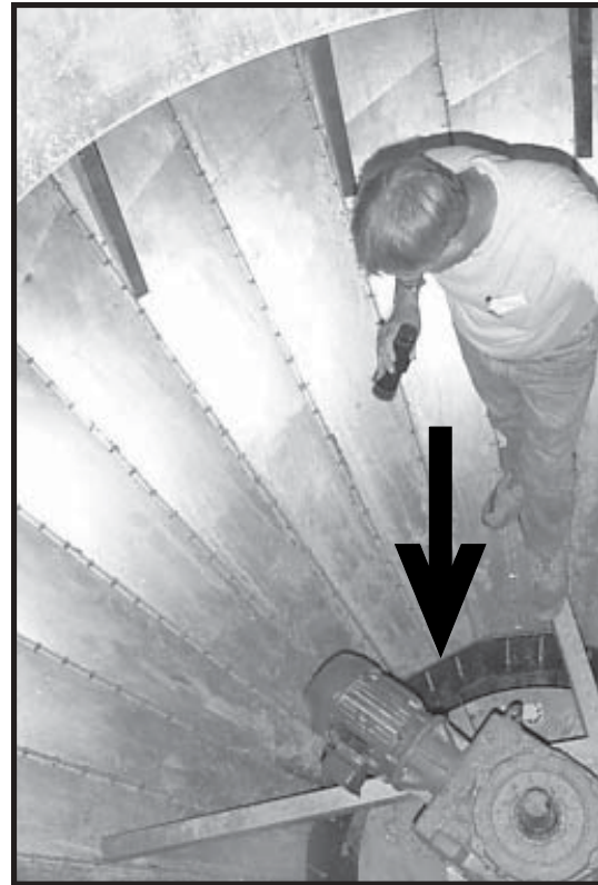
Photo 20-34 Metering Drum Baffles installed (arrow).
