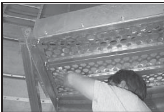
Photo 8-23 Bolting Inside Catwalk Splice Plate to Inside Catwalk Section.
