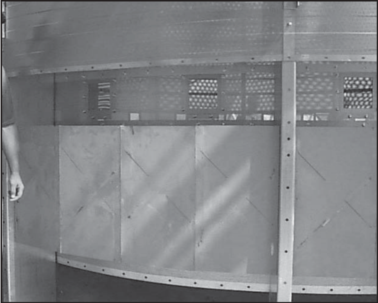
Photo 11-6 Installed Grain Turners.
