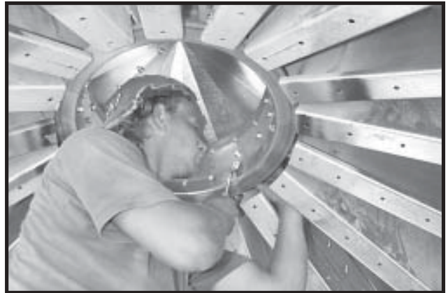
Photo 2-39 Hand tightening Plenum Roof Rafters.
