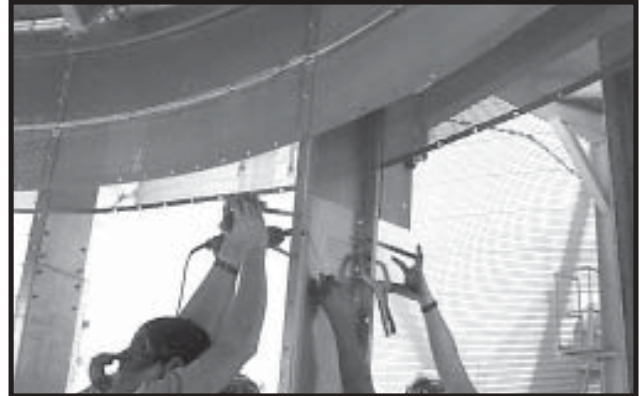
Photo 7-12 Aligning Vertical Channels.
