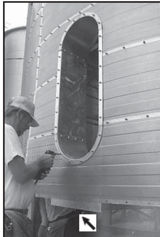
Photo 16-27 Bolt Window Frame to Outside Walls. Note Air Deflector (arrow) is below Window Frame and inside Outside Wall Sheets.
