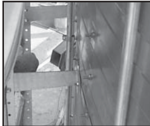
Photo 4-14 Close Up - Outside Ladder Brackets.
