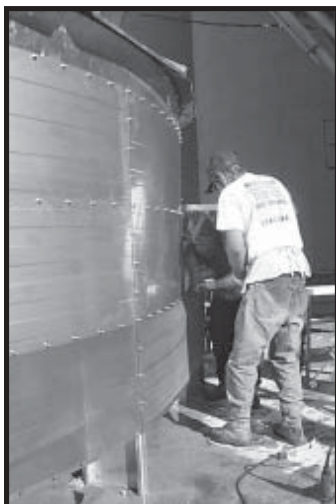
Photo 1-9 Installing Lift Brackets to Outside Wall Sheets of Tower Roof.
