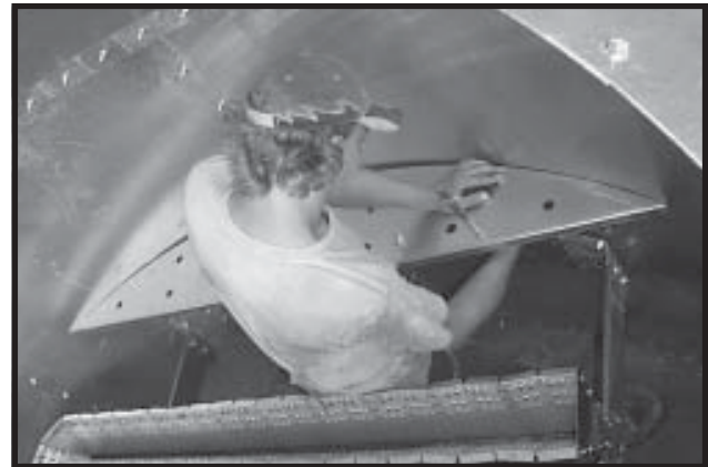
Photo 12-20 Installing Burner Baffles.
