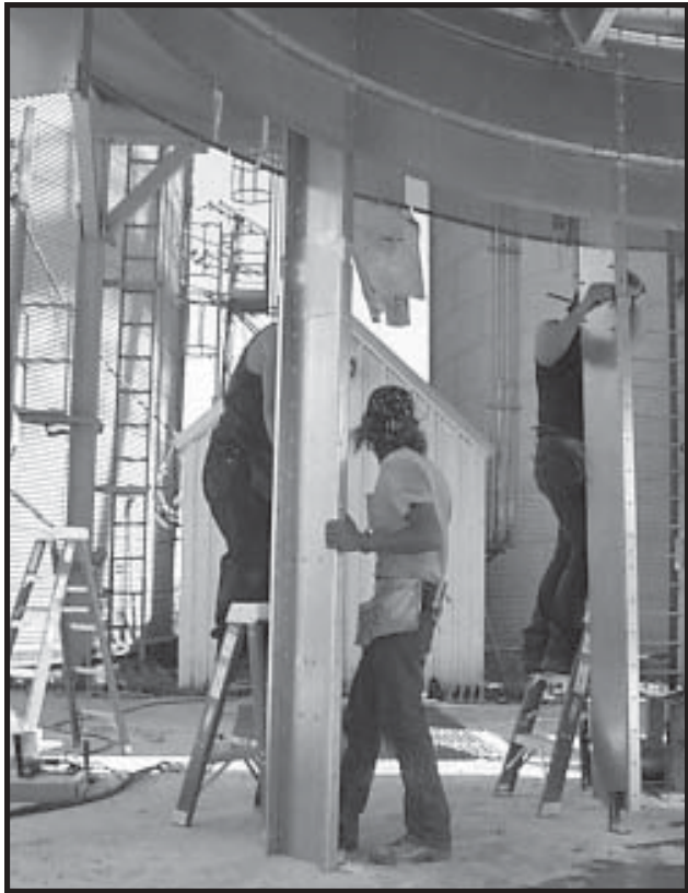
Photo 7-14 Close Up - Bolting Vertical Channels.
