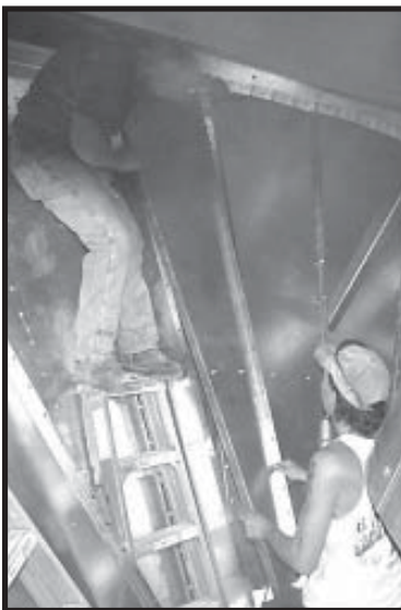
Photo 19-37 Installing Inside Hopper Panels to Hopper Channels.
