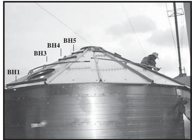
Photo 3-18 Bolt Holes (BH) for Tower Roof Rungs and Expansion Ring Clips.
