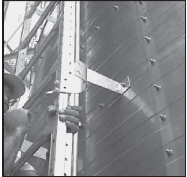
Photo 4-13 Outside Ladder Bracket bolts through 44" Formed Ladder Sections and Outside Ladder Stiffener.
