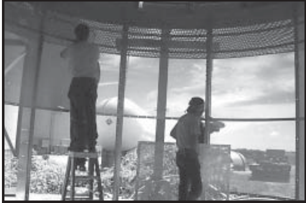
Photo 1-5 Hanging Inside Wall Sheets.
