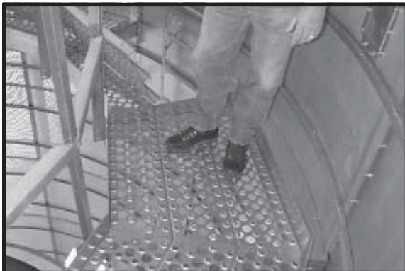
Photo 8-26 View from above - Inside Catwalk Door open.
