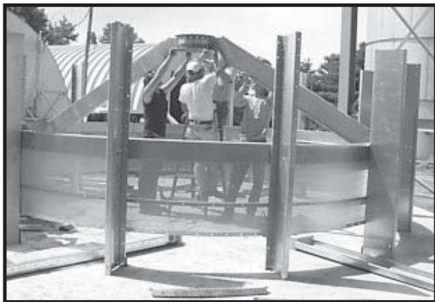
Photo 2-23 Bolt first pair of Plenum Roof Rafters to Plenum Roof Center Collar in center of dryer.
