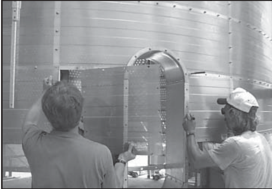
Photo 16-25 Fit Outside Wall Sheets to Window Frame.
