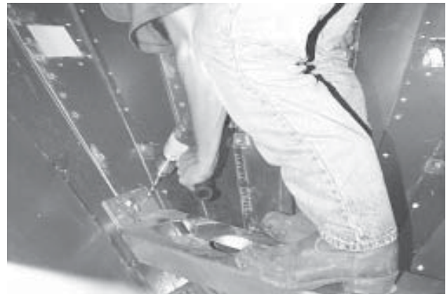
Photo 19-24 Drilling (2) outside bolt holes at each end of Metering Drum Bearing Support. Note center bolt hole (arrow) is bolted with common bolt to a flat edged Outside Hopper Panel seam. Check for level.
