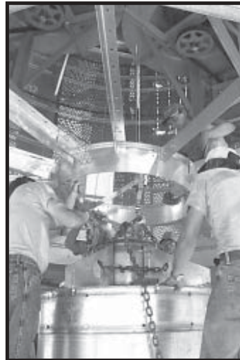
Photo 18-15 Securing Metering Drum for hoisting.
