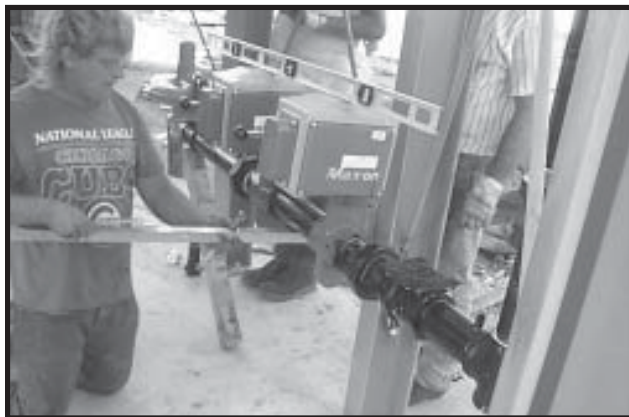
Photo 22-22 Checking Fuel Train is level, then measuring for Fuel Train stands.
