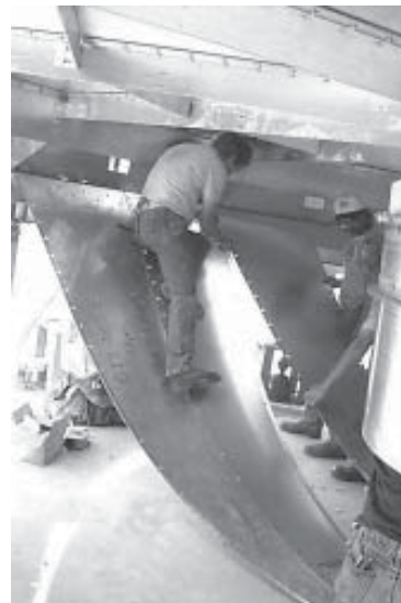
Photo 19-16 Aligning Outside Hopper Panels.
