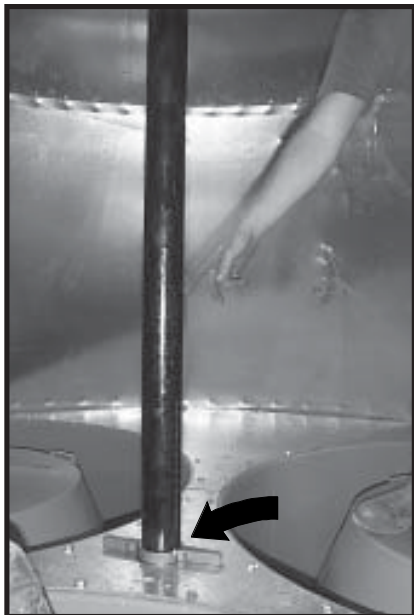
Photo 21-11 Installed Fuel Pipe exits Heat Section through pre-cut hole in center of Fan Housing Splice (arrow).
