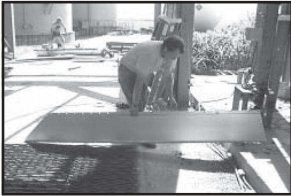
Photo 19-29 Bringing Hopper Channels (RH/LH) into dryer through opening in Cool Section Floor.
