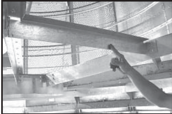
Photo 18-12 Cool Section Floor Crossbeam snug bolted between Cool Section Floor Beams.
