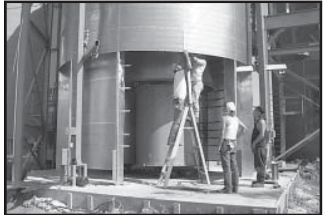
Photo 13-20 Re-installing Vertical Channel after Fans are inside dryer.
