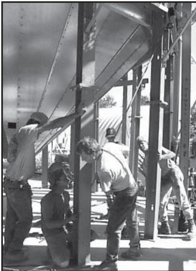
Photo 17-34 Installing X-Bracing Rods to Dryer Legs.
