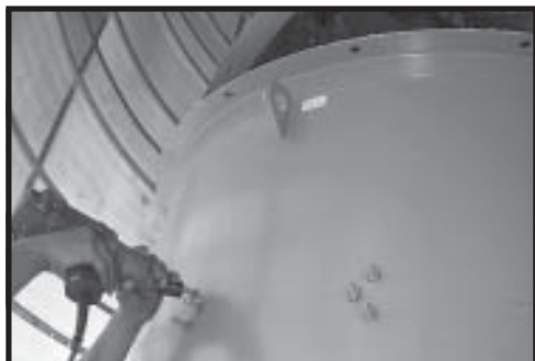
Photo 13-29 Use existing bolts on Fans to install Intermediate Fan Support Beams and some Fan Cross Beam Clips.
