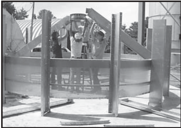
Photo 2-22 Bring first pair of Plenum Roof Rafters together to Plenum Roof Center Collar in center of dryer
