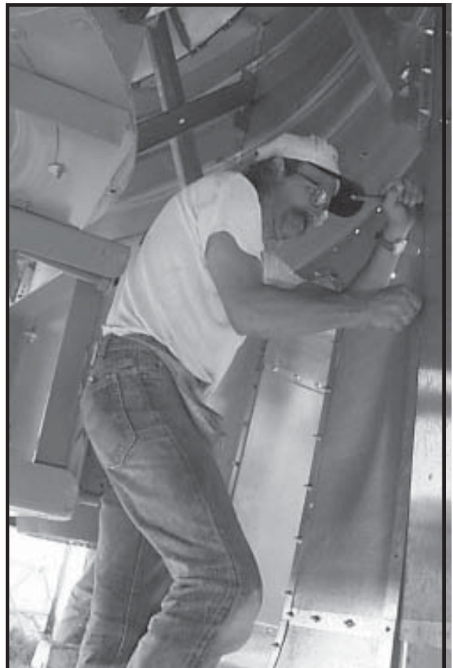
Photo 16-20 Bolt Wall Sheets in place. Install Rolled Plenum Channels. Check that Window Frame is level and square to dryer.
