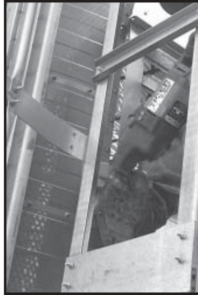
Photo 4-16 Close Up - Securing Safety Hoop to Vertical Support.
