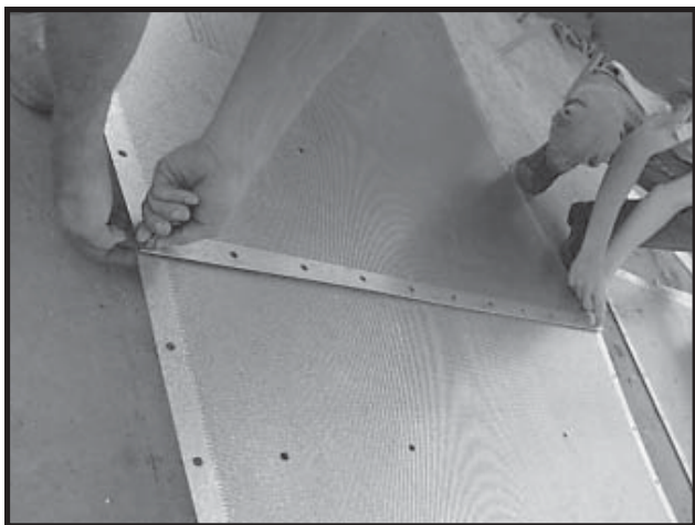
Photo 16-9 Temporarily snug bolt corners of two Wall Sheets.
