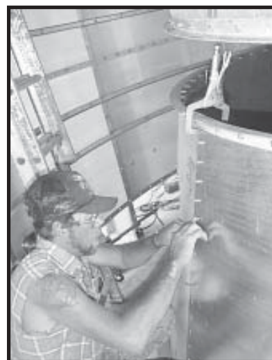
Photo 12-24 Bolting halves of Reducer together.
