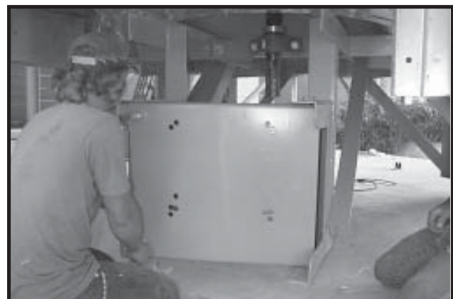
Photo 14-7 Fan Motor Mount installed.
