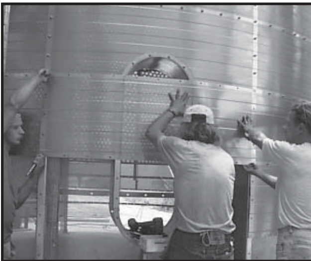
Photo 16-23 Mark Outside Wall Sheets so they will fit inside Window Frame.
