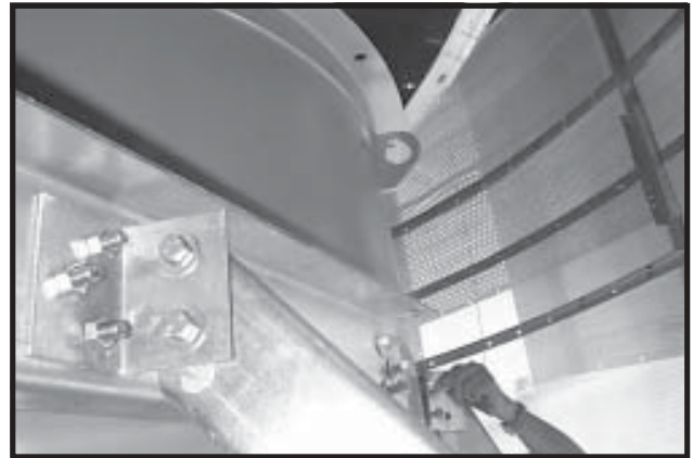
Photo 13-34 Top of Fan - Installing Fan Crossbeam to Fan Crossbeam Clip.
