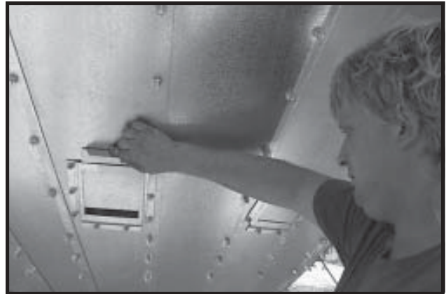
Photos 10-7 Installing Slide Gate Plate to frame on Outside Hopper Panels. (For emergency discharge.)
