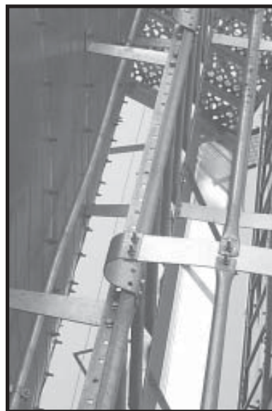
Photo 4-10 Close Up - Shaft of bolts point out of safety cage so climbers do not snag.
