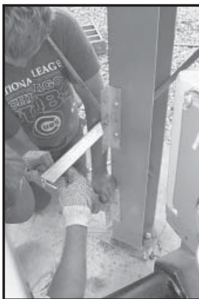
Photo 22-24 Close up - Bolting Fuel Train Stand.
