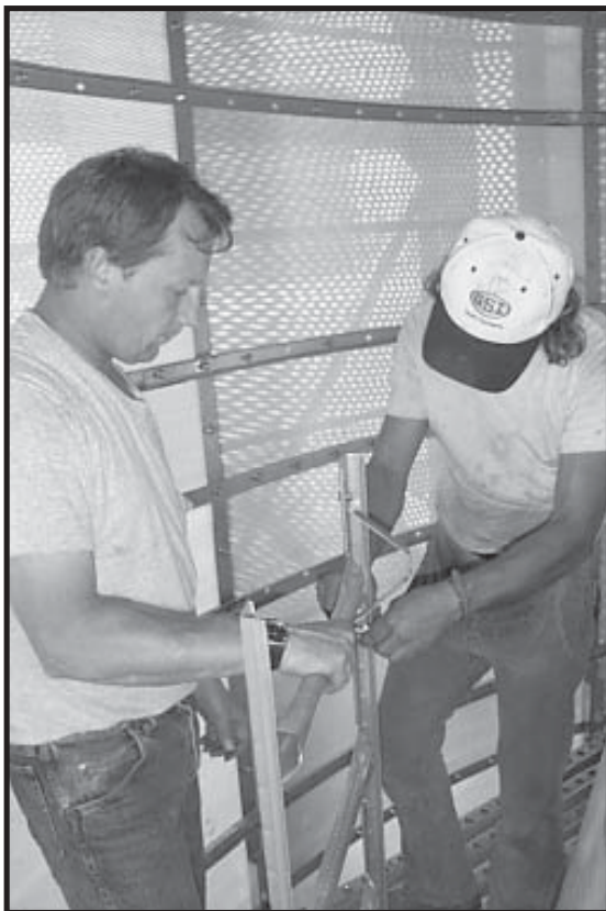
Photo 9-11 Bolting Inside Ladder Standoff to 44" Formed Ladder Section.
