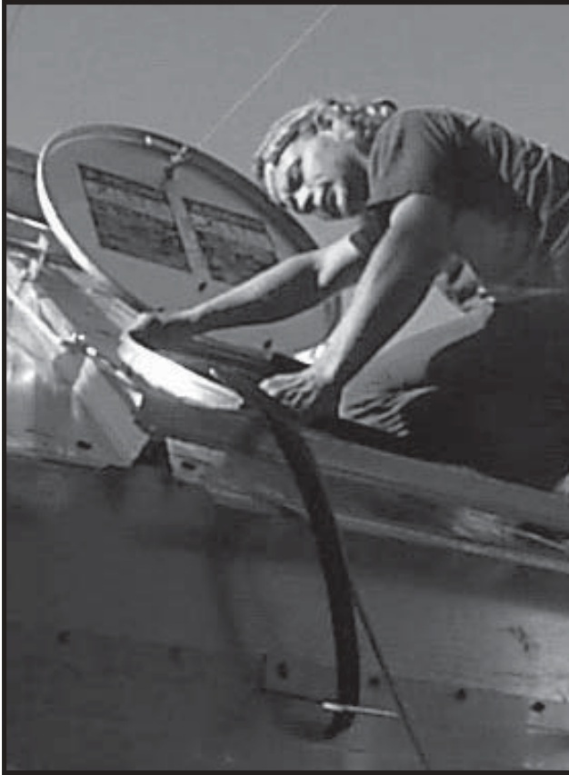
Photo 3-33 Pressing pre-cut Bulb Seal on rim of Access Port cutout on Tower Roof Sheet.
