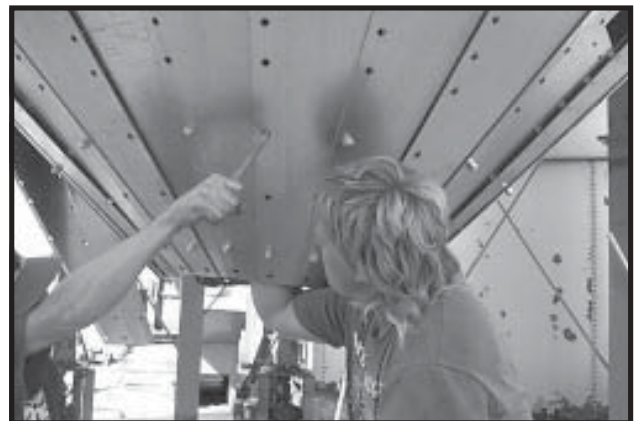
Photo 19-22 Aligning Outside Hopper Panels before installing Hopper Discharge Weldment.
