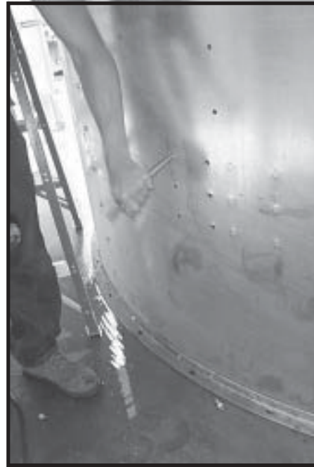
Photo 12-11 Knocking out bolt holes for Burner Mounting Bracket.
