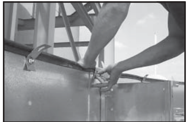
Photo3-8 Installing Eave Clip and Intermediate Eave Clips.
