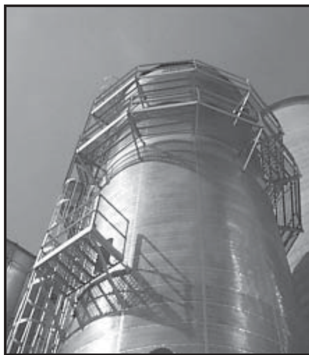
Photo 8-17 Completed Outside Catwalks.
