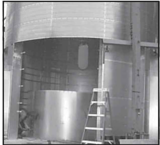
Photo 12-7 Bolting together halves of Burner Housing.
