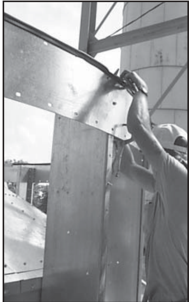
Photo 3-4 Pressing Bulb Seal over top of Roof Band.
