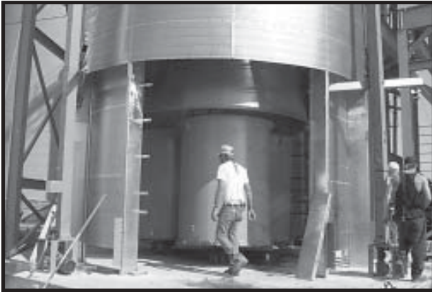
Photo 13-19 Three Fans form a cluster inside dryer.
