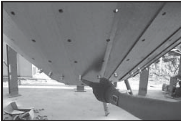
Photo 19-21 Important - After all Outside Hopper Panels are in place, secure against wind with temporary bolts, especially overnight.
