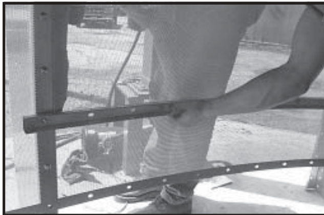
Photo 1-7 Close Up - Installing Rolled Plenum Channels.
