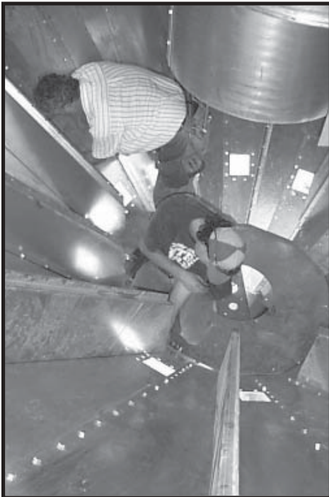
Photo 19-31 View from above - Installing RH and LH Hopper Channels to bracket each other.
