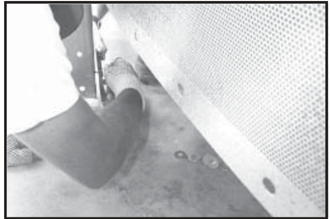
Photo 7-16 Bolting Vertical Channel to Jig Clip.
