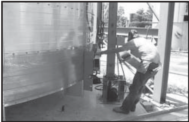
Photo 7-6 Positioning jack next to dryer.
