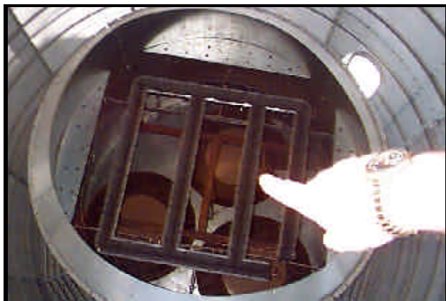
Photo 13-61 Aerial view - Completed installation of Burner, Reducer, Fans, & Divider Hopper under Reducer Walkway.
