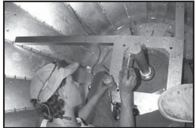
Photo 20-24 Applying anti-seize to top of Metering Drum Drive Shaft before installing Gearbox.
