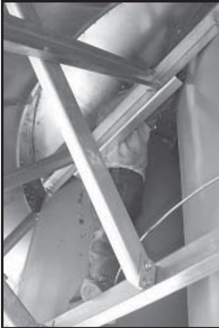
Photo 15-5 Accessing upper Grease Zert.
