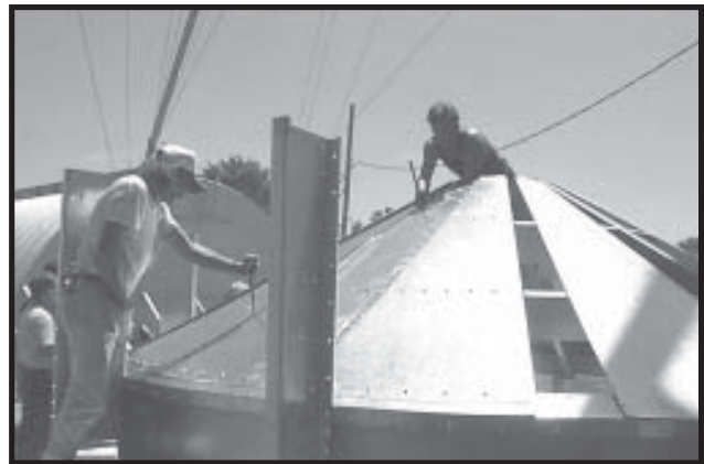
Photo 2-33 Aligning Plenum Roof Sheets.
