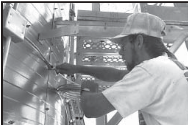
Photo 5-19 Installing copper capillary tubing with Insulated Clips.
