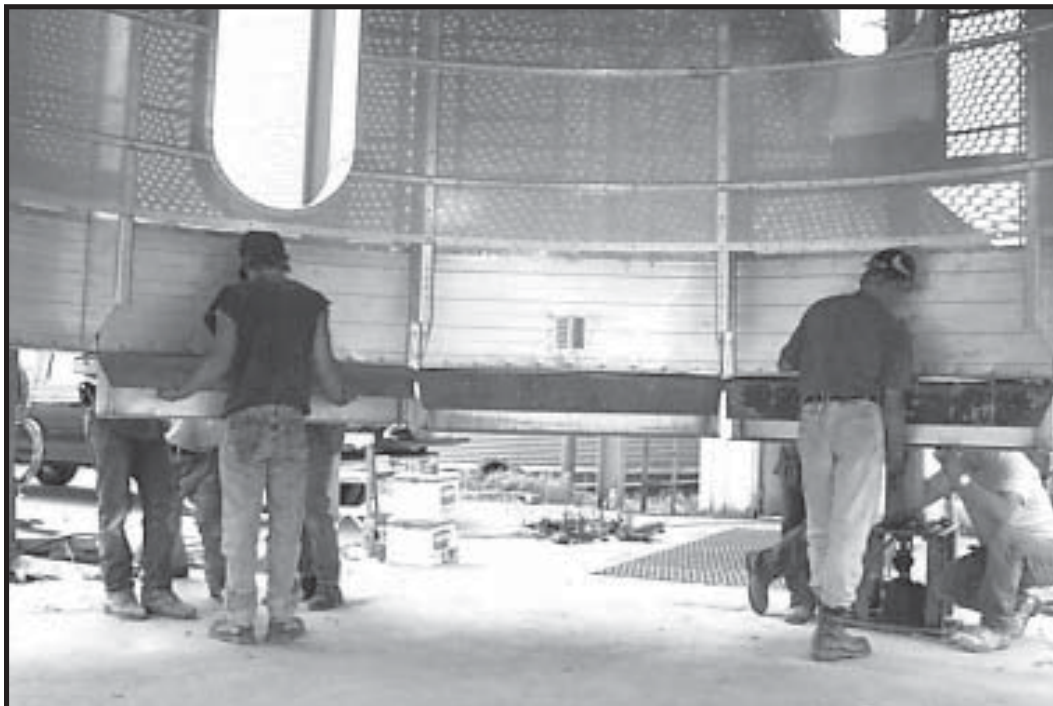
Photo 17-12 Inside View - Installing Compression Angle Weldments. Note Inside Solid Wall Sheet will be installed after Compression Angle Weldment, with one Rolled Plenum Channel in 4th bolt hole.
