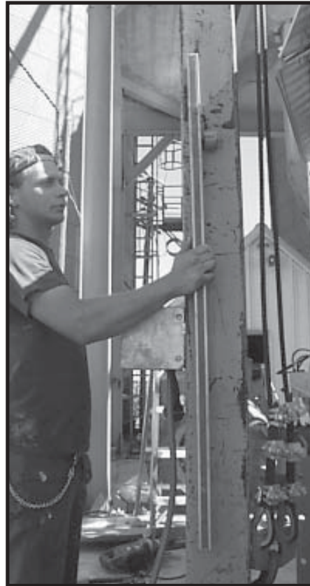
Photo 7-8 Checking jack is plumb and level.
