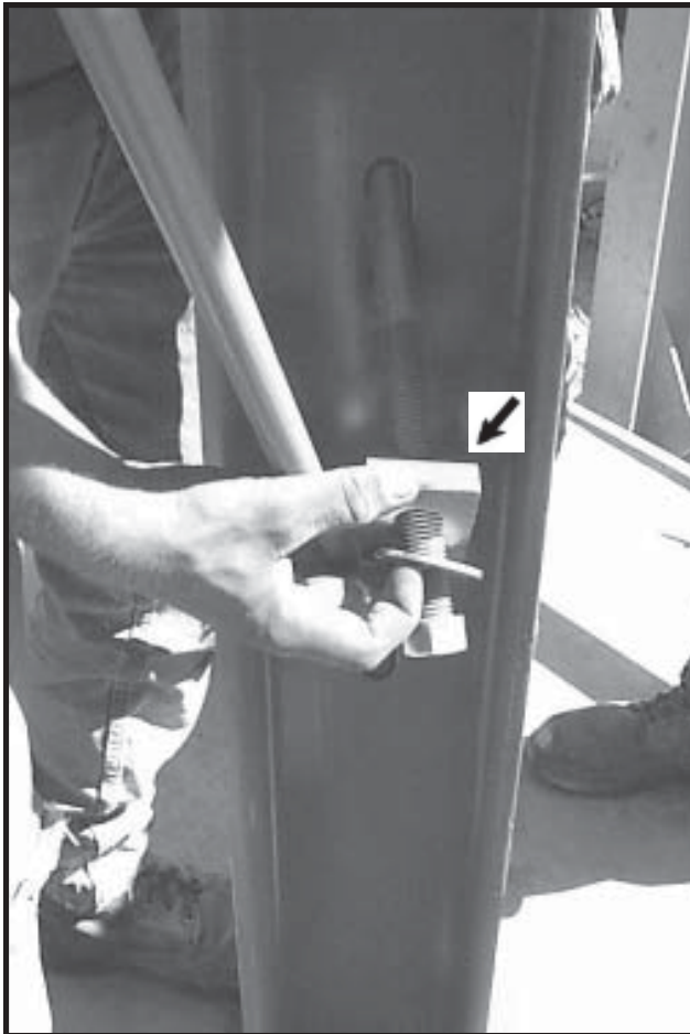
Photo 17-37 Secure X-Bracing Rods with 3/4" nut, 3/4" washer, and cast washer (arrow).
