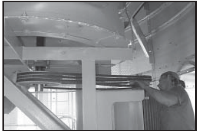
Photo 14-26 Running Fan Belts in grooves on sheaves.
