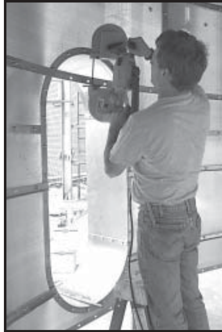
Photo 16-22 Drill and bolt Rolled Plenum Channels, then cut away from Window Frames.
