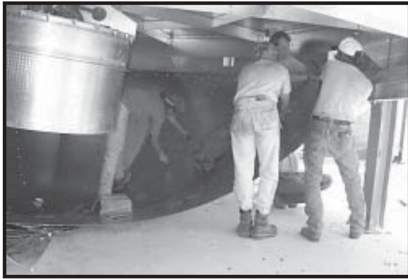
Photo 19-17 While installing Outside Hopper Panels, allow ends to overlap at center of dryer.
