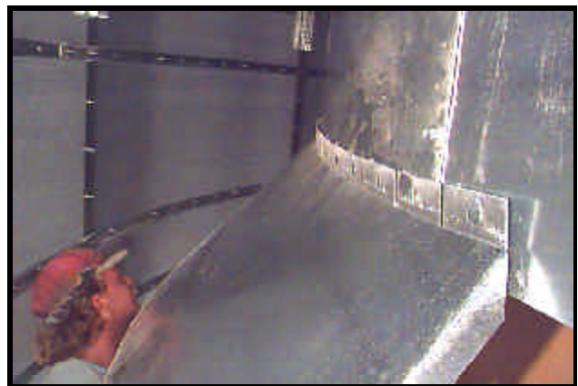
Photo 13-47 Bolting top tabs of Inner Divider Hopper to bottom of Fan Skirting.
