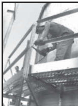
Photo 8-13 Tightening Outside Catwalk bottom Handrail.
