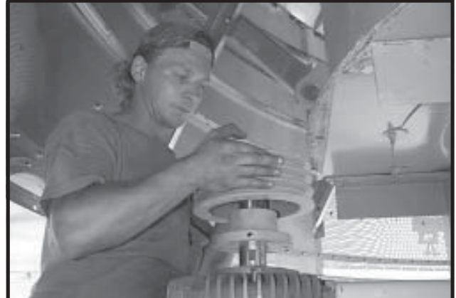
Photo 14-16 Sliding Motor Sheave on Motor Drive Shaft.
