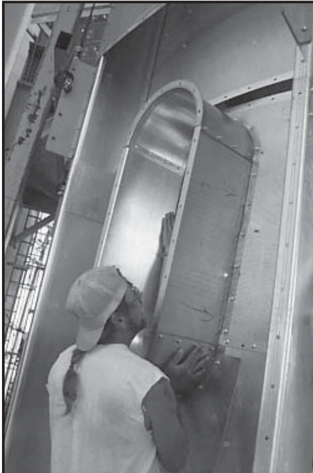
Photo 16-19 Hang Pre-assembled Wall Sheets, Window Frame, and Air Deflector.
