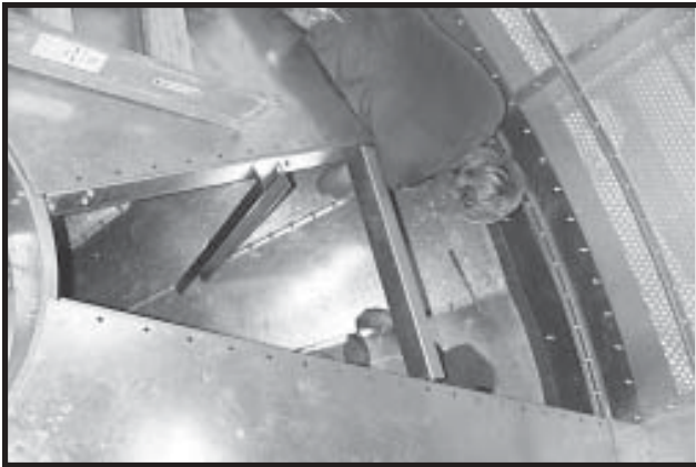
Photo 19-41 View from above - Tightening Inside Hopper Panels.
