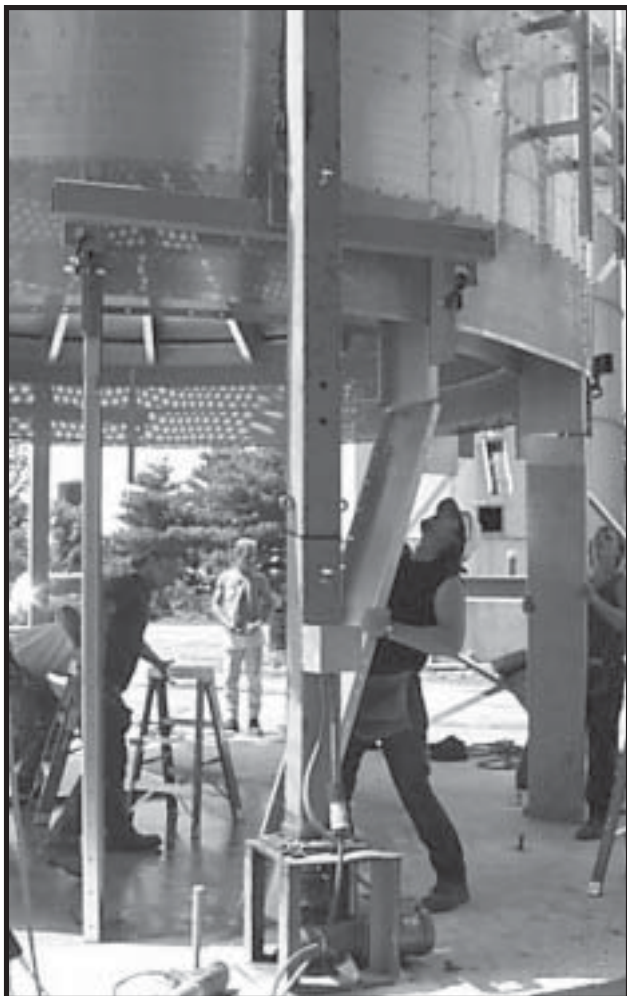
Photo 7-11 Sliding Vertical Channel up to Vertical Channel on dryer.
