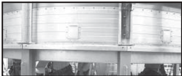
Photos 10-6 Slide Gate installed to Outside Bottom Wall Sheet. (For emergency discharge.)
