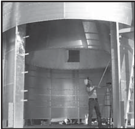
Photo 13-11 Checking clearance for Fan under Reducer/Burner.
