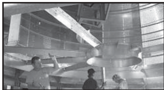
Photo 18-11 Snug bolting pairs of Cool Section Floor Beams to Cool Section Floor Center Collar.
