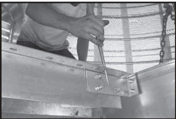
Photo 18-10 Aligning Cool Section Floor Beam Bracket to Cool Section Floor Center Collar.
