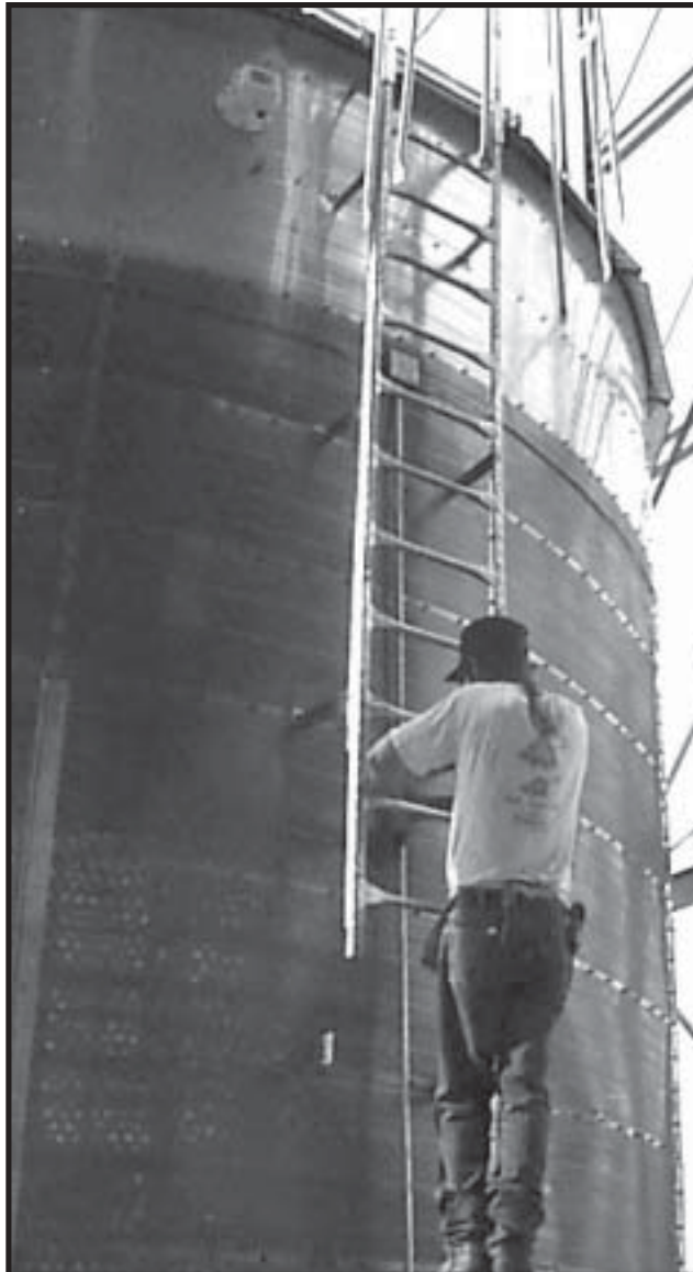
Photo 5-14 Upper Hi-Limit installed with junction box under Outside Ladder (arrow).
