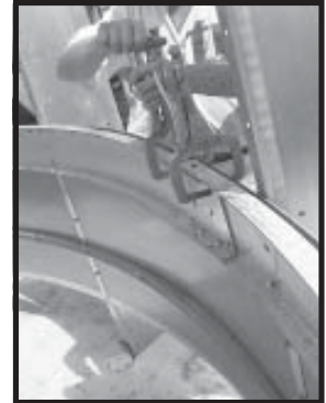
Photo 2-14 Splicing Plenum Eave Channels.
