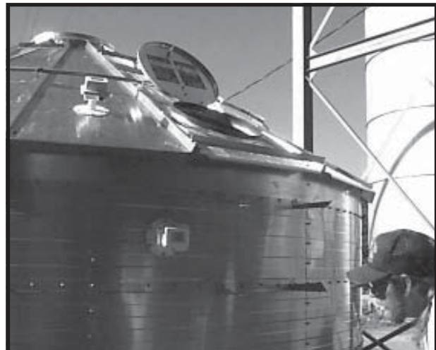
Outside View - access port installed with decals in place.
