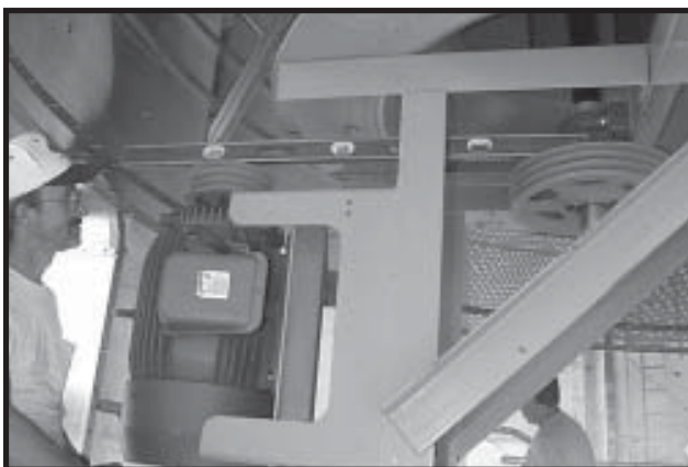
Photo 14-22 Checking top of Motor Sheave is level with top of Fan Sheave.
