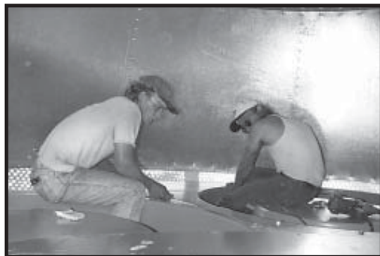
Photo 13-27 Bolting Fan Reducer Panel.
