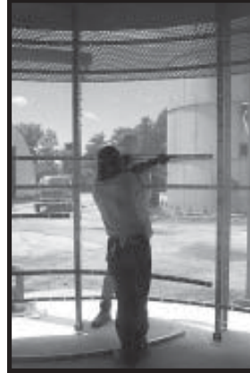
Photo 1-6 Installing Rolled Plenum Channels.
