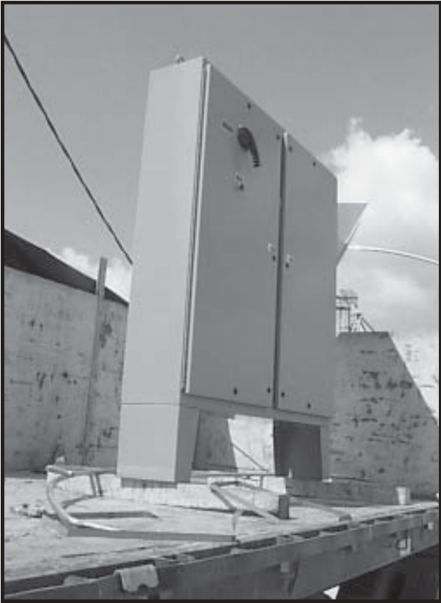
Photo 23-2 Electrical Control System.
