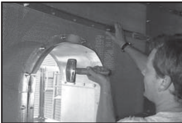
Photo 16-44 Tap hammering Heat Section Door Sleeve around inside of Door Frame.
