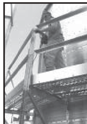
Photo 8-14 Tightening Outside Catwalk top Handrail.
