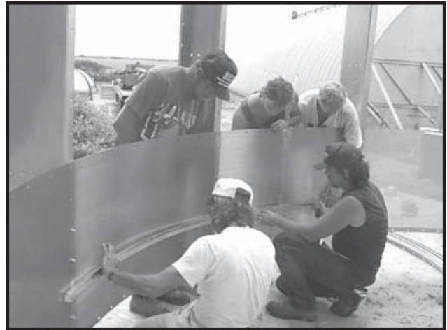
Photo 2-10 Installing Rolled Plenum Channel to Inside Top Wall Sheets.
