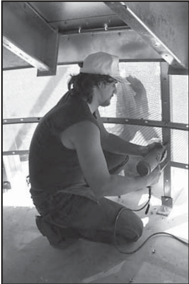
Photo 2-38 Tightening Inside Top Wall Sheets.
