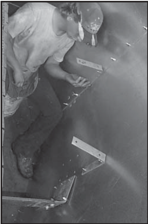
Photo 12-19 Installing Burner Baffle Supports.
