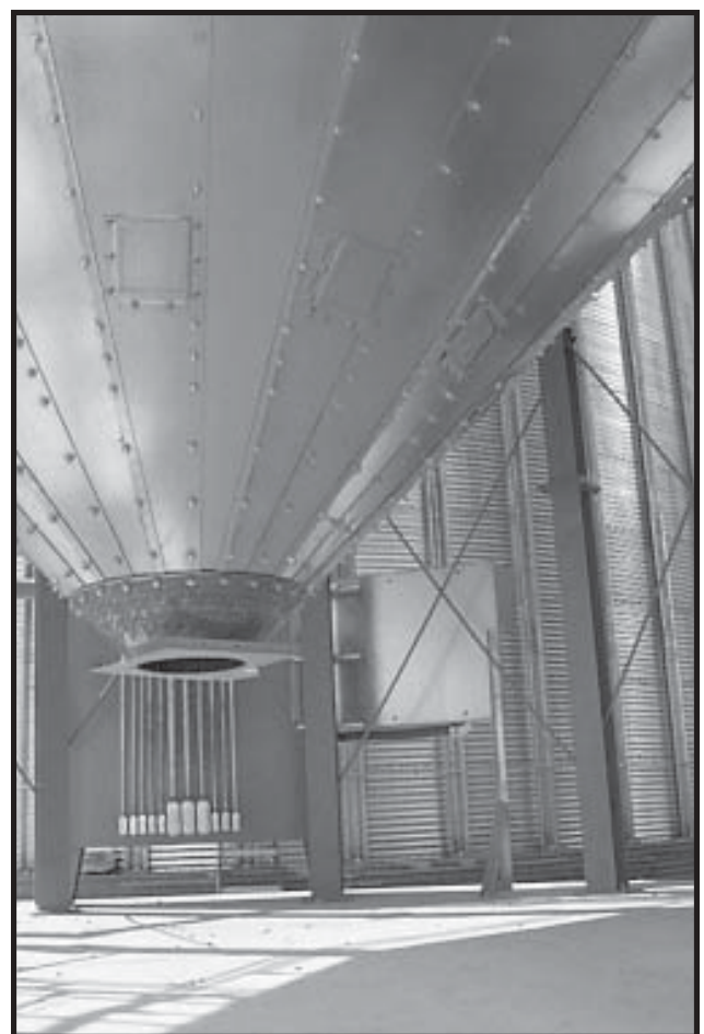
Photo 19-44 Hopper installed with Emergency Discharge Slide Gates (See Step 10, "Slide Gates".)
