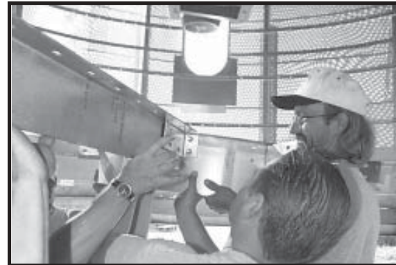
Photo 18-9 Close up - Bringing Cool Section Floor Beam to Cool Section Floor Center Collar.
