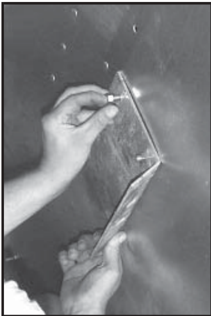
Photo 12-12 View inside Burner Housing - Installing Burner Mounting Bracket.
