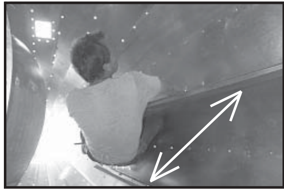
Photo 19-30 View from above - RH and LH Hopper Channels bracket each other (arrow).
