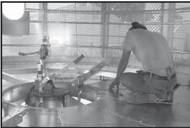
Photo 18-20 Snug bolting Cool Section Floor Sheets.
