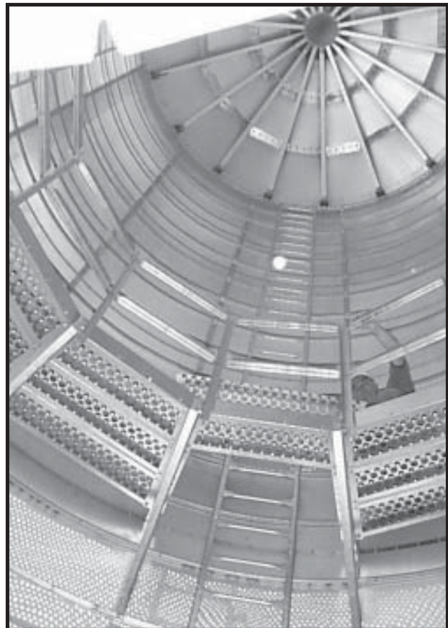
Photo 8-28 View from below - Inside Catwalk installed. (Inside Catwalk Door is open.)
