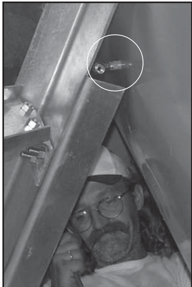
Photo 15-9 Elbow and Brass Compression Union installed to Fan (circled).
