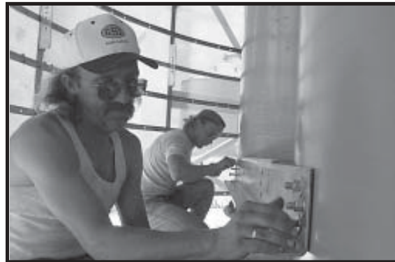
Photo 13-31 Installing bottom Intermediate Fan Support Beam across (2) Fans.
