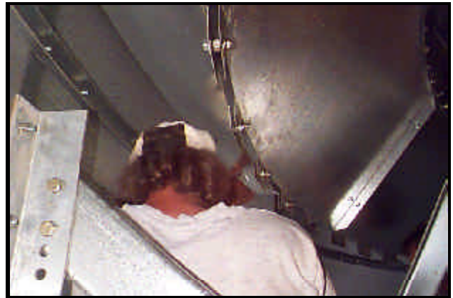
Photo 13-49 Bolting Outer Divider Hopper to Inner Divider Hopper.
