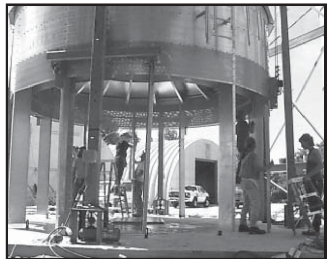
Photo 7-13 Bolting Vertical Channels.
