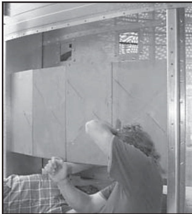
Photo 11-4 Installing middle Grain Turner Sections.
