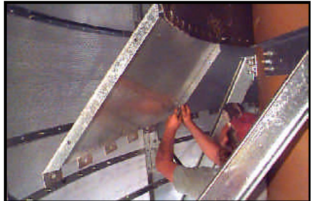
Photo 13-48 Bolting Inner Divider Hopper Sections together.
