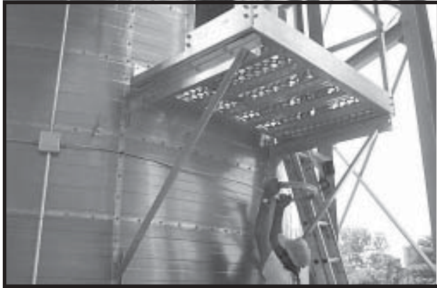
Photo 5-18 Installing Lower Hi-Limit. Note: Outside Ladder will install over Junction Box.
