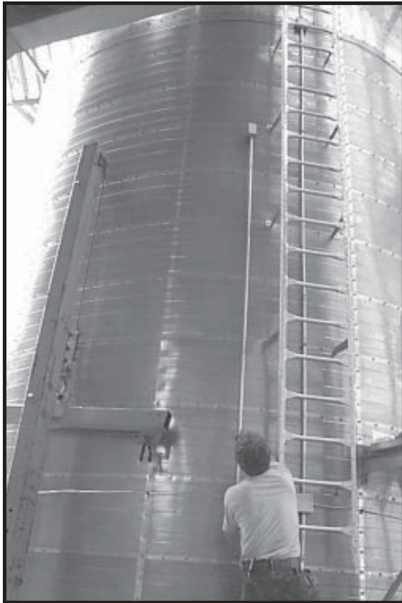
Photo 5-23 Installing LH pair of RTDs.
