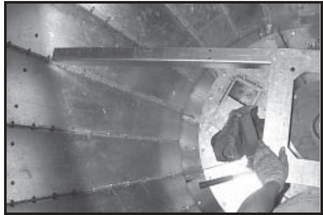
Photo 20-21 Gearbox Torque Arm Assembly installed to Inside Hopper Wall.
