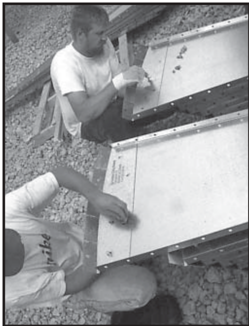
Photo 19-34 Pre-assembling (1) Inside Hopper Flange to each Inside Hopper Panel.
