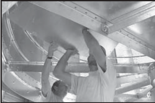
Photo 18-18 View from below - Placing Cool Section Floor Sheets.
