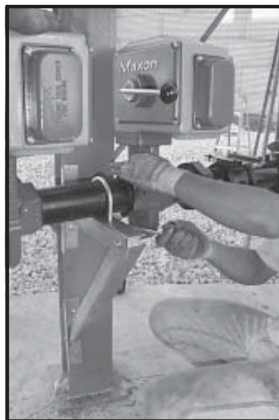
Photo 22-25 Securing Fuel Train to Fuel Train stand with 3" U-Bolt.
