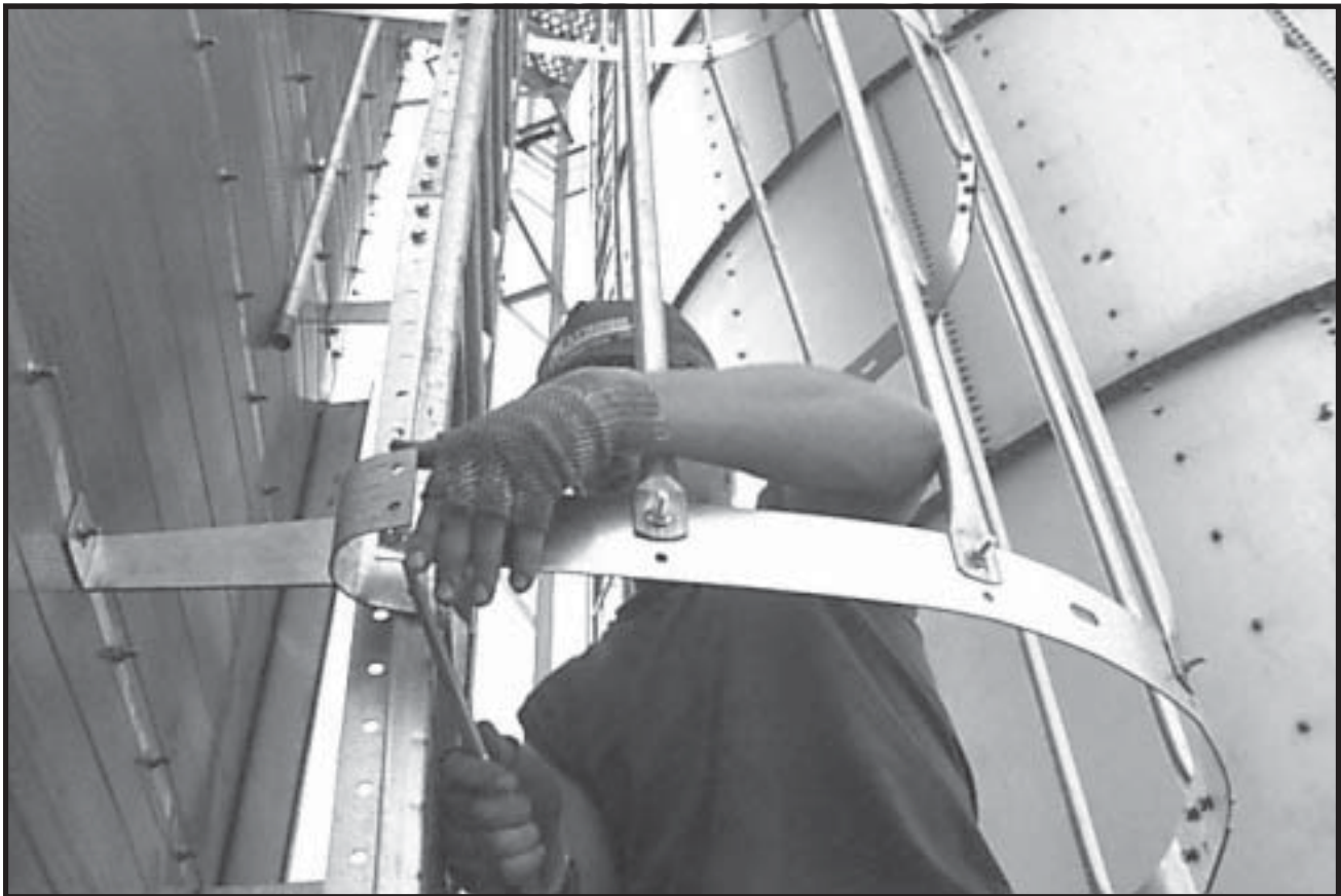
Photo 4-21 Close Up - installing Bell Safety Cage.
