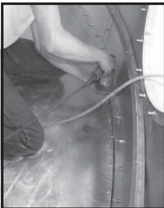
Photo 18-22 Tightening self tapping screws on perimeter of Cool Section Floor.
