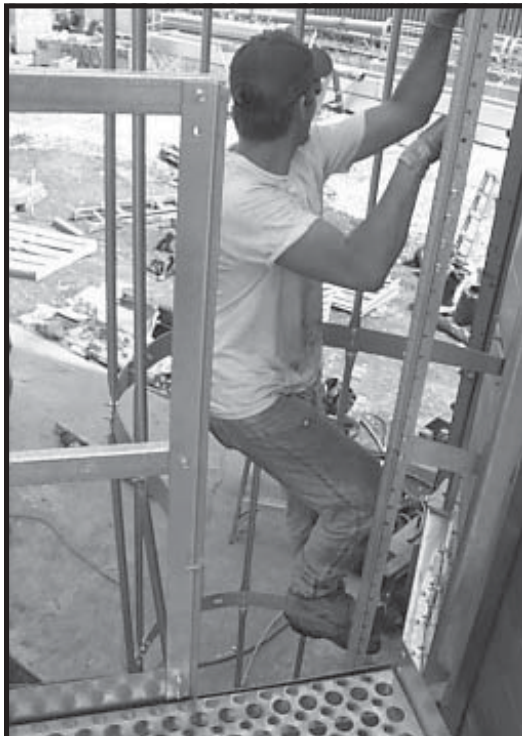
Photo 4-19 View from Platform - Safety Hoops installed to Platform Vertical Supports.
