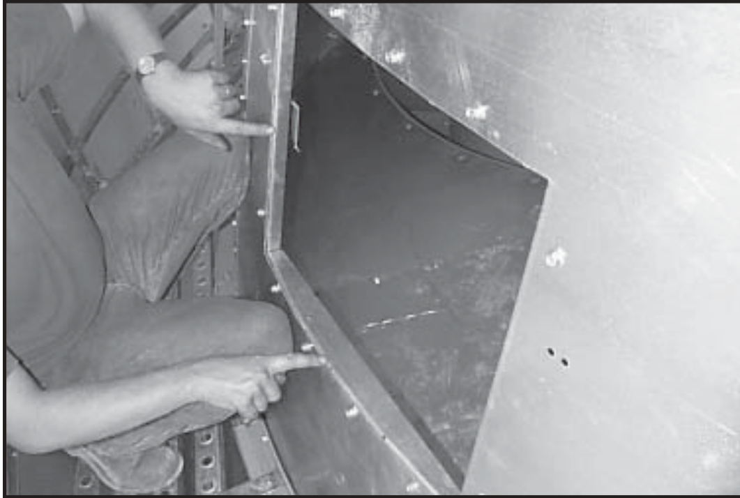
Photo 16-54 Front of installed Reducer Door.
