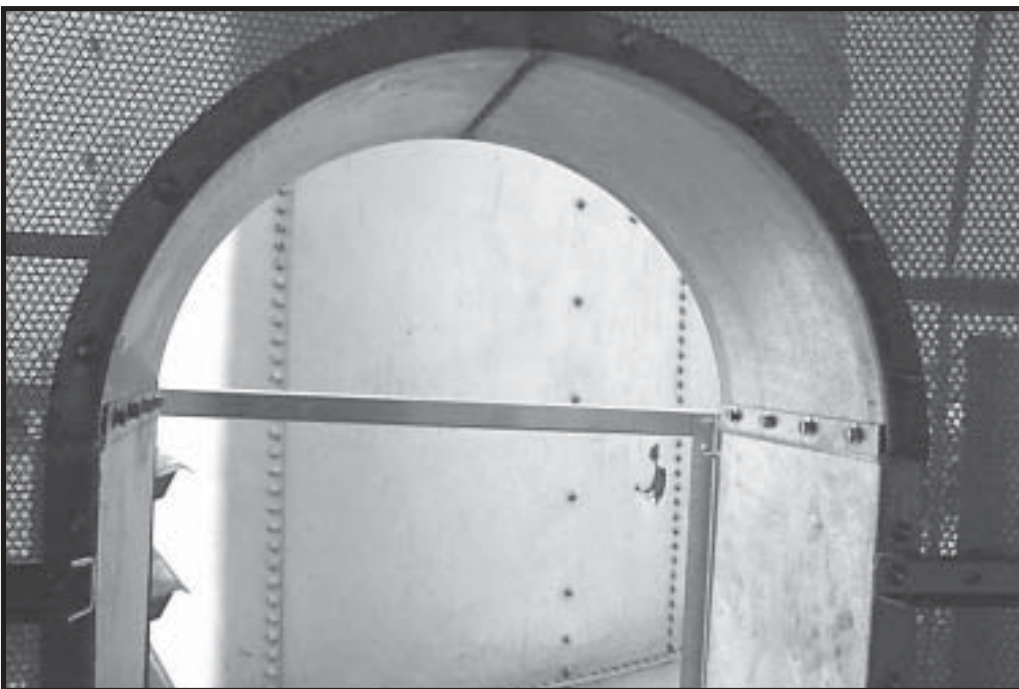
Photo 16-32 Close up - 18" Window installed. (Screening is not yet installed.)
