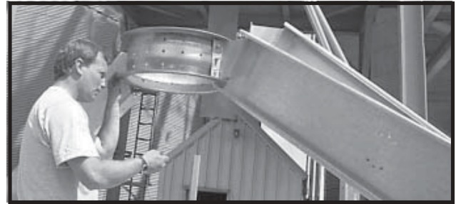
Photo 2-24 Close Up - Bolt top of Plenum Roof Rafters to Plenum Roof Center Collar.
