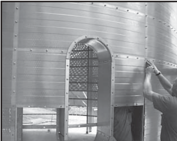
Photo 16-26 Bolt Outside Wall Sheets inside Window Frame.
