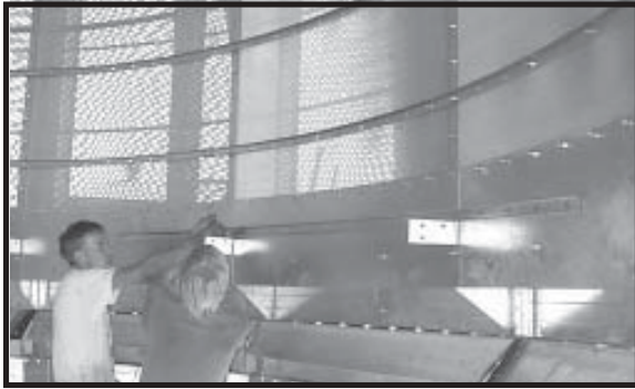
Photo 18-6 Installing last ring of Rolled Plenum Channel.
