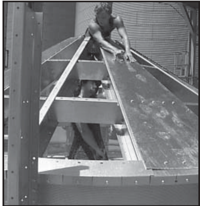
Photo 2-31 Bolting Plenum Roof Sheets.
