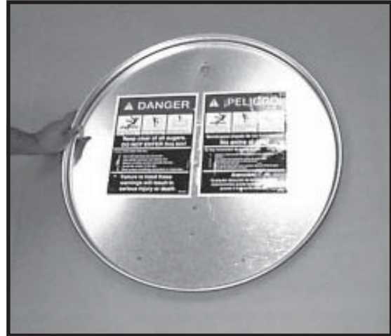
Tower roof access port with decals in place.
