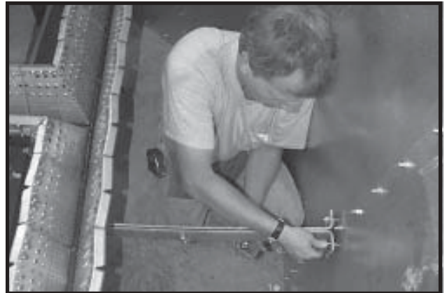
Photo 12-17 Installing a pair of Burner Support Tees (back to back) to Burner Housing.
