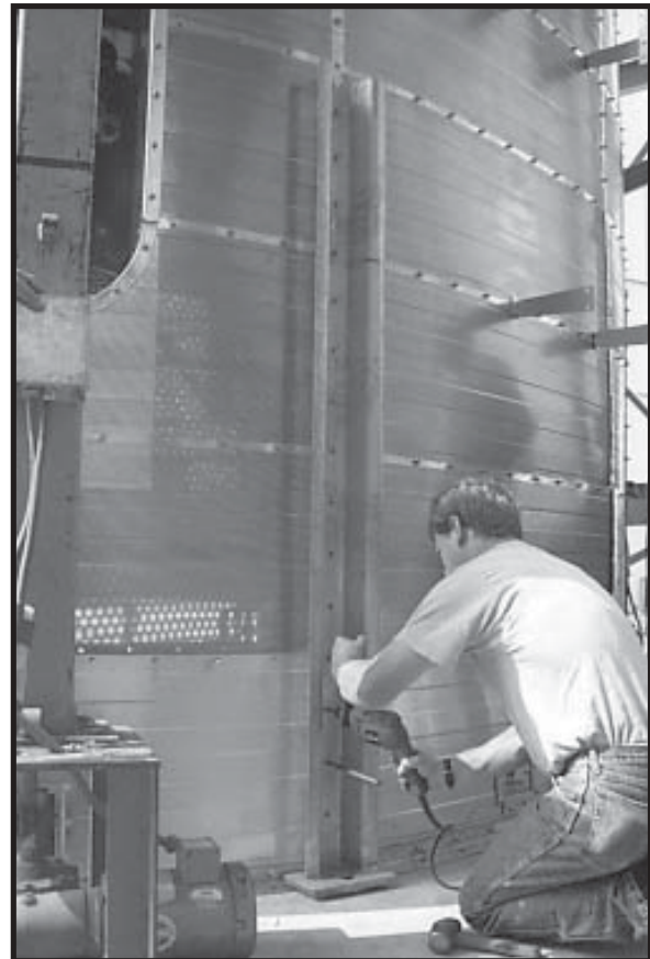
Photo 17-7 Tightening Base Stiffener Weldment to Vertical Base Channel.
