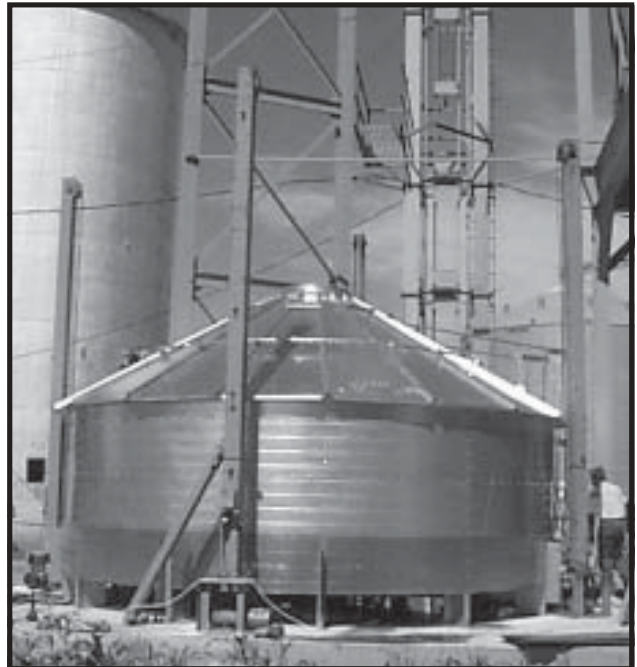
Photo 7-9 Jacks in place around dryer.
