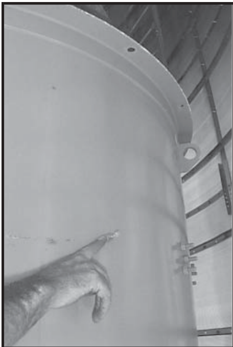
Photo 13-23 Note location of upper Grease Zert for installation of Grease Tube in later step.
