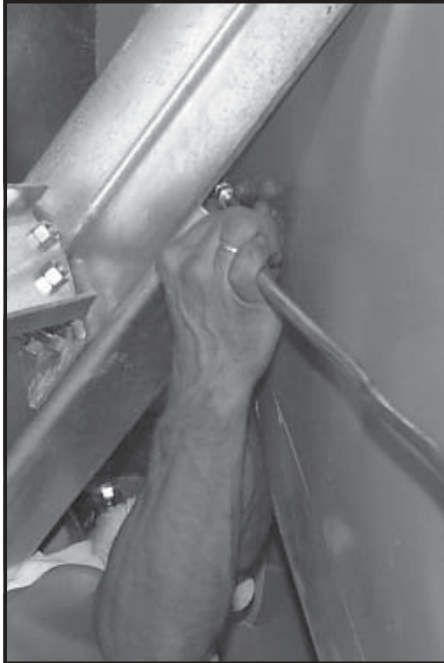
Photo 15-10 Attaching Grease Tube to Brass Compression Union.
