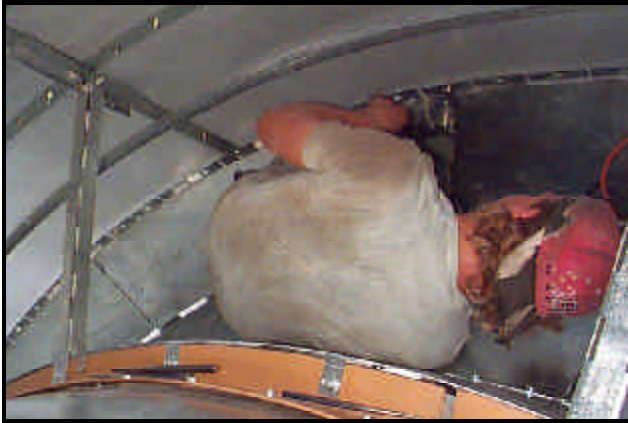
Photo 13-51 Drilling bolt holes in Inside Wall Sheets to bolt to Outer Divider Hopper.
