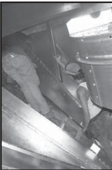
Photo 19-39 Bolting Cool Section Floor Support to Cool Section Floor Beam.
