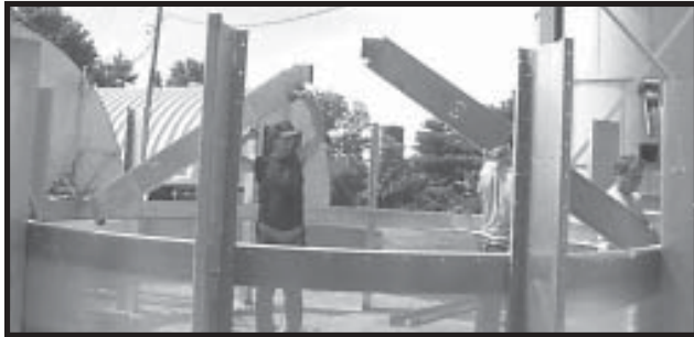
Photo 2-21 From opposite sides of dryer, bring a (RH and LH) pair of Plenum Roof Rafters together in center of dryer.
