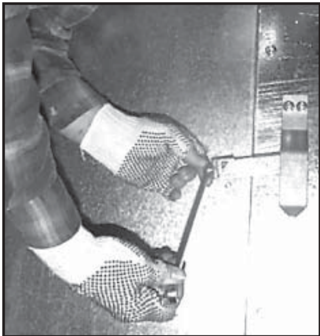
Photo 16-50 Adjusting bolt on Latch Bar.
