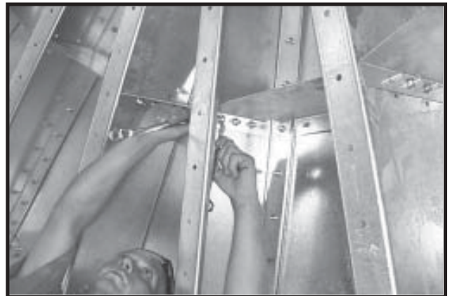
Photo 2-40 Hand tightening Rafter CrossMembers.
