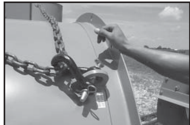
Photo 13-14 Lifting tackle is attached to Fan Lift Eyelets.
