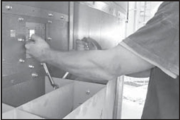
Photo 11-5 Tightening Grain Turner Sections.
