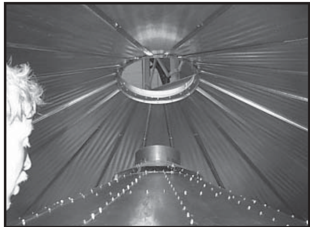
Photo 3-16 Inside view - peak of Tower Roof Sheets bolts to bottom of Tower Roof Center Collar.
