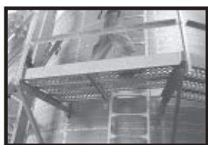
Photo 8-16 Outside Catwalk Door - closed.
