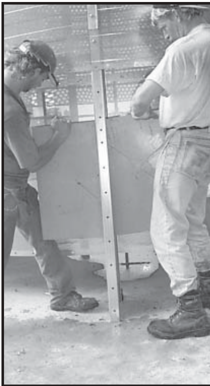
Photo 11-3 Installing outside Grain Turner Sections.
