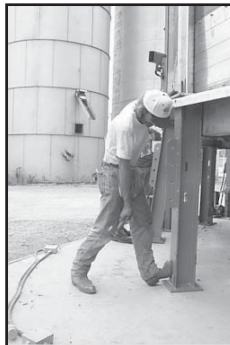
Photo 17-17 Placing Upper Leg directly under Base Stiffener Weldment.
