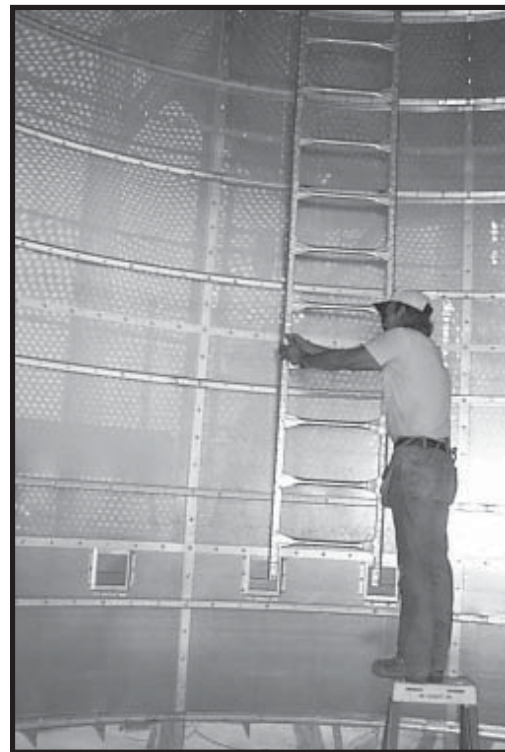
Photo 9-7 Installing first Auxiliary Ladder past Slide Gates - Clean Out (Grain Turners).
