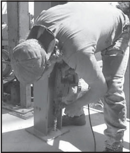
Photo 17-30 Drill proper size hole.
