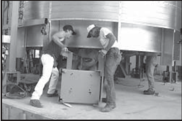
Photo 14-3 Moving Fan Motor Mount under Fan.
