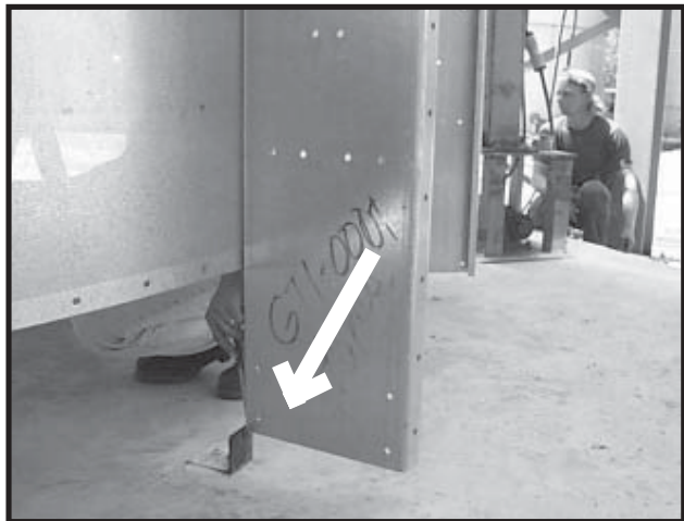
Photo 7-15 Lowering Vertical Channel on outside of Jig Clip.
