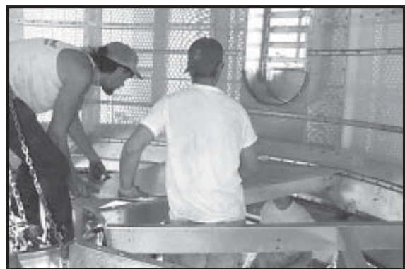
Photo 18-17 Placing Cool Section Floor Sheets.
