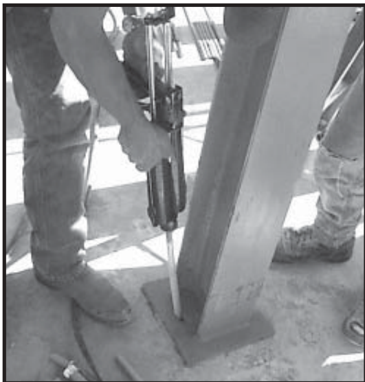
Photo 17-32 Fill hole with Ceramic Epoxy.
