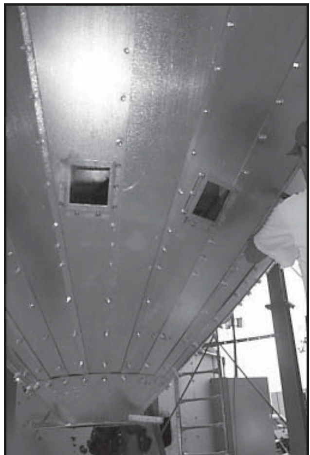
Photos 10-8 Slide Gate installed to Outside Hopper Panels. (For emergency discharge.)
