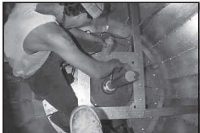
Photo 20-23 Applying anti-seize to Metering Drum Drive Shaft.
