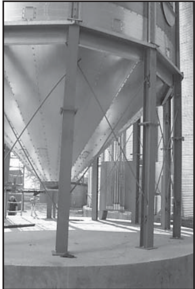
Photo 17-38 X-Bracing Rods installed.
