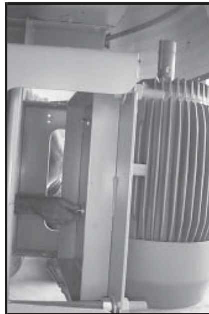
Photo 14-10 Bolting Fan Motor to Fan Motor Mount.
