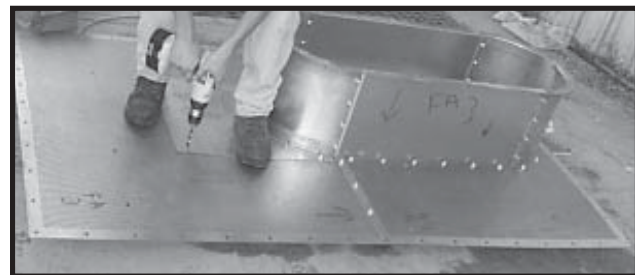
Photo 16-18 Bolt Window Frame to Wall Sheets.
