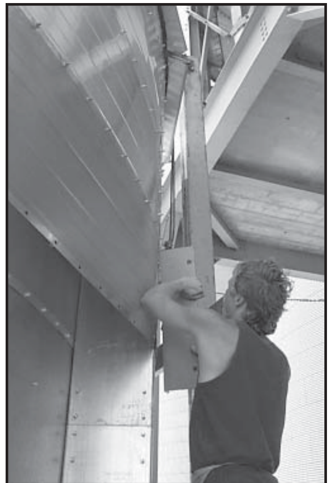
Photo 7-17 Removing Lift Bracket.
