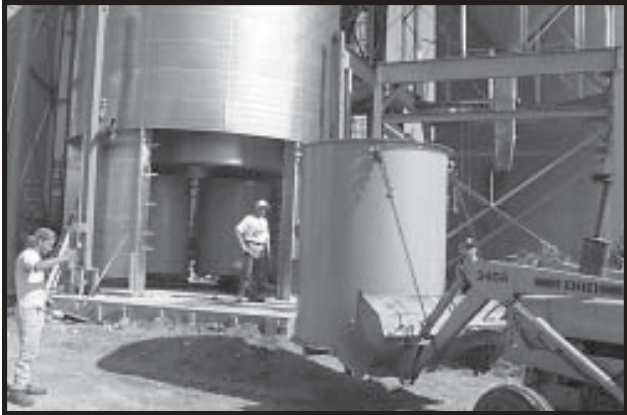
Photo 13-17 Move Fans to dryer.
