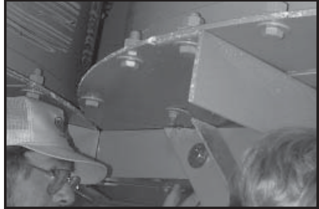
Photo 14-4 Align Fan Motor Mount and bolt to Fan.
