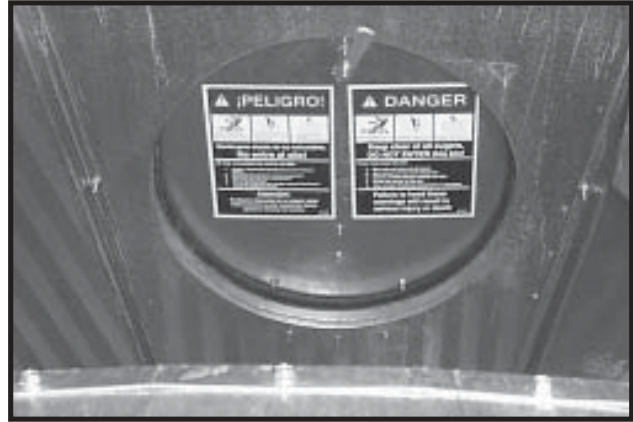
Photo 3-35 Inside View - Access Port Cover installed.
