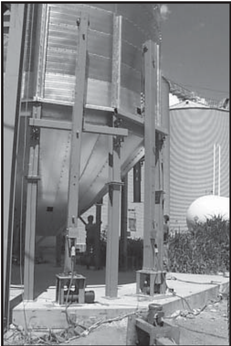
Photo 17-25 Dryer Legs are installed. Dryer is round and vertical.
