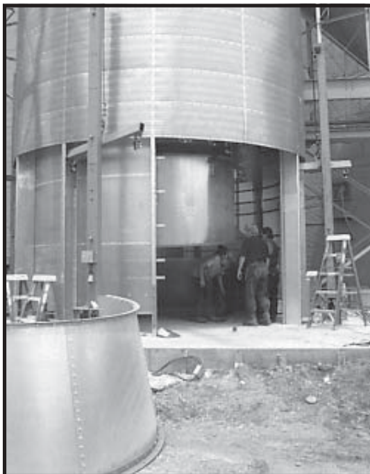
Photo 12-21 Remove Rolled Plenum Channels, and lift Burner/Burner Housing to provide access for Reducer.
