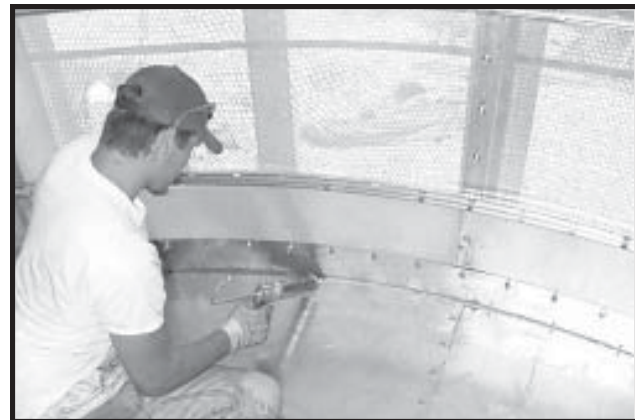
Photo 18-23 Caulking outside edge of Cool Section Floor.
