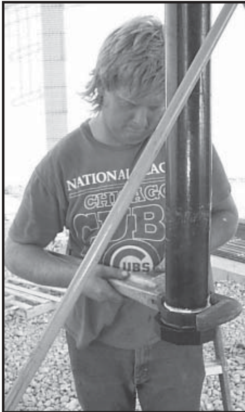
Photo 22-15 Attaching Union to Fuel Pipe.
