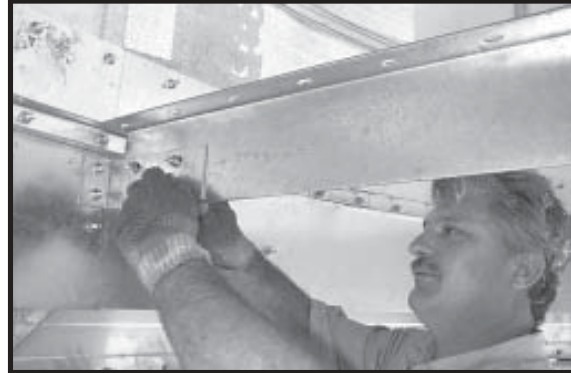
Photo 18-7 Snug bolting Cool Section Floor Beam to Cool Section Floor Beam Bracket (on Inside Solid Wall Sheet).
