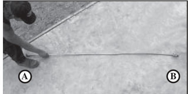
Photo 15-2 Grease Tube for upper bearing on Fan.
