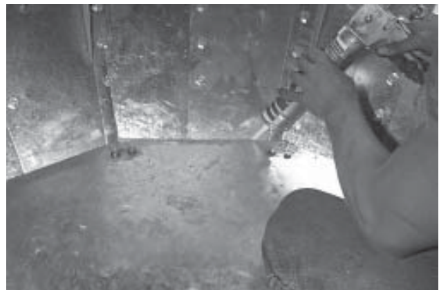
Photo 19-28 Caulking Metering Drum Floor with silicone caulk.
