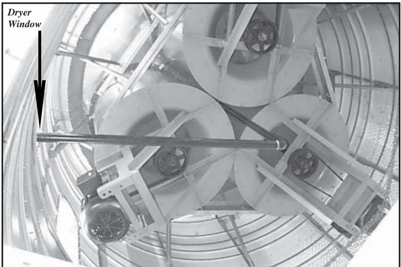
Photo 21-14 Just below Fans, installed Fuel Piping turns 90 degrees, and exits Cool Section through Dryer Window.
