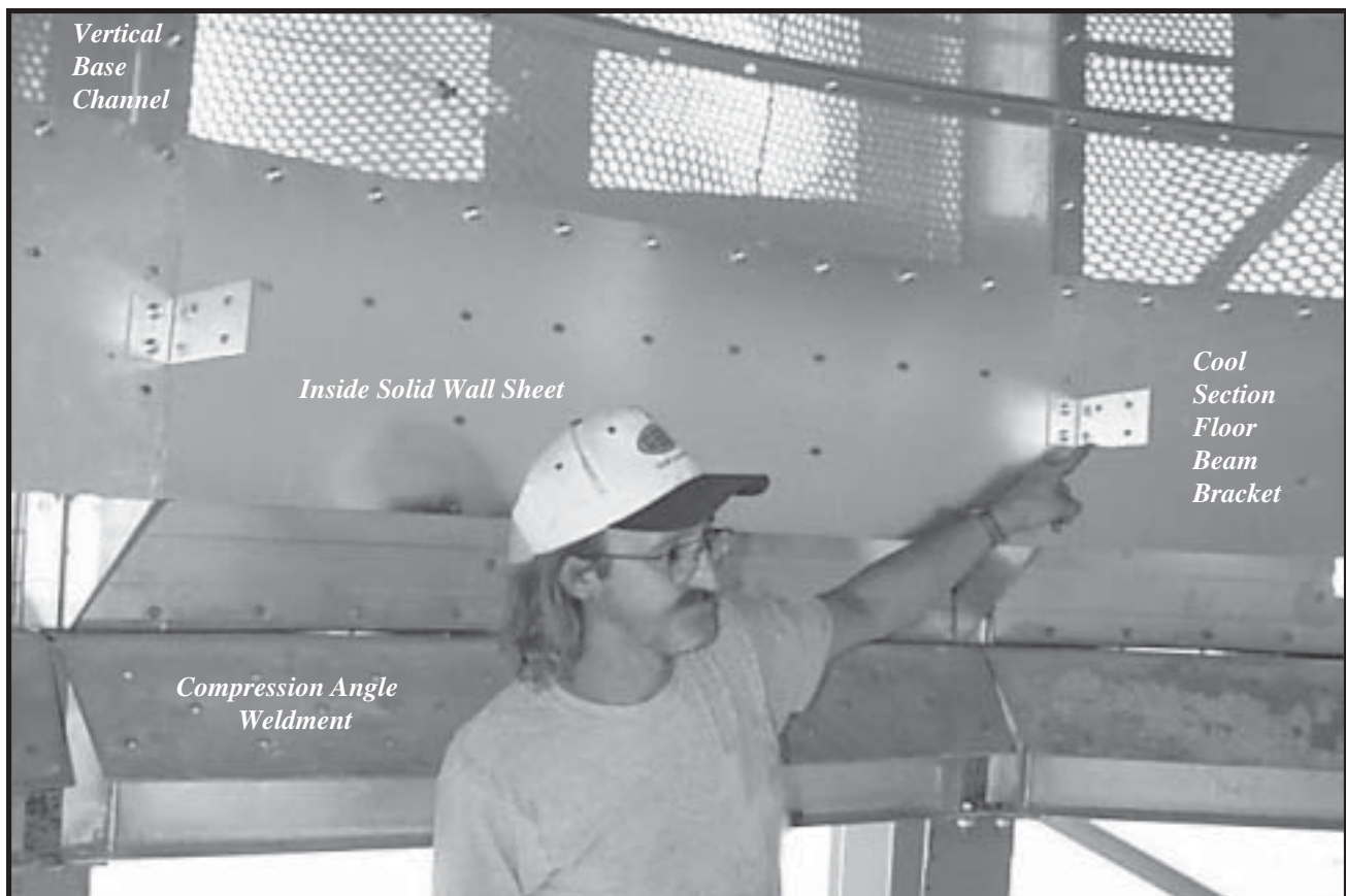
Photo 17-14 Bolt Cool Section Floor Beam Bracket (through Inside Solid Wall Sheets) to each Vertical Base Channel.
