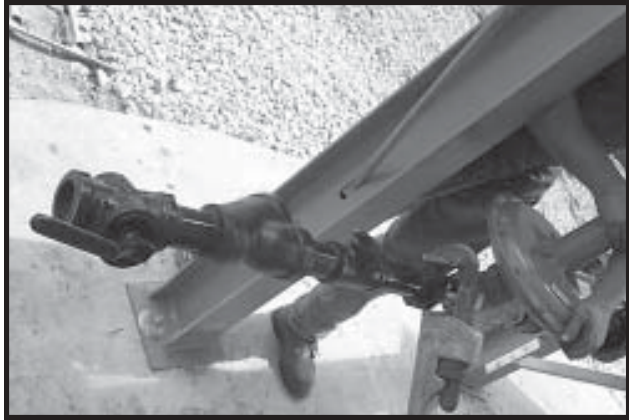
Photo 22-26 Installing Shutoff Section.
