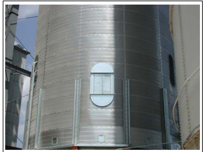
Figure 18AJ Outsided View - Installed 24" louvered window, with louvers open.
