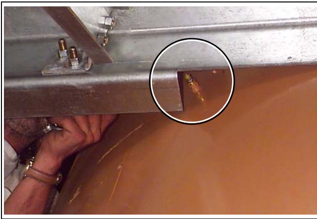
Figure 17F Grease zerk on fan (circled).
