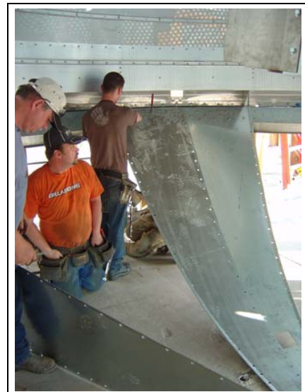
Figure 21P Aligning Outside Hopper Panels
