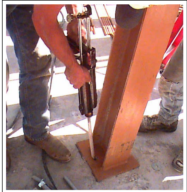
Figure 19AG Fill hole with ceramic epoxy.
