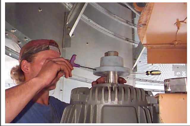
Figure 16O Tightening set screw on motor hub.
