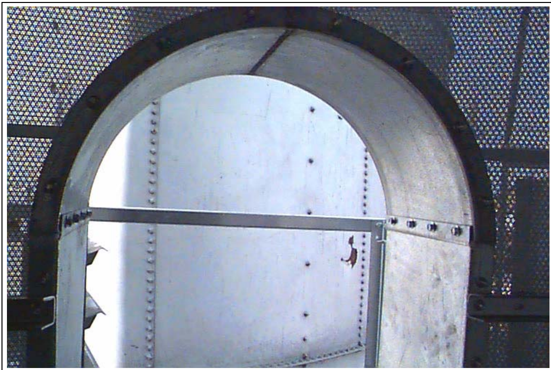
Figure 18AF Close Up - 18" Window installed. (Screening is not yet installed.)
