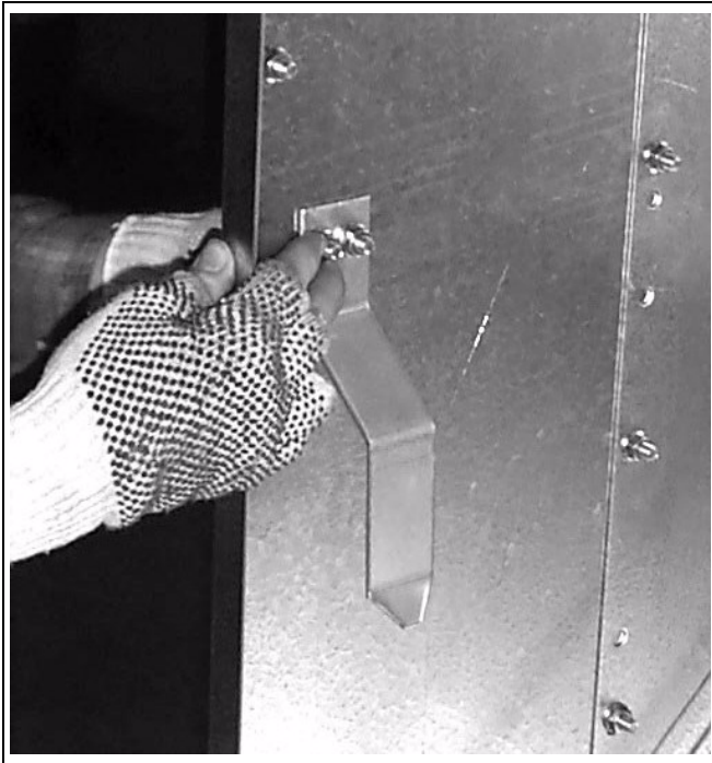
Figure 18AW Bolting door latch in pre-drilled bolt holes inside reducer.
