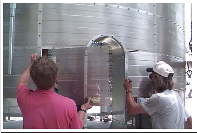
Figure 18Y Fit outside wall sheets to window frame.
