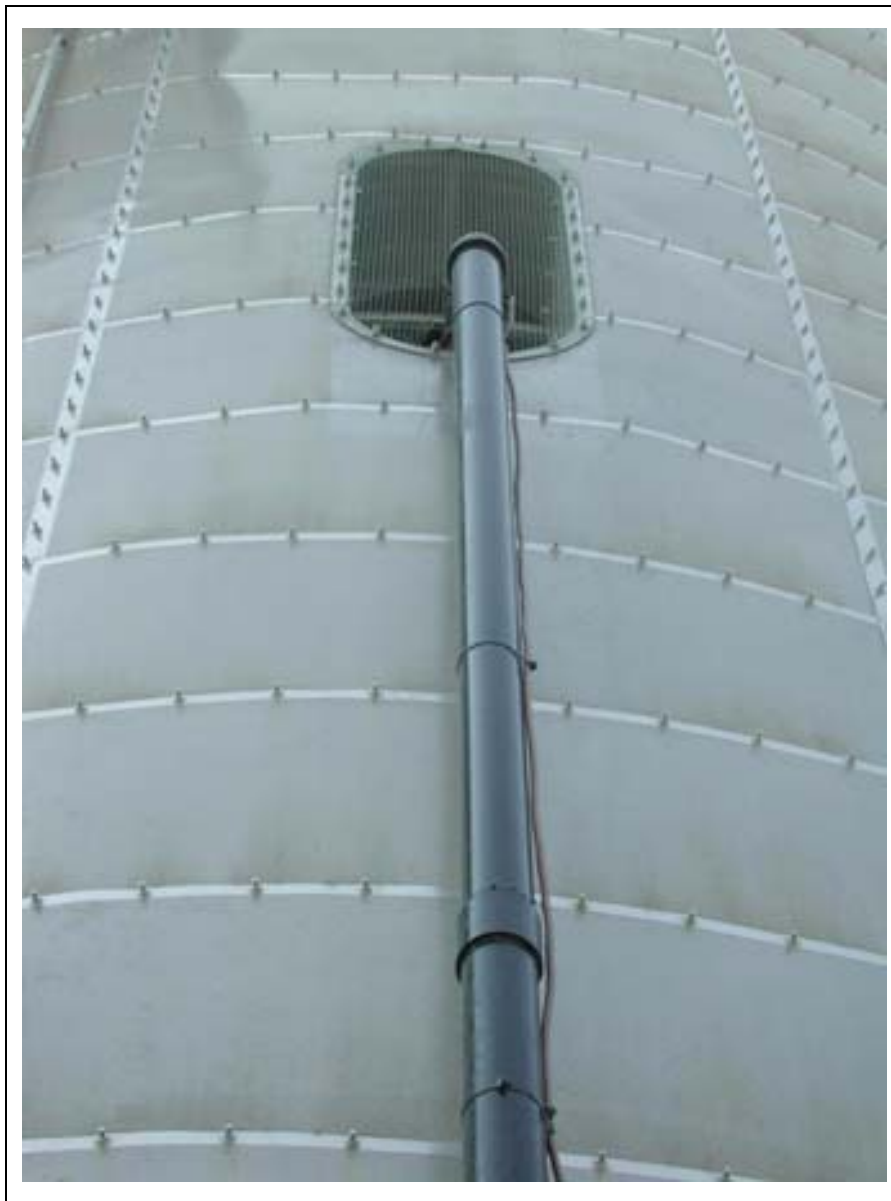
Figure 24AC Fuel train installed. (Typical)
