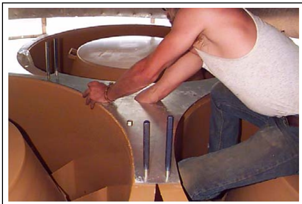
Figure 15AC Bolting fan housing splice, centered on top of fan cluster.
