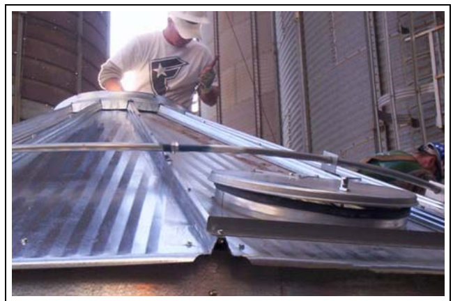
Figure 6AF Tightening center collar flashing bolts.
