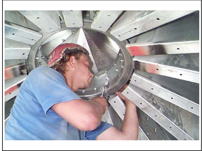
Figure 5AX Hand tightening plenum roof rafters, wall sheets, eave channels, cross members, etc.
