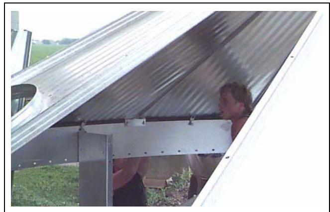
Figure 6T Inside view - Tower roof sheets bolt to eave clips, and intermediate eave clips.
