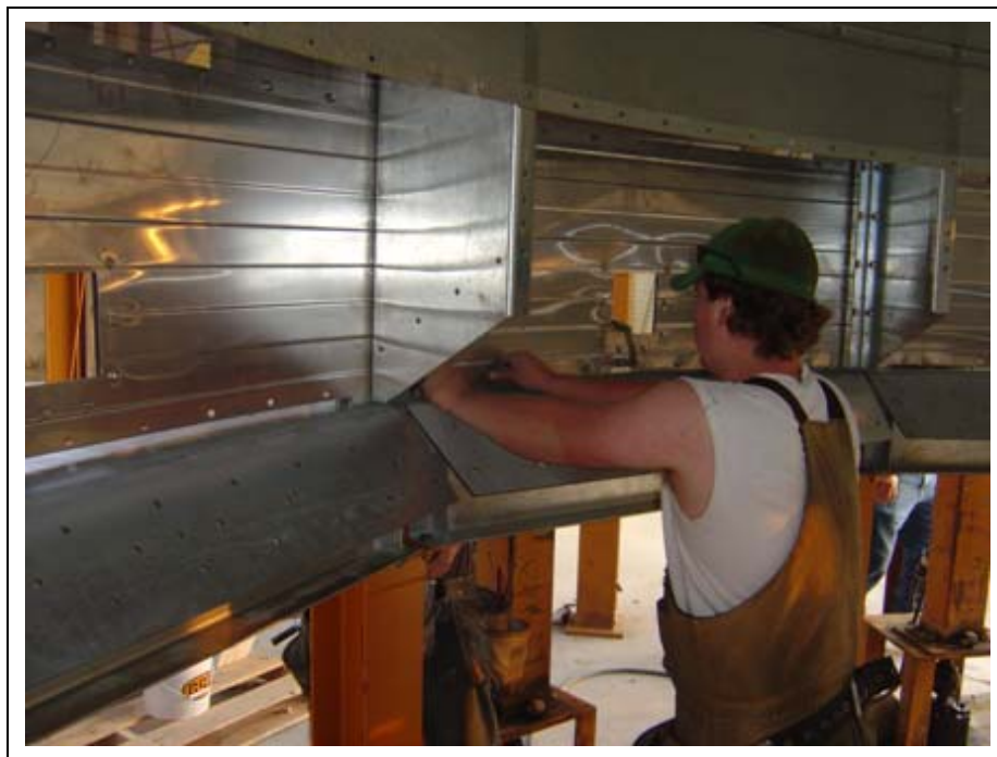
Figure 19O Inside view - Installing compression angle weldments.
