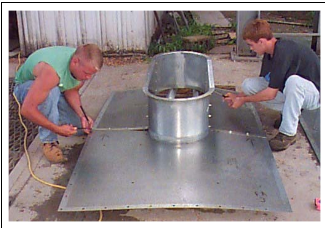
Figure 18O After cutting window outline, realign window frame to wall sheets and drill out bolt holes.
