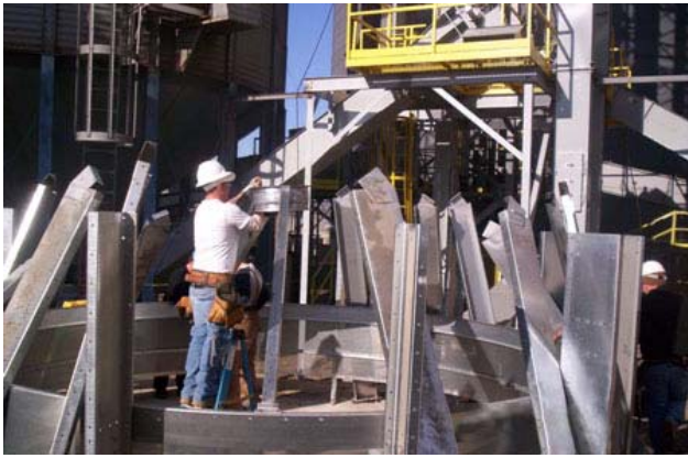
Figure 5AF From opposite sides of dryer, bring a (R.H. and L.H.) pair of plenum roof rafters together in center of dryer.
