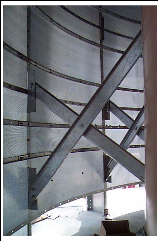
Figure 15AP X-Bracing installed.
