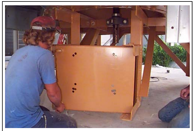
Figure 16G Fan motor mount installed.
