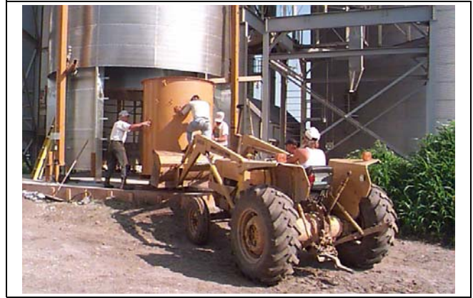
Figure 15V Pushing fans into dryer.
