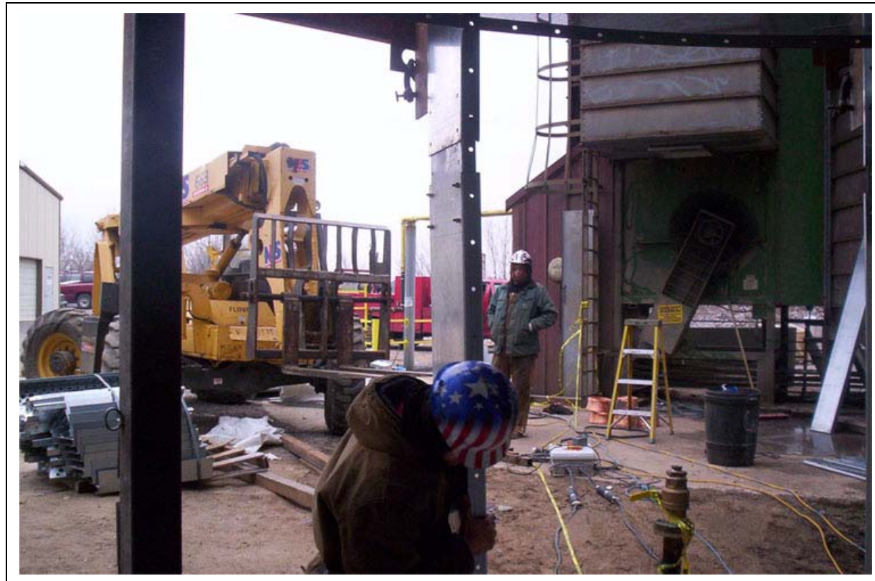
Figure 9Q Removing lift bracket.
