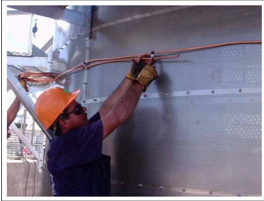
Figure 8O Upper High-Limit installed with junction box under outside ladder (arrow).
