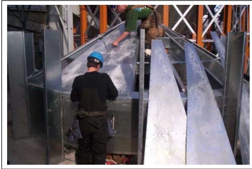
Figure 5AP Bolting Plenum Roof Sheets
