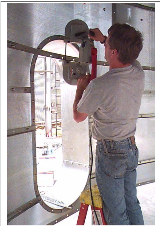
Figure 18V Drill and bolt rolled plenum channels, then cut away from window frames.
