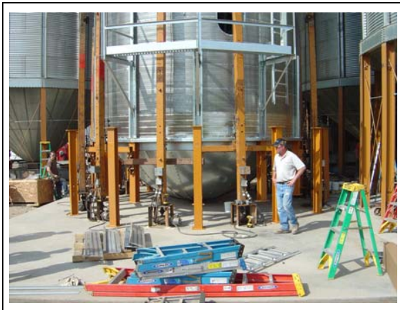
Figure 21S Installing outside hopper panels.
