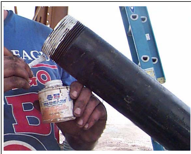
Figure 23I Seal all threaded pipe connections with heavy duty pipe sealing compound.
