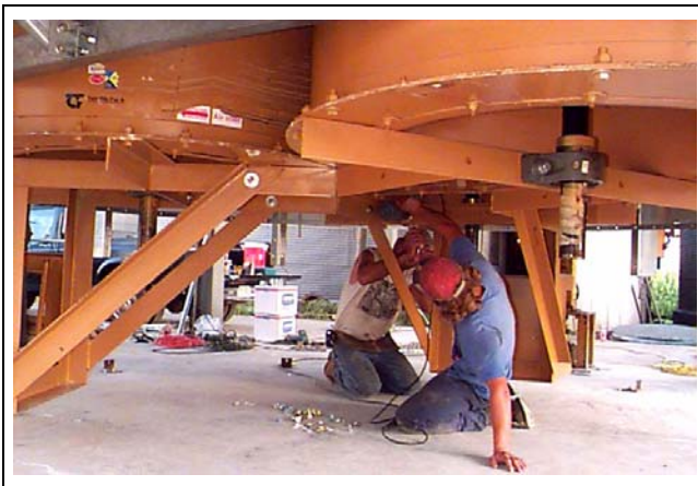
Figure 16F Tightening bolts on fan motor mount.
