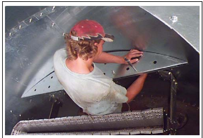
Figure 14V Installing burner baffles.
