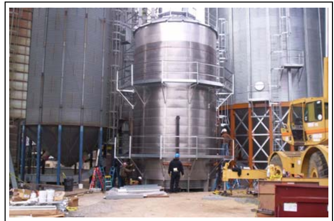
Figure 10Z Completed Outside Catwalks
