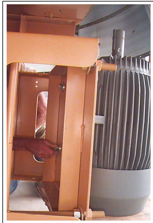
Figure 16J Bolting fan motor to fan motor mount.
