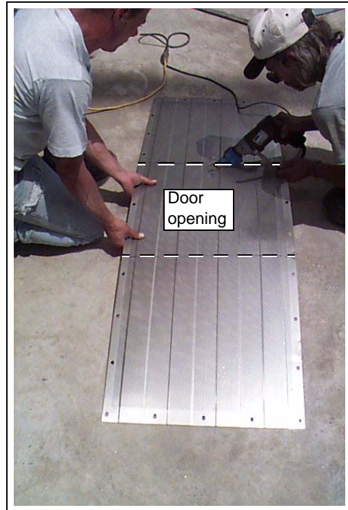
Figure 18X Cut outside wall sheets on inside of marked line so they will fit inside window frame. Drill bolt holes and bolt cut rolled plenum channels to window frame.
