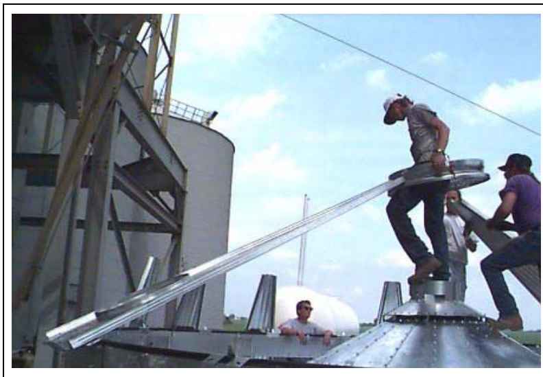
Figure 6R Bringing two (2) opposing tower roof sheets to tower roof center collar. Position tower roof sheet with access port cut out directly above where outside ladder will be.
