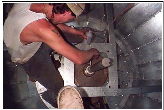
Figure 22S Applying anti-seize to metering drum drive shaft.
