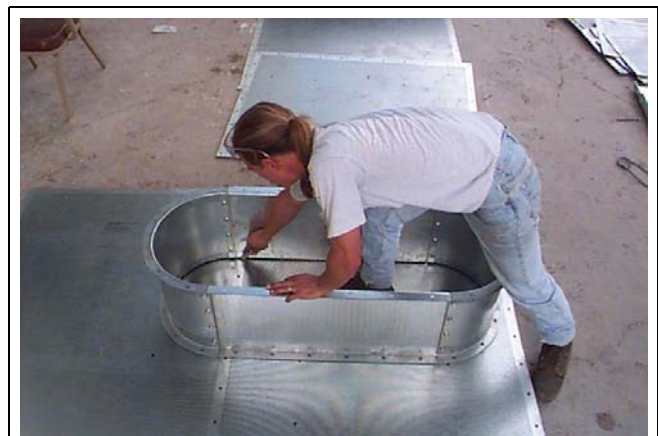
Figure 18L Mark around inside perimeter of window frame.
