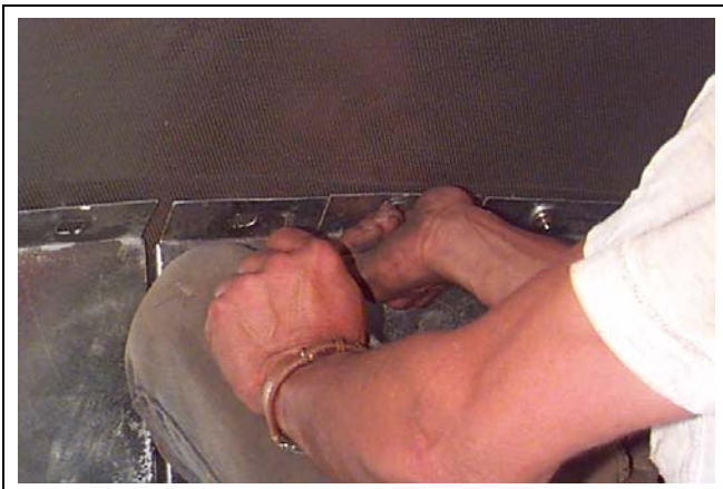
Figure 15BD Close Up - bolting outer divider hopper to inside wall sheet.
