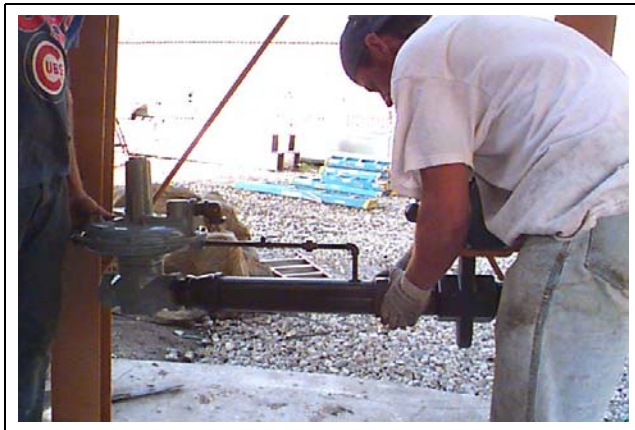
Figure 24V Installing regulator section.
