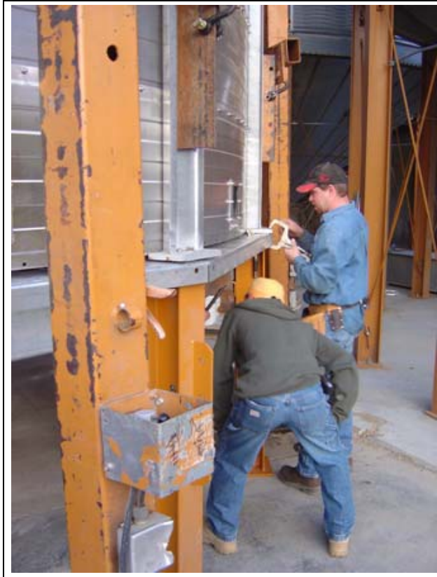
Figure 19N Compression angle weldments encircle base of dryer.
