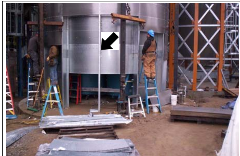
Figure 15X Re-installing vertical channel after fans are inside dryer.
