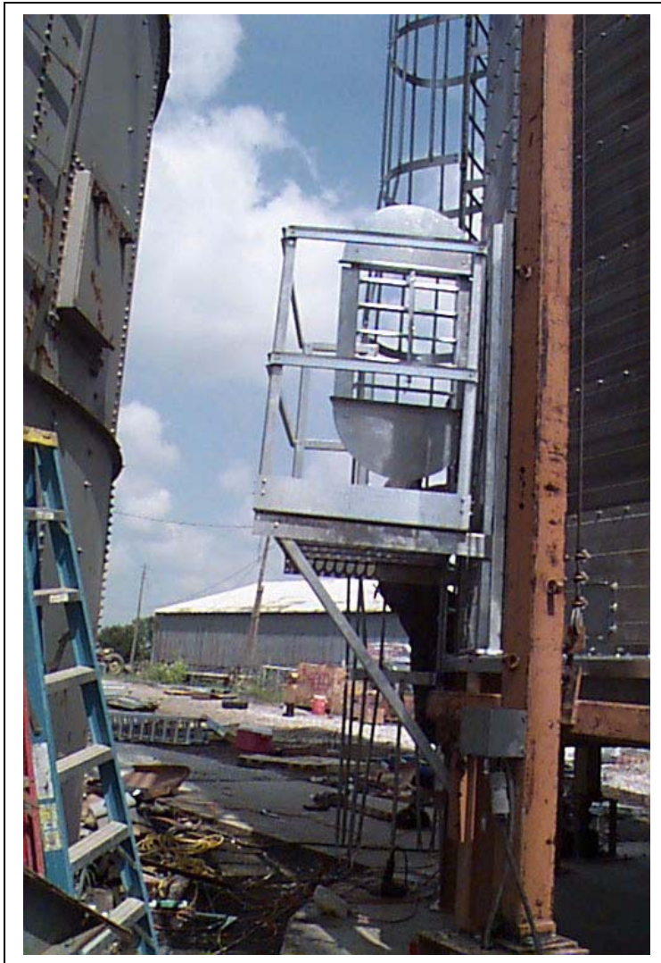
Figure 18AK Cool section door is installed.
