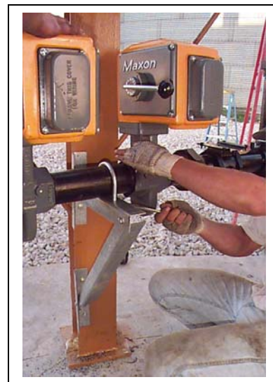
Figure 24Z Securing fuel train to fuel train stand with 3" U-bolt.
