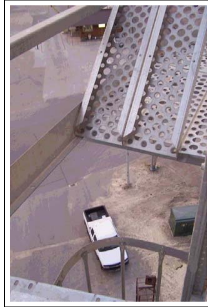
Figure 10X Outside Catwalk Door - Open
