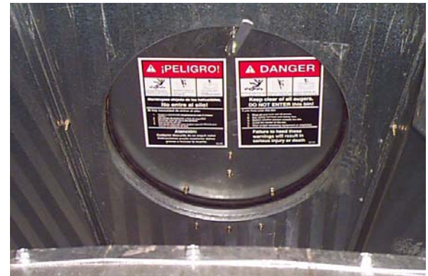
Inside view - Access port installed with decals in place.
