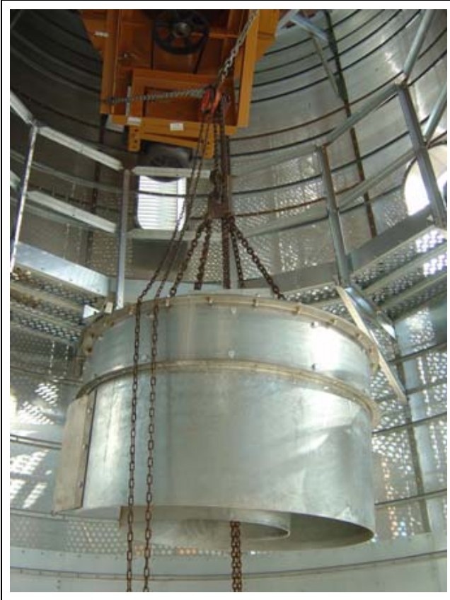
Figure 22B Metering Drum
