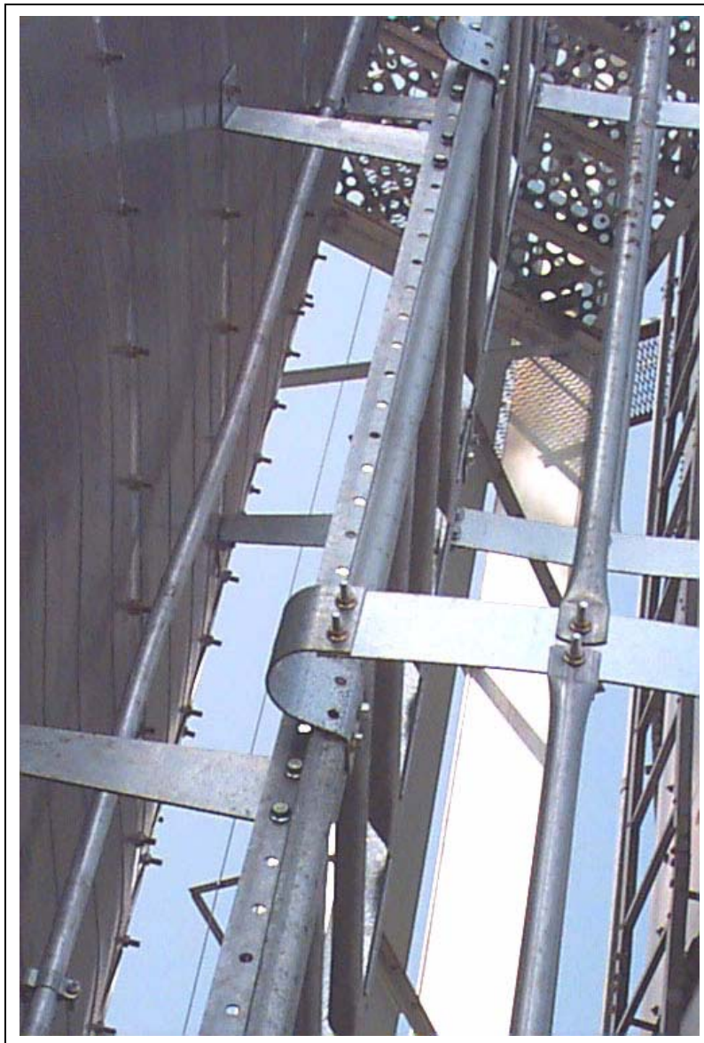
Figure 7J Close Up - Shaft of bolts point out of safety cage so climbers do not snag.
