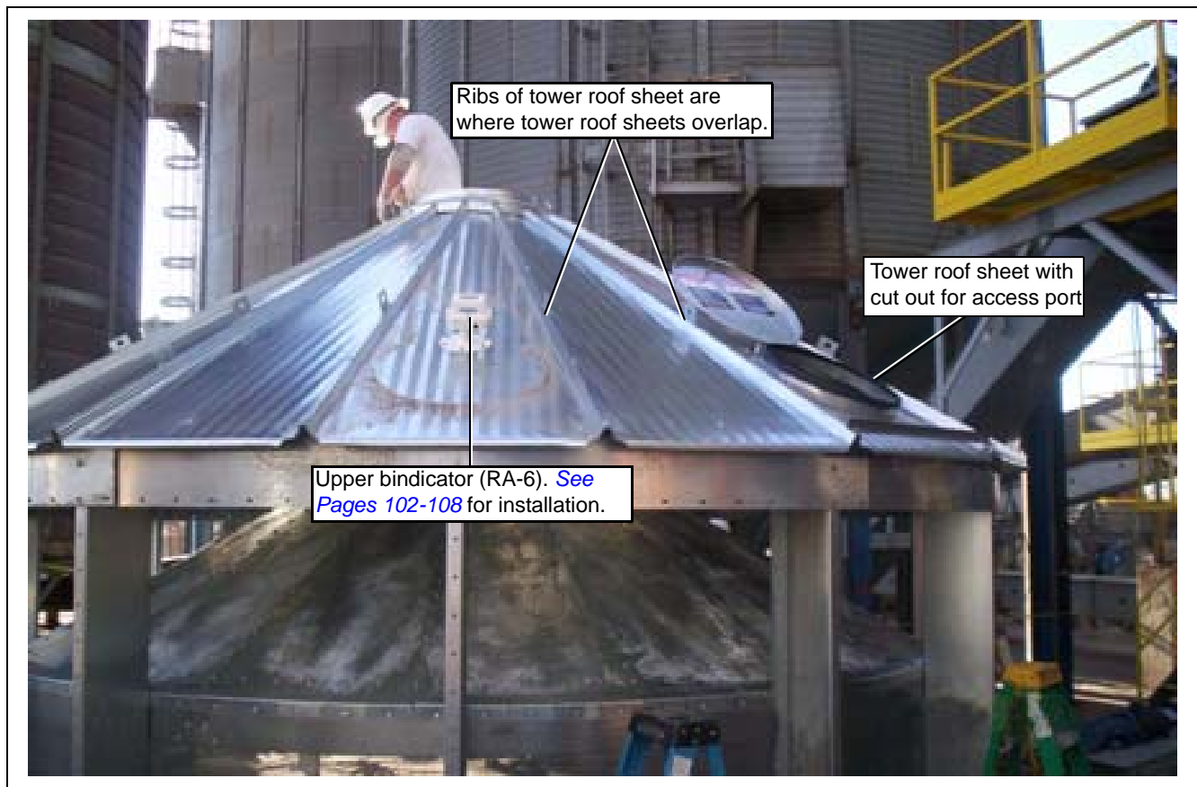
Figure 6Q Install roof rungs on ribs of the tower roof sheet with cut out for access port.
