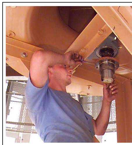
Figure 16T Tightening set screw on fan hub.
