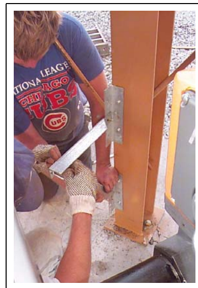
Figure 24Y Close Up - Bolting fuel train stand.
