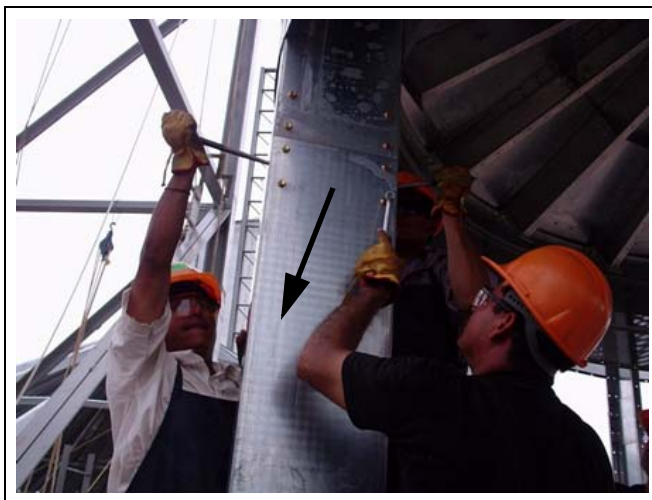
Figure 9O Lowering vertical channel on outside of jig clip.
