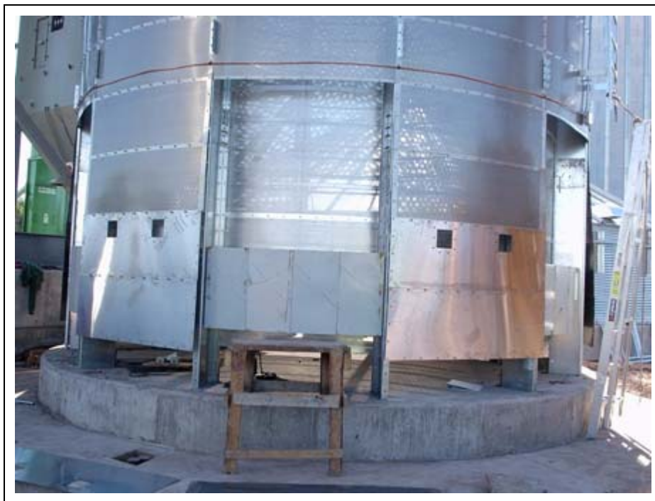
Figure 13F Installed grain turners.
