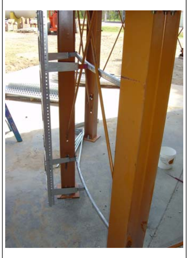
Figure 19AM X-Bracing rods installed.
