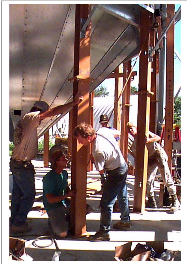
Figure 19AI Installing X-bracing rods to dryer legs
