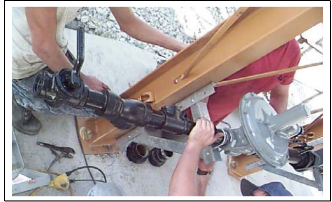
Figure 24AB Second fuel train stand installed.
