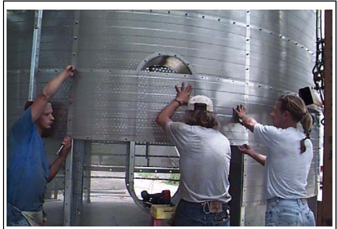
Figure 18W Mark outside wall sheets so they will fit inside window frame.
