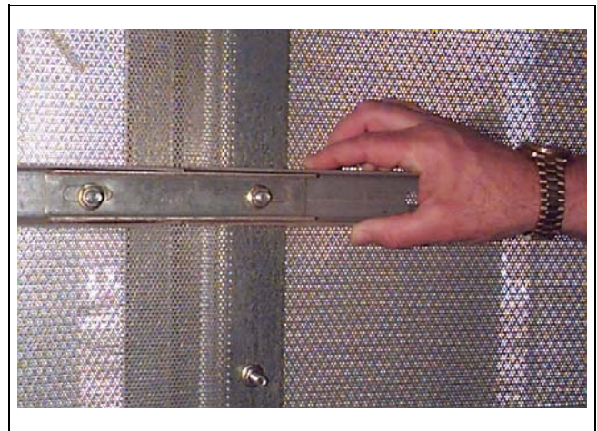
Figure 5T Plenum channel splice installed.
