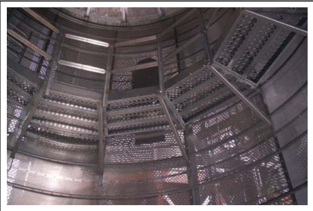
Figure 10AG View from below - Completed inside catwalk.
