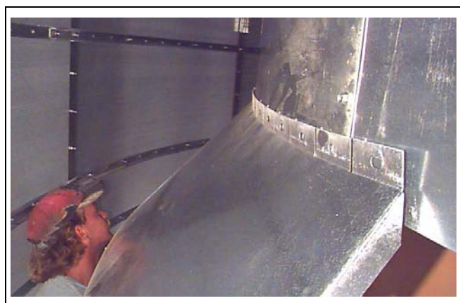
Figure 15AY Bolting top tabs of inner divider hopper to bottom of fan skirting.
