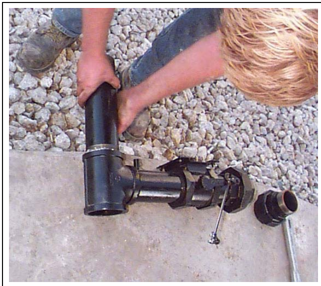
Figure 24Q Attaching 12" nipple to modutrol section.
