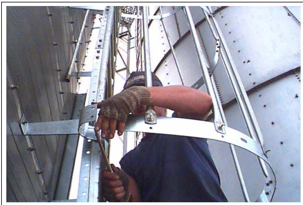
Figure 7U Close Up - Installing bell safety cage.
