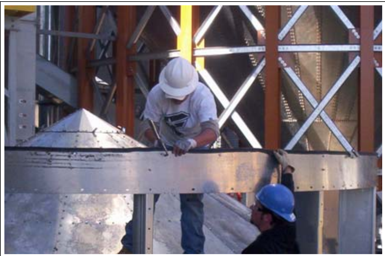
Figure 6E Installing roof band sections to overlap around (outside) top of vertical channels.
