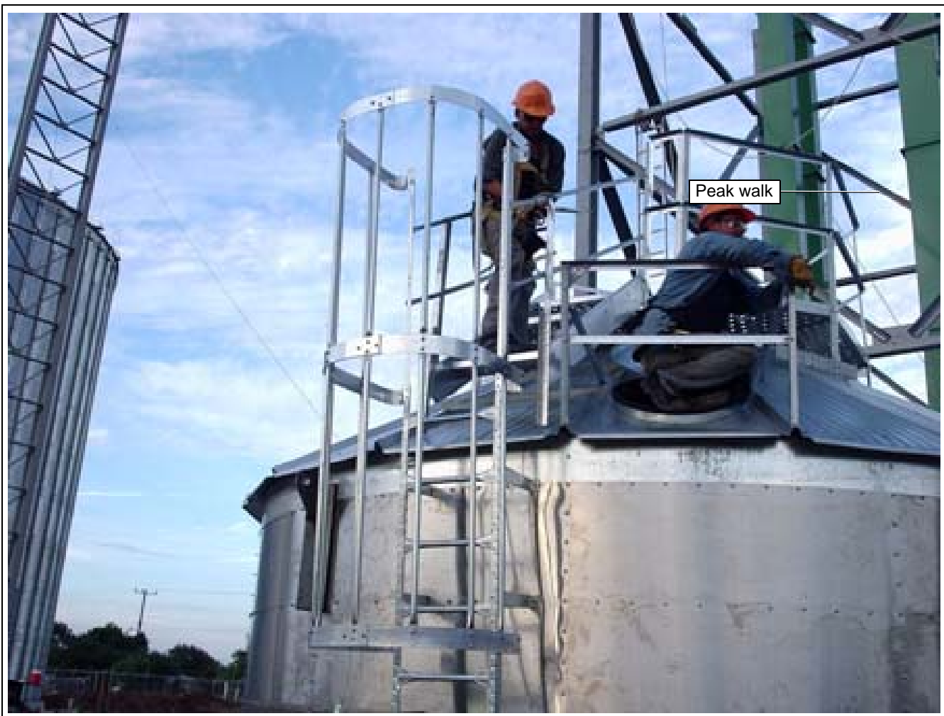
Figure 7K Installing top safety railing and peak walk to tower roof.
