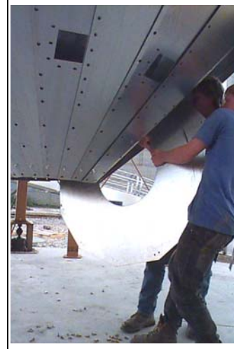
Figure 21T Bring metering drum floor into outside hopper before closing in with last panel.
