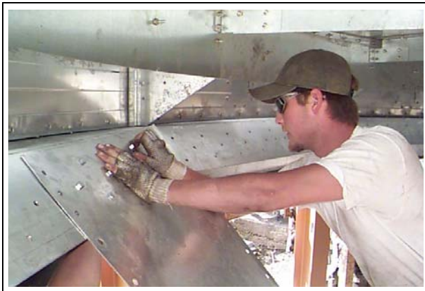
Figure 21M View from above - Bolting outside hopper panels over compression angles and compression angle splices.
