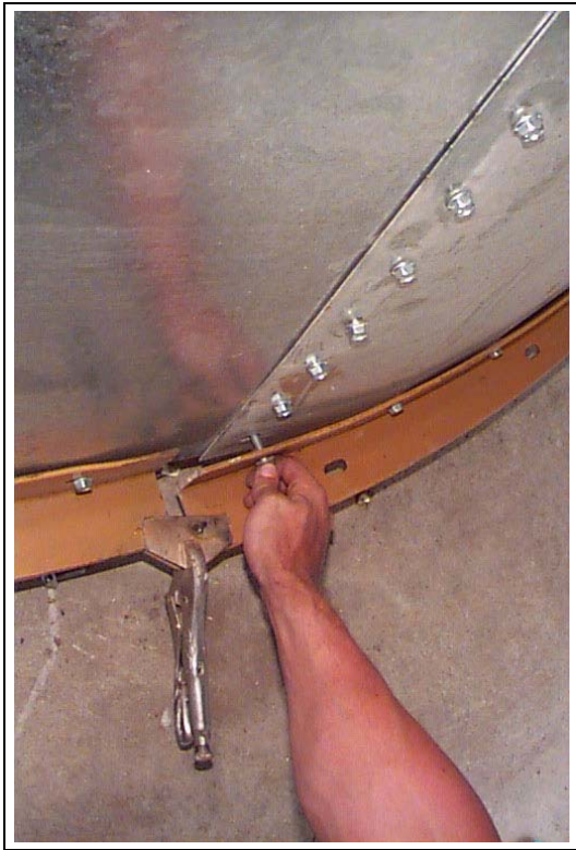
Figure 14AA Close Up - Bolting sections of reducer ring together.
