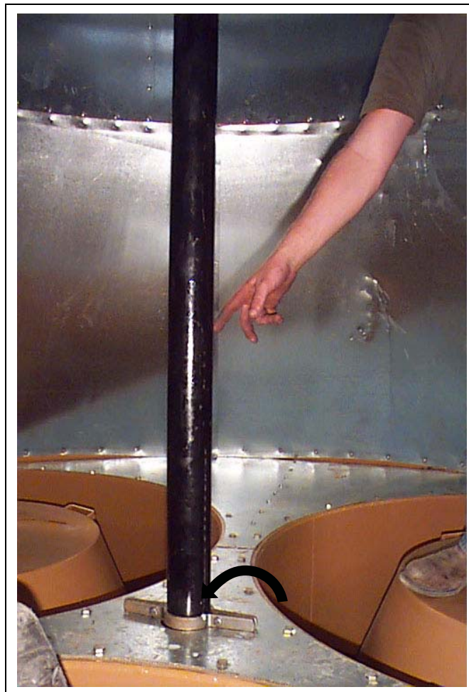
Figure 23K Installed fuel pipe exits heat section through pre-cut hole in center of fan housing splice (arrow).
