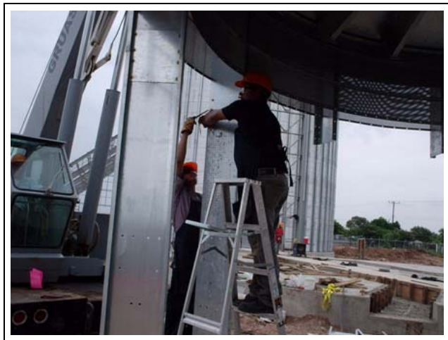
Figure 9L Aligning vertical channels.
