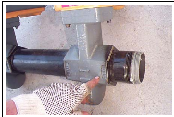
Figure 24T Close Up - Maxon. NOTE: Fuel flow indicators on all components.
