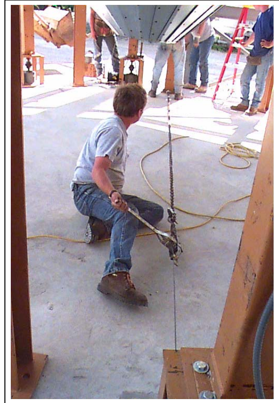
Figure 19Y Winching dryer legs into position.
