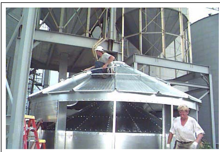
Figure 6AA Installing expansion ring to expansion ring clips.
