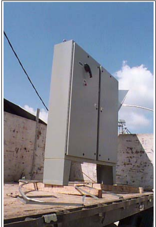
Figure 25B Electrical Control System
