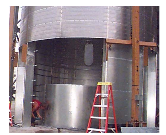
Figure 14I Bolting together halves of burner housing.
