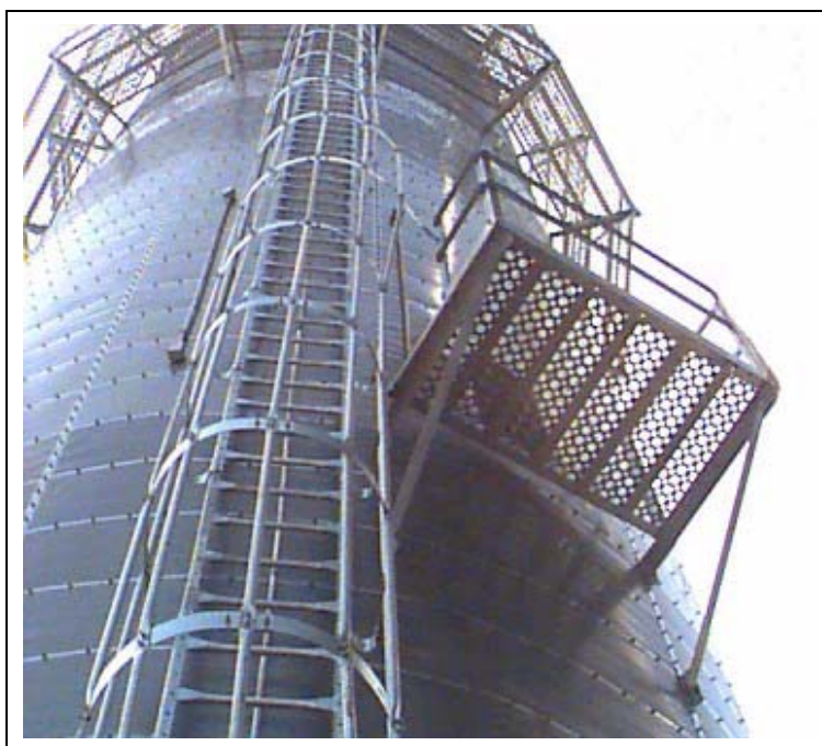
Figure 7Q Ground view - Ladder with safety cage installed through catwalks and to platform.
