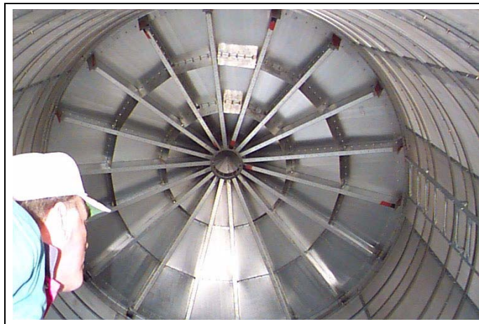
Figure 5AZ Interior View after lifting dryer - Completed plenum roof.
