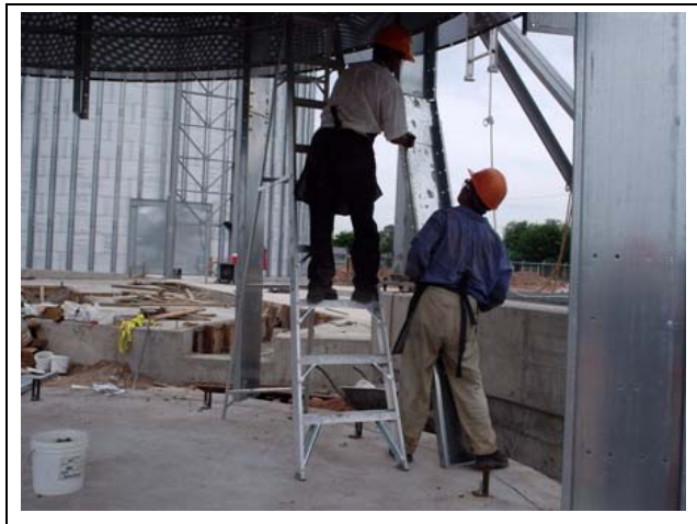
Figure 9K Sliding vertical channel up to vertical channel on dryer.
