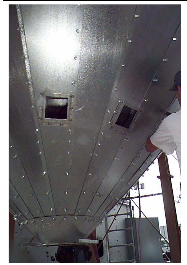
Figure 12E Use 5/16" x 3/4" galvanized at hopper clean outs. Slide gate installed to outside hopper panels. (For emergency discharge.)
