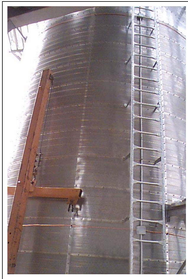
Figure 8W Installing L.H. Pair of RTDs
