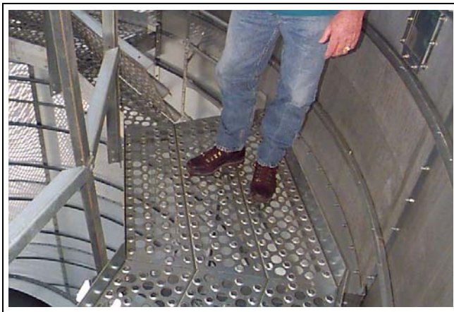
Figure 10AI View from above - Inside catwalk door open.
