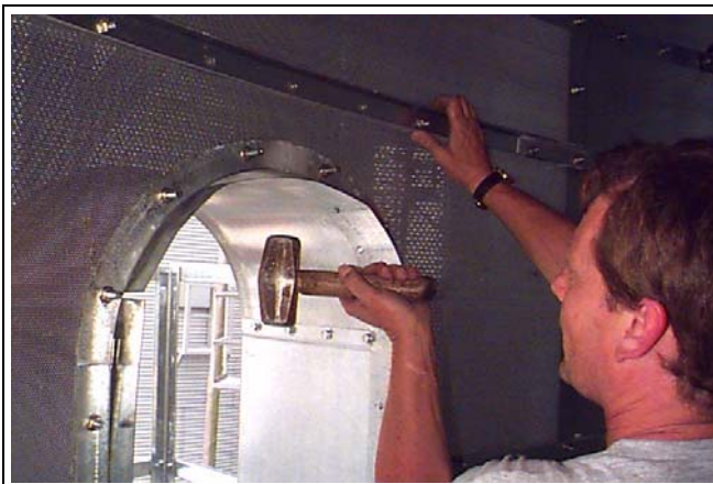
Figure 18AR Tap hammering heat section door sleeve around inside of door frame.
