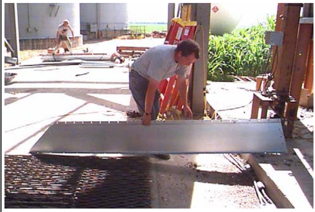
Figure 21AC Bringing hopper channels (R.H./L.H.) into dryer through opening in cool section floor.
