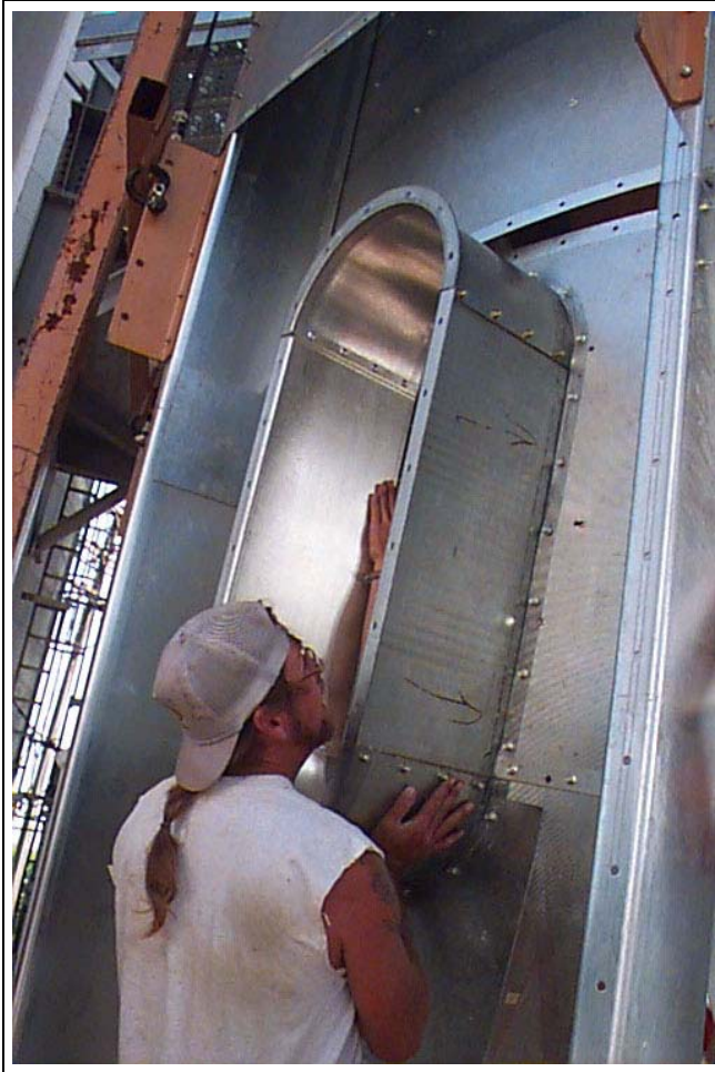
Figure 18S Hang pre-assembled wall sheets, window frame, and air deflector.
