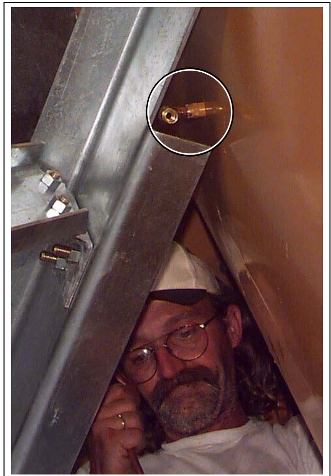
Figure 17I Elbow and brass compression union installed to fan (circled).
