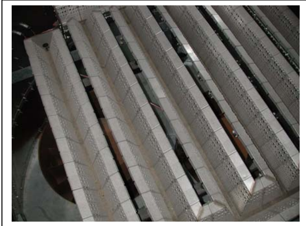
Figure 14P First burner support bracket installed to burner mounting bracket.
