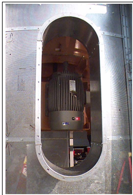
Figure 18AB Window is centered on fan motor.
