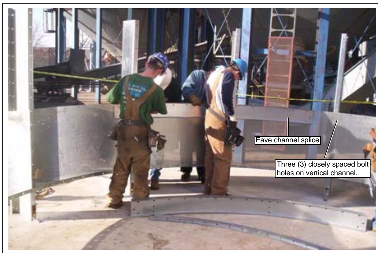
Figure 5X Installing eave channels to vertical channels.
