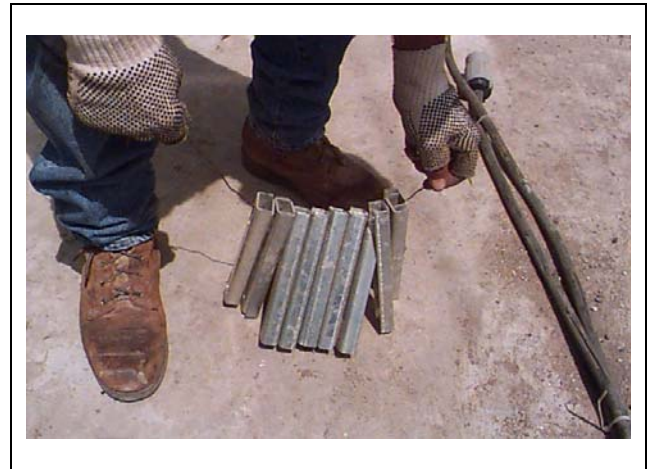
Figure 5Q Plenum Channel Splices - as shipped.
