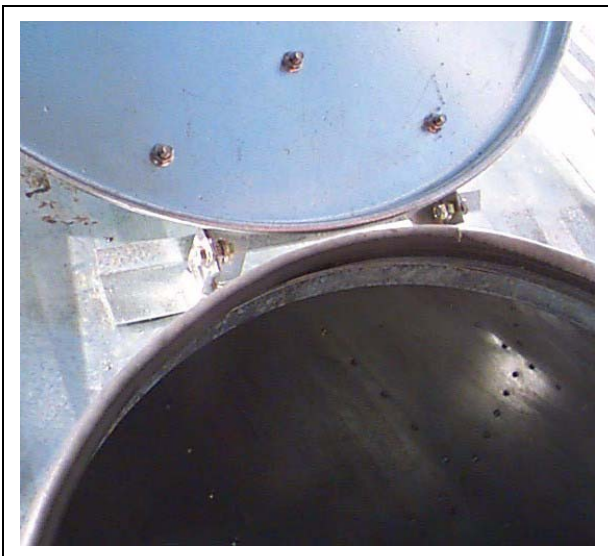
Figure 6AK Close Up - Access port cover installed.
