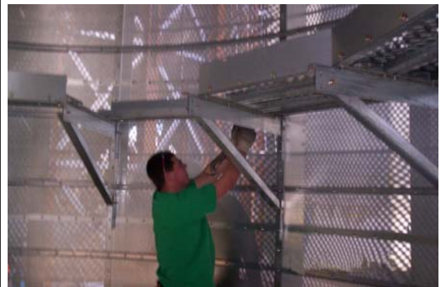
Figure 10AF Bolting inside catwalk splice plate to inside catwalk section.
