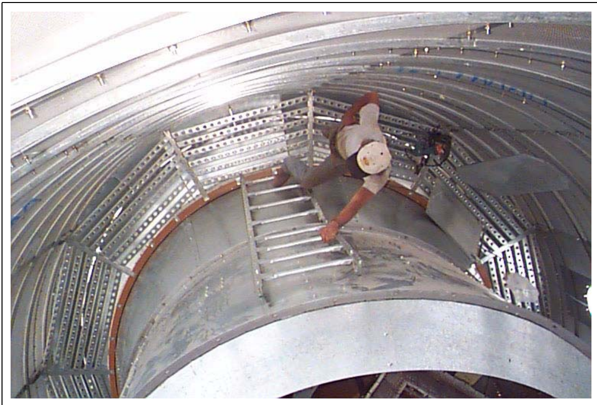
Figure 11N Installed burner housing ladder.
