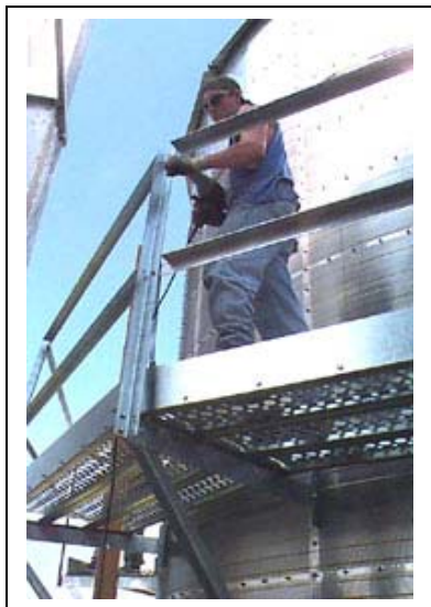
Figure 10W Tightening outside catwalk top handrail.
