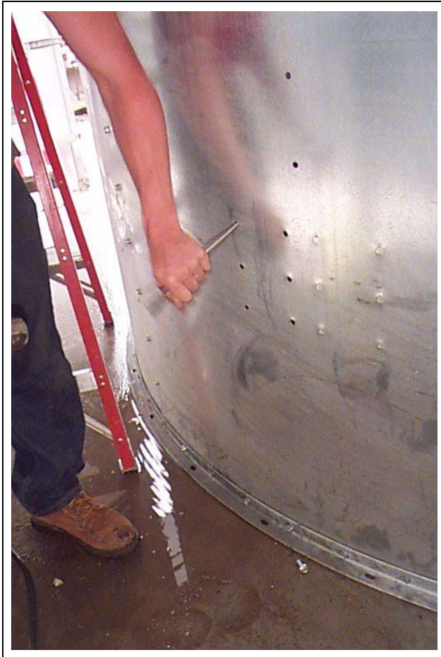
Figure 14M Knocking out bolt holes for burner mounting bracket. (May be pre-drilled at factory also.)
