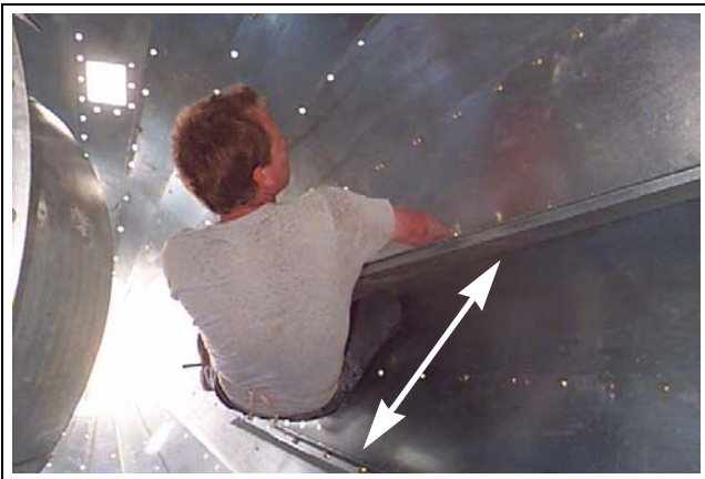
Figure 21AD View from above - R.H. and L.H. hopper channels bracket each other (arrow).
