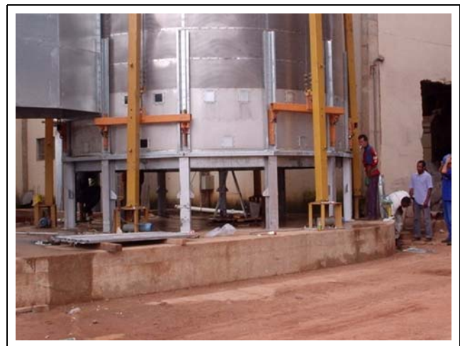
Figure 19U Upper legs are installed.
