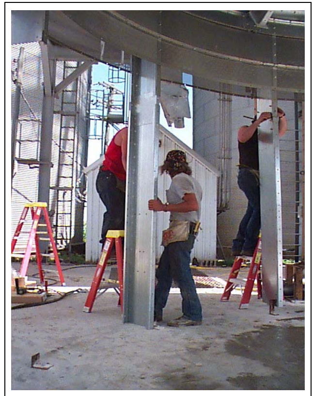
Figure 9N Close Up - Bolting vertical channels.
