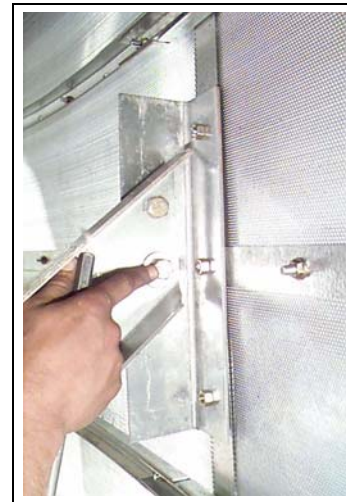
Figure 15AN R.H. View of bracing installed to fan support clip.
