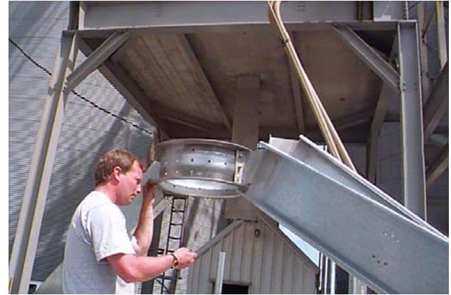
Figure 5AI Close Up - Bolt top of plenum roof rafters to plenum roof center collar.
