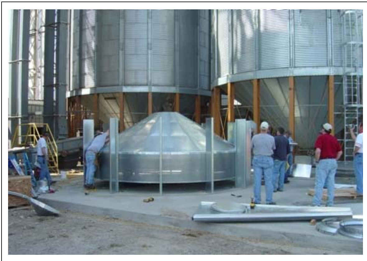
Figure 5AS Plenum roof is ready for peak cap assembly installation.
