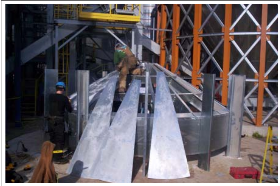
Figure 5AR Aligning Plenum Roof Sheets
