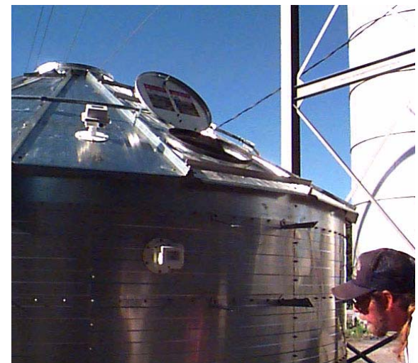
Outside view - Access port installed with decals in place.
