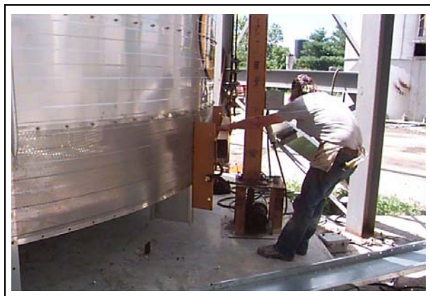
Figure 9F Positioning jack next to dryer.
