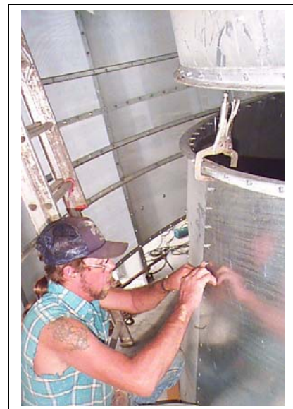
Figure 14Z Bolting halves of reducer together.
