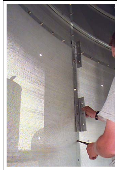
Figure 10AC Catwalk support clip is installed with angle up on R.H. side.
