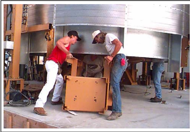
Figure 16C Moving fan motor mount under fan.
