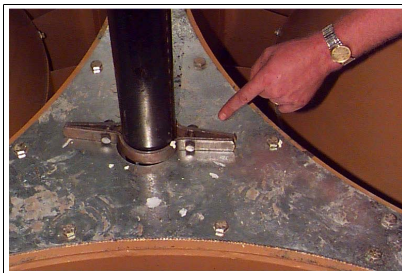
Figure 23L Close Up - Installed fuel piping exits heat section through pre-cut hole in center of fan housing splice. NOTE: 3" Pipe riser clamp.
