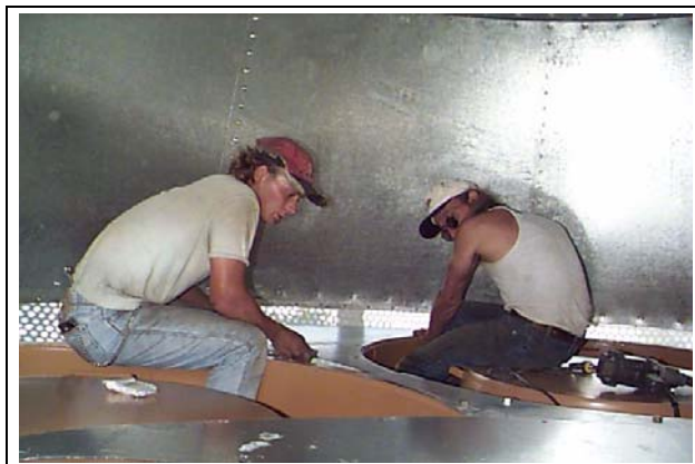
Figure 15AE Bolting fan reducer panel.
