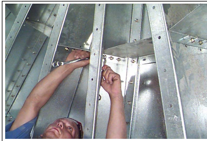
Figure 5AY Hand tightening rafter crossmembers.
