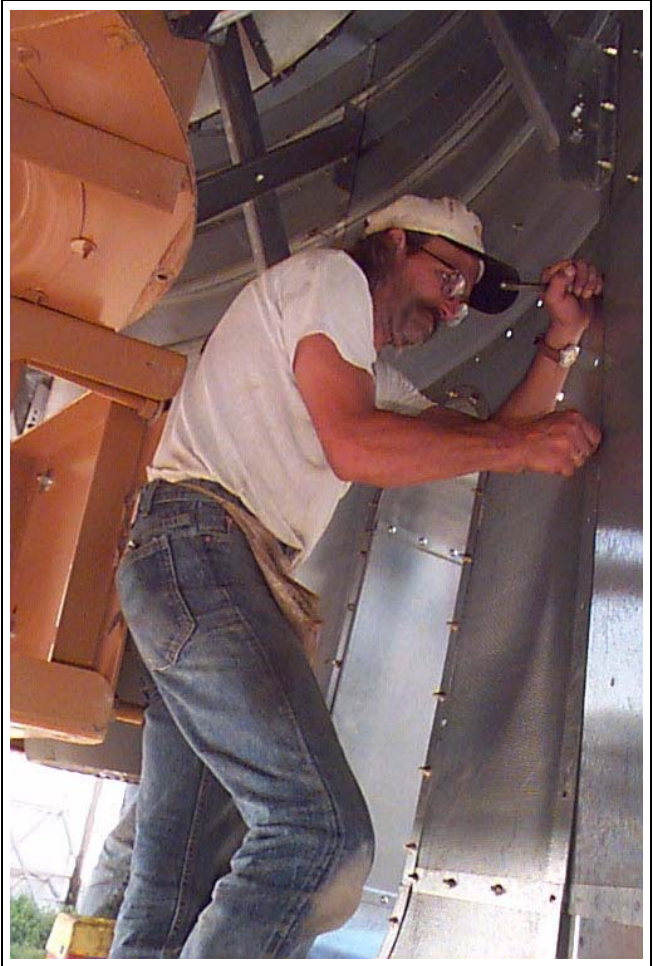
Figure 18T Bolt wall sheets in place. Install rolled plenum channels. Check that window frame is level and square to dryer.
