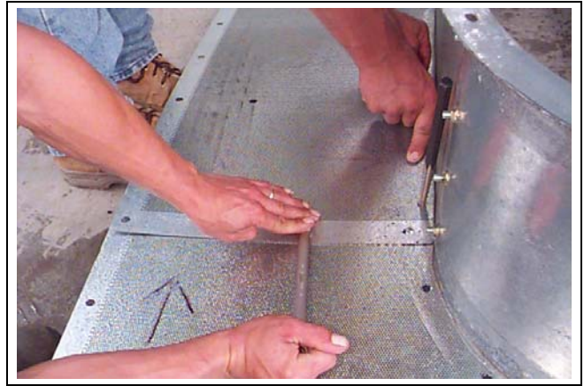
Figure 18P Close Up - Aligning wall sheets to window frame so bolt holes can be drilled. Note wall sheets are installed on top of window frame flange.
