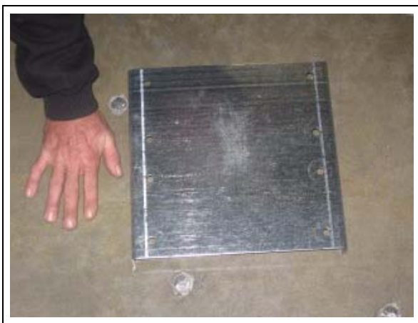
Figure 9A Vertical channel splice, 10 gauge.
