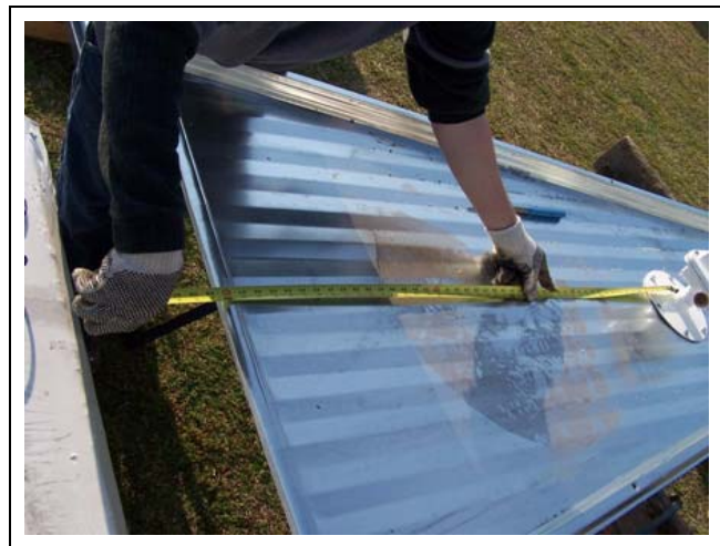
Figure 8K Installing upper bindicator.
