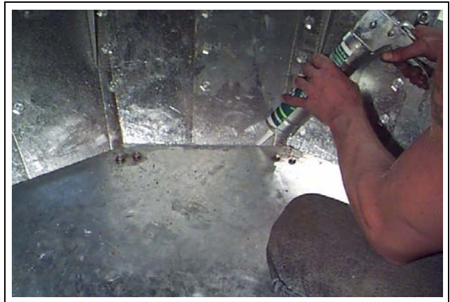
Figure 21AB Caulking metering drum floor with silicone caulk.
