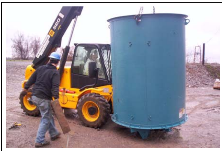
Figure 15T Stand fan up vertical with drive shaft down on dolly.
