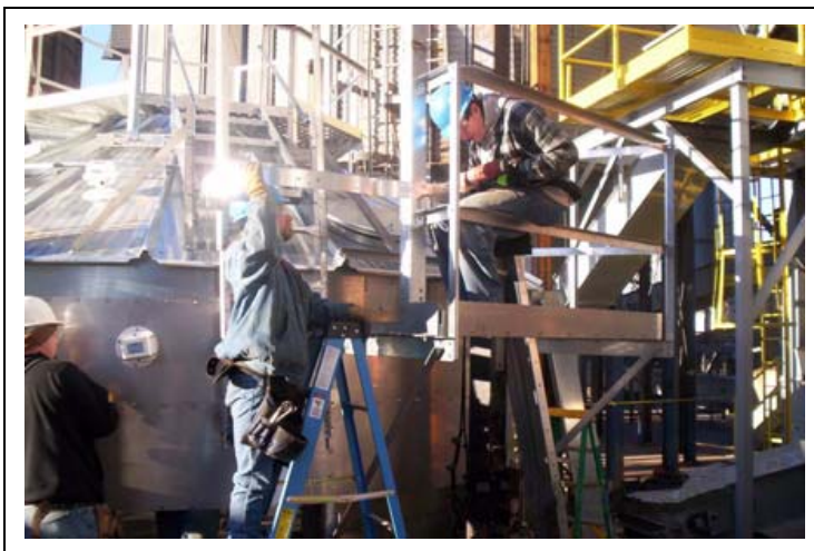
Figure 7R Close up - Installing upper and lower safety hoops to platform vertical supports.
