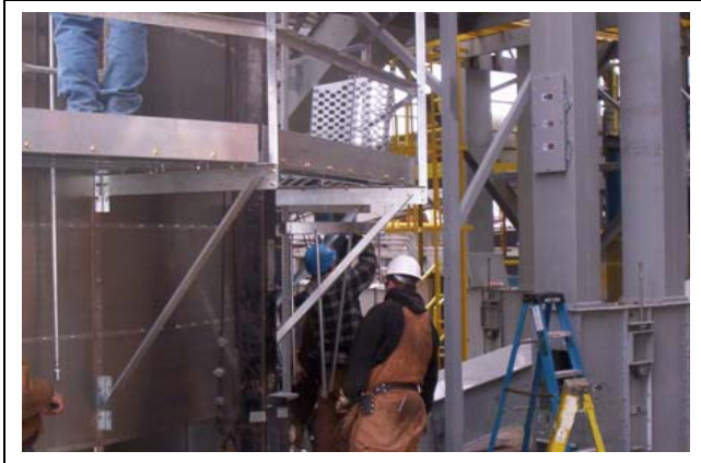
Figure 10U Tightening outside catwalk.
