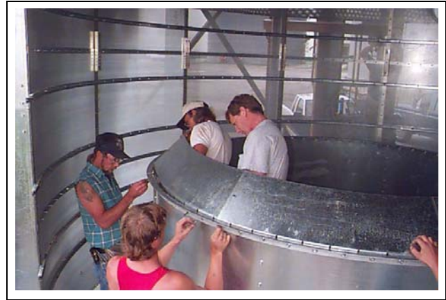
Figure 14J Installing burner housing outlet baffle to top rim of burner housing.
