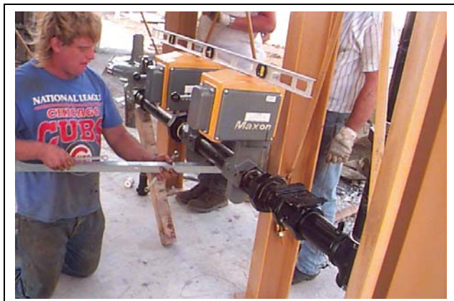
Figure 24W Checking fuel train is level, then measuring for fuel train stands.
