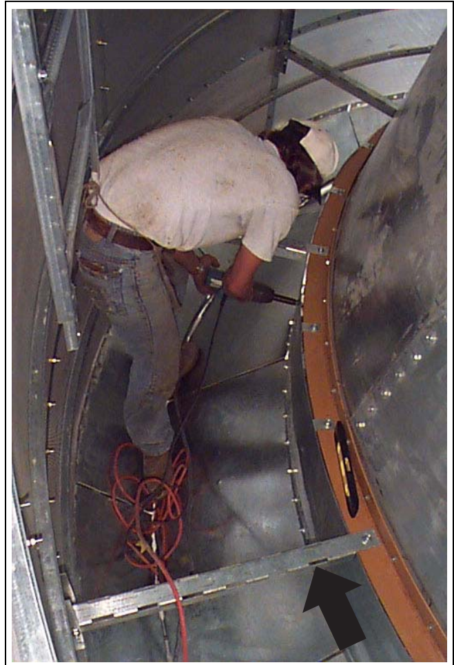
Figure 15BF View from above divider hopper NOTE: Wait to tighten divider hopper and fan skirting until after installing reducer walkway support beam (arrow).
