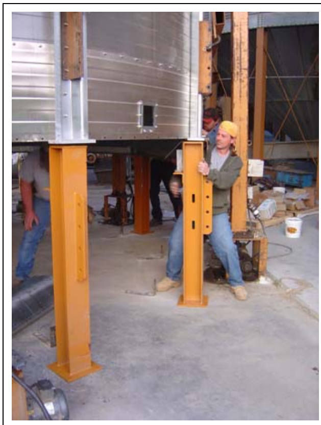
Figure 9P Bolting vertical channel to jig clip.
