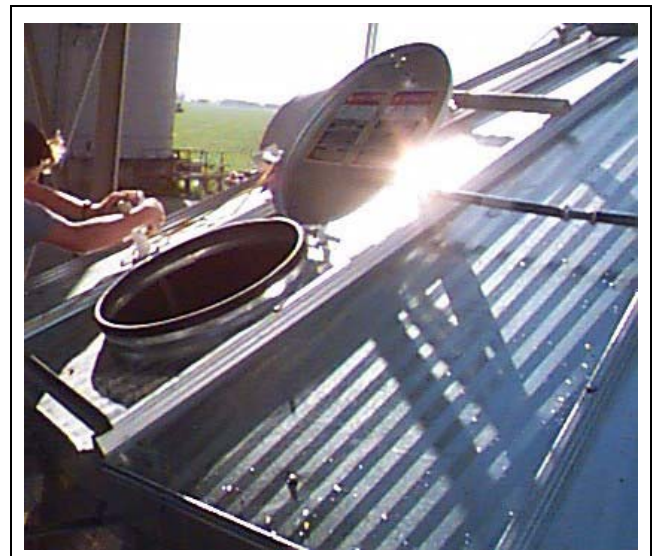
Figure 6AM Outside View - Access port cover installed.
