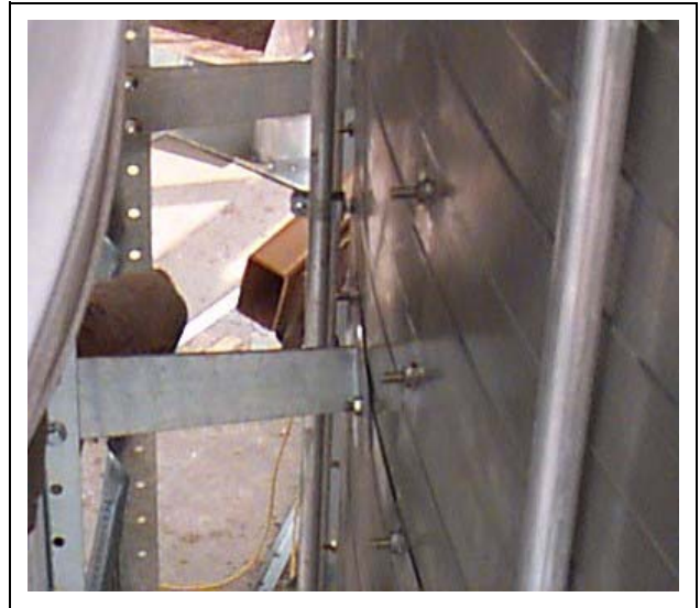
Figure 7N Close Up - Outside Ladder Brackets
