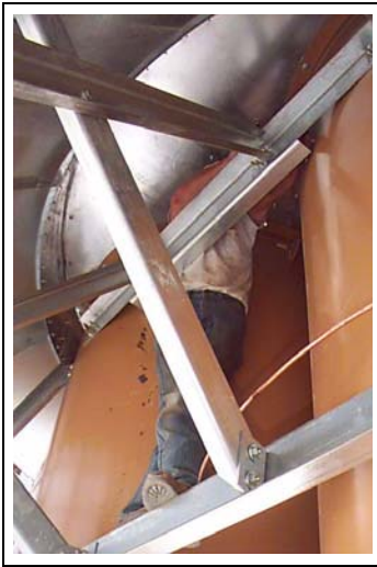
Figure 17E Accessing upper grease zerk.
