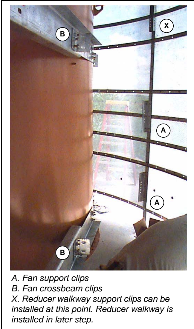
Figure 15AK Clips installed.
