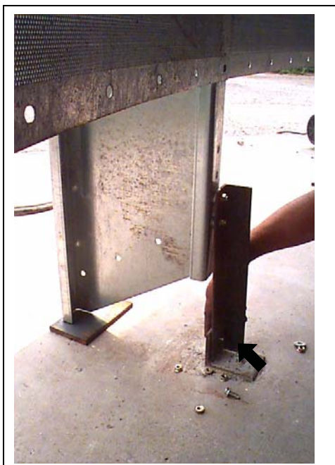
Figure 19E Use jig clips extenders (arrow) to attach vertical base channel to jig clip.
