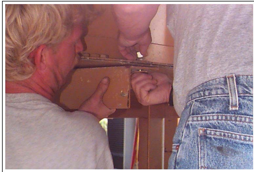
Figure 16E Bolting motor mount to bottom ring of fan.
