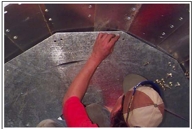
Figure 21AA Close Up - Installing metering drum floor to metering drum floor clips.
