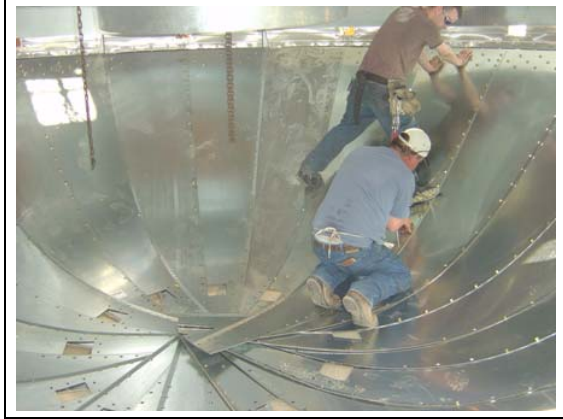
Figure 21Q While installing outside hopper panels, allow ends to overlap at center of dryer.
