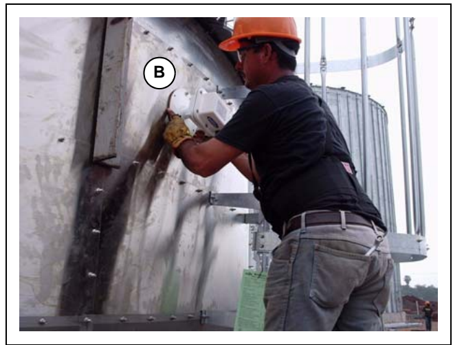
Figure 8L Upper bindicator (A) and lower bindicator (B) installed.
