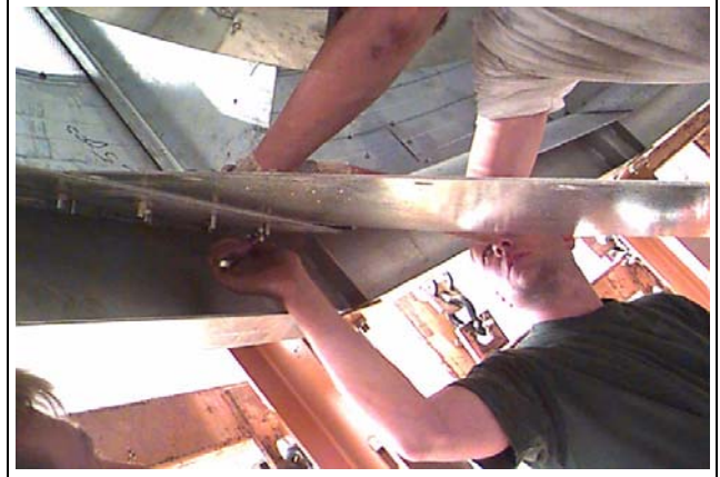
Figure 21N View from below - Bolting outside hopper panels over compression angles and compression angle splices.
