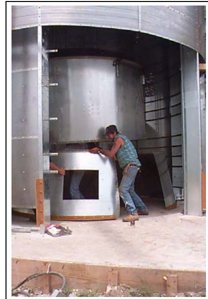
Figure 14Y Orient reducer door cut out so it faces same vertical channel as heat section burner door.
