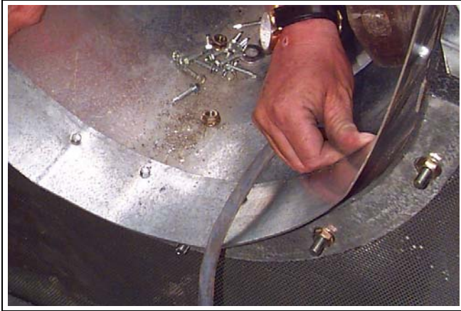
Figure 18AQ Close Up - Installing heat section door sleeve.
