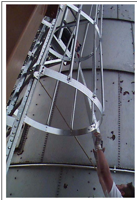
Figure 7V Bell safety cage installed.
