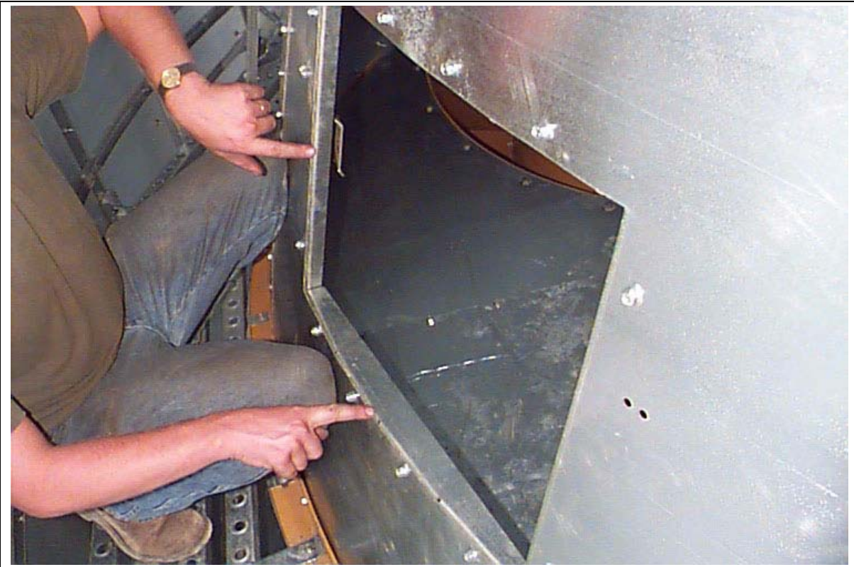
Figure 18BB Front of installed reducer door.
