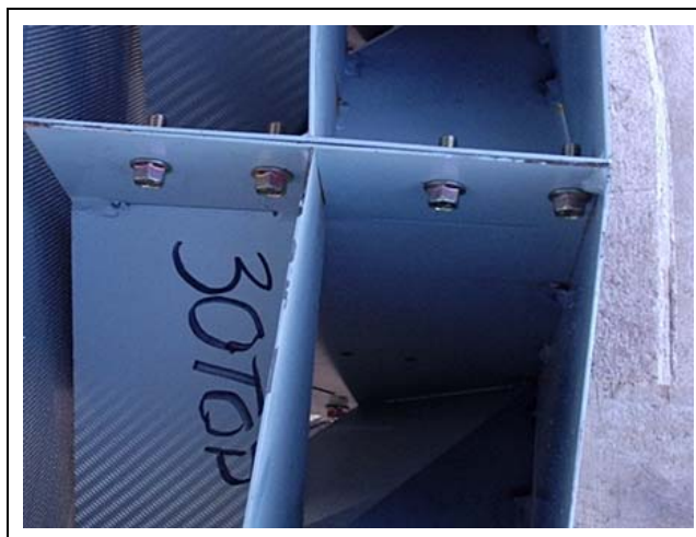
Figure 13D Installing middle grain turner sections.
