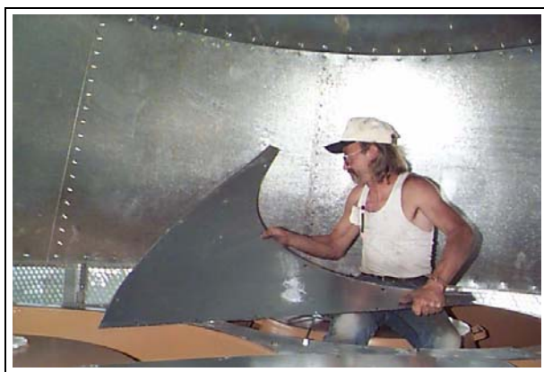
Figure 15AD Positioning fan reducer panel.
