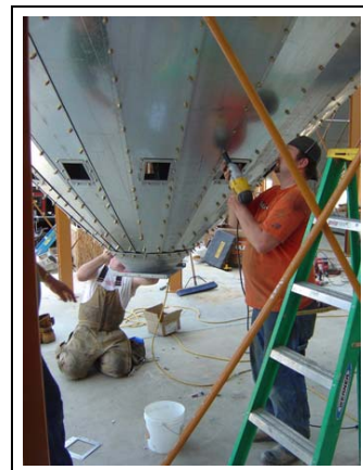
Figure 21V Aligning outside hopper panels before installing hopper discharge weldment.
