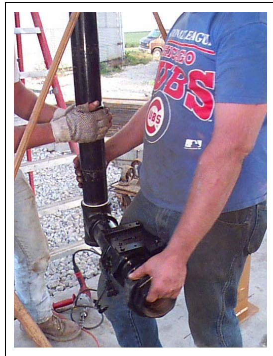
Figure 24R Connecting modutrol section to fuel pipe.
