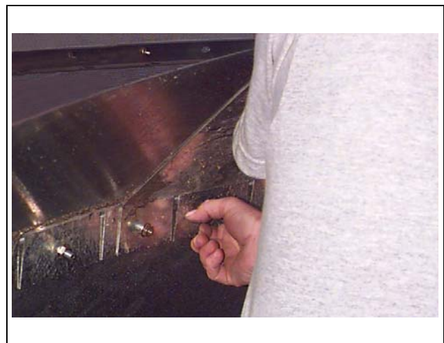
Figure 14K Close up inside burner housing - Installing burner housing outlet baffle to top rim of burner housing.
