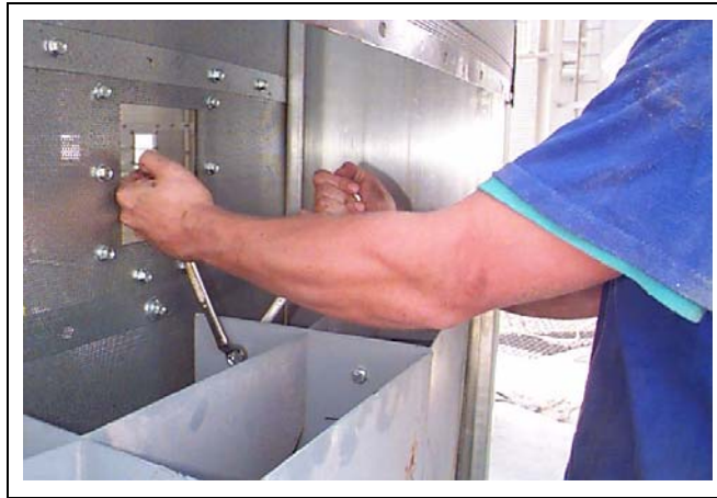
Figure 13E Tightening grain turner sections.
