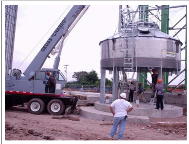
Figure 9J Raising Dryer (Crane shown here).
