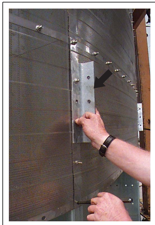
Figure 10S Catwalk support clip is installed with angle up on R.H. side.
