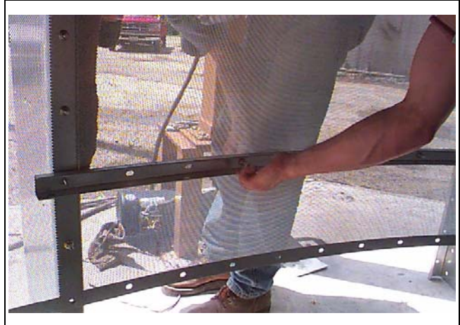
Figure 4X Close Up - Installing rolled plenum channels.
