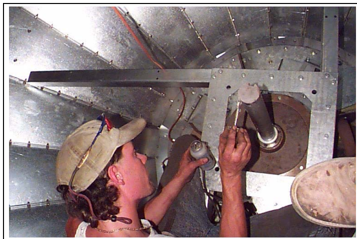
Figure 22T Applying anti-seize to top of metering drum drive shaft before installing gearbox.
