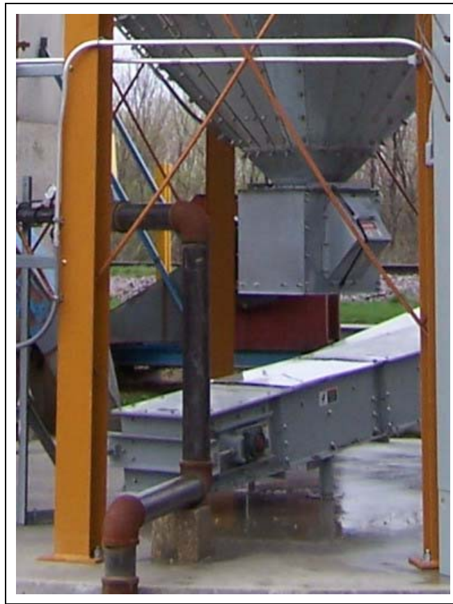
Figure 10AA Dry Sensor Installations at GSI Tower Dryer
