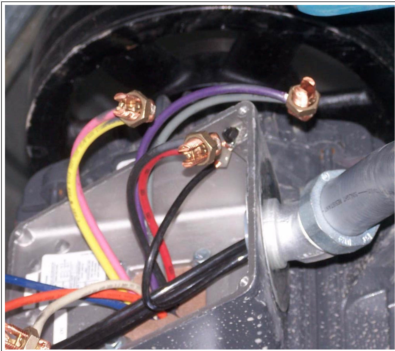
Figure 5L Connections (split bolt connectors) wrapped in electrical tape, then in mastic tape.
