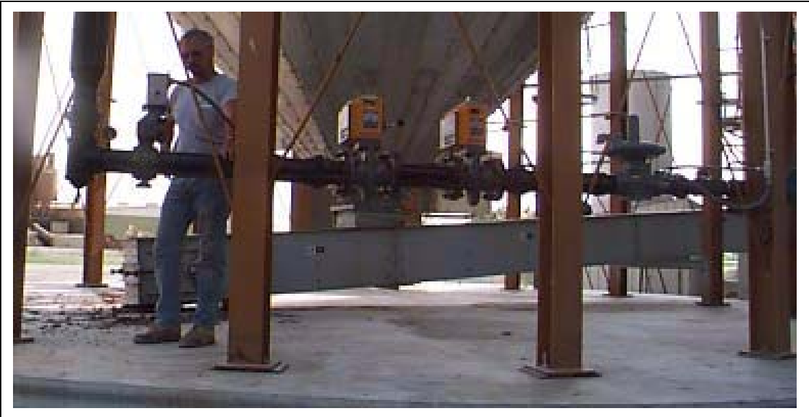
Figure 12AD Fuel Train on 2000 BPH Dryer.
