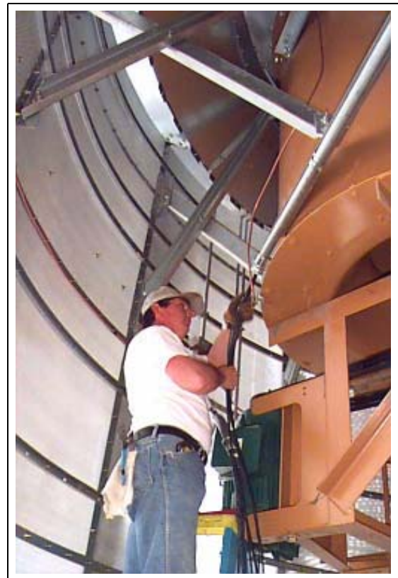
Figure 5K Drill hole in angle iron for mini clamp.
