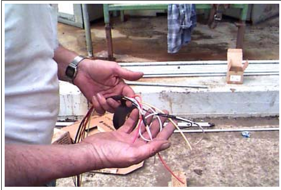
Figure 4AH Pairing off wires for pilot fuel train.
