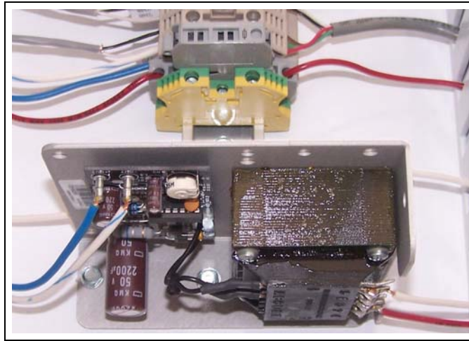
Figure 10V Moisture Sensor Power Supply and Terminal Strip Locations
