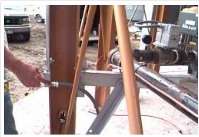
Figure 12S Running Flexible Conduit
