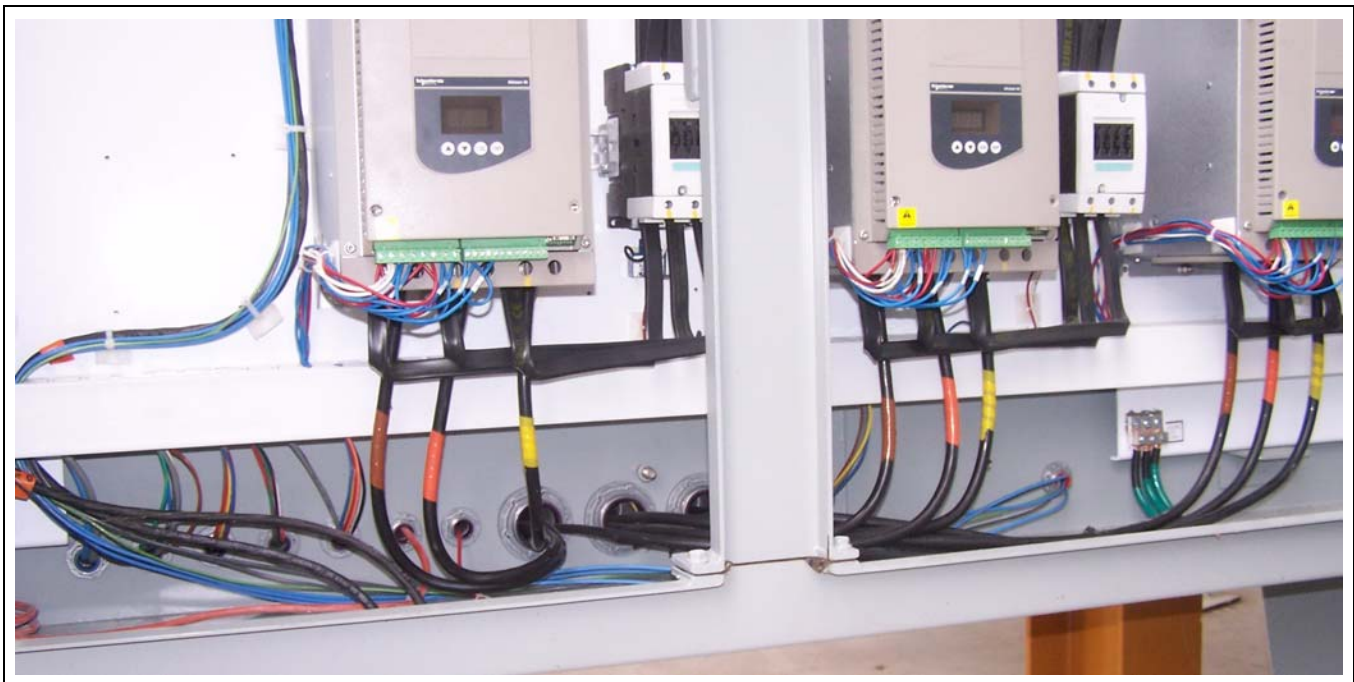
Figure 4V Interior View of Power Box - With myers hubs installed to knock outs.
