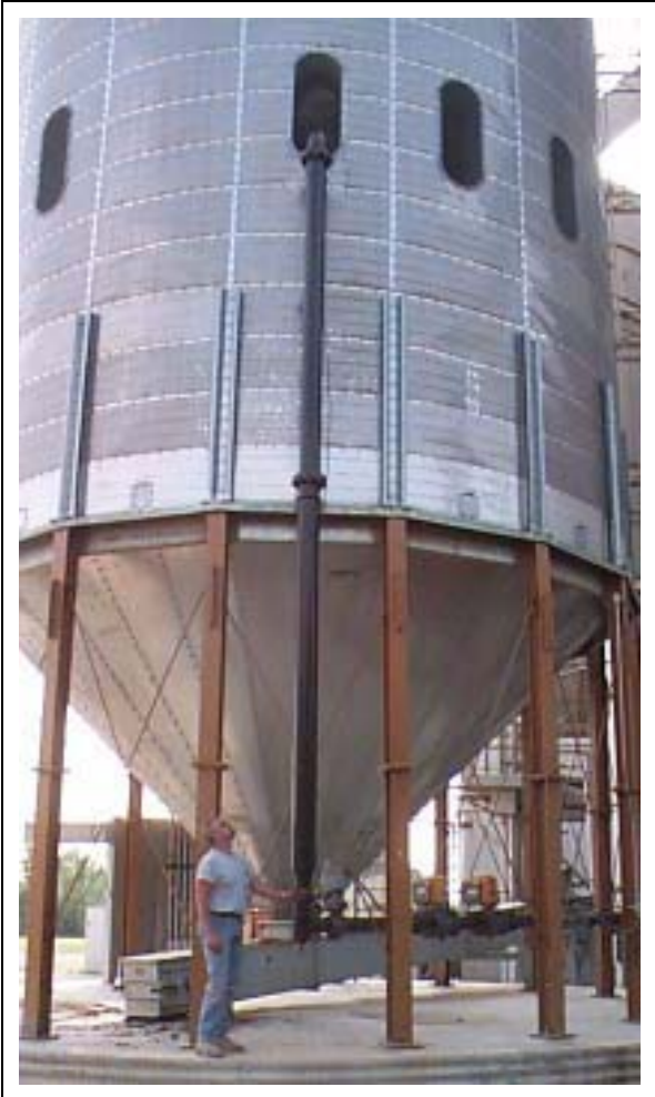
Figure 12AC Fuel Piping and Pilot Fuel Piping
