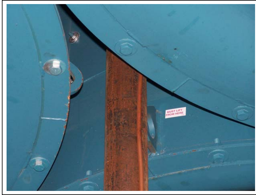
Figure 12AH 3/8" Pilot fuel copper tubing up through center of 3 fan dryer.
