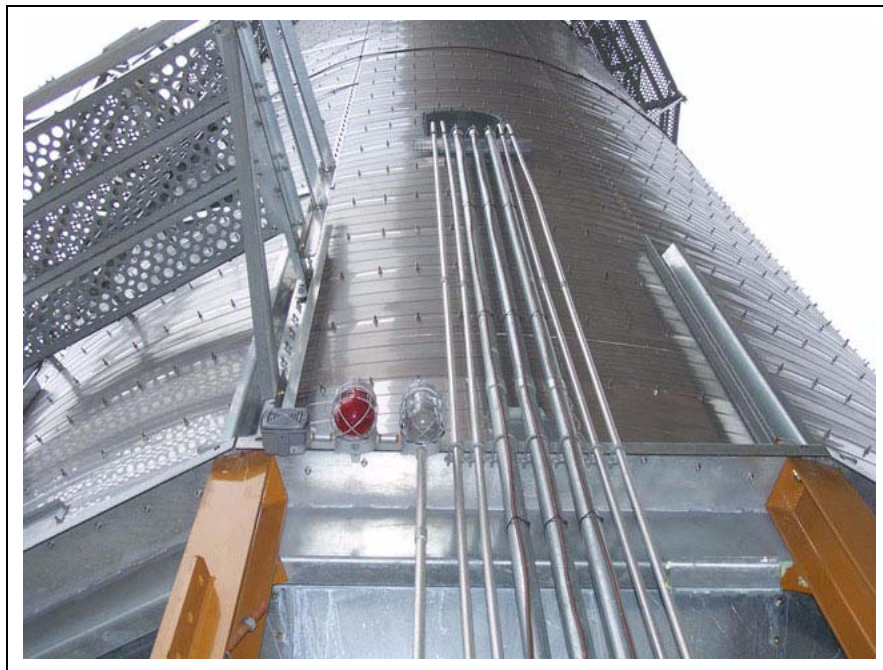
Figure 6K Air Switch Tubing Installed
