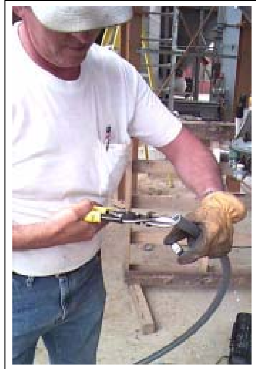
Figure 12AA Cutting Seal-Tight
