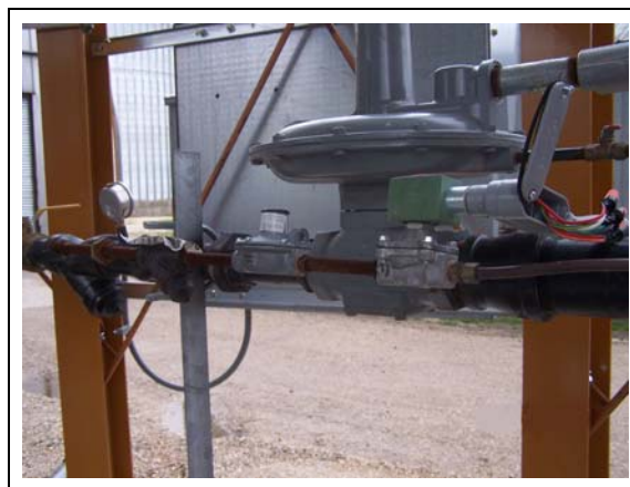
Figure 12AG Pilot fuel train installations almost completed.
