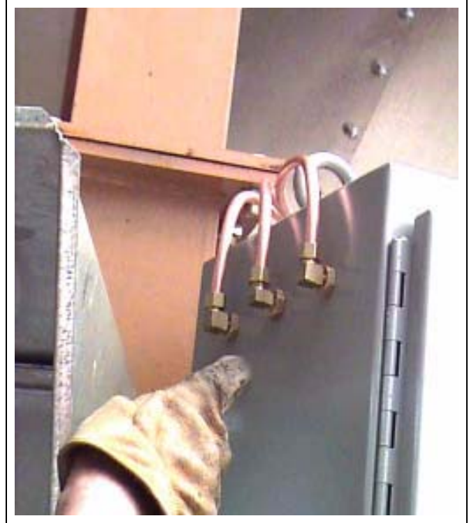
Figure 6J Brass connectors connect 3/8" copper tubing to air switches.
