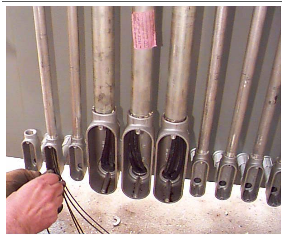
Figure 4AI Close Up - Pulling wires from rear of power box.
