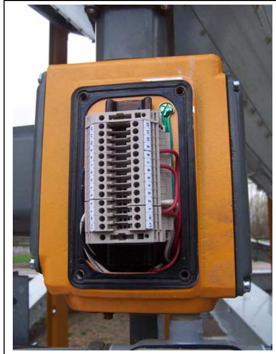
Figure 12V Standard Wiring for Primary/Upstream Electronically Controlled Maxon
