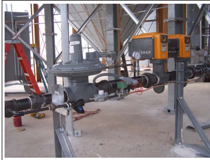
Figure 12AE Standard Pilot and Fuel Trains Securely Mounted
