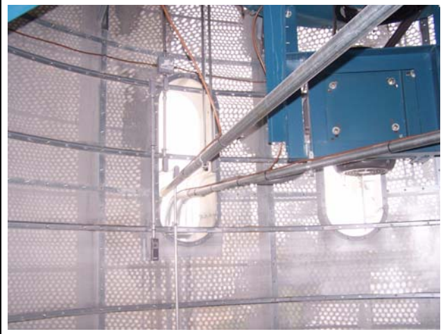
Figure 6B L.H. View - Fan motors wired and air switch tubing installed.
