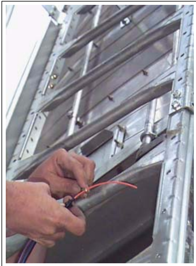
Figure 4AJ Tying wire to fish tape prior to pulling it through conduit.
