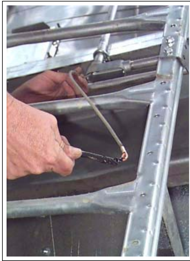
Figure 4AK Pulling wires to exterior high-limits.
