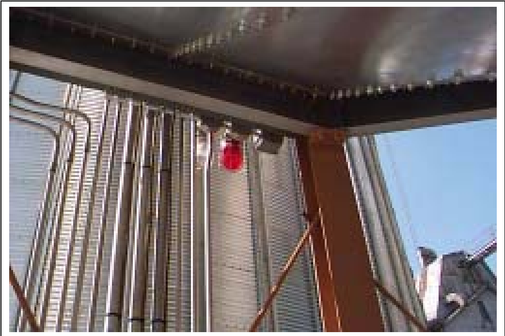
Figure 13C Rear View - Lights and safety package installed on 3 fan dryer.
