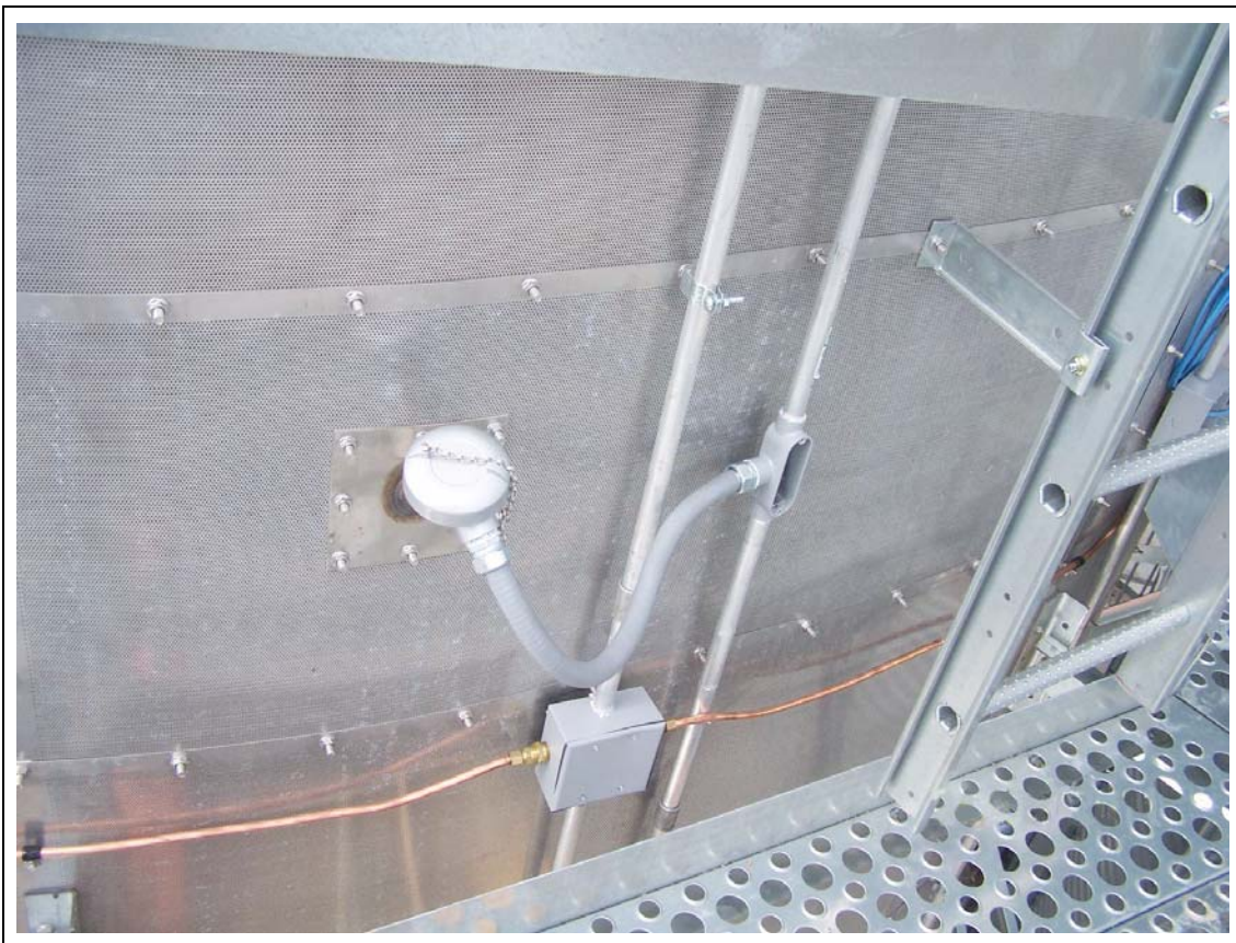
Figure 10L Grain RTD mounted and conduit tee with seal-tight completed and tight.
