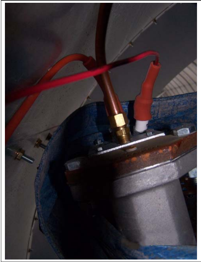
Figure 12N 3/8" Compression fitting completed from maxon pilot port continuing at 3/8" pilot fuel.
