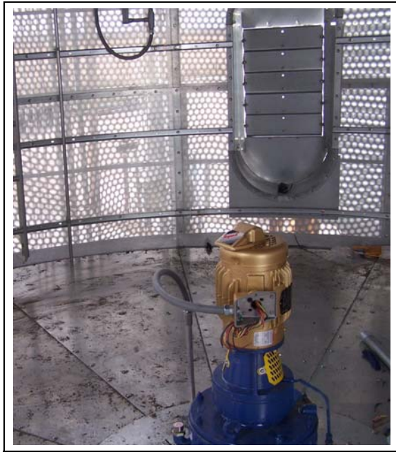
Figure 7B Typical conduit installations for a Zimmerman unload system.
