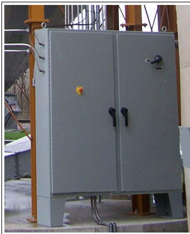
Figure 4L Power Box Installed (3 Fan Dryer).
