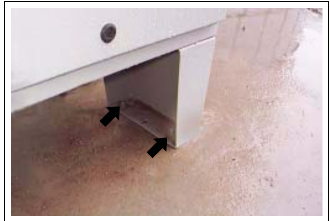
Figure 4J Heavy duty expanding anchor bolts (red heads) anchor power box to dryer foundation.
