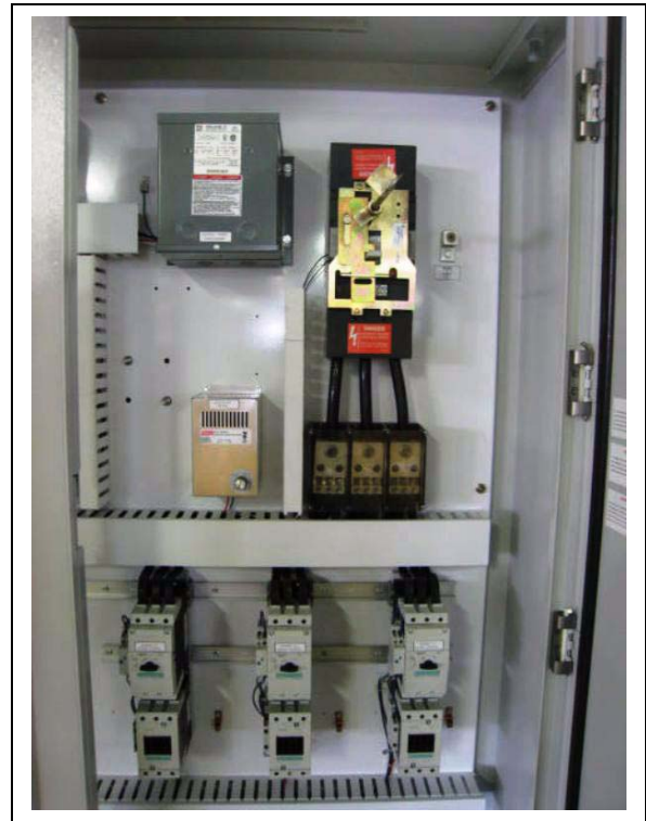
Figure 4F Close Up - Blower motor starters (for 4 fan dryer) as shipped.
