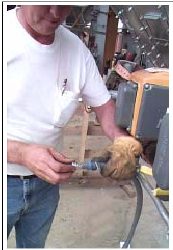
Figure 12AB Attaching Seal-Tight Fitting to Seal-Tight
