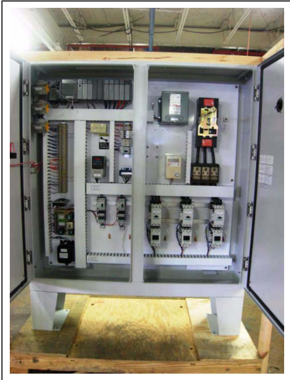
Figure 4C Interior of Power Box
