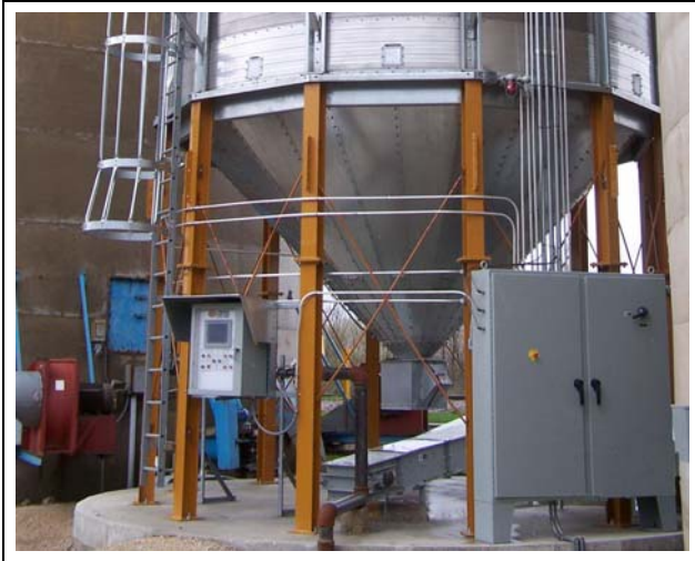
Figure 4Q Front View - Conduit installed on 4 fan dryer.
