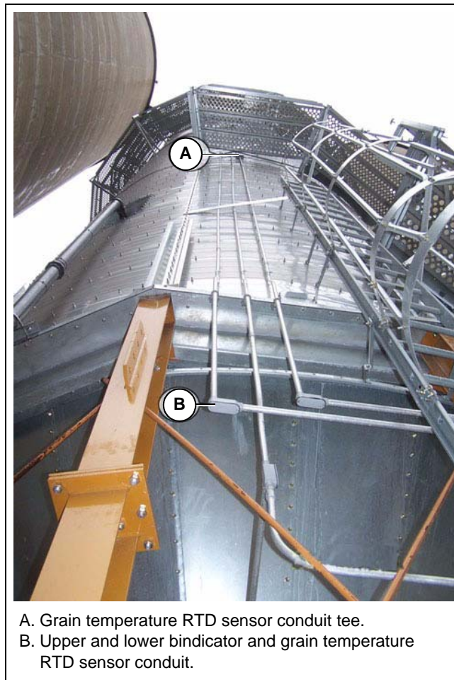
Figure 10J Installing conduit tee on bindicator conduit for grain temperature sensors cables.
