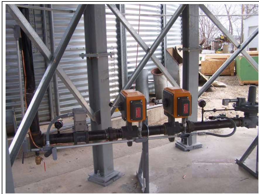
Figure 12U 1/2" Fuel and Pilot Conduit Installed
