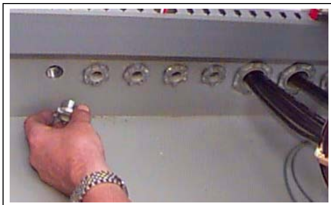
Figure 15B Weather-tight Myers Hub - Portion installed inside power box.
