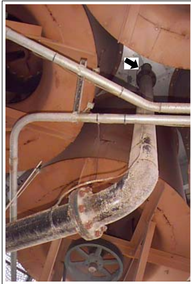
Figure 12AI Pilot fuel train piping and fuel piping runs up through divider hopper.
