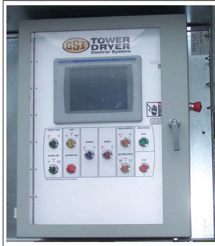
Figure 4K Control box with electronic monitoring control system installed.
