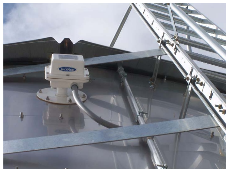
Figure 10F One option available for installations. Lower bindicator.
