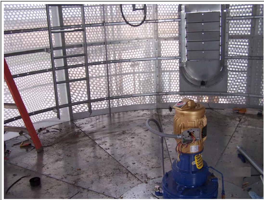
Figure 7F Typical Zimmerman Style Unload Metering Device Installations
