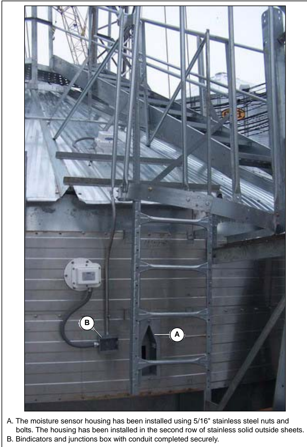
Figure 10Z Tower Dryer Roof Sections with Bindicators and Wet Sensor Housing Mounted
