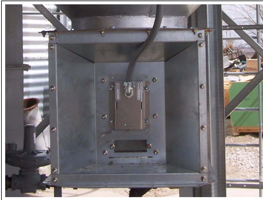
Figure 10AI Zimmerman Tower Dryer
