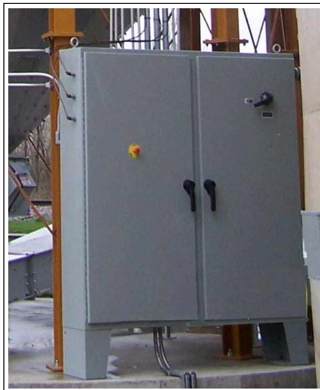
Figure 4L Power Box Installed (3 Fan Dryer).
