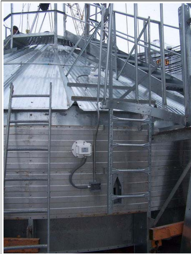
Figure 10G Typical install at bindicator's with the wet moisture = Sensor housing installed.
