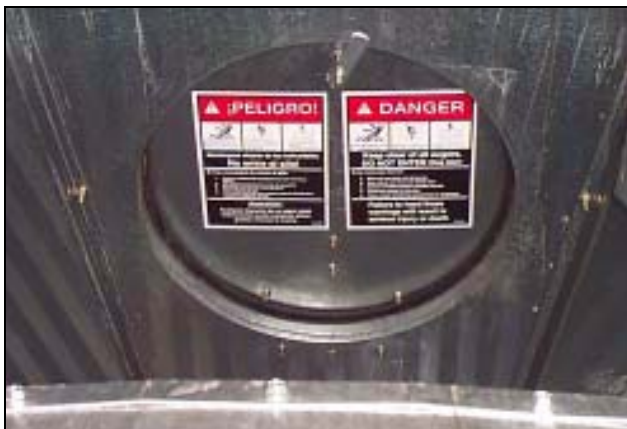
Hatch door with decals in place.
