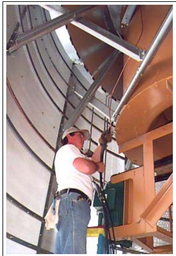
Figure 5K Drill hole in angle iron for mini clamp.
