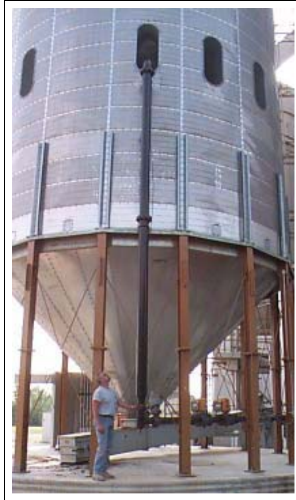
Figure 12AC Fuel Piping and Pilot Fuel Piping
