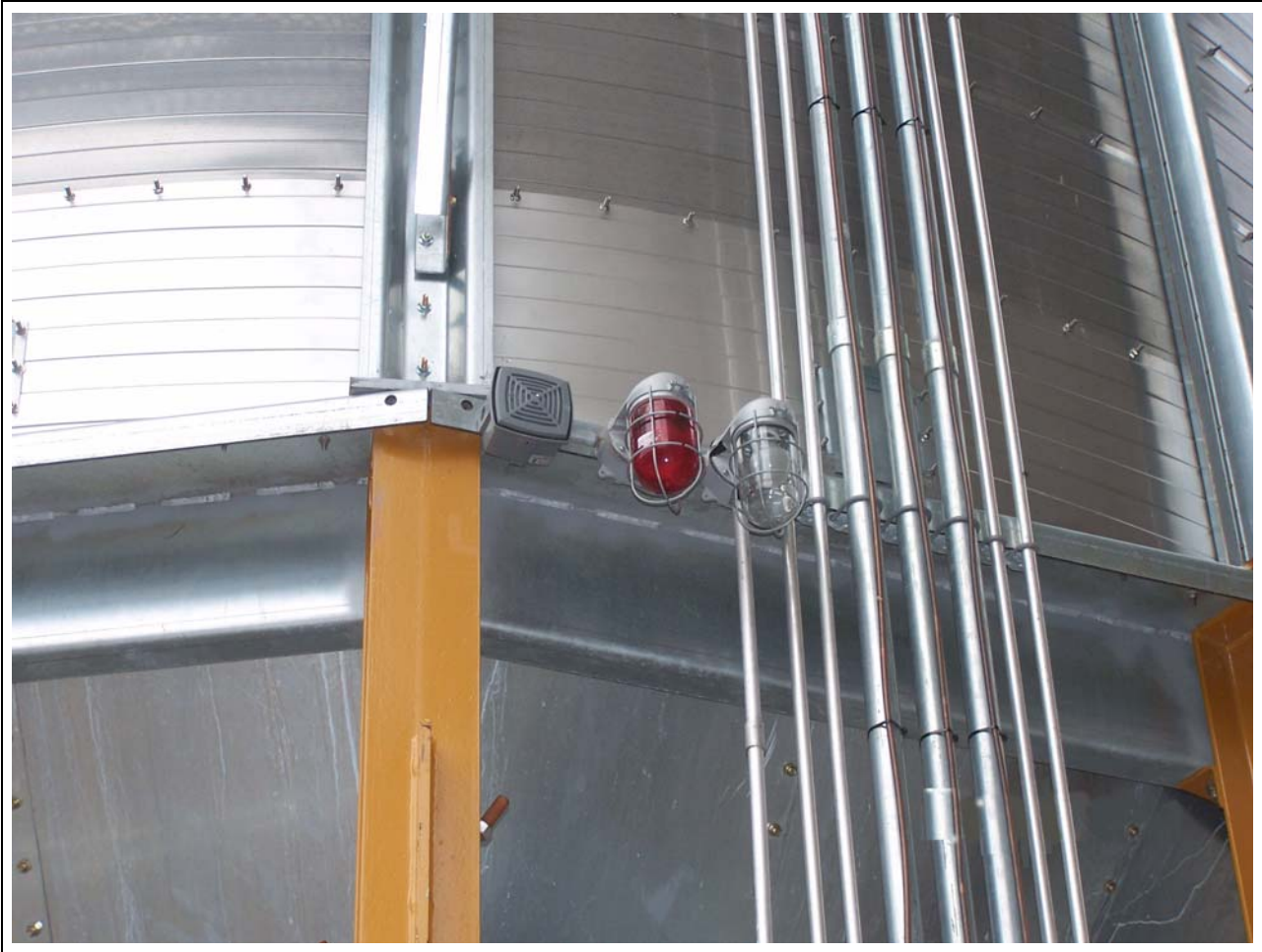
Figure 13B Front View - Lights and safety package installed on 3 fan dryer.
