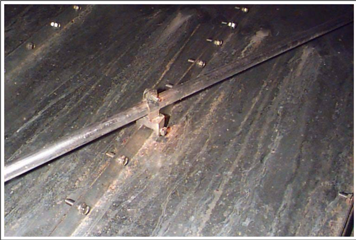
Figure 7I Close Up - Beam Clamp
