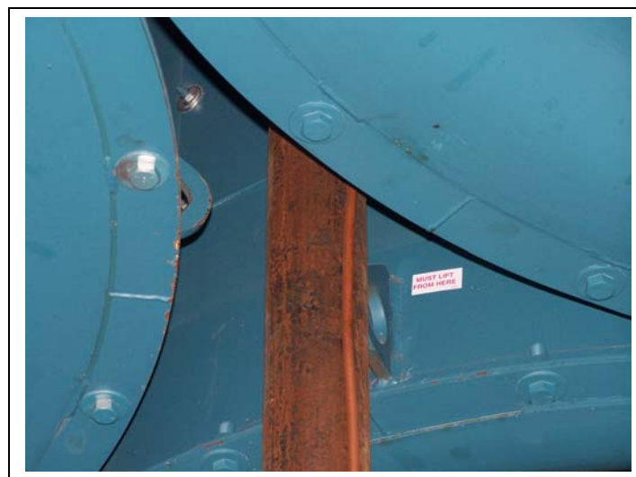
Figure 12K Pilot copper tubing continuing inside dryers cooling section and up through the fan/blowers to the terminations point in the burner. NOTE: Notice un-painted pipe line.
