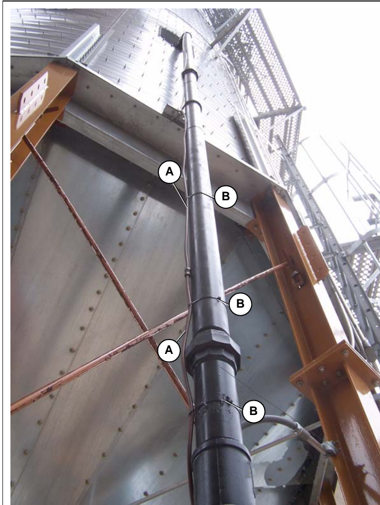
Figure 12J Completed 3/8" copper pilot tubing and 4" natural gas pipe. All attached securely and fresh paint complete a tower dryer fuel train.
