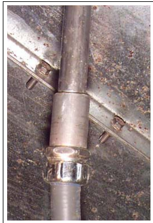
Figure 7K Liquid-Tight Conduit Straight Connector
