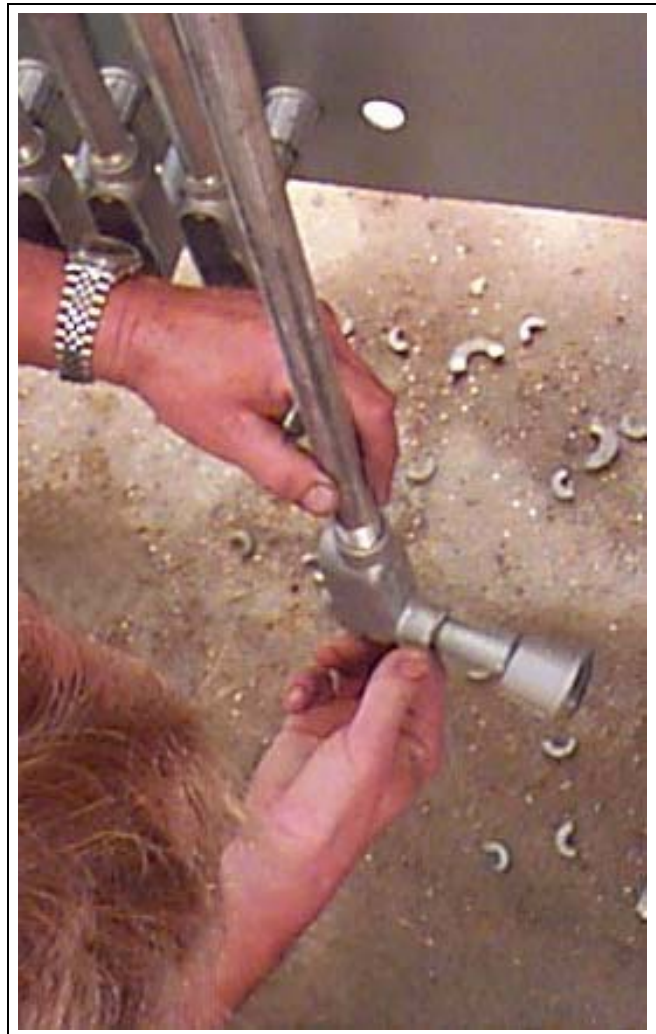
Figure 15C Weather-tight Myers Hub - Portion installed to rear of power box (connects to portion inside power box).
