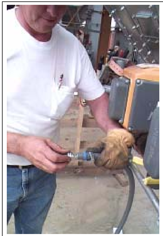
Figure 12AB Attaching Seal-Tight Fitting to Seal-Tight
