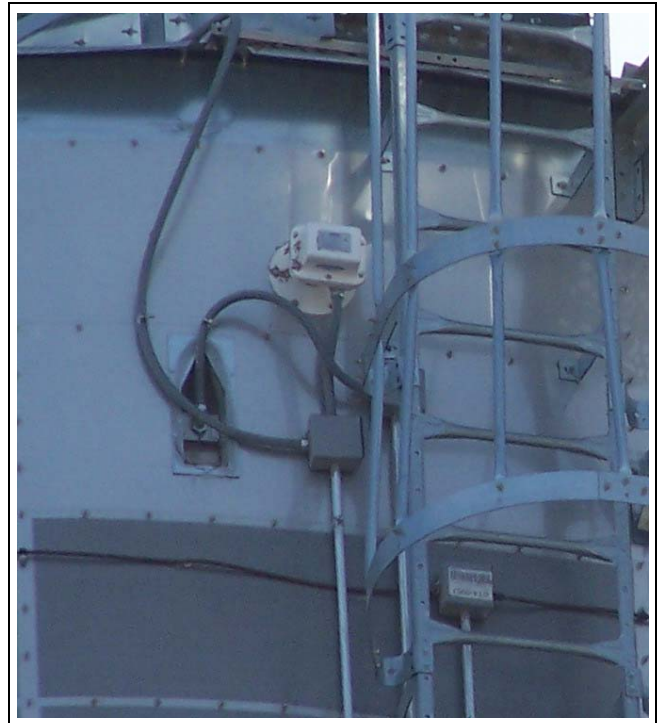
Figure 10H Excessive length's of flex seal-tight conduit is discouraged.
