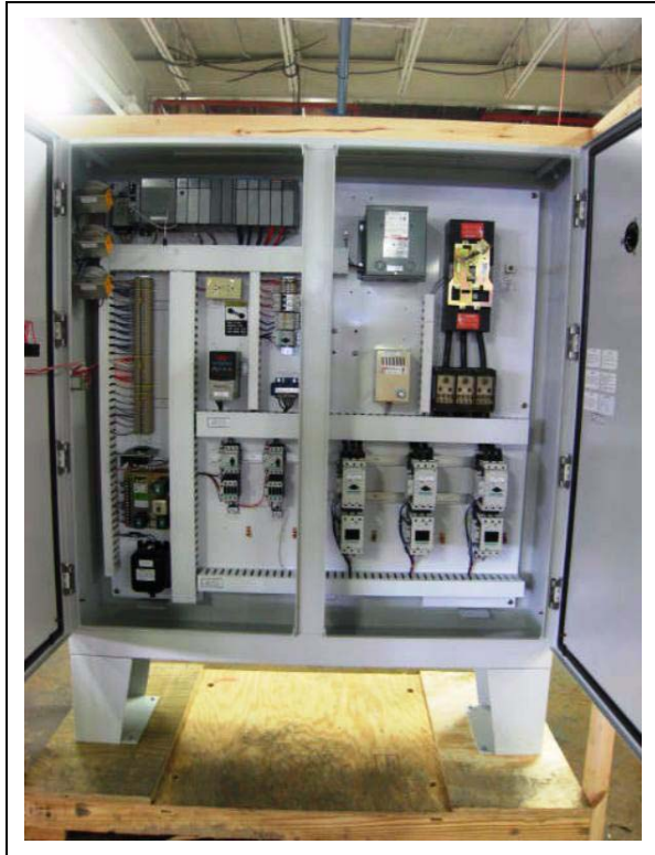
Figure 4C Interior of Power Box
