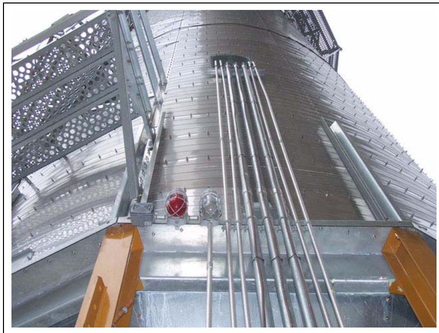
Figure 6K Air Switch Tubing Installed
