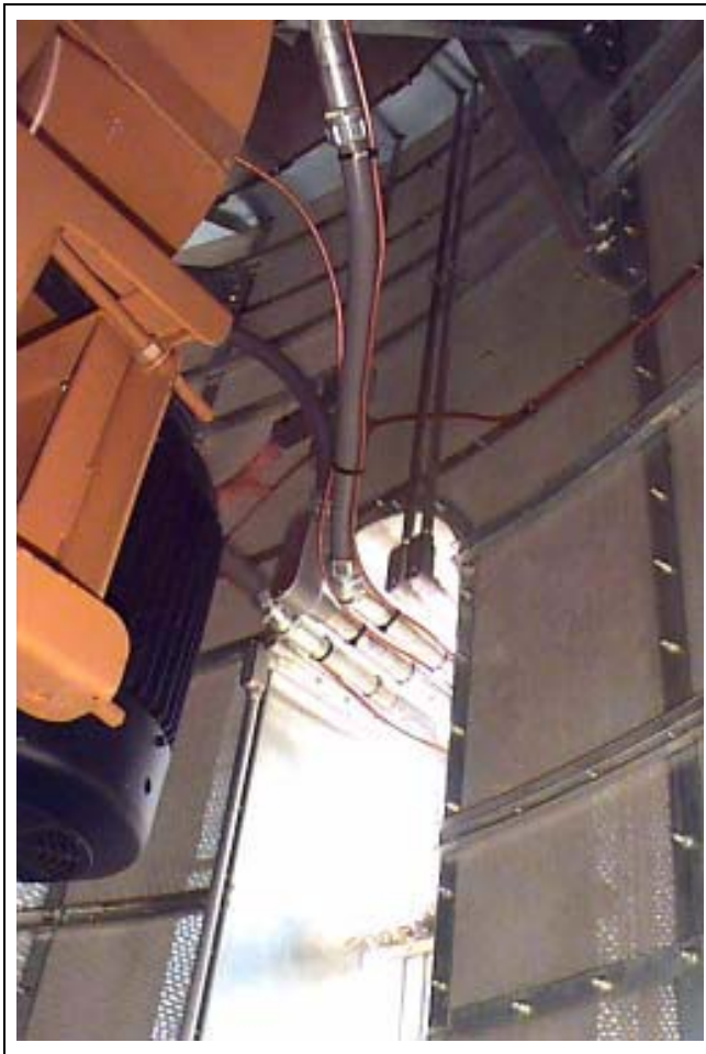
Figure 6C R.H. View - Fan motors wired and air switch tubing installed.
