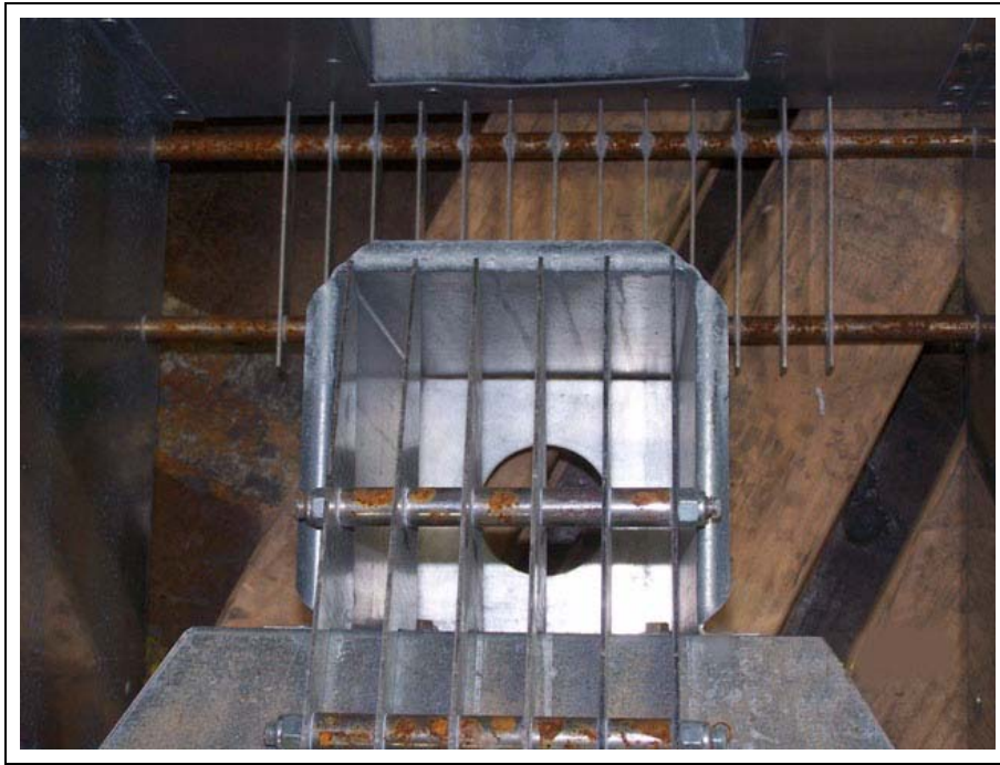
Figure 10AG Sensor basket with gate and grills installed.
