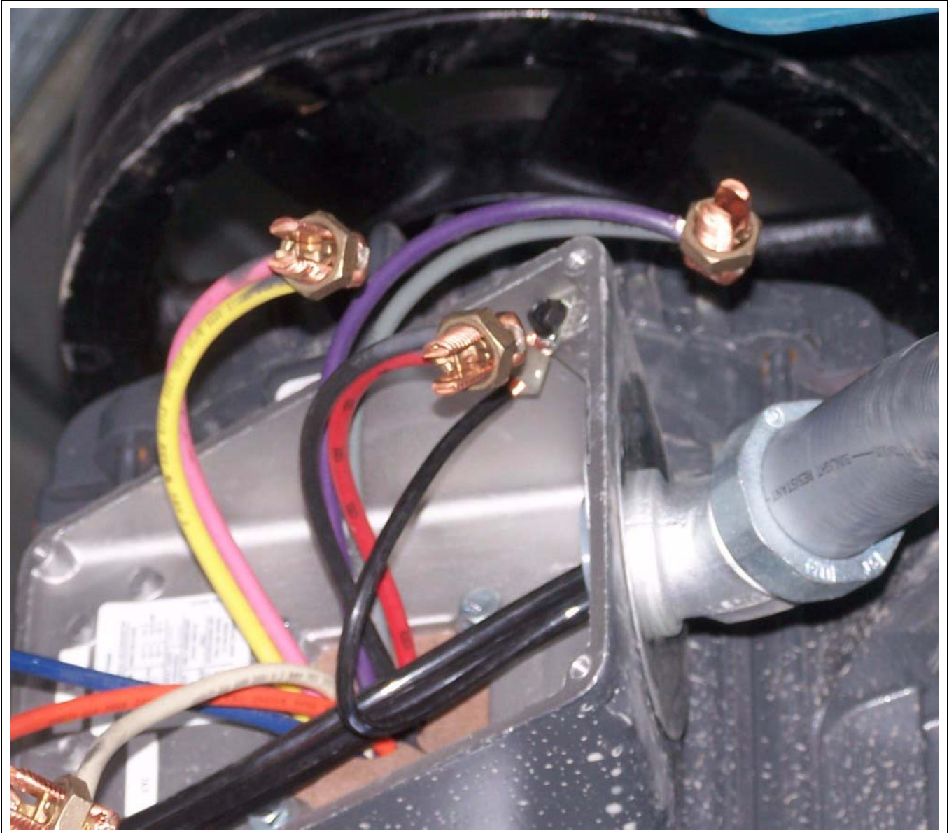
Figure 5L Connections (split bolt connectors) wrapped in electrical tape, then in mastic tape.
