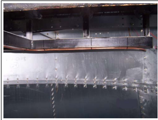
Figure 12M Running 3/8" pilot fuel line up along burner manifold to connecting point in burner pilot section. Wire tie.
