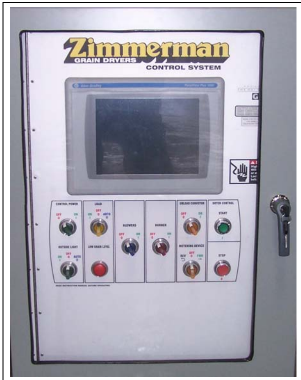
Figure 4D Interior of control box with electronic monitoring control system.
