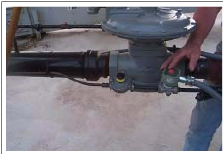
Figure 12AF 3/8" Pilot Copper Tubing Secured to Fuel Train
