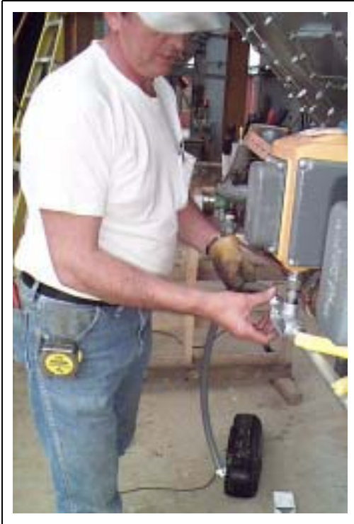
Figure 12Z Attaching seal-tight to conduit tee on maxon valve.
