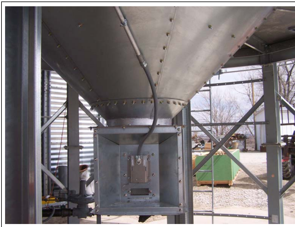
Figure 10AB Dry Sensor Installations at Zimmerman Tower Dryer
