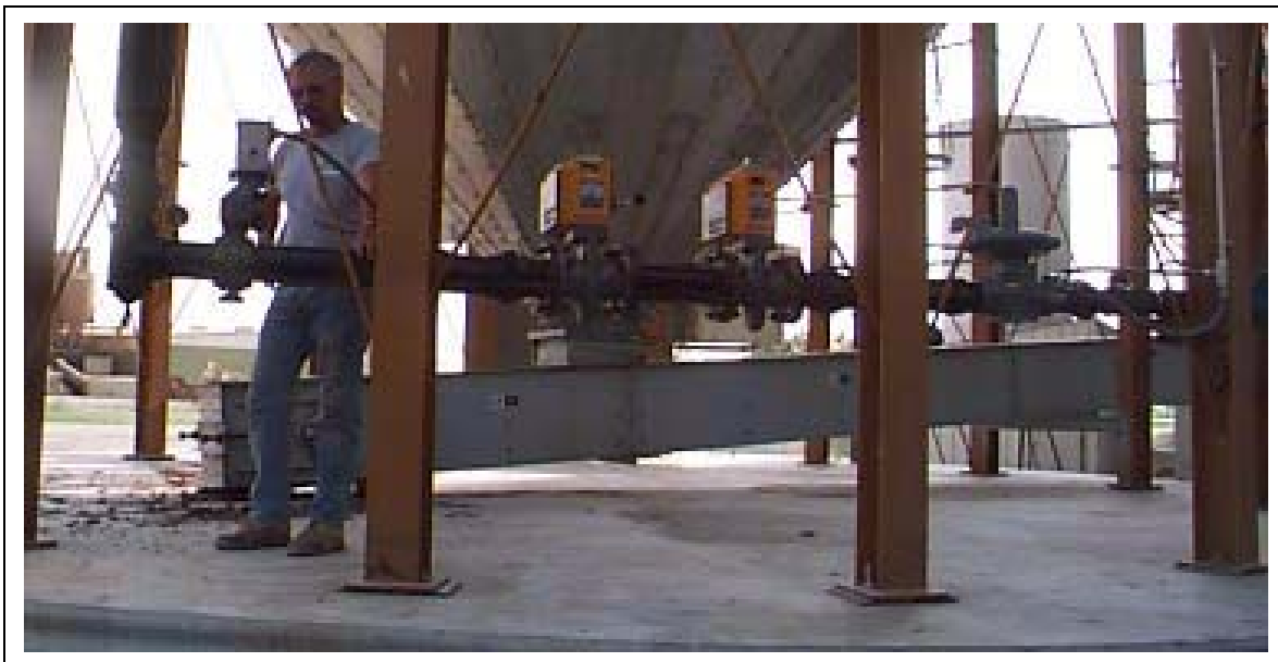
Figure 12AD Fuel Train on 2000 BPH Dryer.
