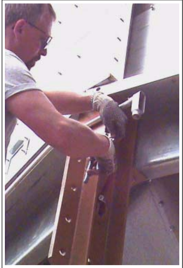
Figure 12T Putting kon clamp on conduit.
