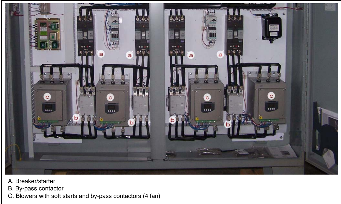
Figure 4N Close Up - Power Box Wired
