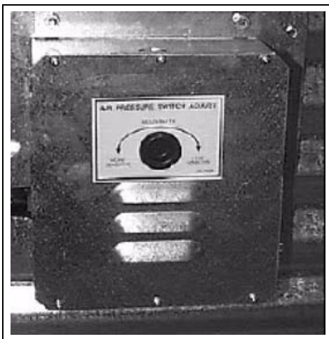
Figure 11B Air Switch Adjustment
