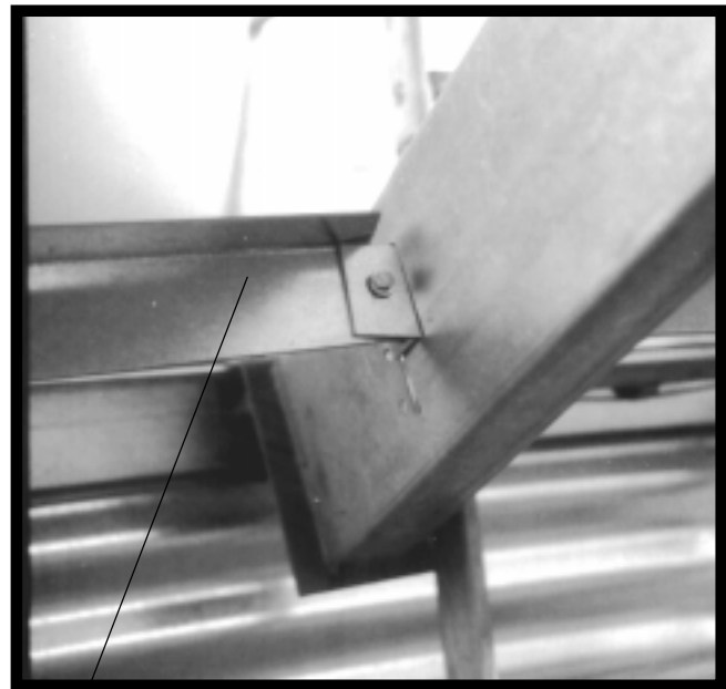
Floor Support Angle Assembly
