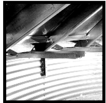
Chutes in closed position
