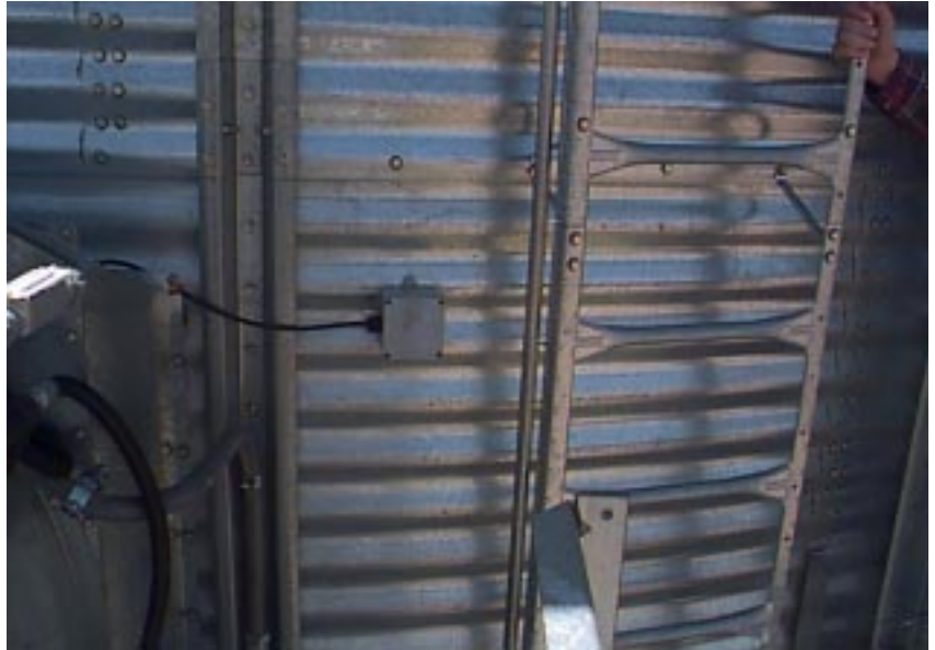
Plenum temperature sensor on the bin sidewall.
