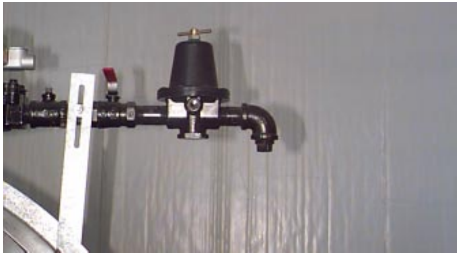
NG line field connection.
