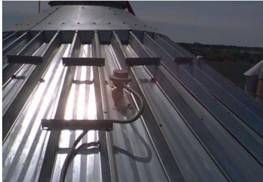
Drying chamber overflow rotary switch.
