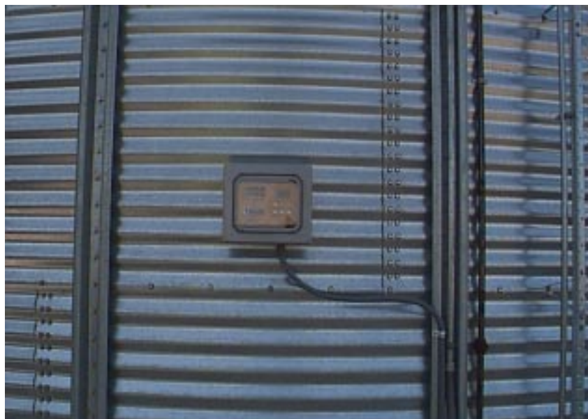
Control box mounted on bin.
