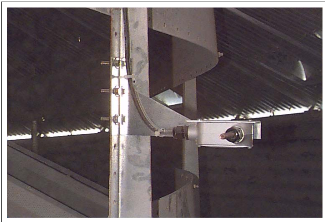
Figure 3D Grain Temperature Sensor Bracket Mounted on Leveling Band Post
