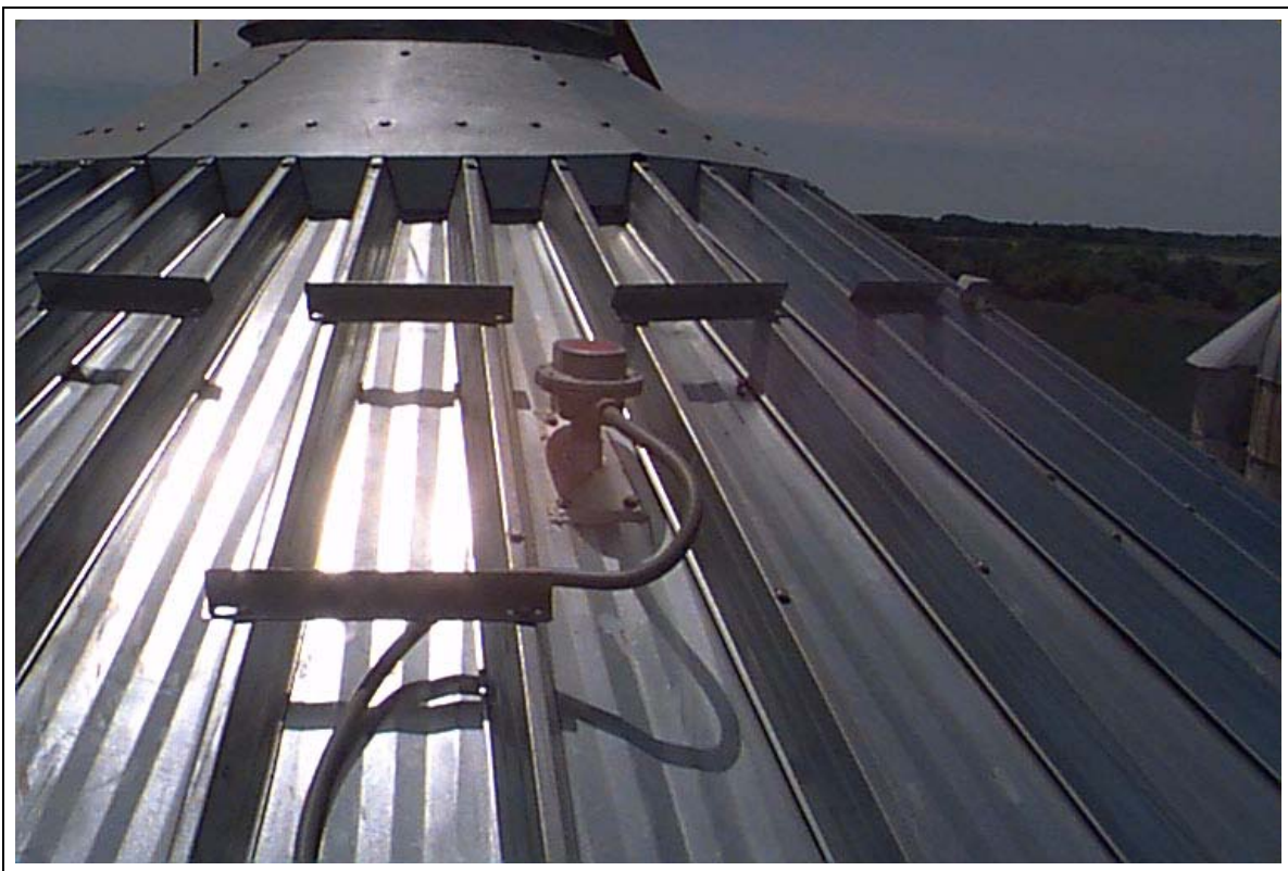
Figure 3K Drying Chamber Overflow Rotary Switch
