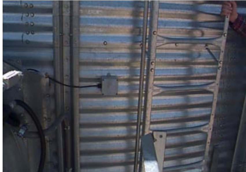
Plenum temperature sensor on the bin sidewall.
