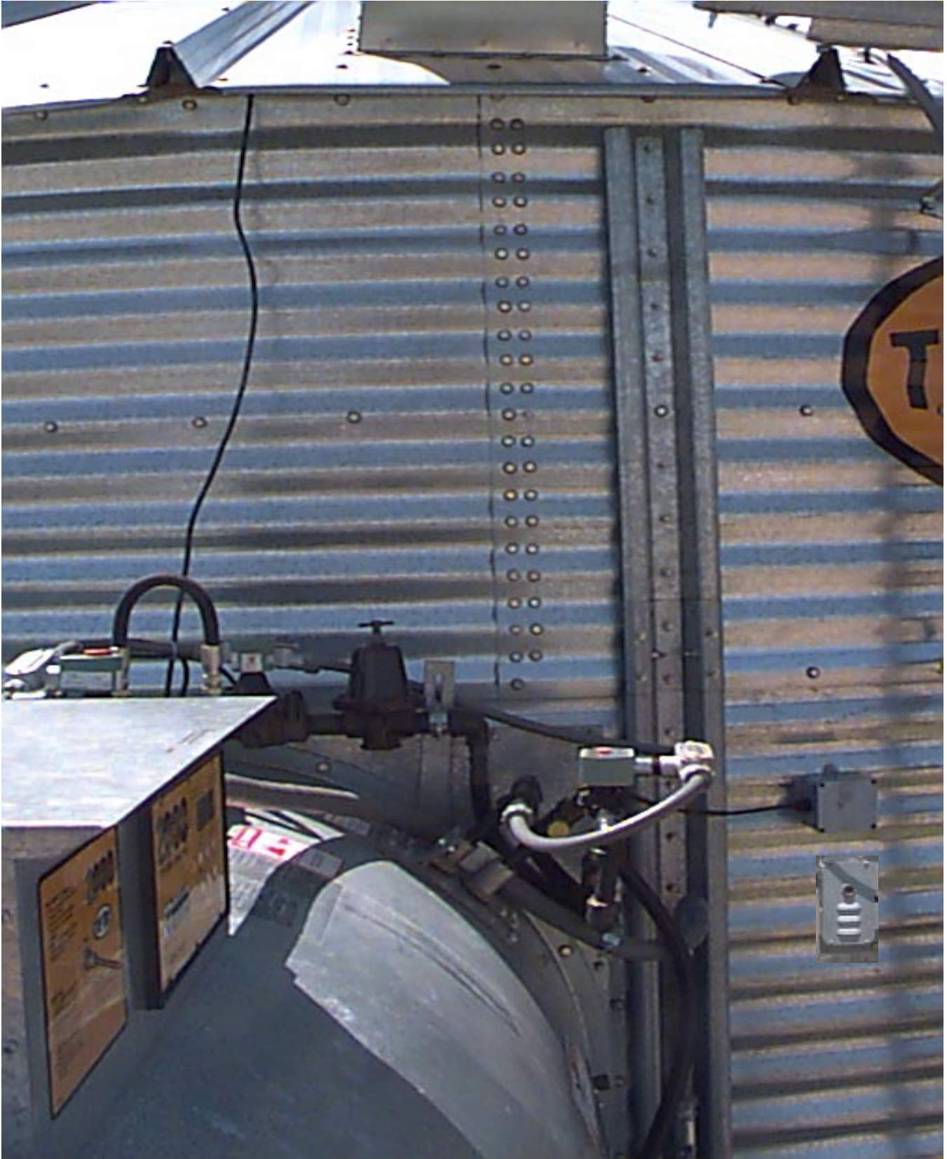
Fan/heater unit mounted to the bin, showing the plenum high limit, the airswitch, and cord going through the eave to the grain temperature sensor bracket.
