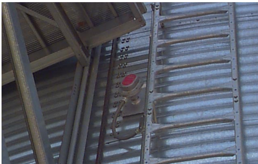
Storage chamber rotary switch.
