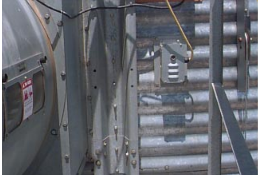
Airswitch mounted on the bin sidewall.
