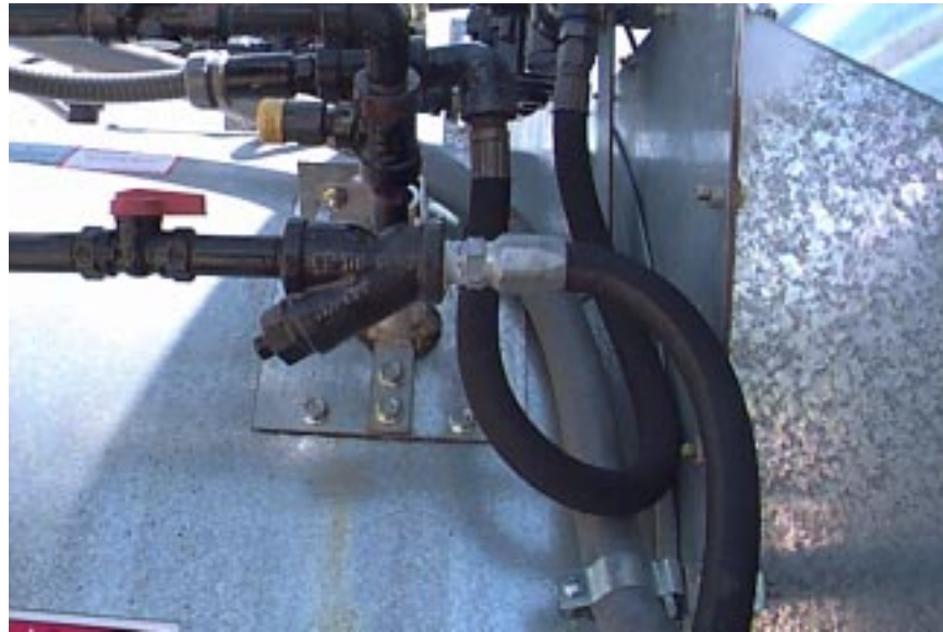
LP line field connection.
