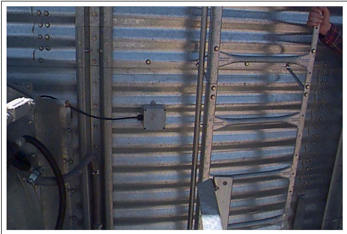
Figure 3J Plenum temperature sensor on the bin sidewall.
