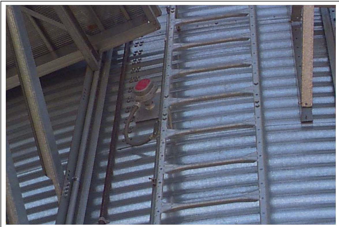
Figure 3N Storage Chamber Rotary Switch
