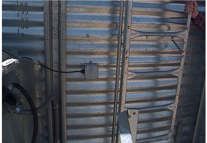
Plenum temperature sensor on the bin sidewall.
