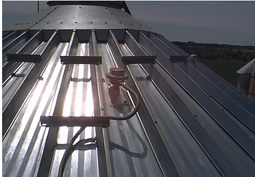
Drying chamber overflow rotary switch.
