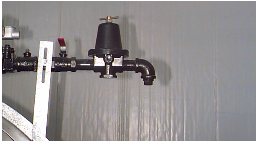
NG line field connection.
