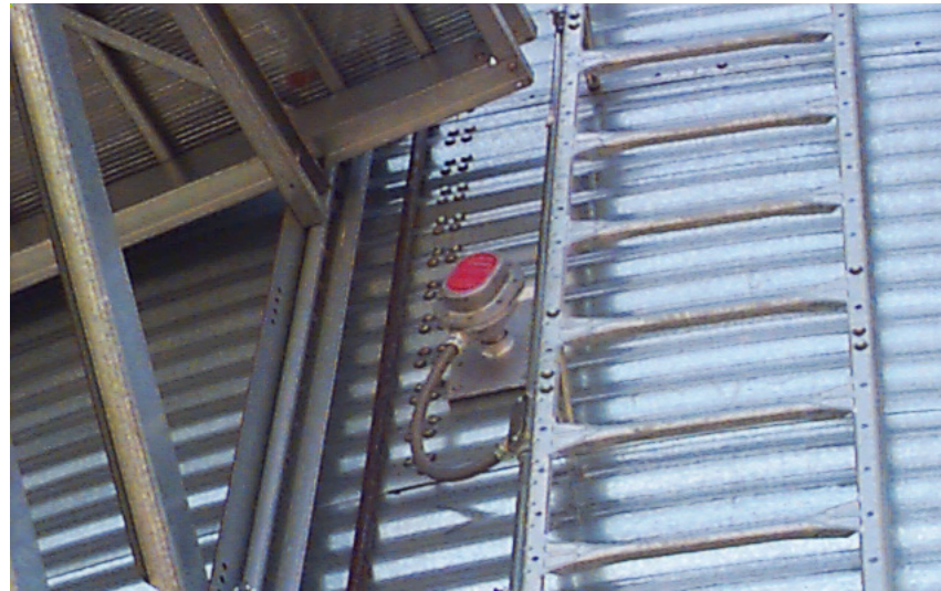
Storage chamber rotary switch.
