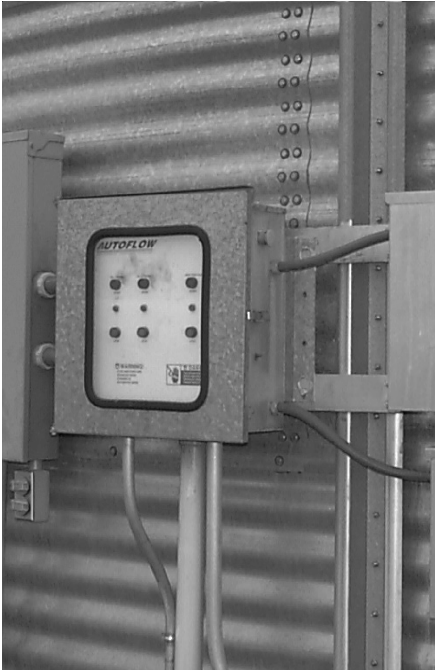
Fill System Control Box Mounted to Bin
