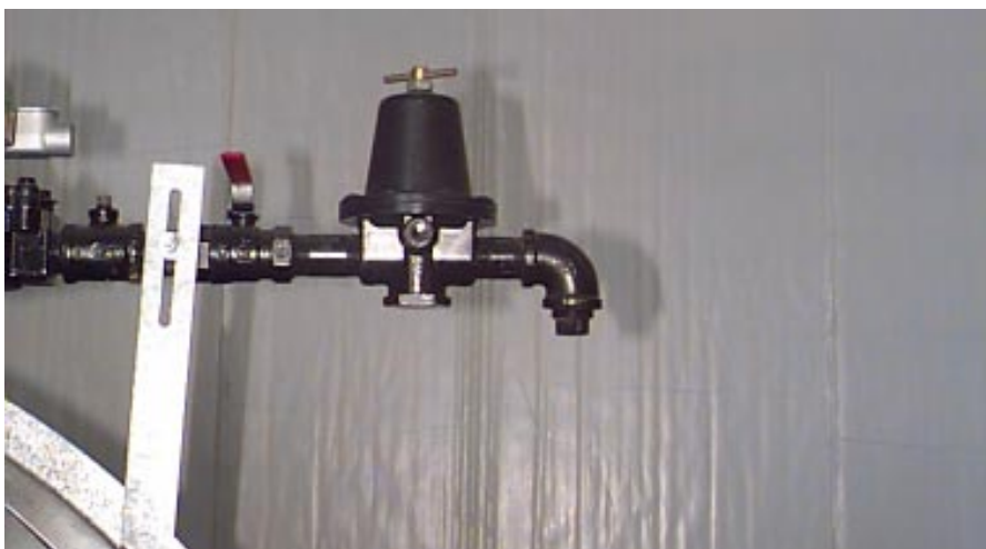
NG line field connection.
