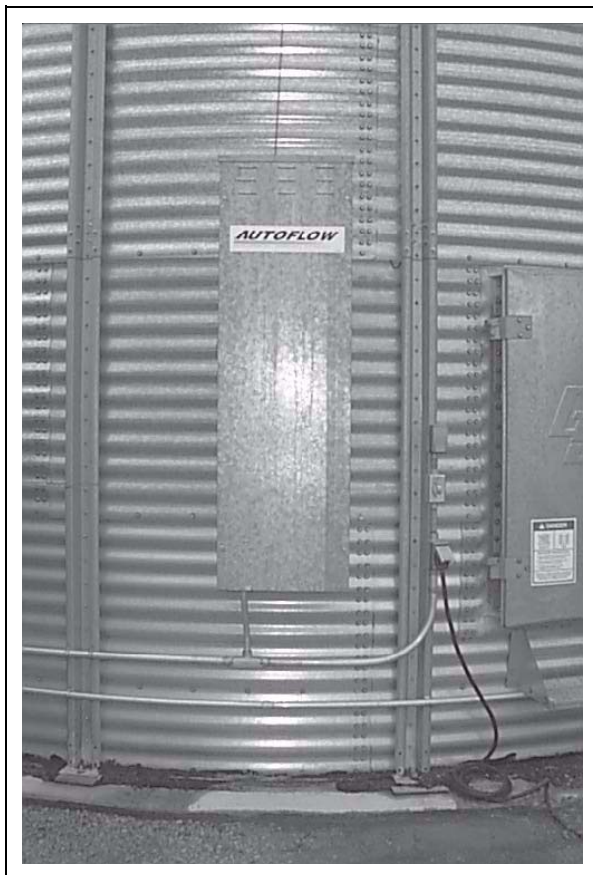
Figure 3F Old Actuator Control Box Mounted to Bin
