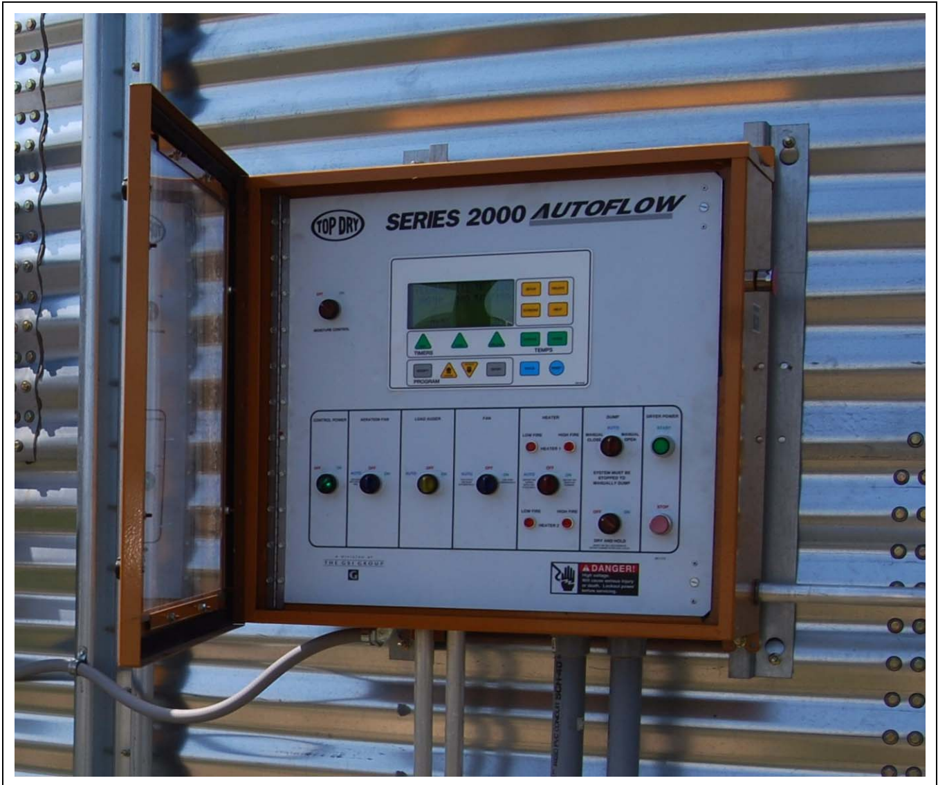
Figure 3A Autoflow Control Box Mounted on Bin
