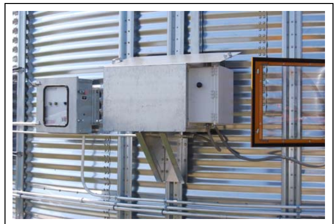
Figure 3G New Chute Controller
