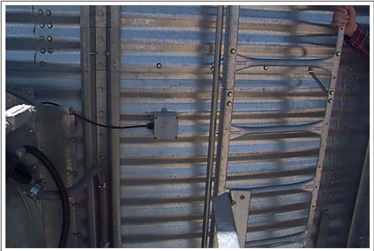
Figure 3K Plenum Temperature Sensor on the Bin Sidewall
