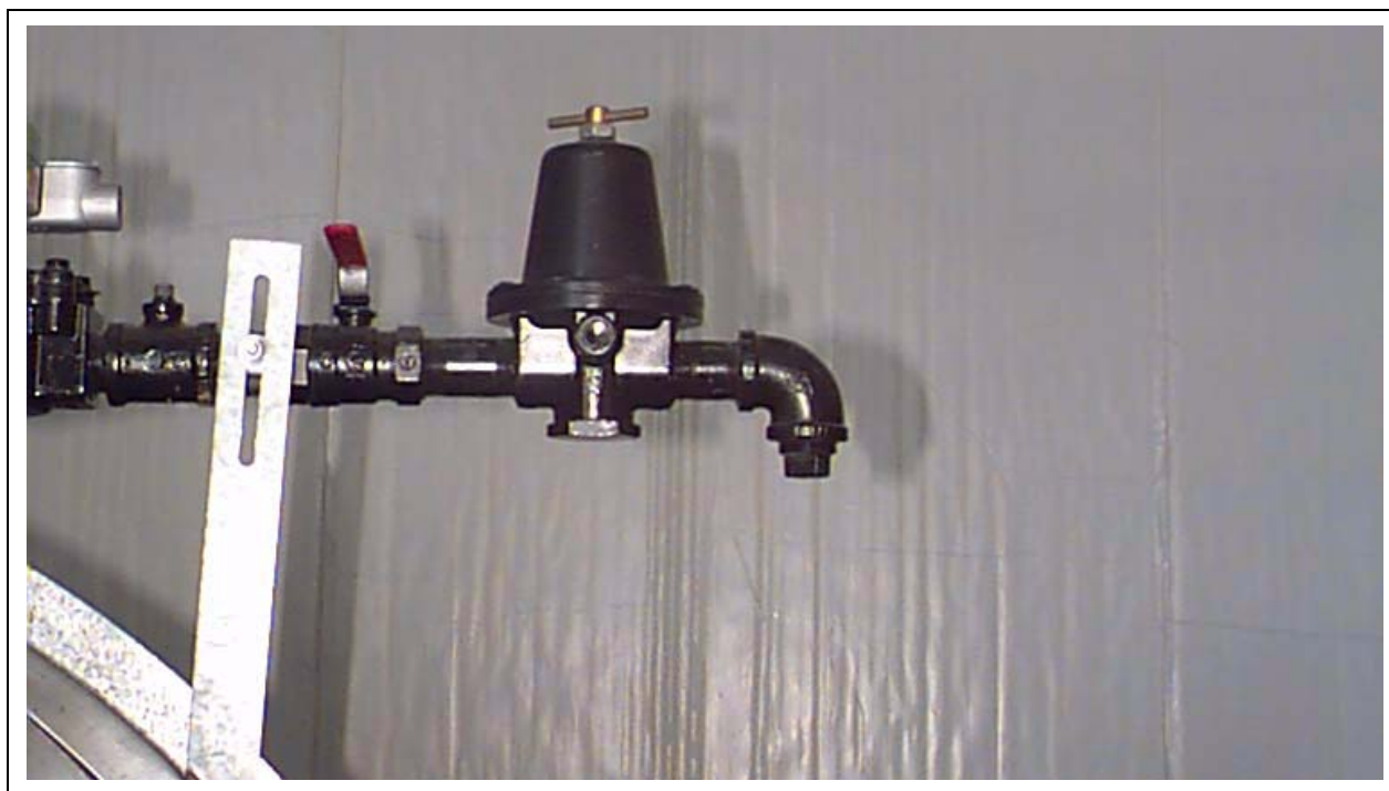
Figure 3W NG Line Field Connection
