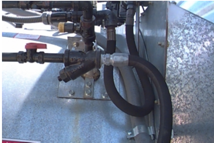
LP line field connection.
