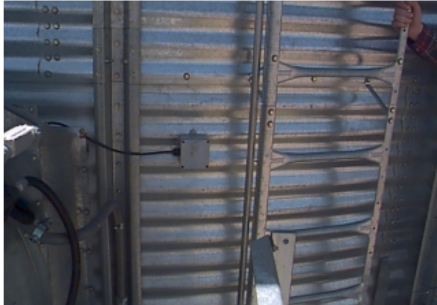
Plenum temperature sensor on the bin sidewall.
