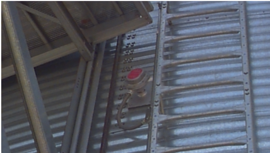
Storage chamber rotary switch.
