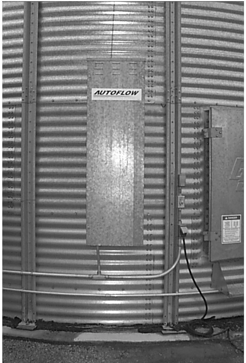
Actuator Control Box Mounted to Bin
