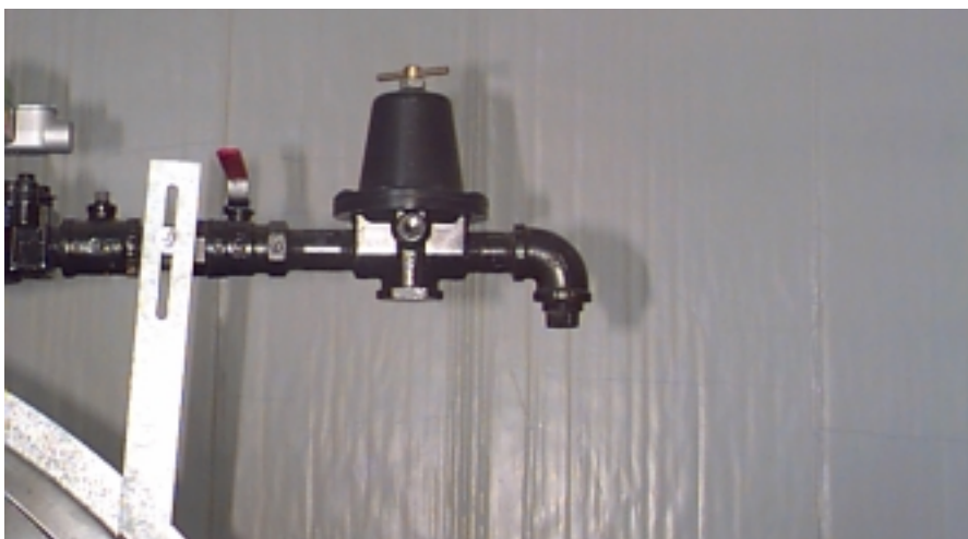
NG line field connection.
