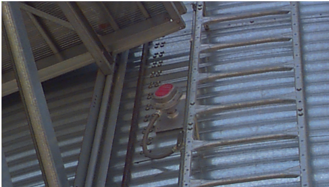
Storage chamber rotary switch.
