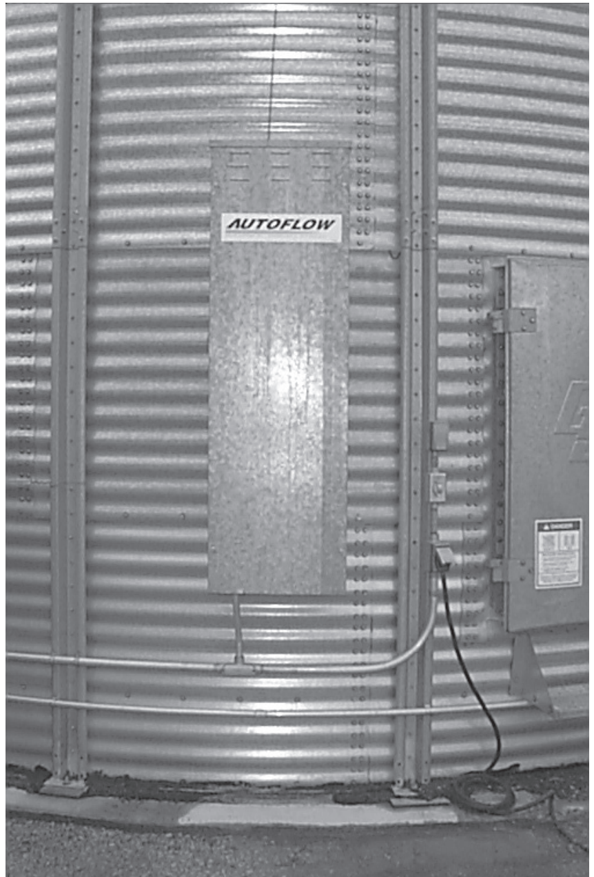
Actuator Control Box Mounted to Bin
