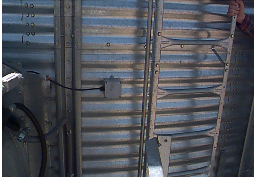
Plenum temperature sensor on the bin sidewall.
