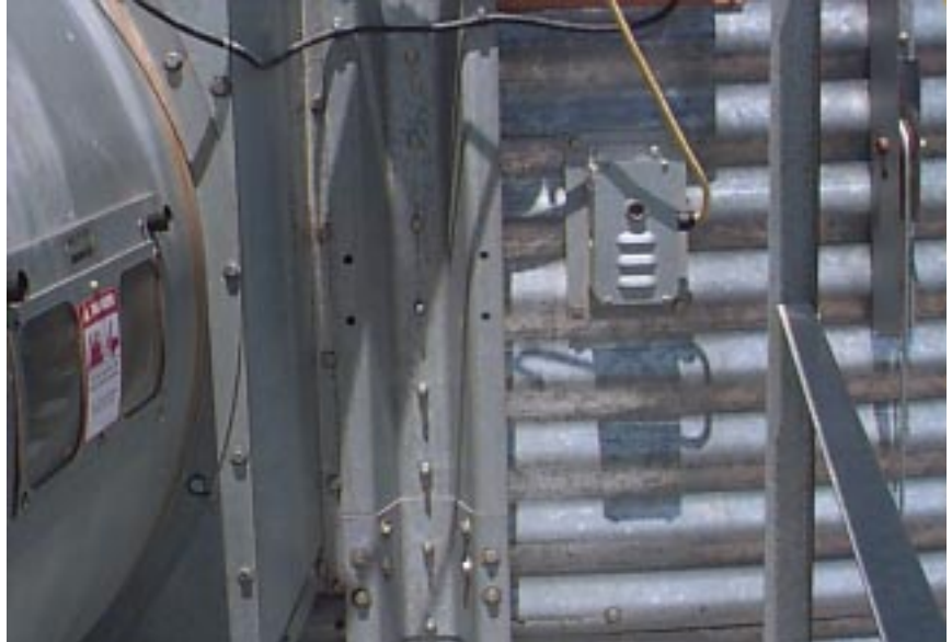
Airswitch mounted on the bin sidewall.
