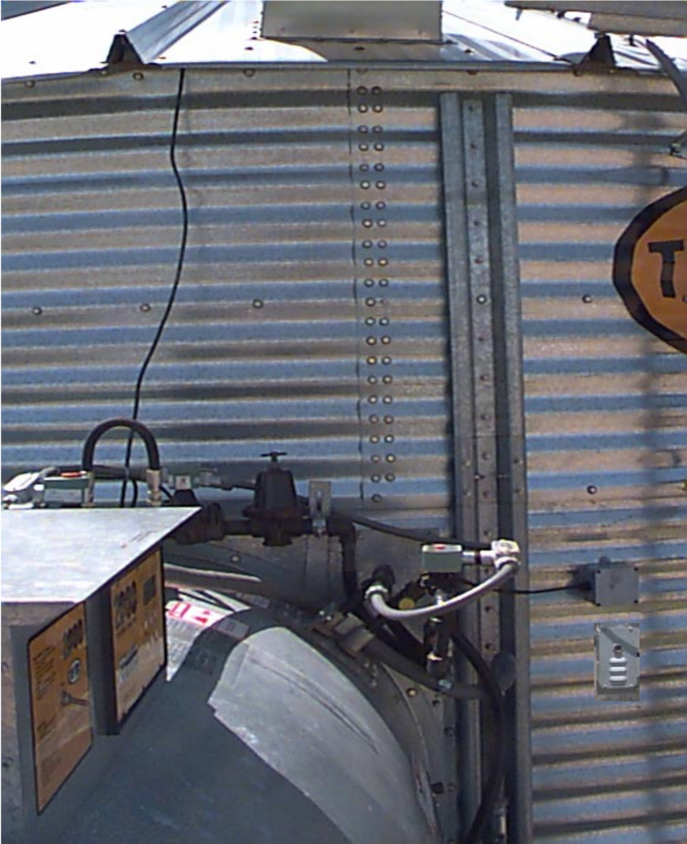
Fan/heater unit mounted to the bin, showing the plenum high limit, the airswitch, and cord going through the eave to the grain temperature sensor brackets.
