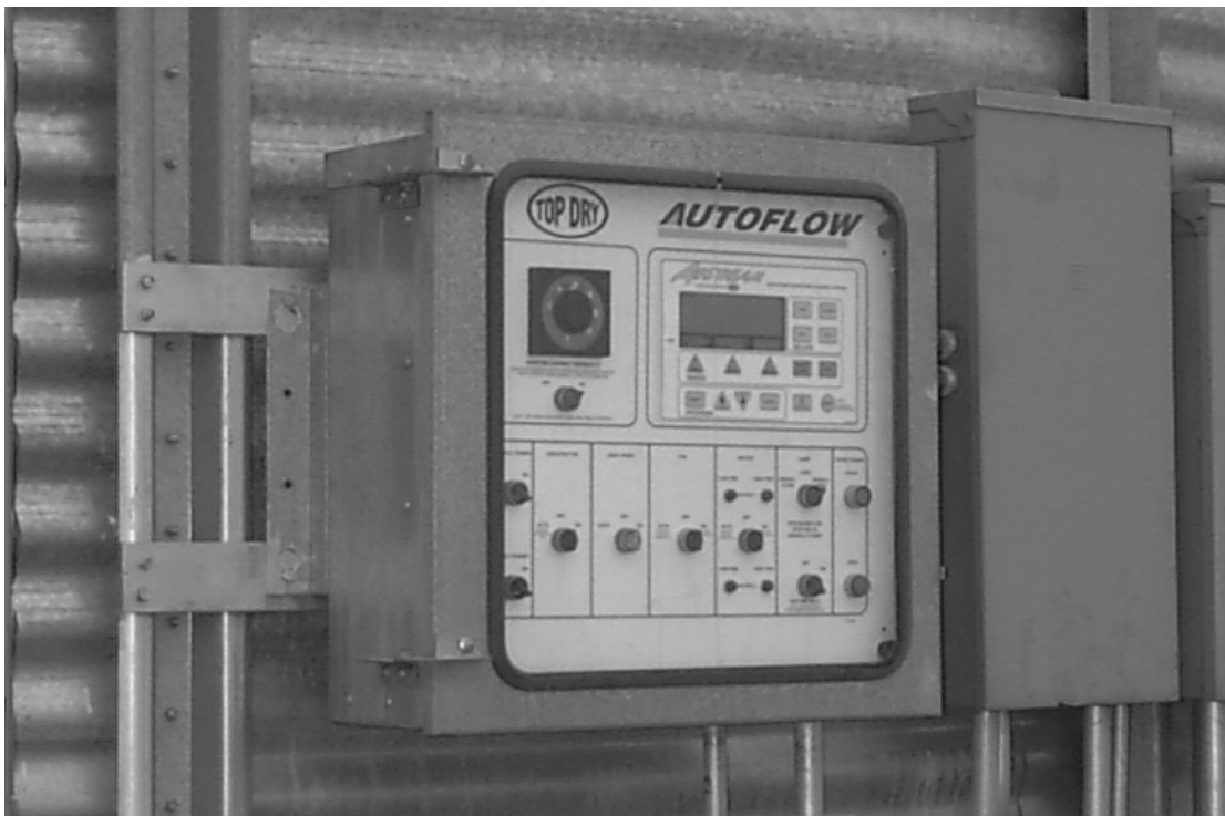
Autoflow Control box mounted on bin.
