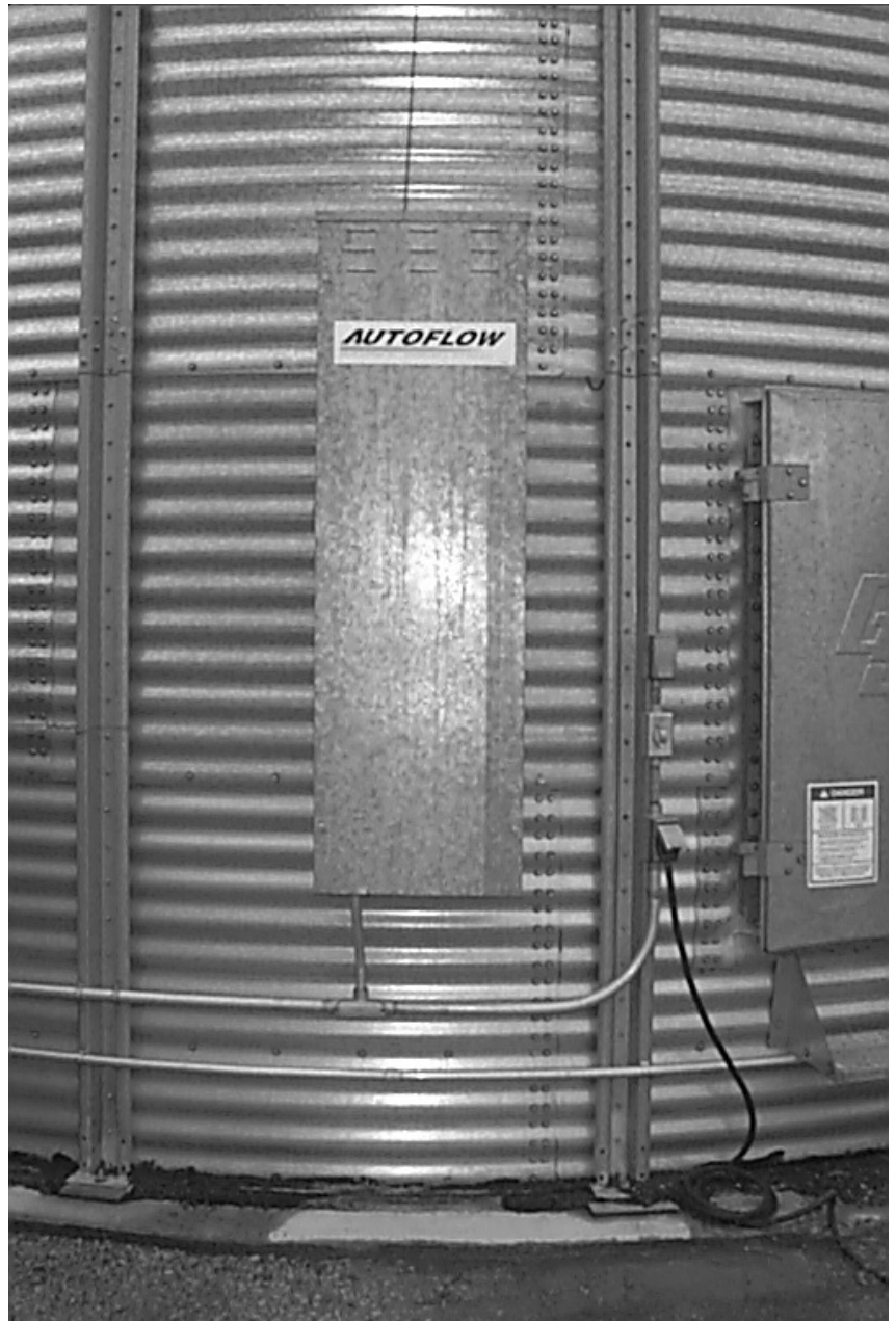
Actuator Control Box Mounted to Bin
