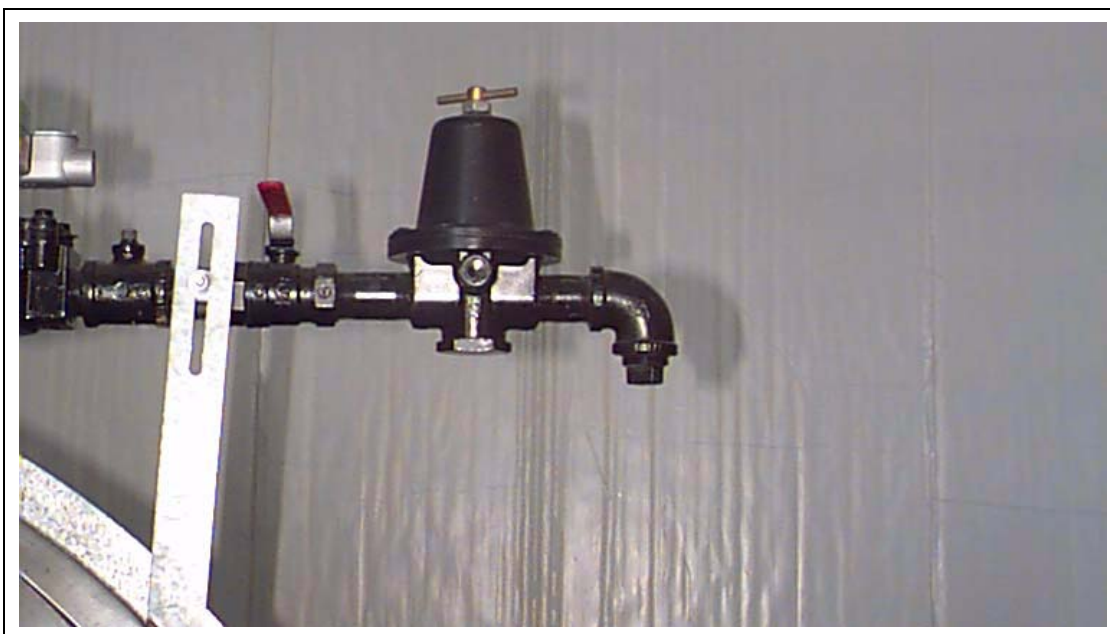
Figure 3Y NG Line Field Connection
