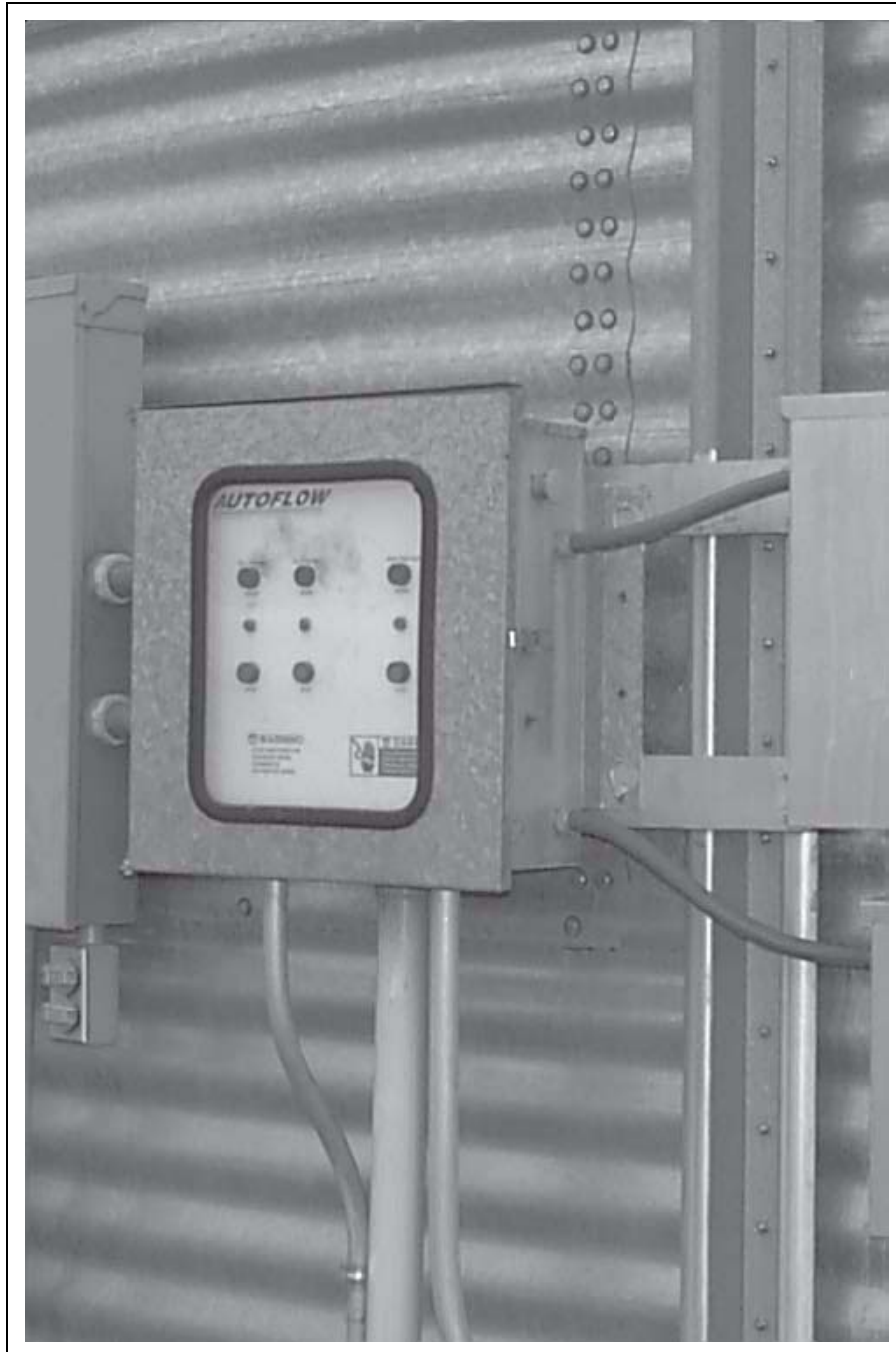
Figure 3D Fill System Control Box Mounted to Bin
