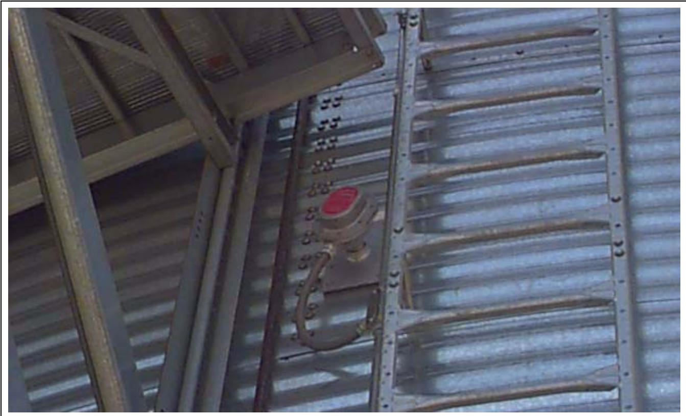
Figure 3Q Storage Chamber Rotary Switch
