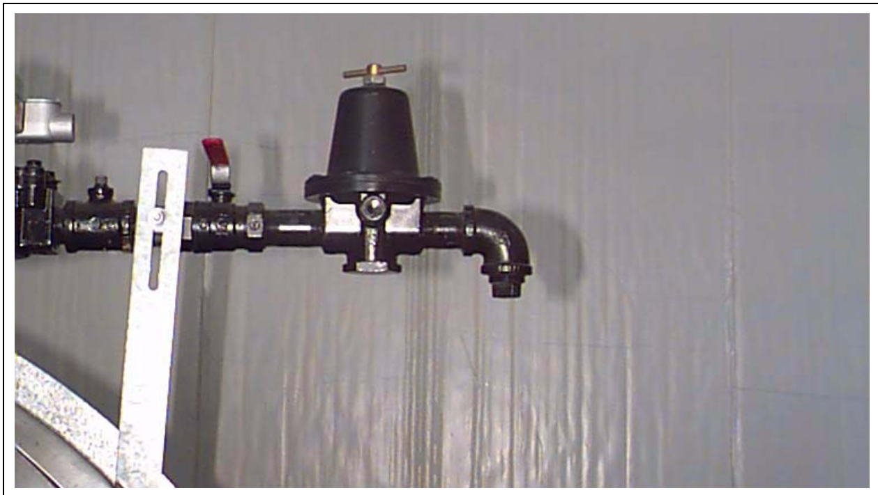
Figure 3Y NG Line Field Connection
