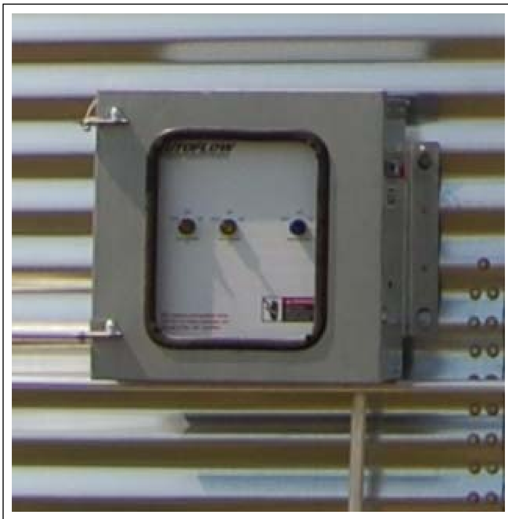
Figure 3D Fill System Control Box Mounted to Bin
