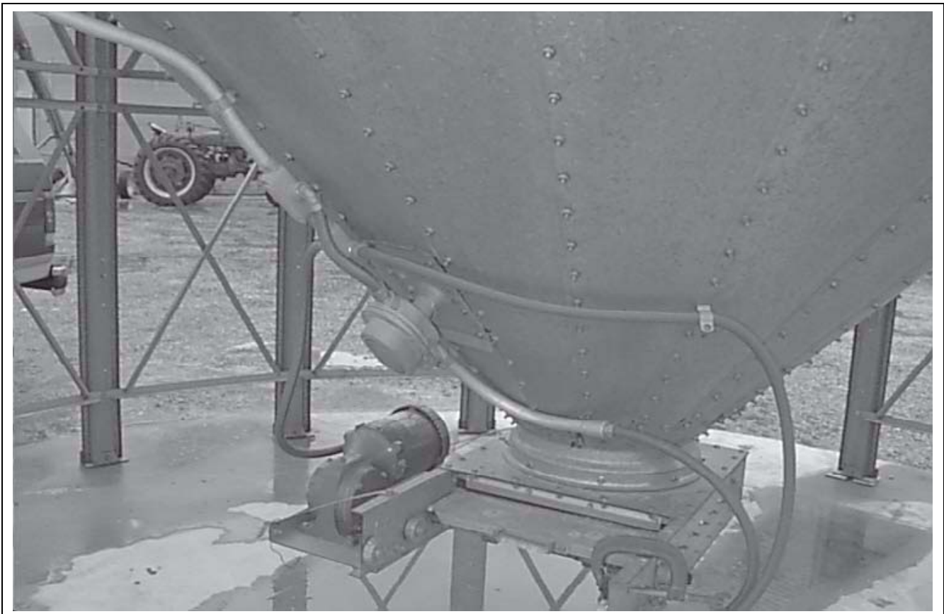
Figure 3N Wet Supply Rotary Switch Mounted on Wet Supply Tank
