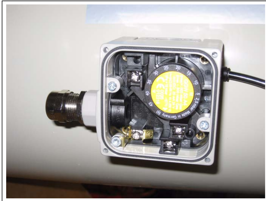
Figure 3A Pressure Switch Setting Dial
