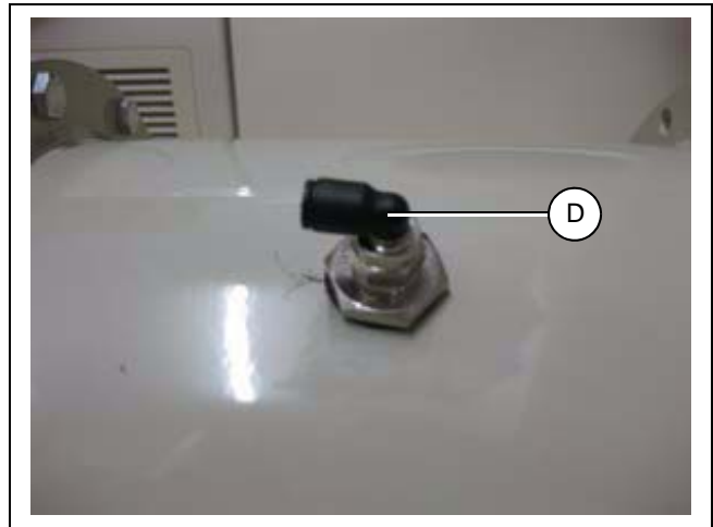
Figure 2G Tapping on Small Duct
