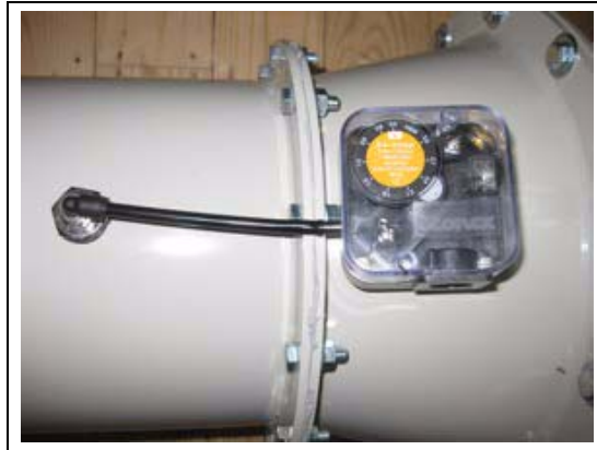
Figure 2E Pressure Switch
