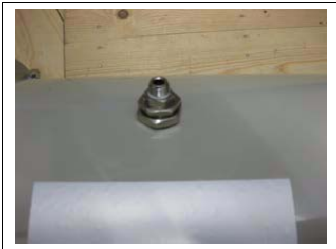
Figure 2F Tapping on Large Duct
