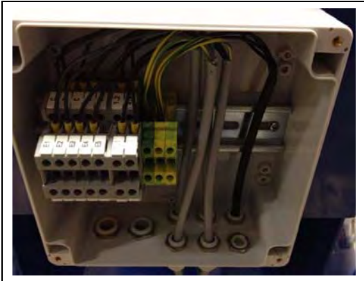
Figure 12B Junction Box with Marked Terminals
