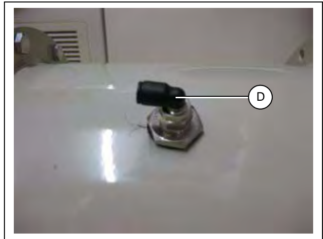
Figure 2G Tapping on Small Duct
