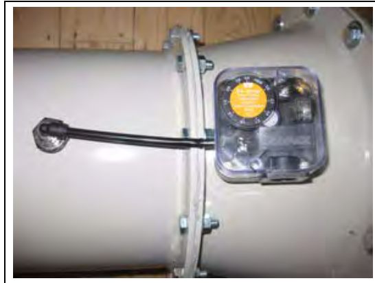
Figure 2E Pressure Switch
