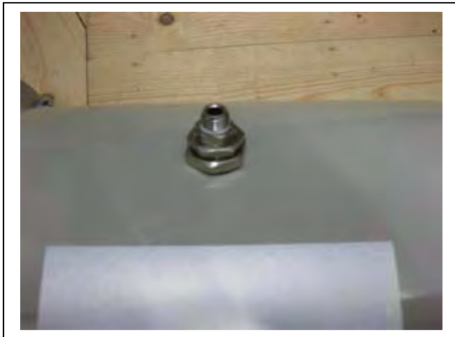
Figure 2F Tapping on Large Duct
