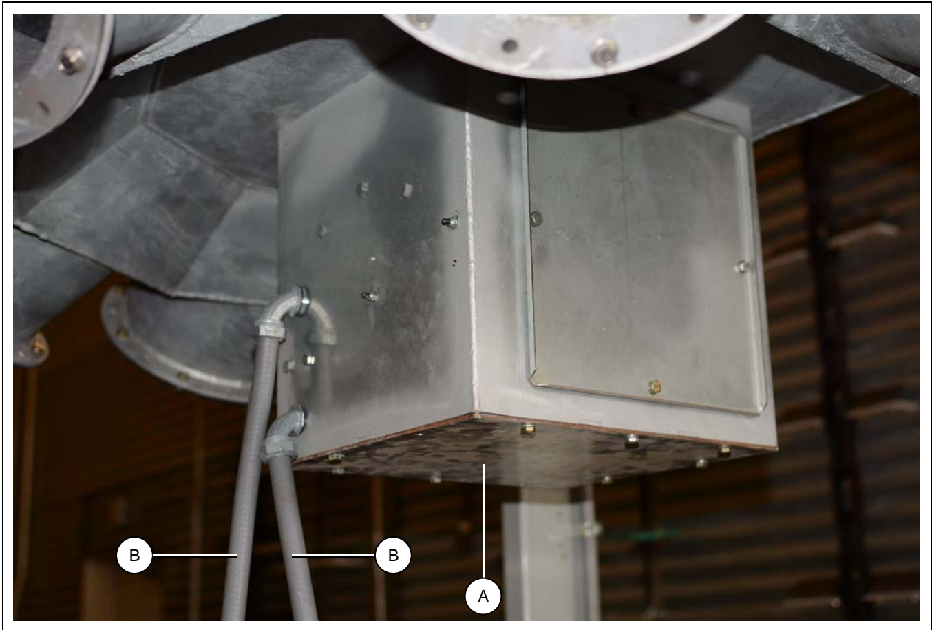
Figure 3B Cable Fitting Connections to Distributor Enclosure
