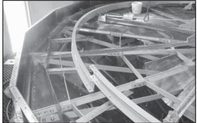
9-E. Drive Channel Halves During Installation.
