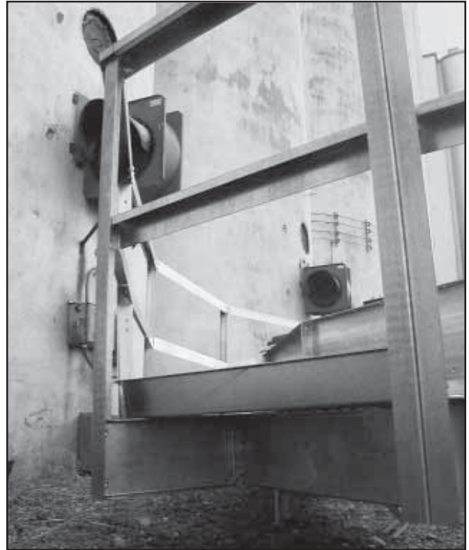
8-D. Platform Support Channels. RMS 15K Shown.
