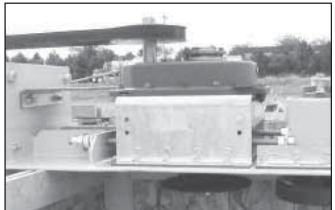
11-E. Drive shaft and sprocket installed.
