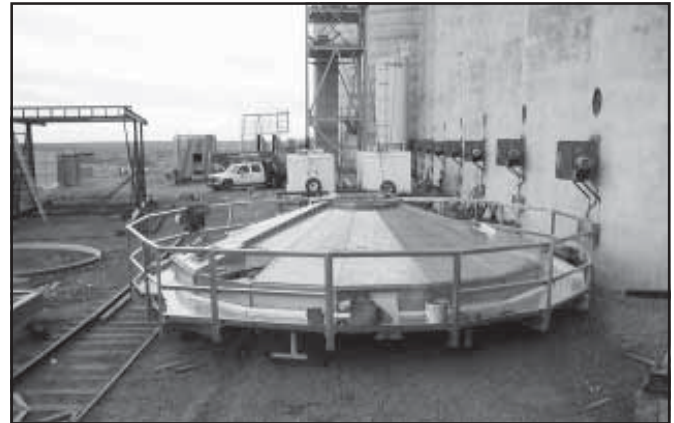
8-A. Platform during assembly. 50 KSS Shown.
