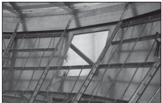
4-C. Installed Screen Frames on 50 K Scalper/Screeners.
