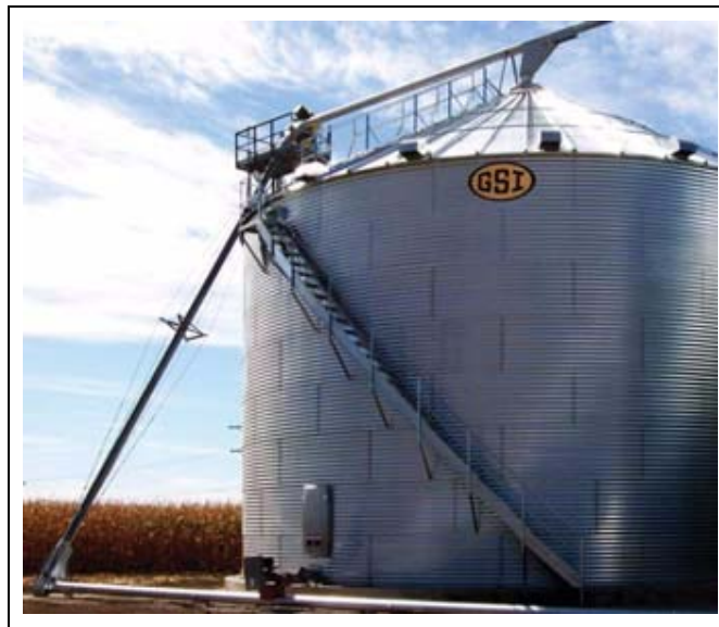
Figure 4B Angle Installation
