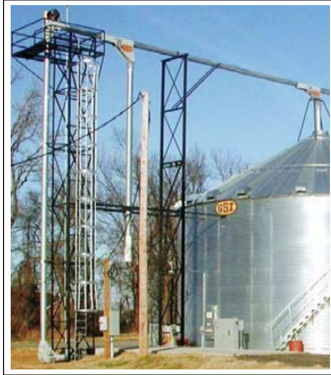
Figure 4A Vertical Installation
