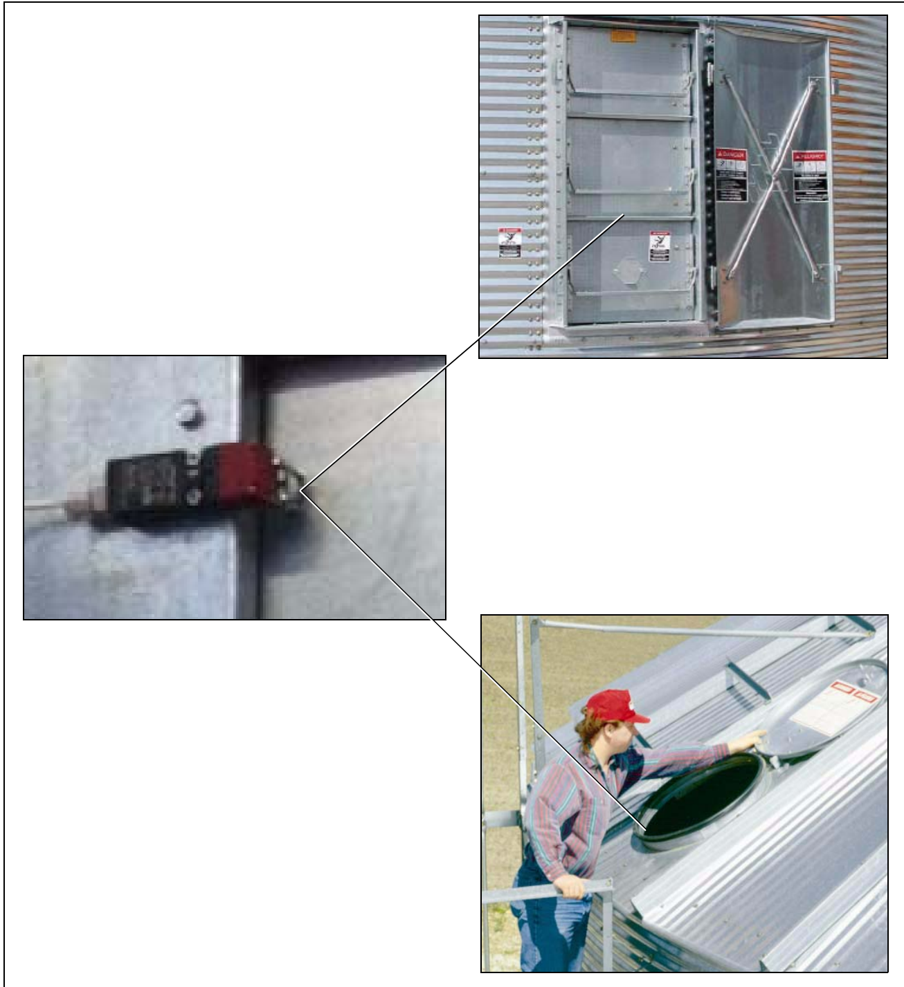
Figure 1B Door Interlock Locations
