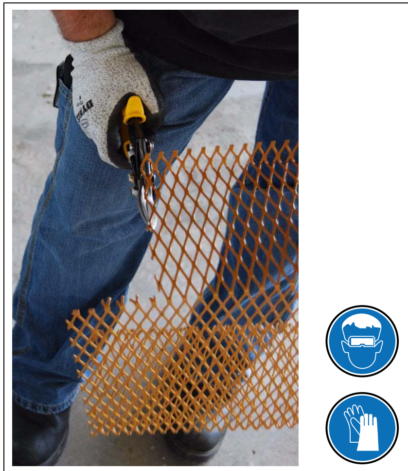
Figure 3AE Cut First Guard to Size
